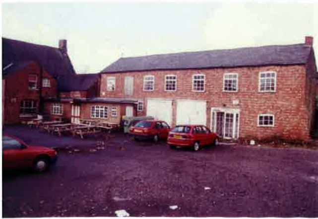
Plate 7: General view of pub from north-east
