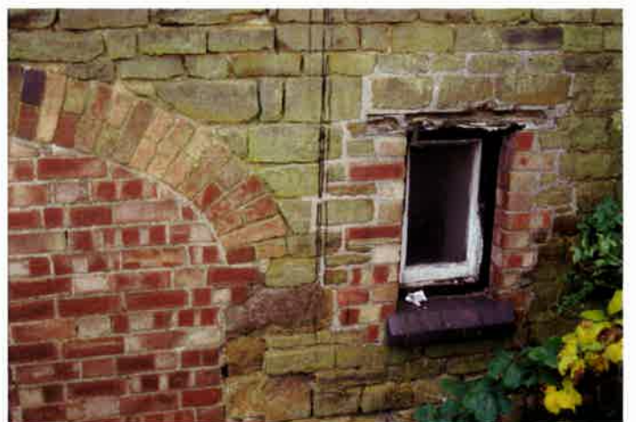
Plate 6: Inserted window and edge of former arched opening
