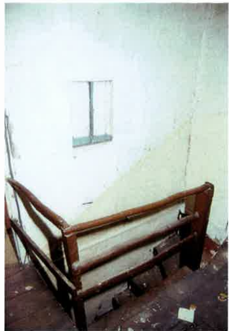
Plate 16: Stairs at second floor level and internal window to S2
