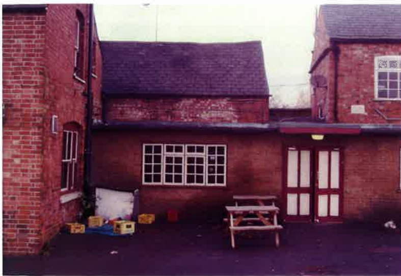
Plate 9: Junction between four secondary extensions
