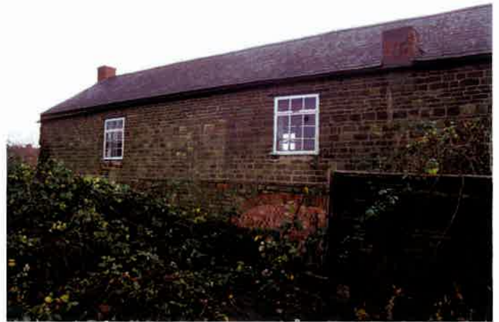
Plate 4: Rear (west) face of former stable block
