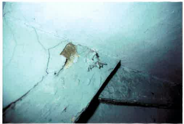
Plate 14: Detail of forelock bolt in truss between S1 and S2
