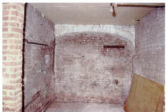
Plate 12: Internal view of blocked arch in former stables
