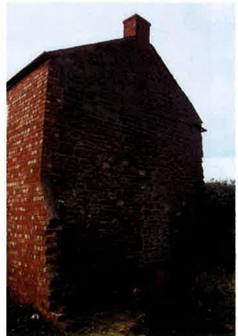
Plate 10: North wall of rebuilt former stables
