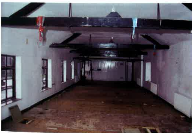
Plate 11: Interior of first floor of Phase IV building
