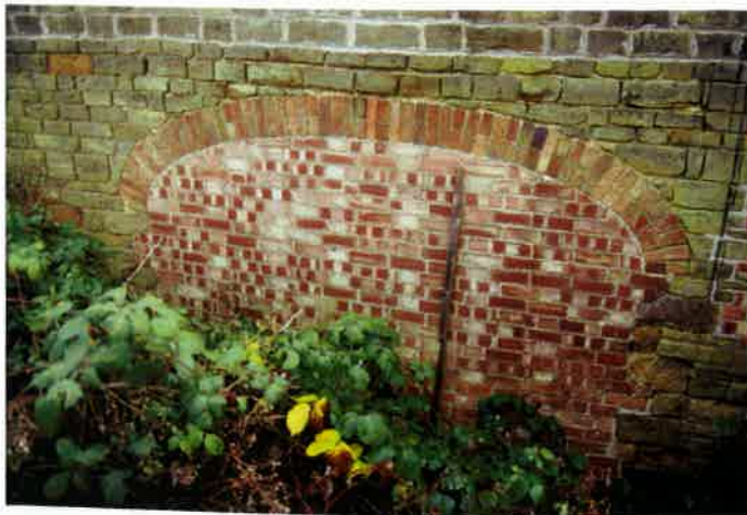
Plate 5: Blocked arched opening in rear of former stable block
