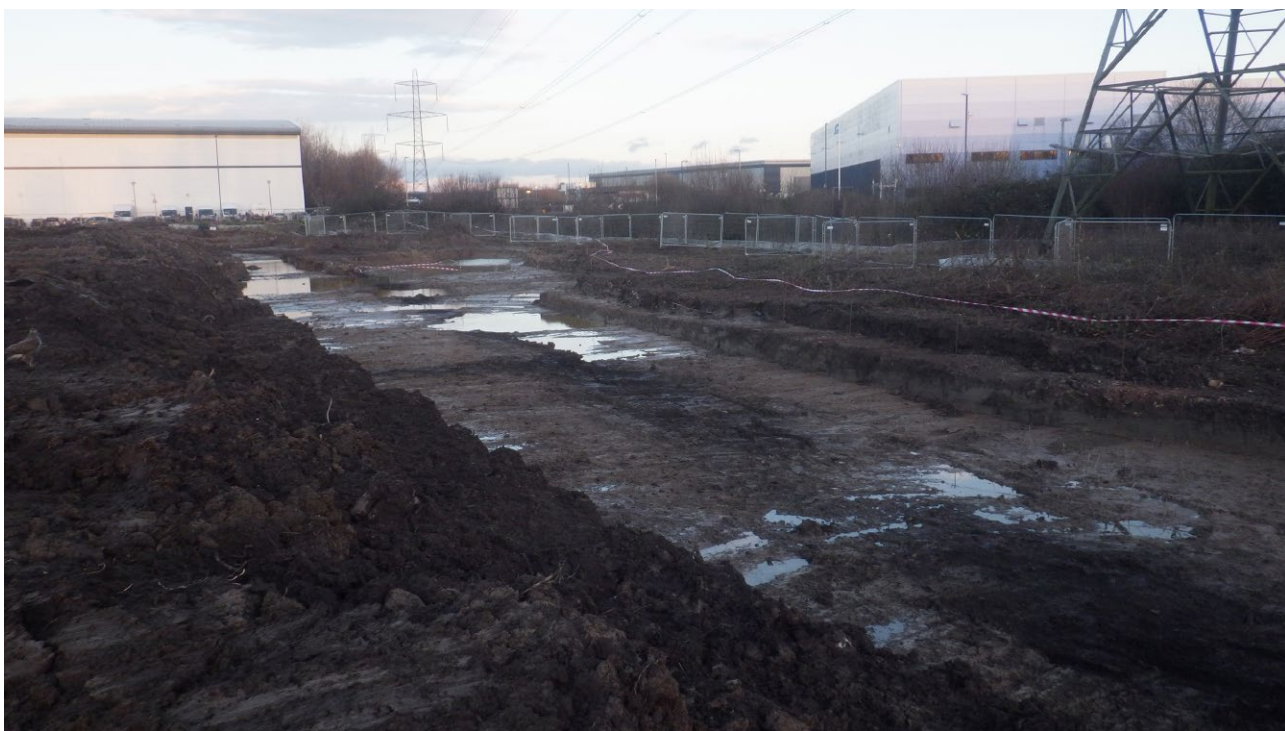
Plate 2: General view of site, looking E
