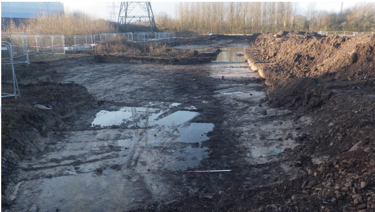
Plate 1: General view of site, looking SW
