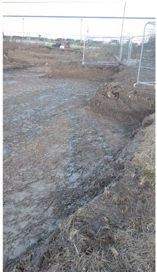
Plate 4: Ditches 5 and 7, looking N
