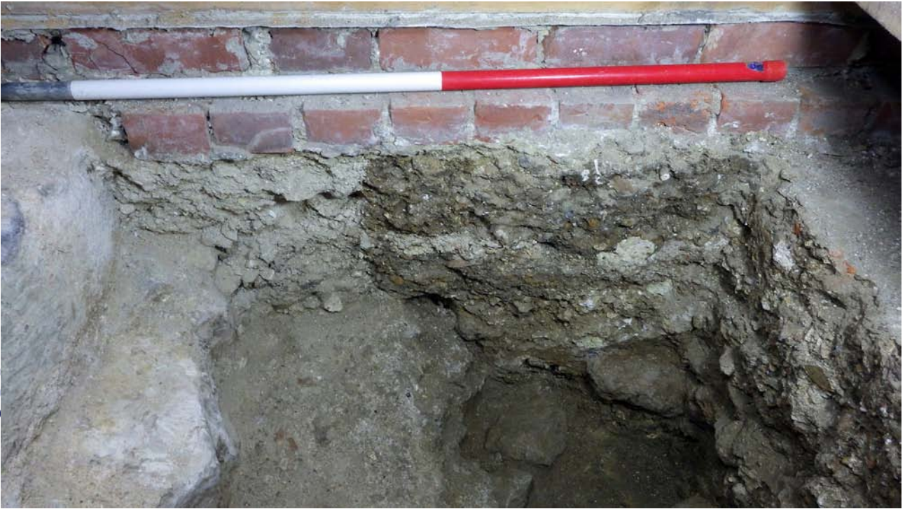
Plate 1: East facing section of test pit 3 showing foundations 303 and 300
