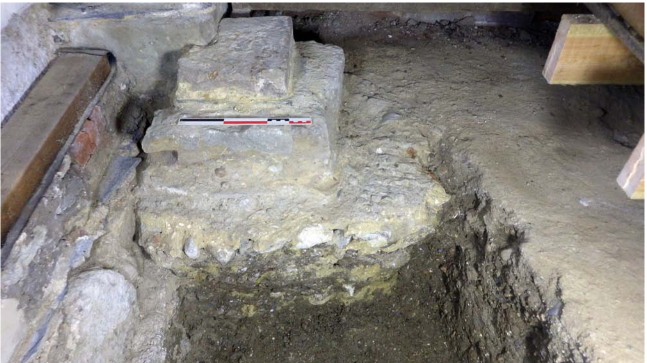
Plate 2: West facing section of test pit 5, showing foundations 501 and 504
