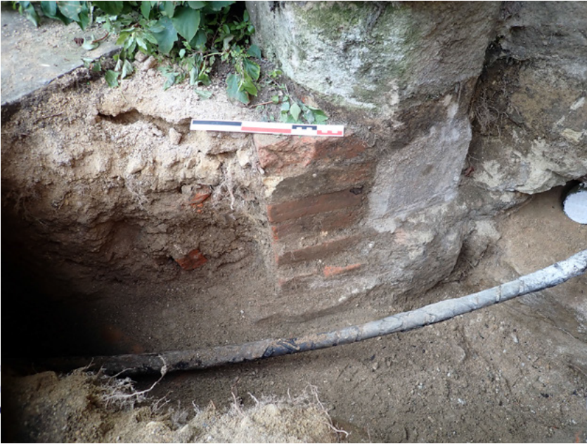
Plate 1: Trench 2, showing foundation wall 205, looking south
