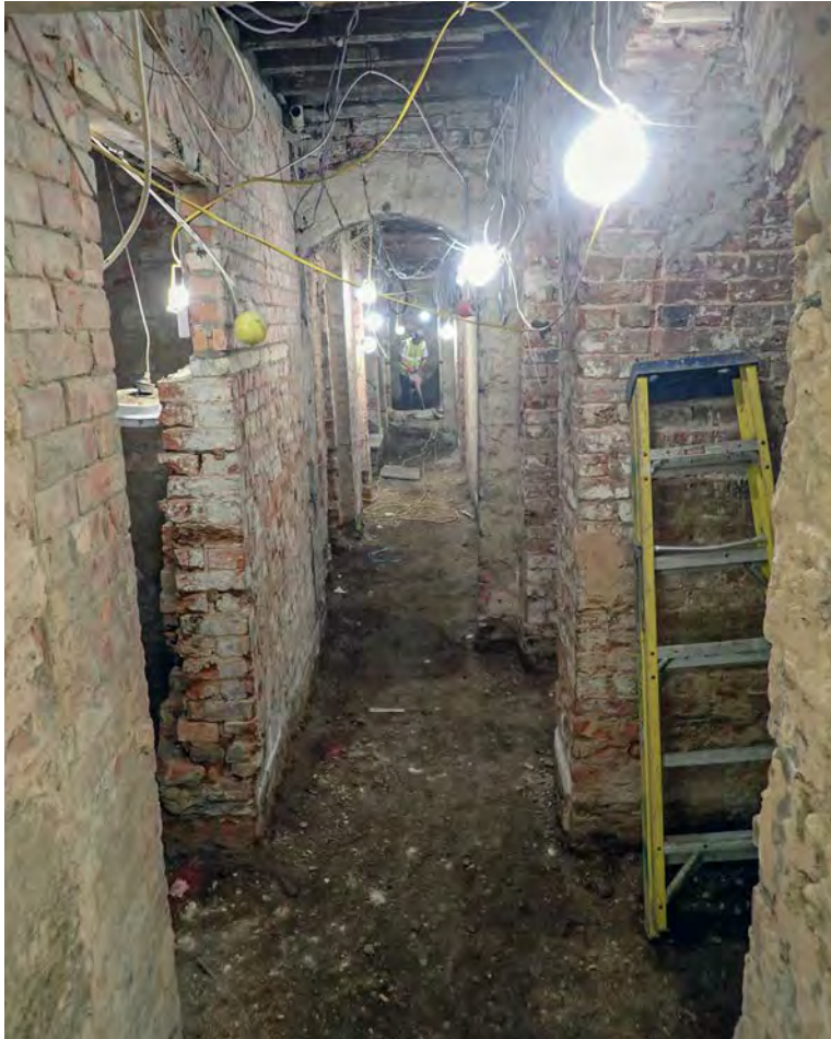
Plate 1: General View of works along central corridor
