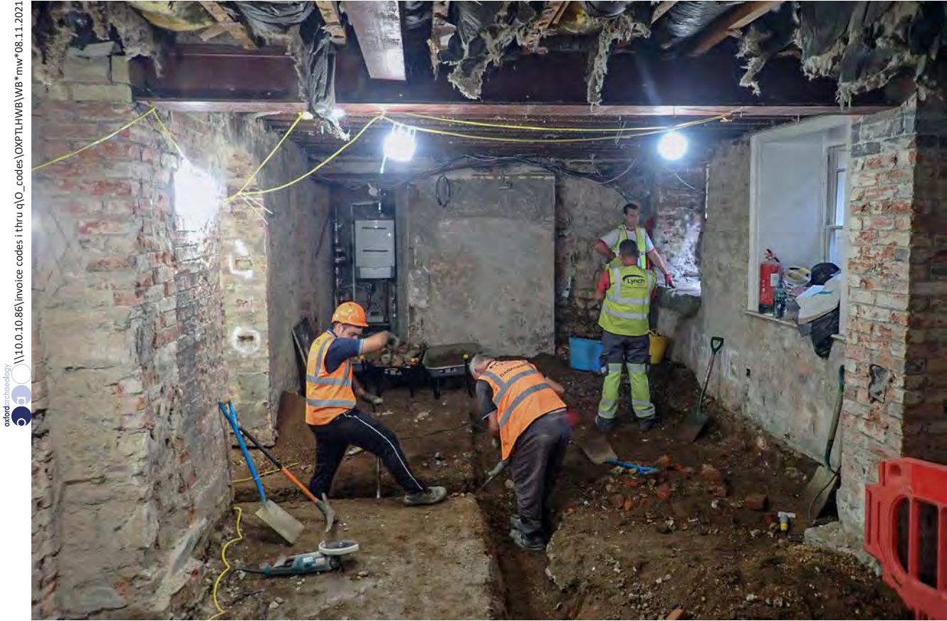
Plate 5: General View of Works
