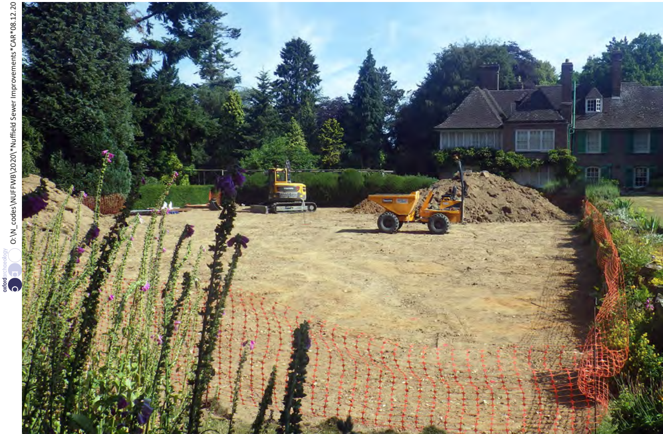
Plate 1: General view of works
