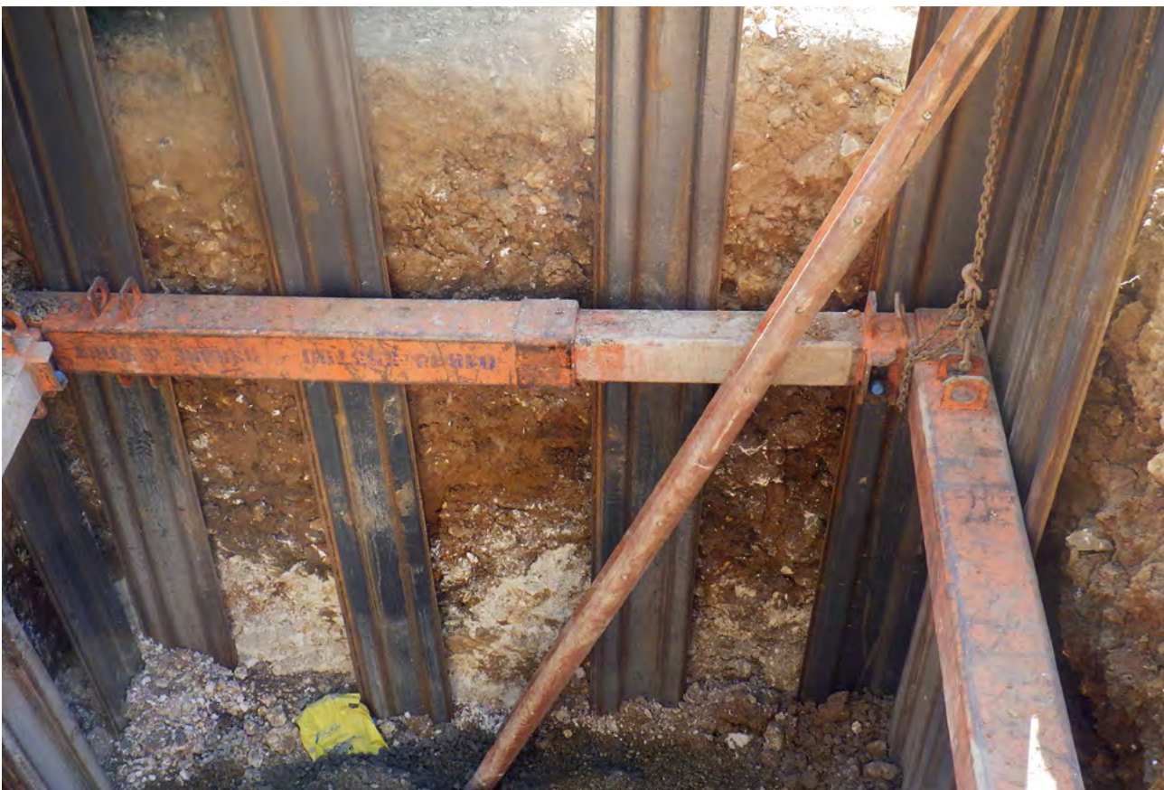
Plate 2: Trench 1, view to N
