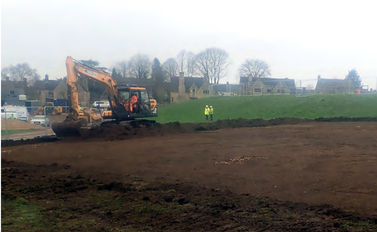
Plate 4: Working shot: stripping topsoil, view to NW
