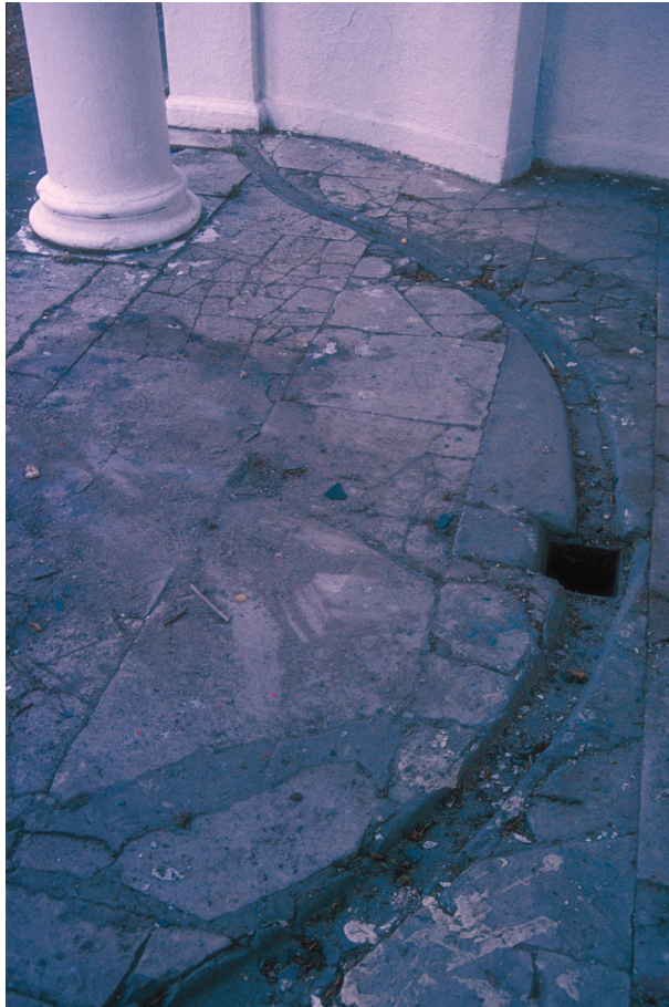
Plate 5: Drainage channel and sump on south elevation of Temple, looking west
