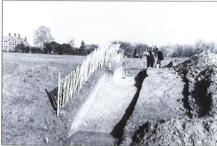
Plate 2: The DOE excavation
