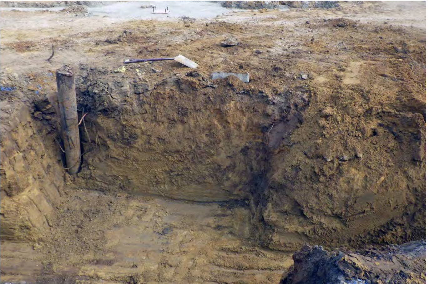
Plate 5: Section of ground beam trench
