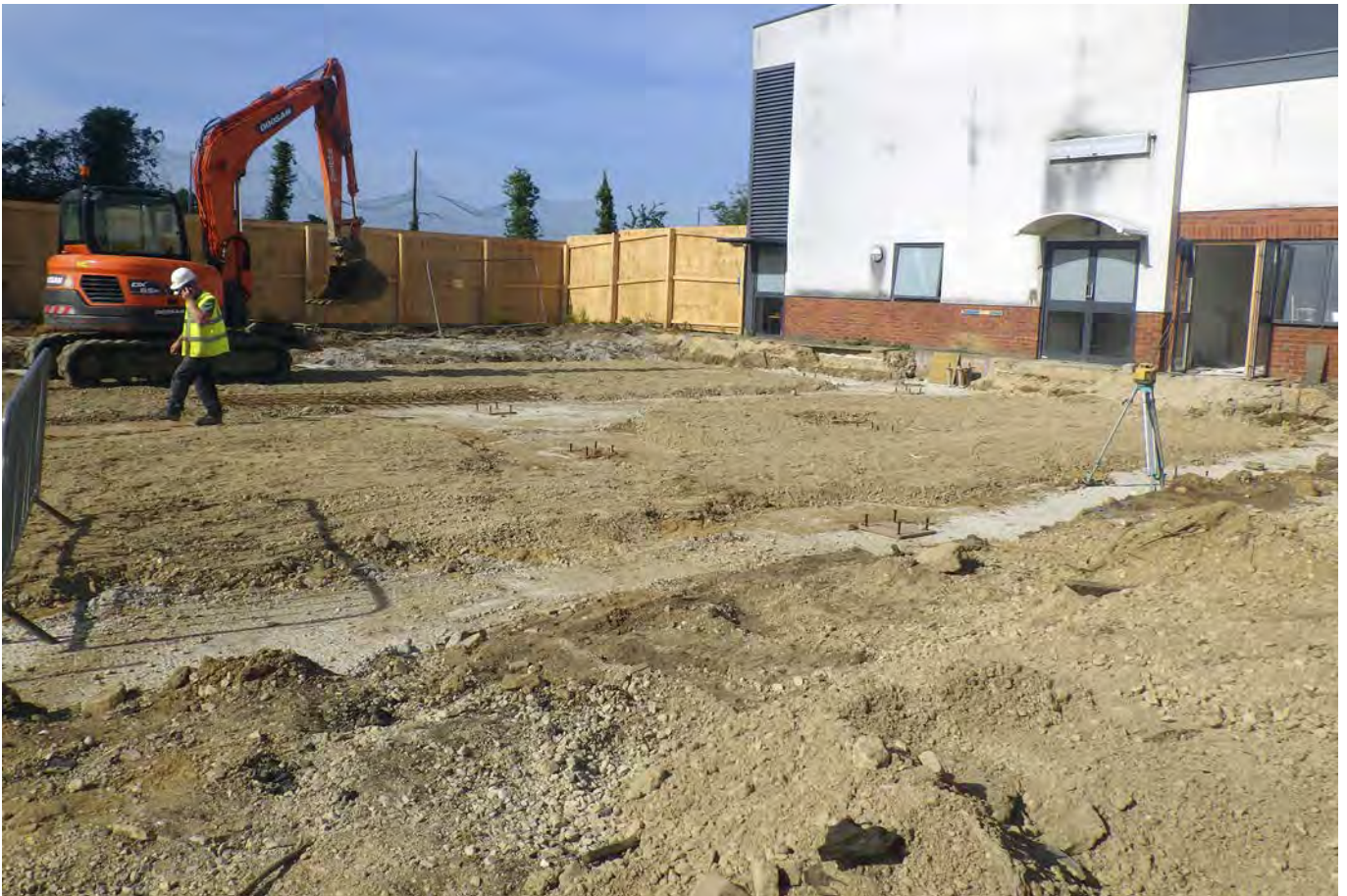
Plate 11: Foundation trenches filled in with concrete
