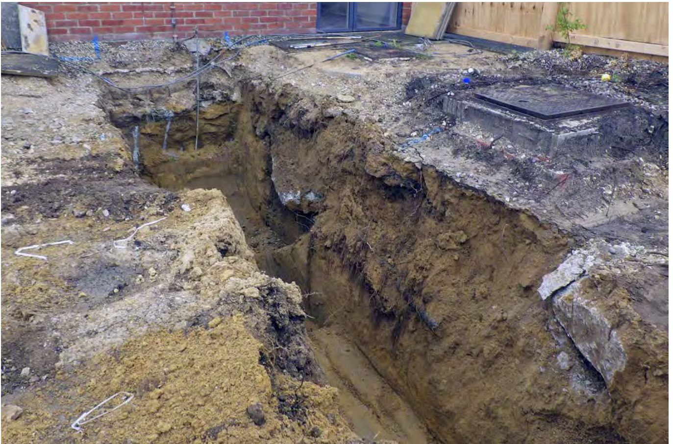
Plate 2: Section of ground beam trench showing modern disturbance
