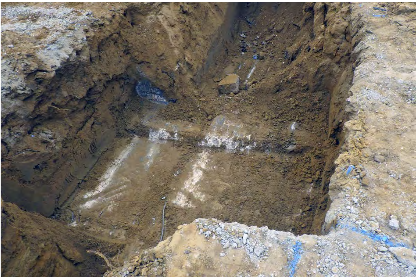
Plate 10: One of the concrete chambers encountered on site
