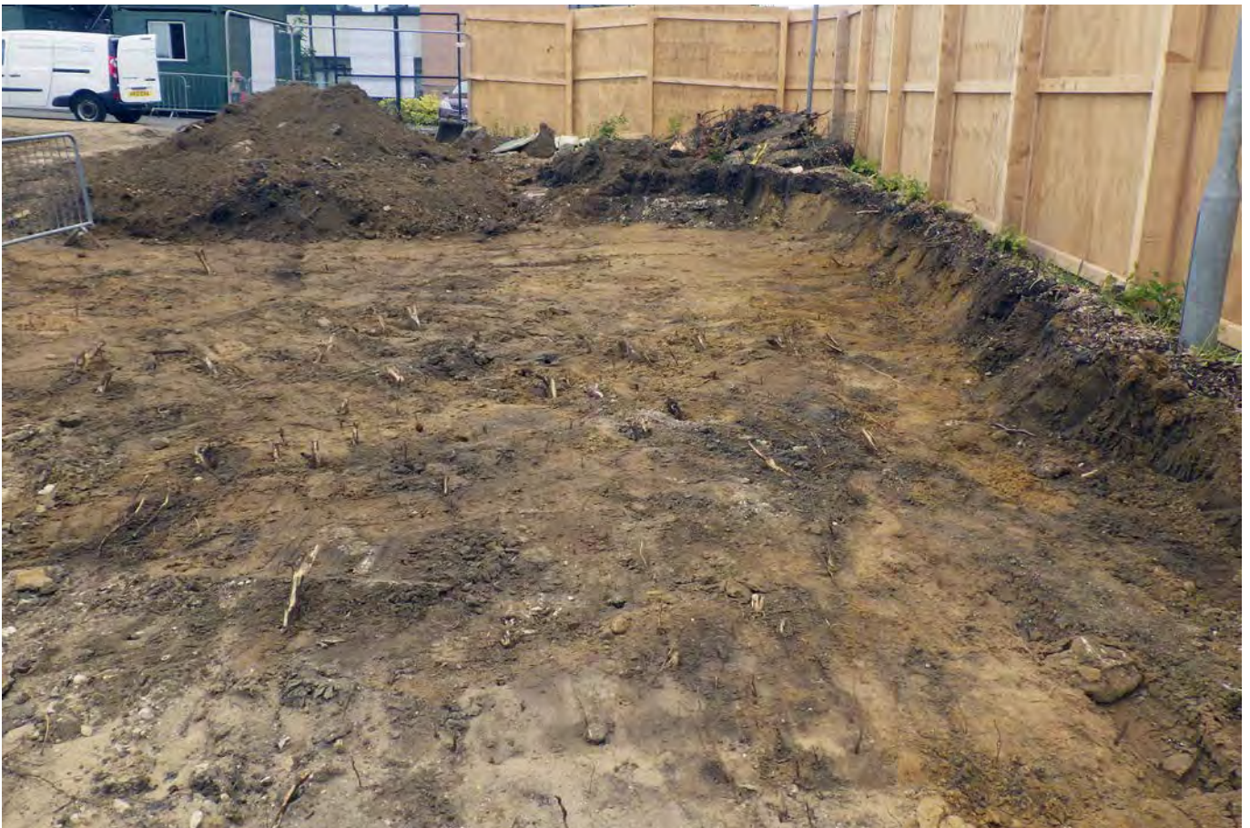
Plate 4: Evidence of ground disturbance after initial machine strip
