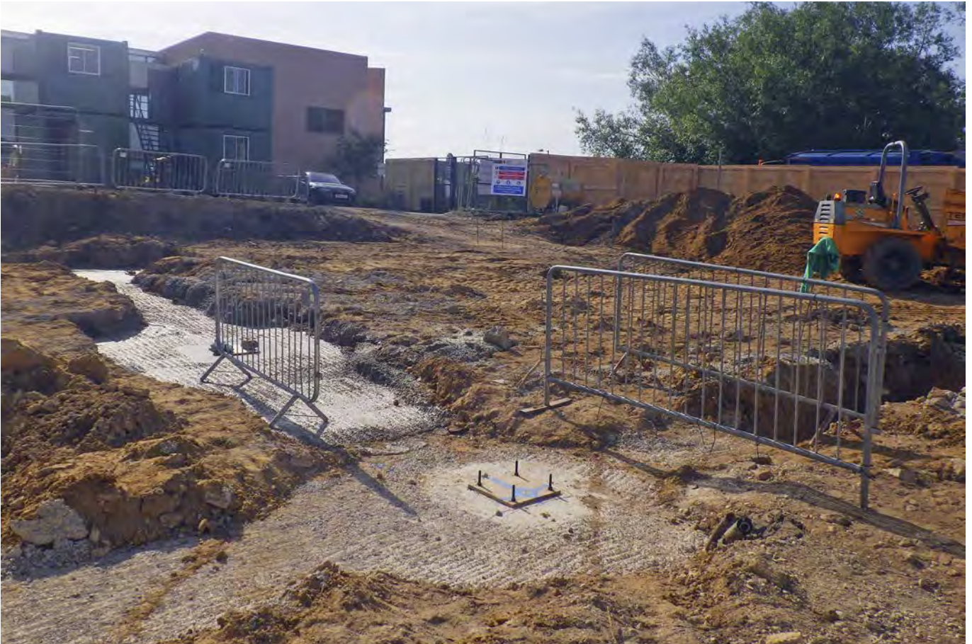
Plate 13: View of infilled ground beam trenches
