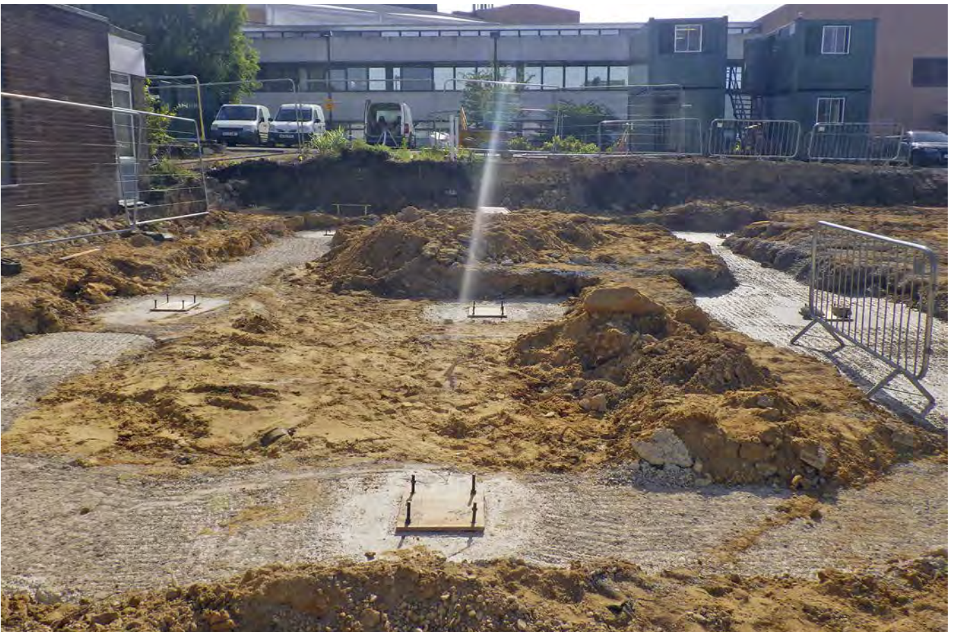
Plate 14: Infilled ground beam trenches in the eastern part of site
