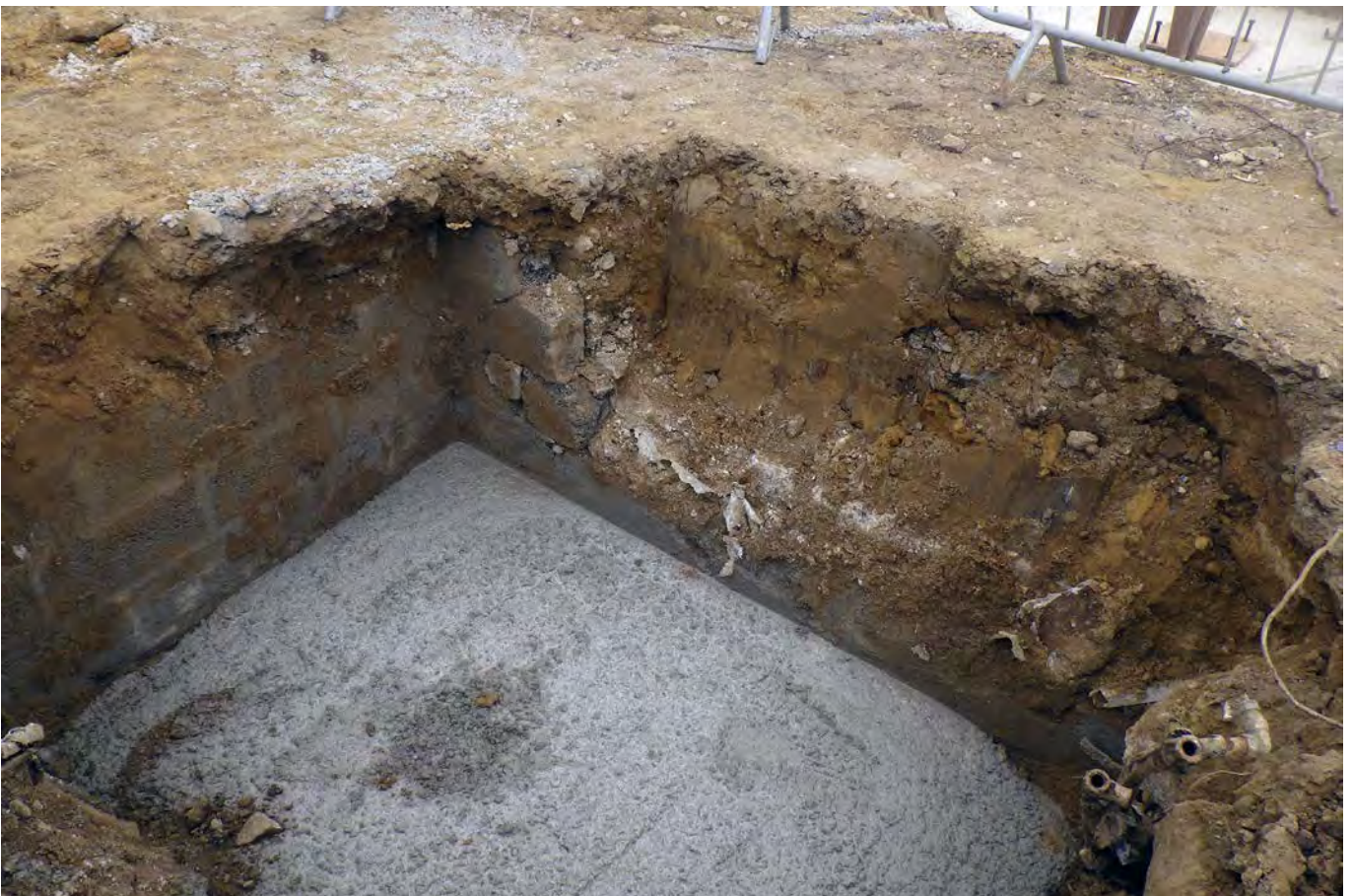
Plate 6: Modern concrete truncations within pad 2
