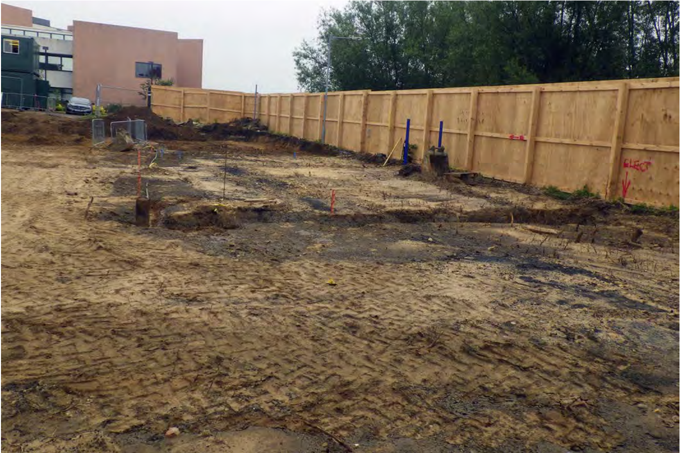
Plate 3: Eastern area after initial machine strip
