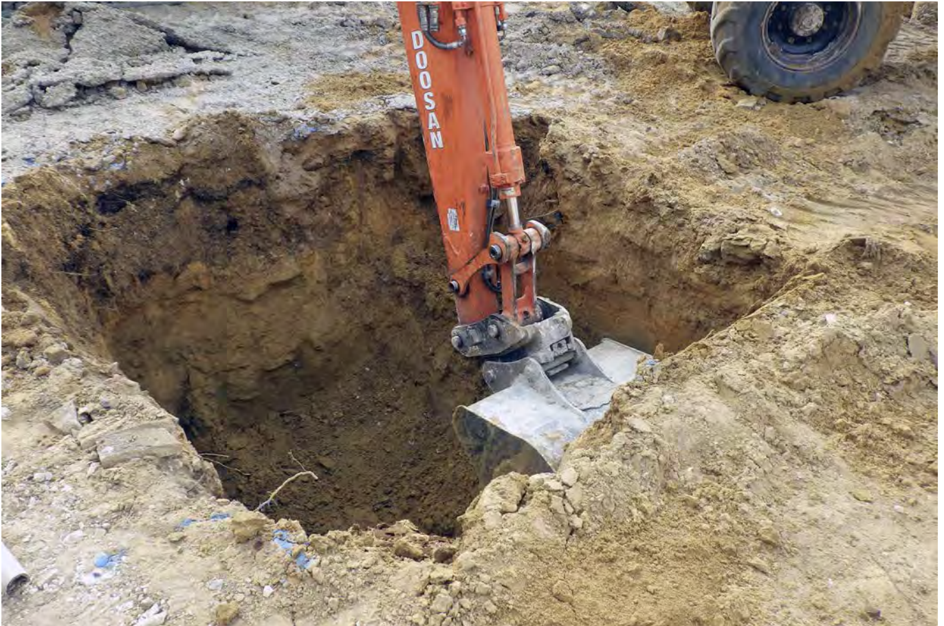
Plate 9: Pad 3, showing made ground and natural
