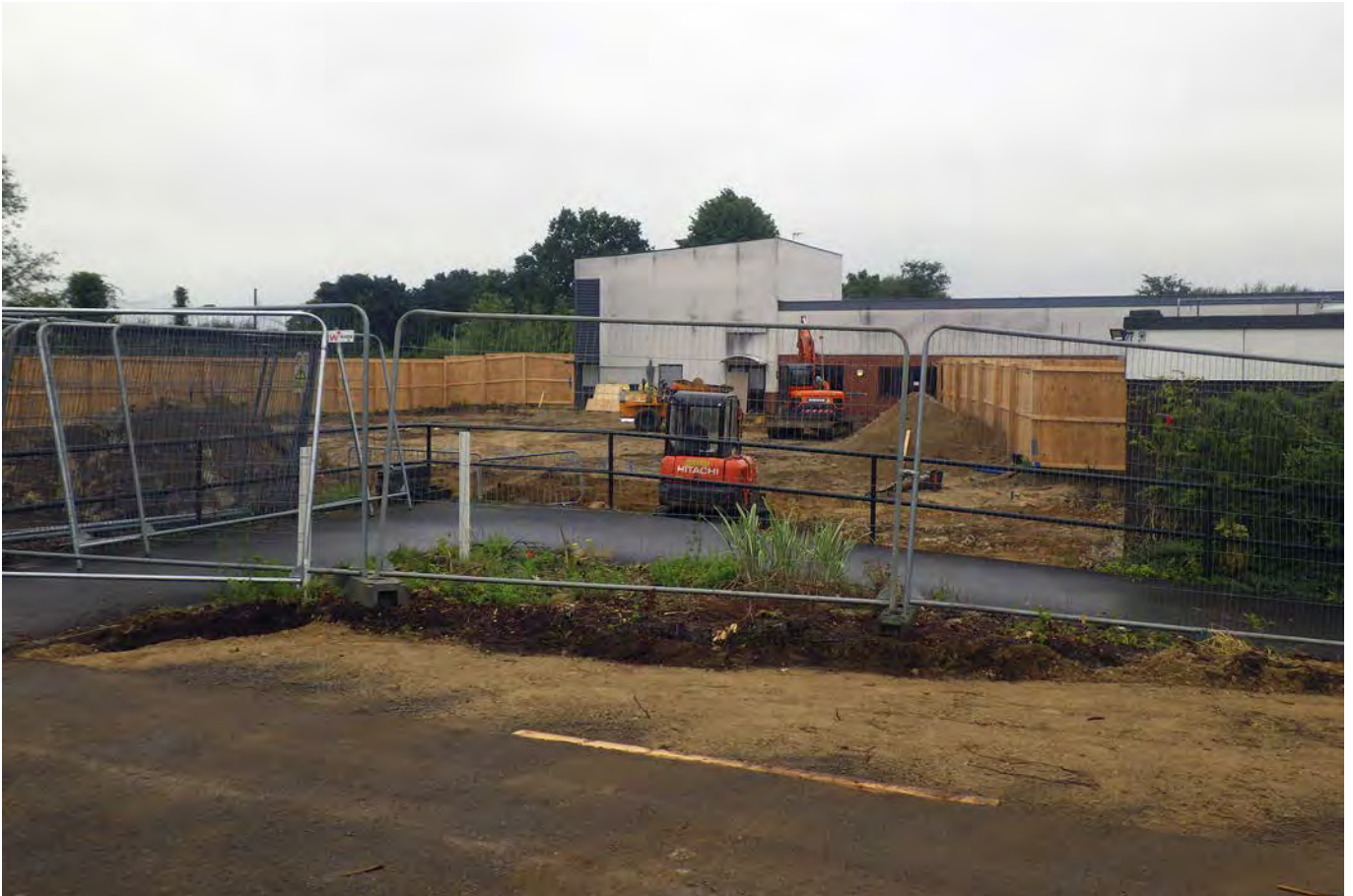
Plate 1: General view of site
