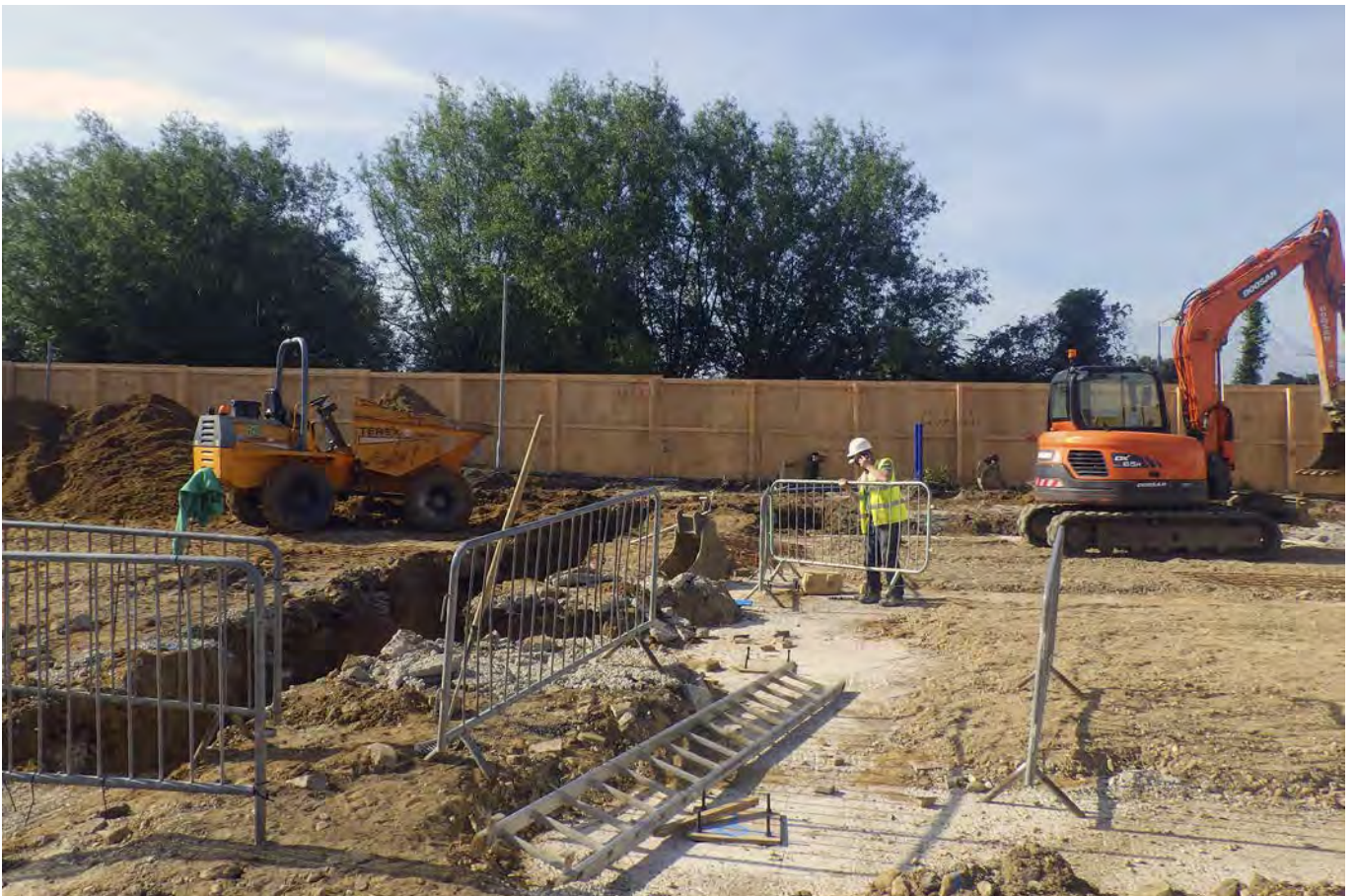
Plate 12: General view of work being carried out
