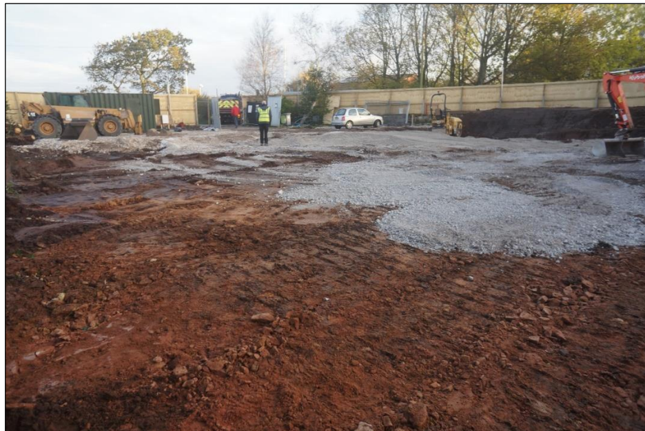
Plate 2: General view of site showing aggregate backfilling, looking north-east
