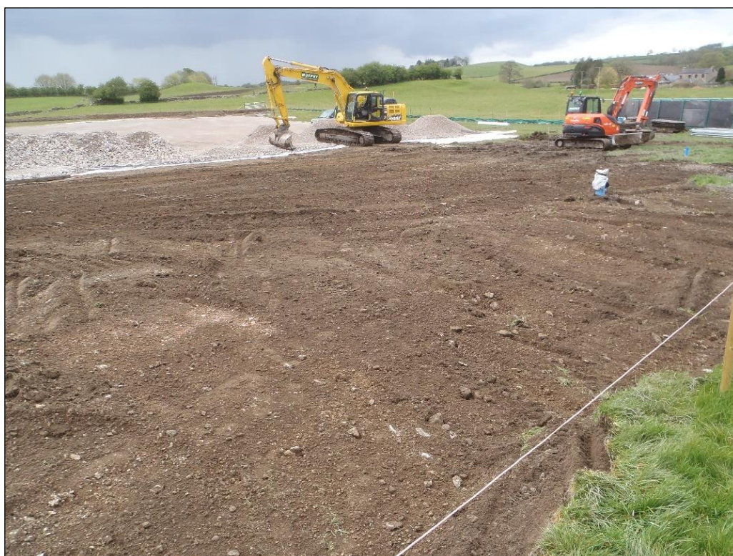
Plate 1: East end of strip area, looking south-east
