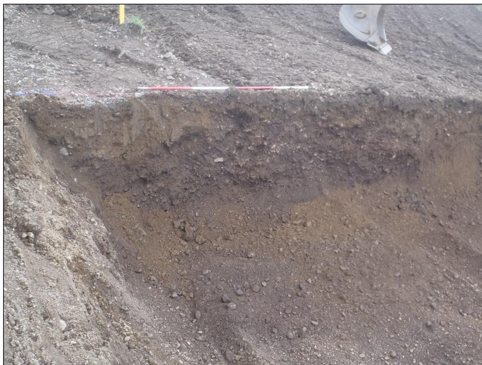
Plate 2: Excavation into the natural geology at the western end of the crane pad, looking north
