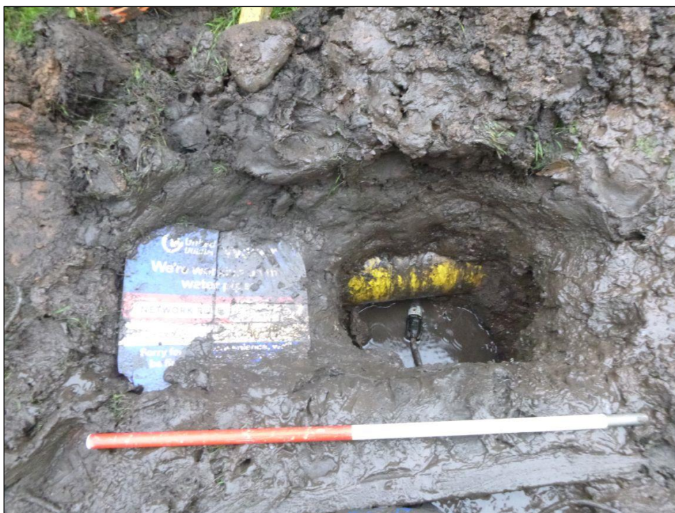
Plate 1: South-east-facing section of the trench, scale 1m
