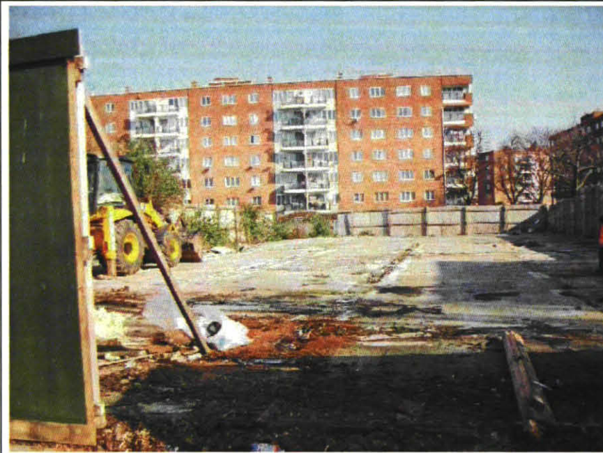
Plate 1: Concrete floor slab of the former neighbourhood office prior to demolition (looking west)
