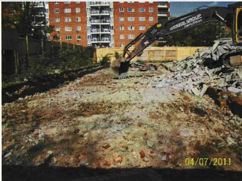
Plate 3: Modern backfill over late post-medieval/early modern foundations revealed after removal of floor slab
