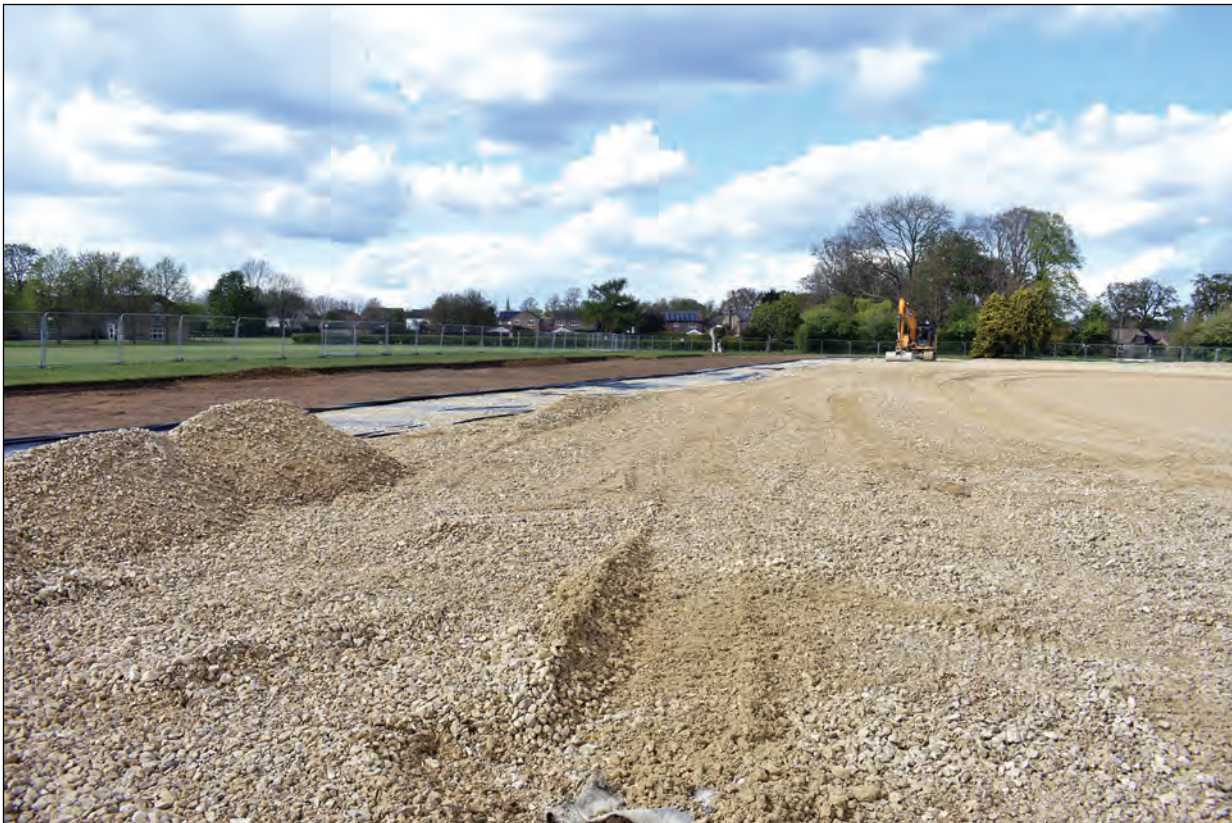
Plate 2: Installation of hardcore, looking north-west
