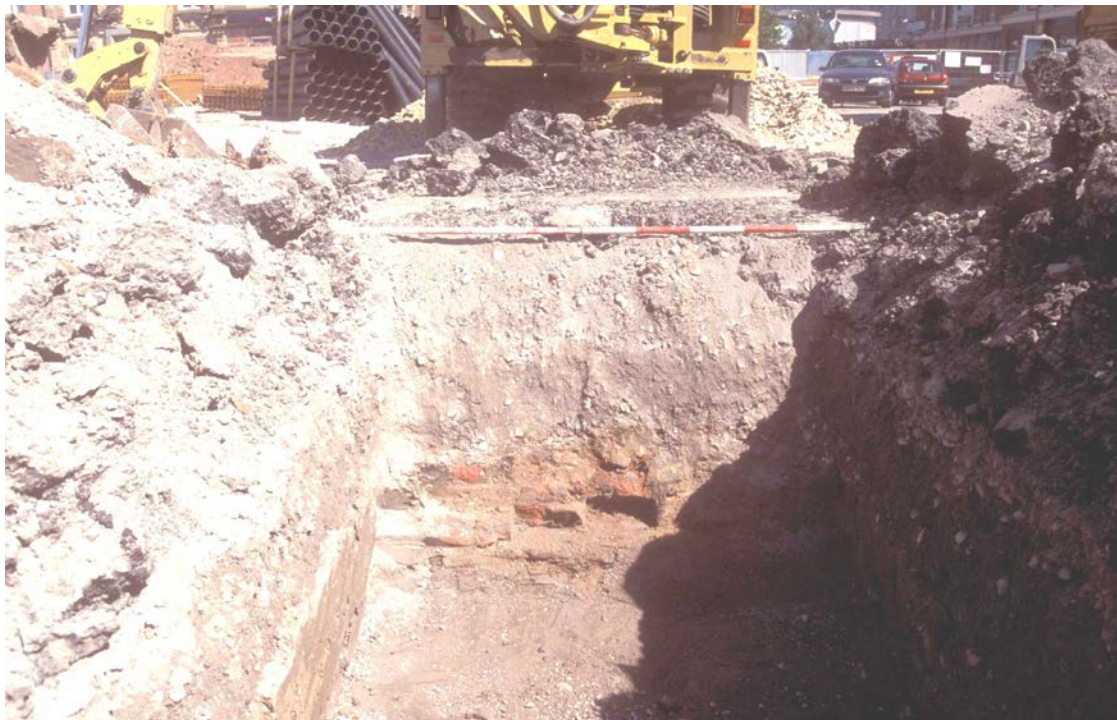
Plate 8: View of wall 907 , looking east
