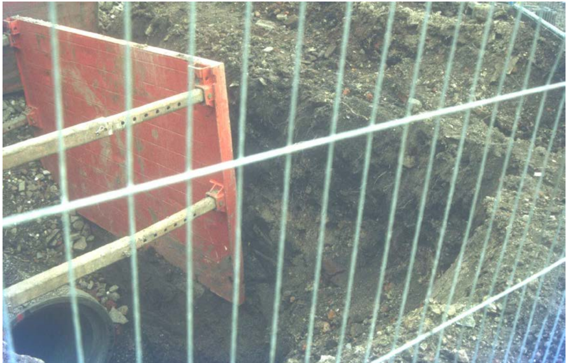
Plate 10: General view of Test Pit 2, looking west
