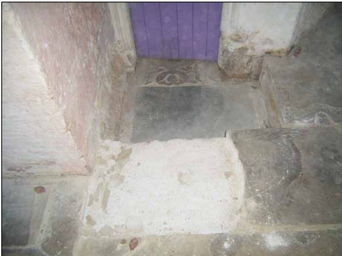
Plate 20. Foundation Pad 6 during excavation
