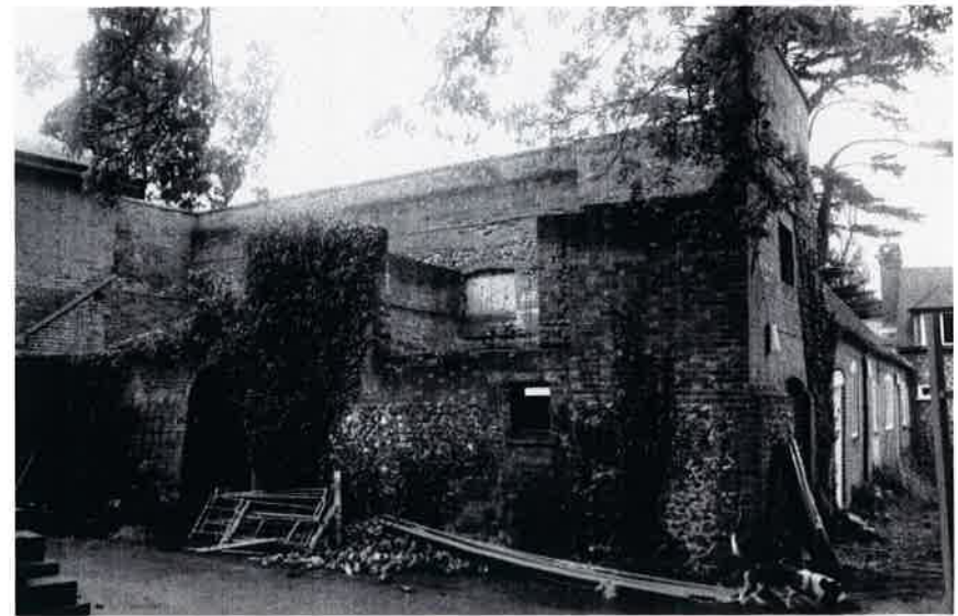
Plate 17: Ruined cottage. Note tapered wall front wall to left
