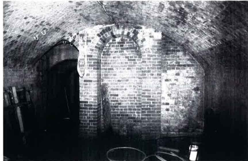
Plate 8: Brick arches in first cellar space
