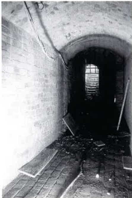
Plate 7: View south within cellar
