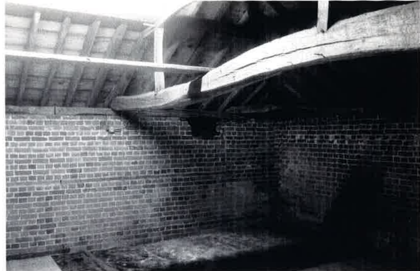
Plate 6: Warped tie beam to north of F3
