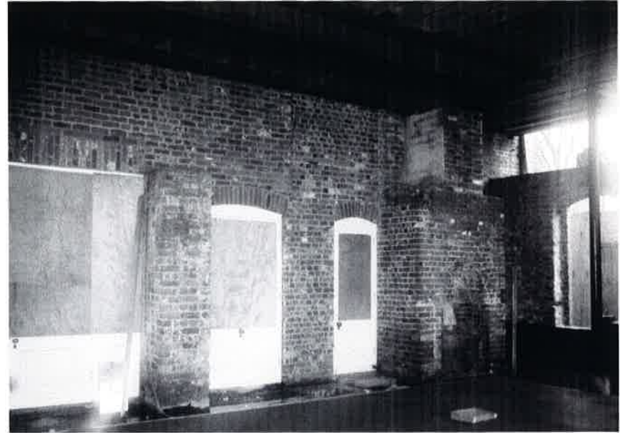
Plate 15: South wall of house during construction of conservatory
