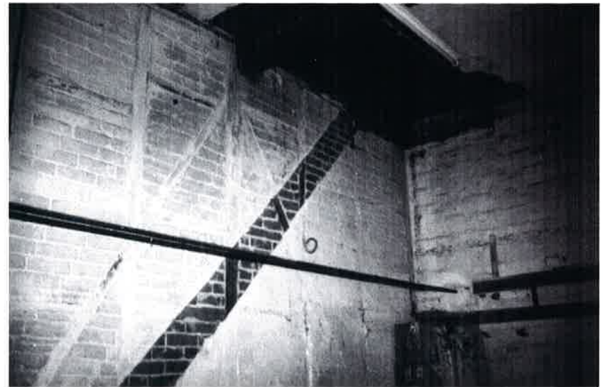
Plate 20: Imprint of former stairs within G4 adjacent to wall with timber frame and brick nogging
