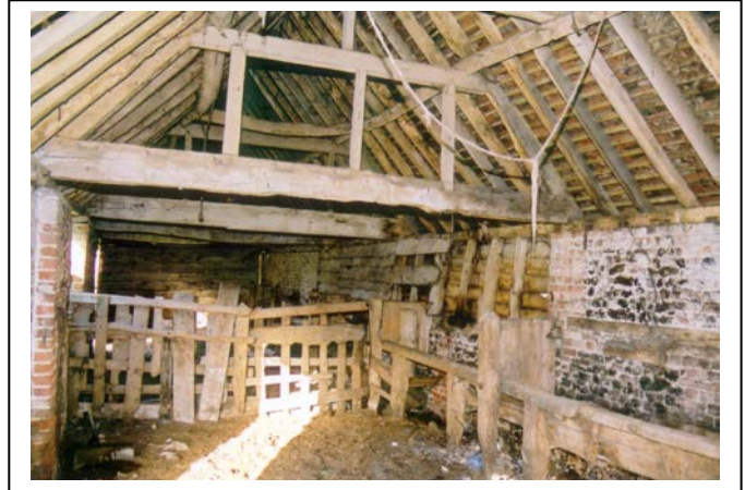
Plate 26: Interior of Building 8
