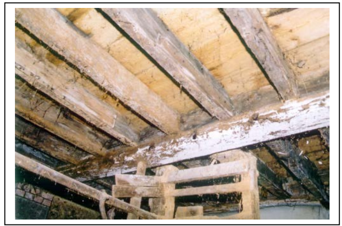
Plate 8: Underside of ground floor within basement
