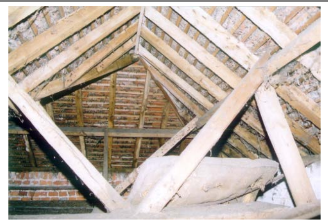
Plate 18: Roof above Bedroom 4
