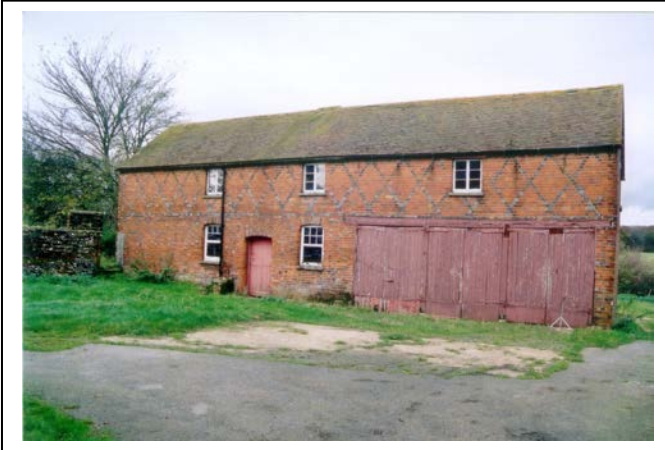
Plate 19: South elevation of Building 4
