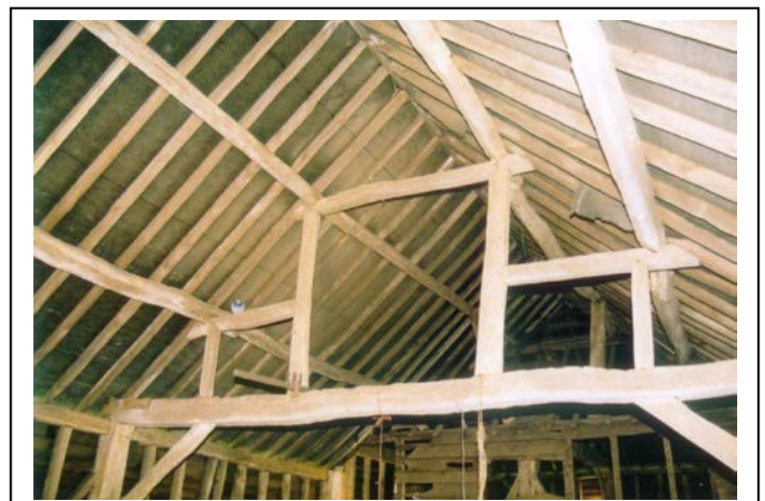
Plate 37: truss in E-W range of Building 11
