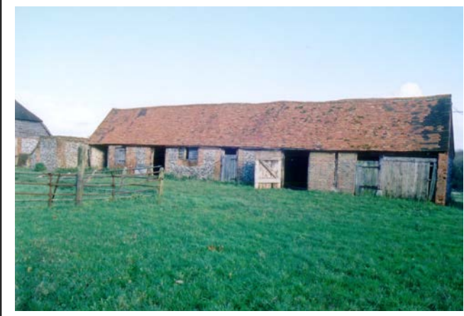
Plate 25: Building 8 from west
