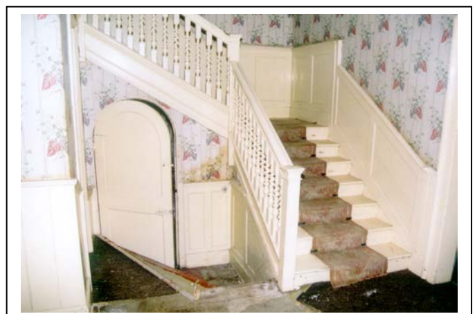
Plate 14: base of staircase
