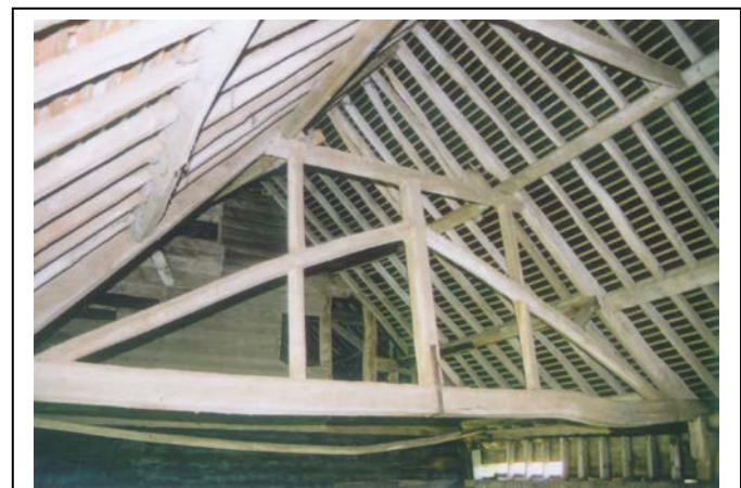
Plate 31: Roof truss in Building 10
