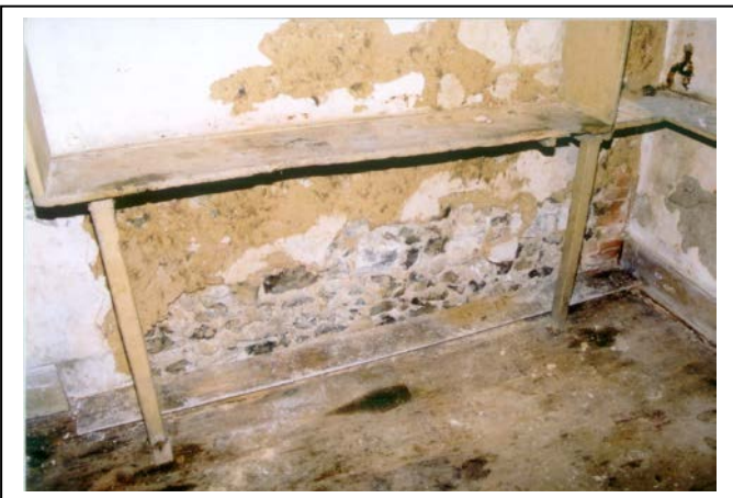
Plate 13: Flint in north wall of parlour
