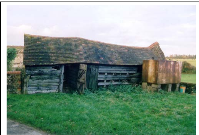
Plate 23: Shed at south end of Area 6
