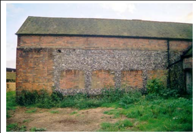
Plate 20: North elevation of Building 4
