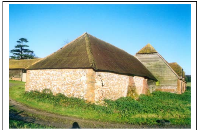
Plate 30: Building 10 from south-east
