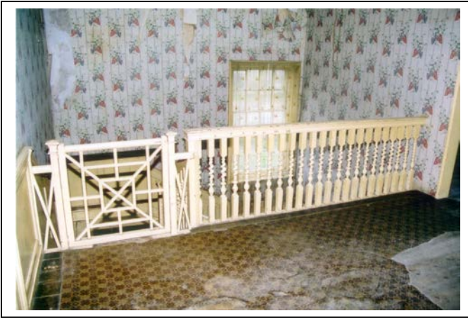
Plate 17: Landing at second floor level
