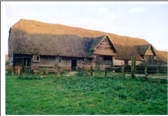
Plate 27: Aisled barn (Building 9) from north-west
