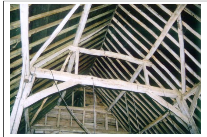
Plate 28: Truss within Building 9
