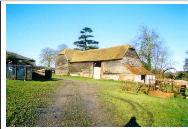
Plate 34: Building 11 from south-east
