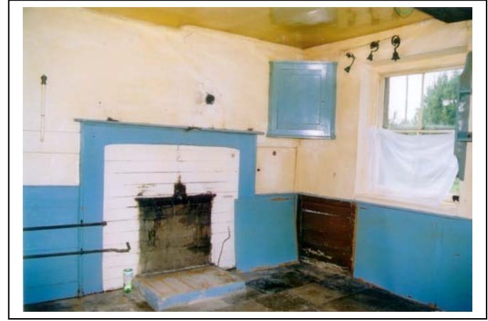
Plate 12: fireplace within kitchen
