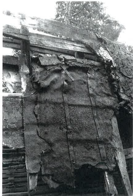
Plate 37 Collapsed phase VII paper-covered roof over room A after removal of several secondary layers of tarred paper, pitch, hessian and asphalt
