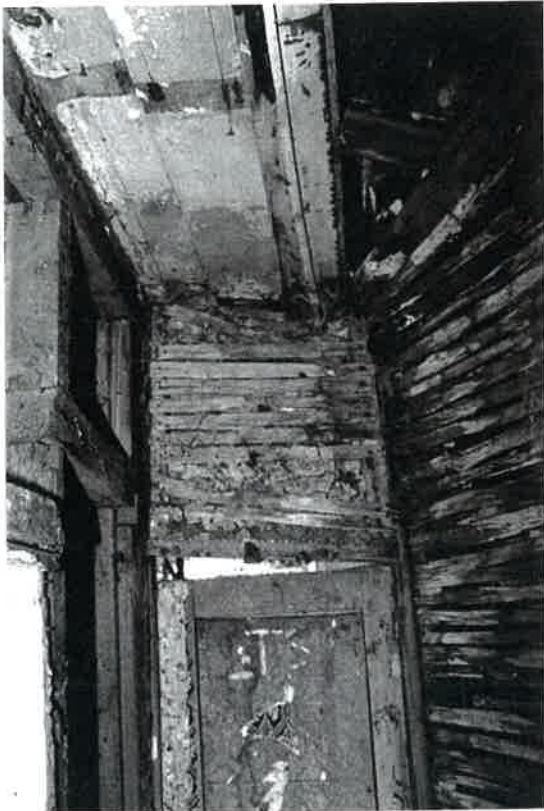
Plate 43 Upper tower room (T), showing lathwork, door to room H and phase I eaves
