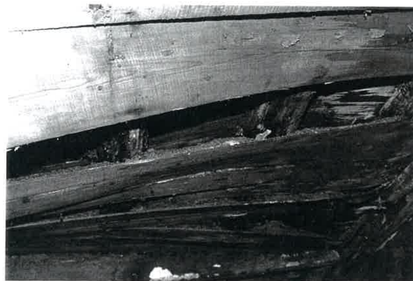
Plate 25 Phase II roof from the underside (room B). Note the halved log common purlins, sawdust fill. The sawdust was originally retained within the roof by a layer of coarse brown paper between the inner boards and the common purlins
