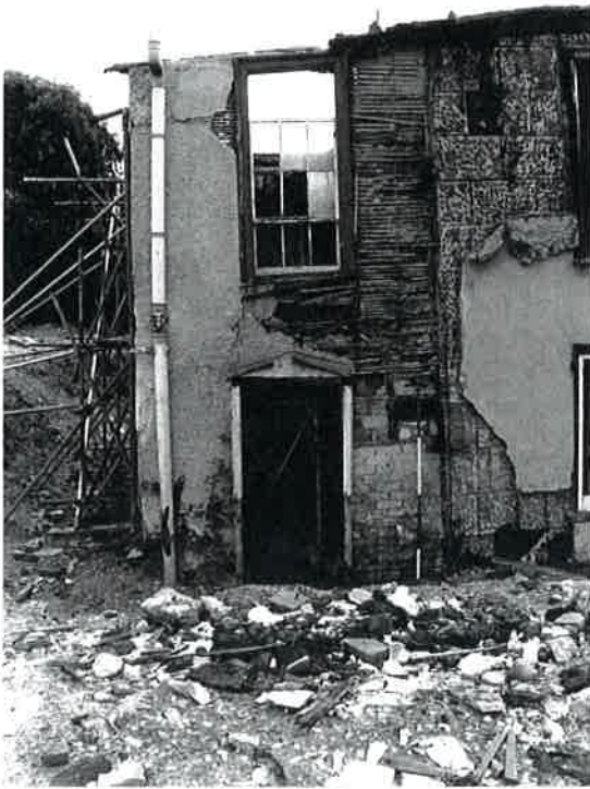
Plate 36 North elevation of phase VII extension (A/J) abutting the phase II extension (B/K). The floor between the ground and first floors was found to contain the paper-covered roof from the phase V single-storey building on the site however, the exterior walls, which were always of lath and render construction, appeared single-phase
