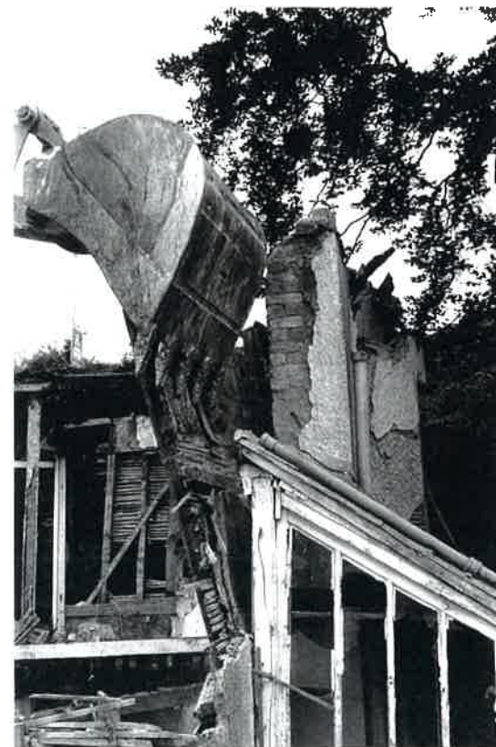
Plate 35 View of the west wall of rooms D/P during demolition showing the primary tarred fibreboard panels and secondary un-tarred faux -ashlar tiles continuing behind the phase VI chimney
