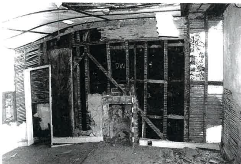
Plate 12 The interior of the phase I west wall of room D showing the inserted fireplace, the tarred fibreboard exterior cladding and later phase II roof. Note the phase IX extension on right with original rafter end incorporated
