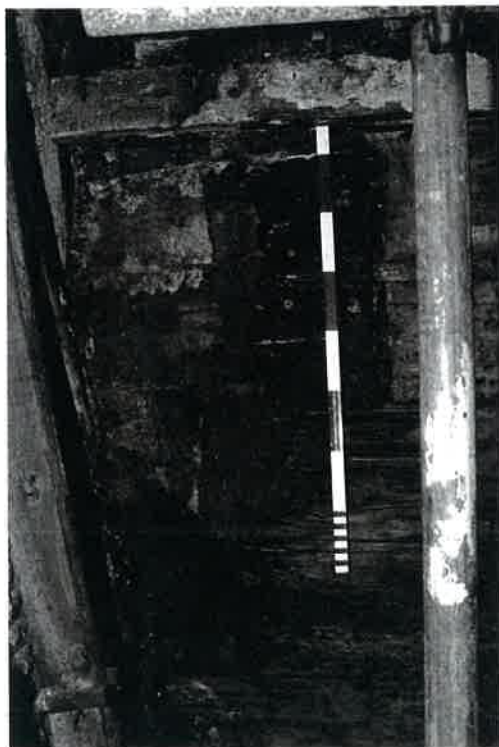
Plate 29 Vestiges of oiled card and tarpaulin on the former exterior boarding of the north wall of room M, visible after removal of later interior boarding in room J
