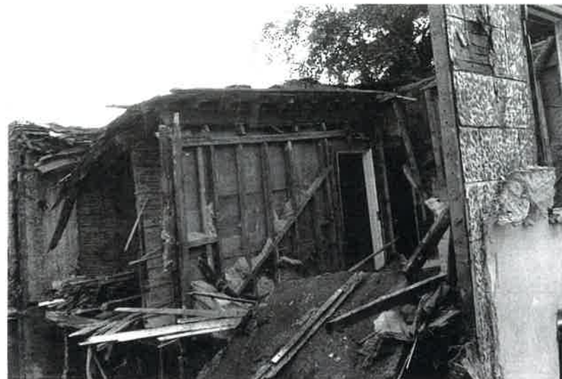
Plate 11 The former north wall of the phase I house showing single diagonal, upper brussumer plate and the eaves of the phase I roof. Prior to dismantling this wall was clad with tarred feather-edge boarding overlain by traces of tarred card
