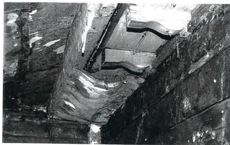
Plate 17 The original eaves of the phase I roof still extant within room B of the phase II extension (B/K). Note the tarred feather-edge boarding of the phase I north wall below
