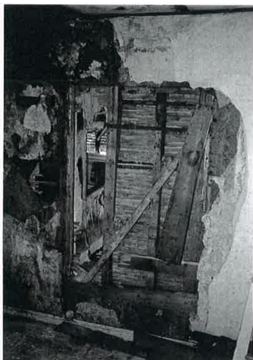
Plate 20 Former phase I south window of room D, blocked with boarding and lathwork of room H. Note fragments of primary wallpaper and phase I plain fibreboard internal wall panels
