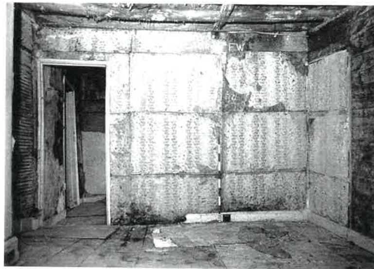
Plate 15 The west wall of room F showing plain fibreboard panels (phase I reused) retaining primary wallpaper. Note phase I roof and blocked door to right
