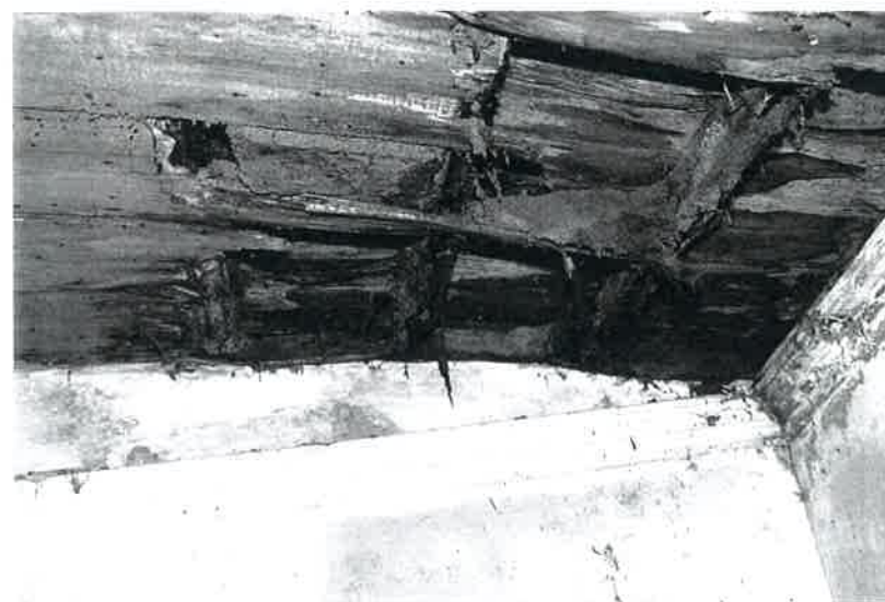
Plate 42 Detail of phase VIII roof, showing common purlins and sawdust-filled cavity
