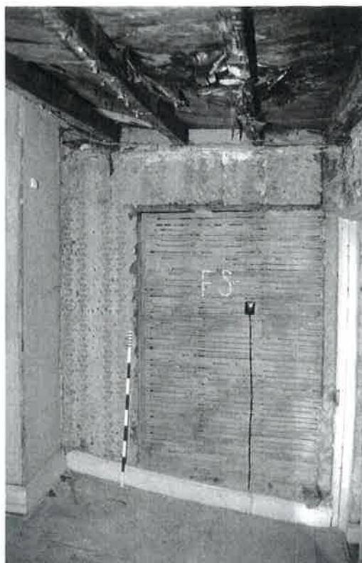
Plate 19 Former phase I south window in room F, blocked with lath and plaster. Note primary plain fibreboard wall panels and wallpaper overlain by phase VI chimney-breast
