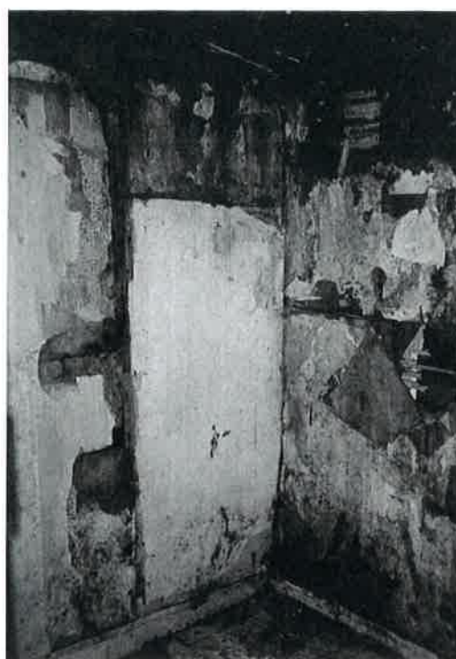
Plate 21 Blocked phase I door between rooms D and E. Note primary wall panels and fragments of original wall paper
