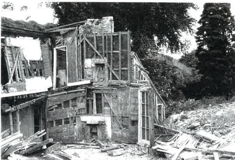
Plate 10 The phase I south and west walls of rooms D/P during demolition showing studding, tarred fibreboard exterior cladding and inserted fireplaces
