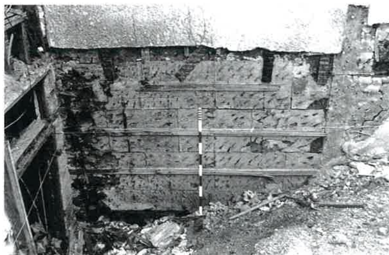
Plate 32 View of the south wall of rooms F/M, showing how the faux -ashlar tiles on phase I section of the wall about those of the Phase IV extension. They also overlay the phase I south windows of both rooms (on left)
