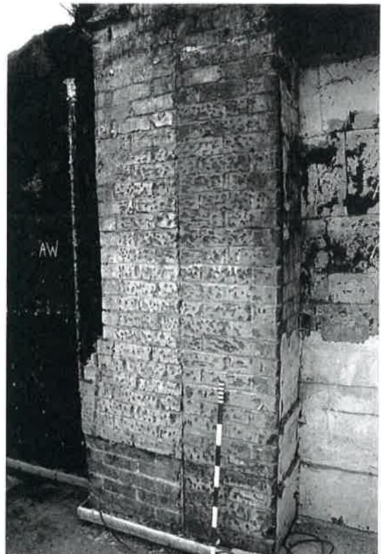
Plate 28 Upper portions of phase 3a and 3b chimneys within room A. Both chimneys overlay the tarred card wall tiles of the former east external wall of the phase II extension (on right). Note the remains of exterior paint on both chimneys and wall tiles
