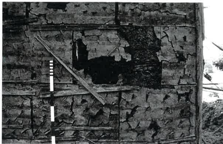
Plate 30 Phase IV tarred paper and untreated faux -ashlar card tiles revealed after the removal of later scribed render and pebbledash on the south wall of F/M extension
