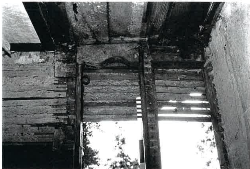
Plate 34 Detail showing west wall of room D showing the former rafter end and eaves and the phase IV northward extension
