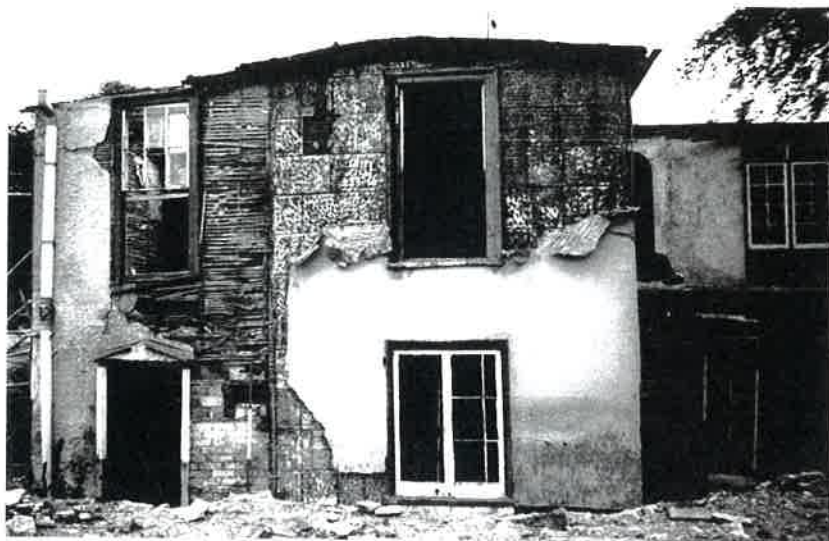
Plate 22 North elevation of phase II extension (B/K), abutted to left by phase V/VII extensions J/A. Note painted tarred card wall tiles and curved roof profile.
