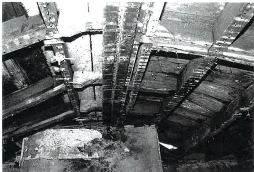
Plate 33 Ceiling/roof of room F showing phase I roof (including former rafter ends) to right and phase IV roof to left. Note length of bridge rail taking the place of the phase I east wall and slightly staggered noggins indicating the possible position of a window or chimney breast
