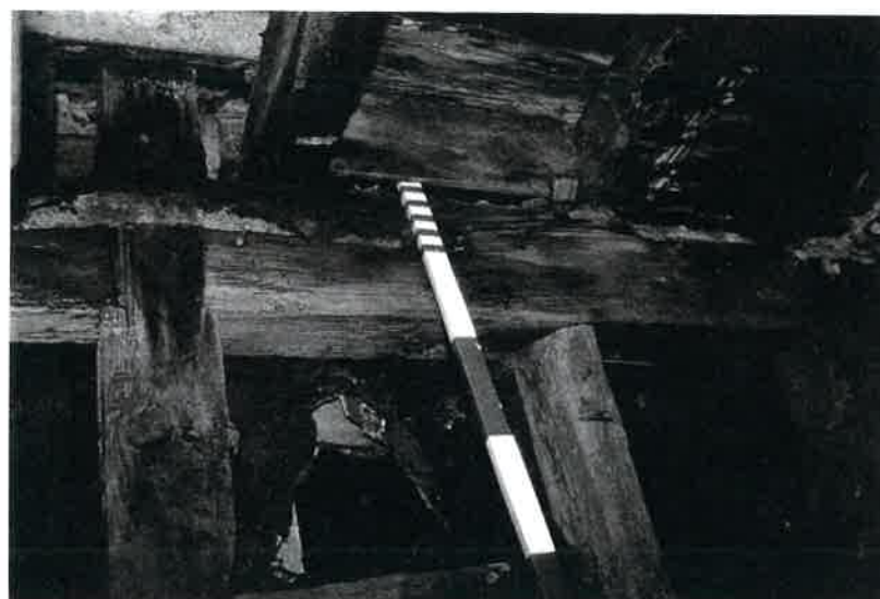
Plate 13 Studding detail within south wall of room P showing first floor brussumer supporting joists and phase I exterior tarred fibreboard behind
