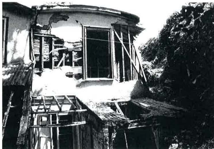
Plate 38 West elevation of phase VIII extension (rooms G/H/I-N/Q) showing the curved profile of the paper-covered roof and stud, lath and render wall construction
