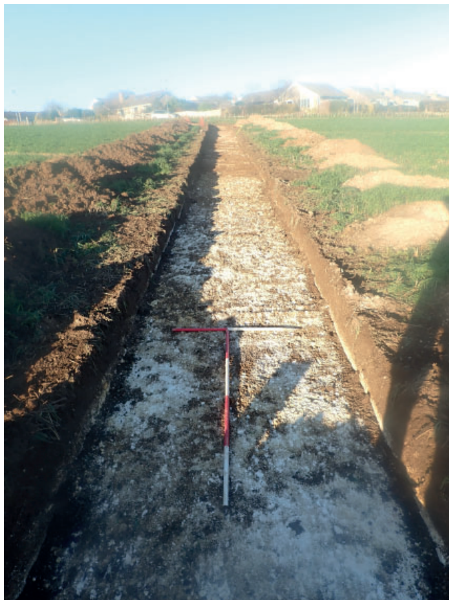
Plate 1: Trench 3, view to NE
