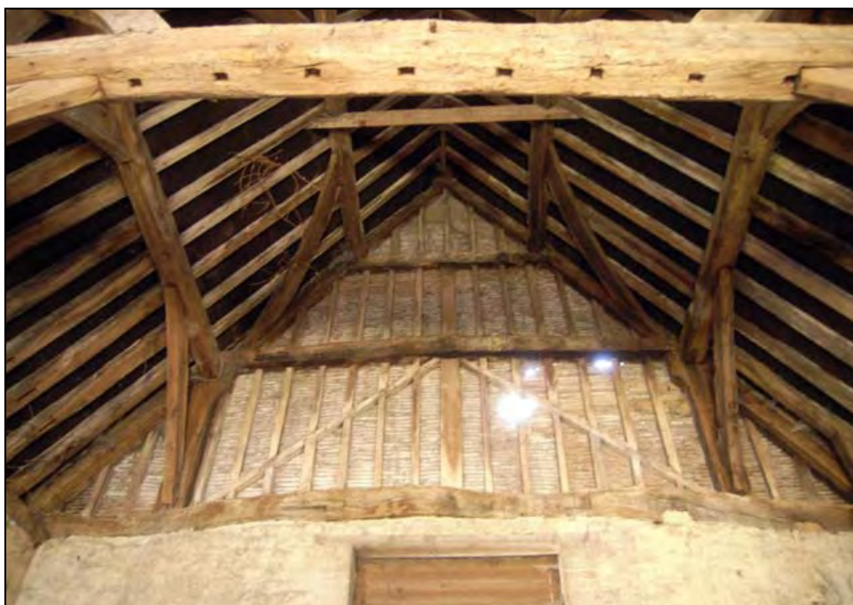
Plate 10: South roof truss with later infill
