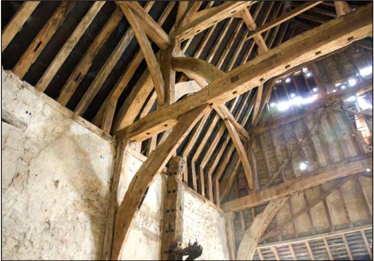
Plate 15: West end of central truss showing complex bracing arrangement
