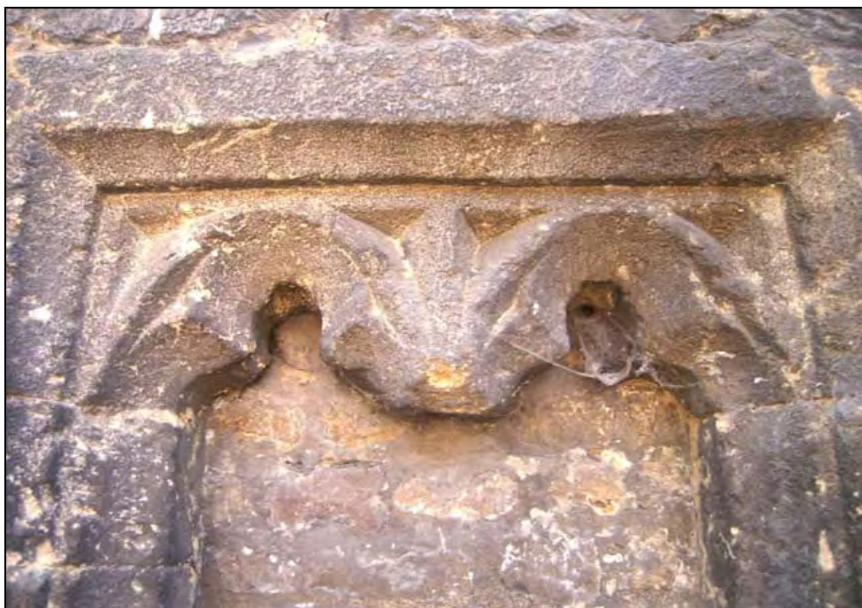
Plate 4: Moulded window head in east wall
