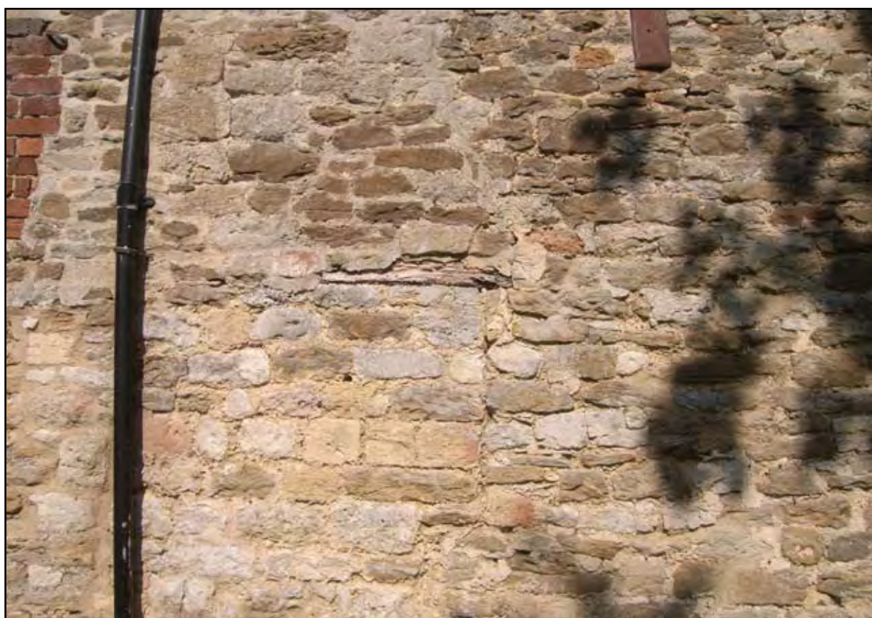
Plate 6: Blocked openings and rebuilt masonry in west wall
