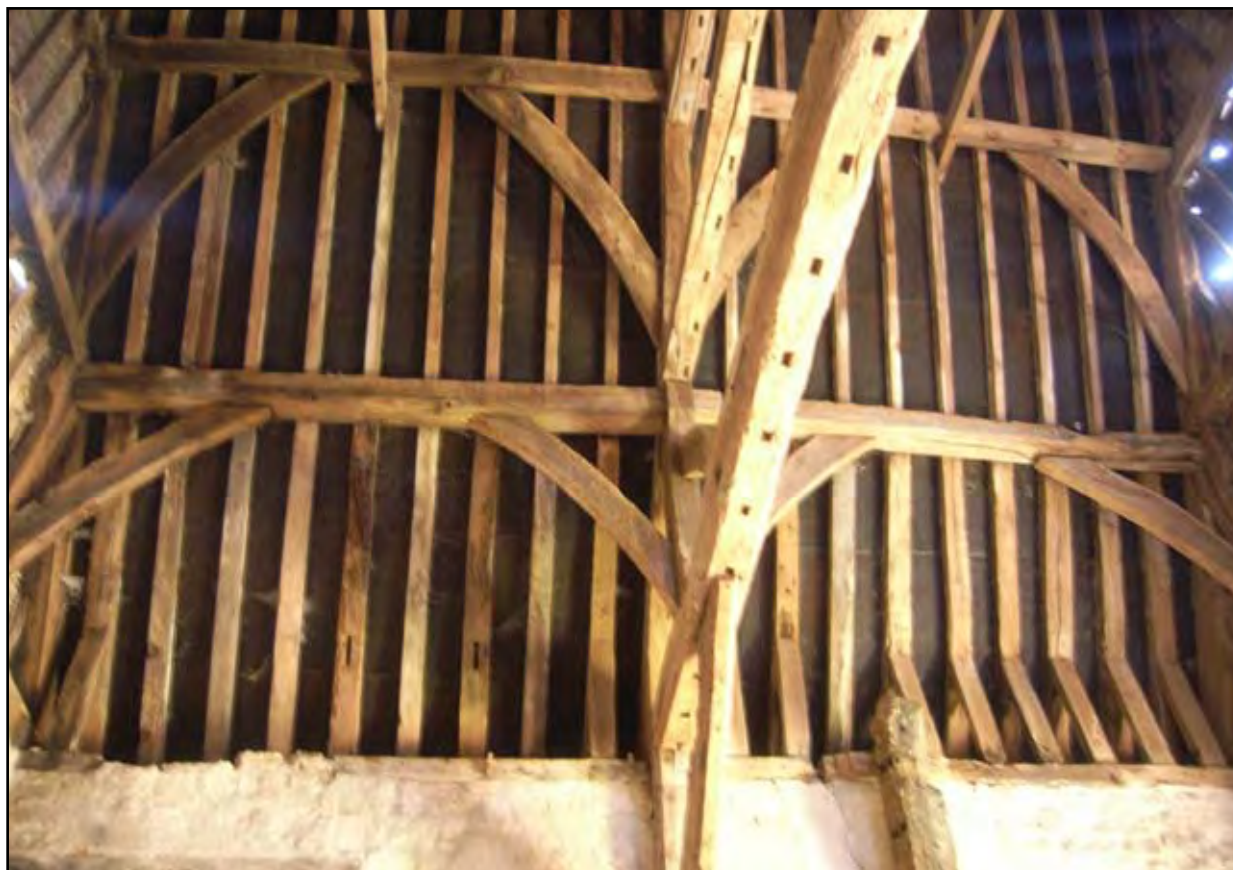
Plate 13: West slope of roof showing rafters and bracing
