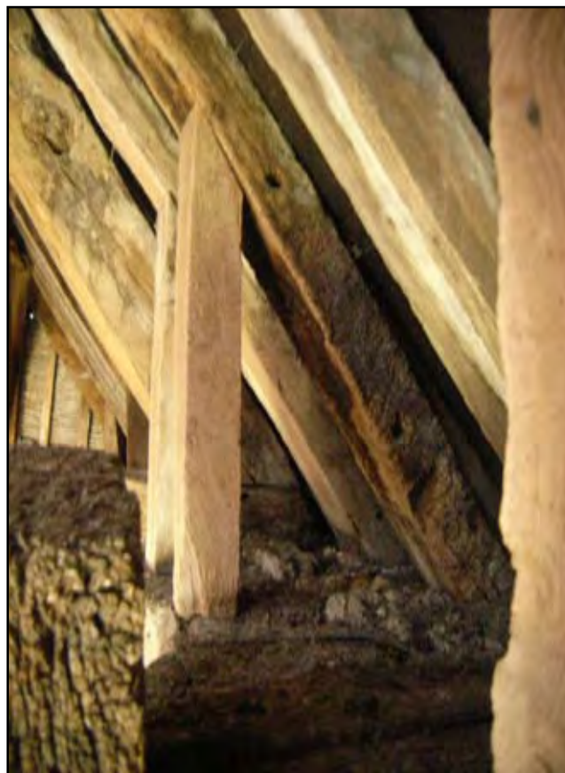
Plate 16: Detail of wallplate, rafter and ashlar piece construction
