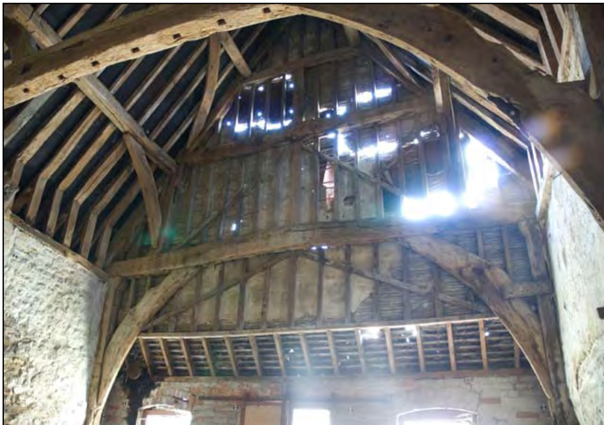
Plate 11: North roof truss with studwork infill
