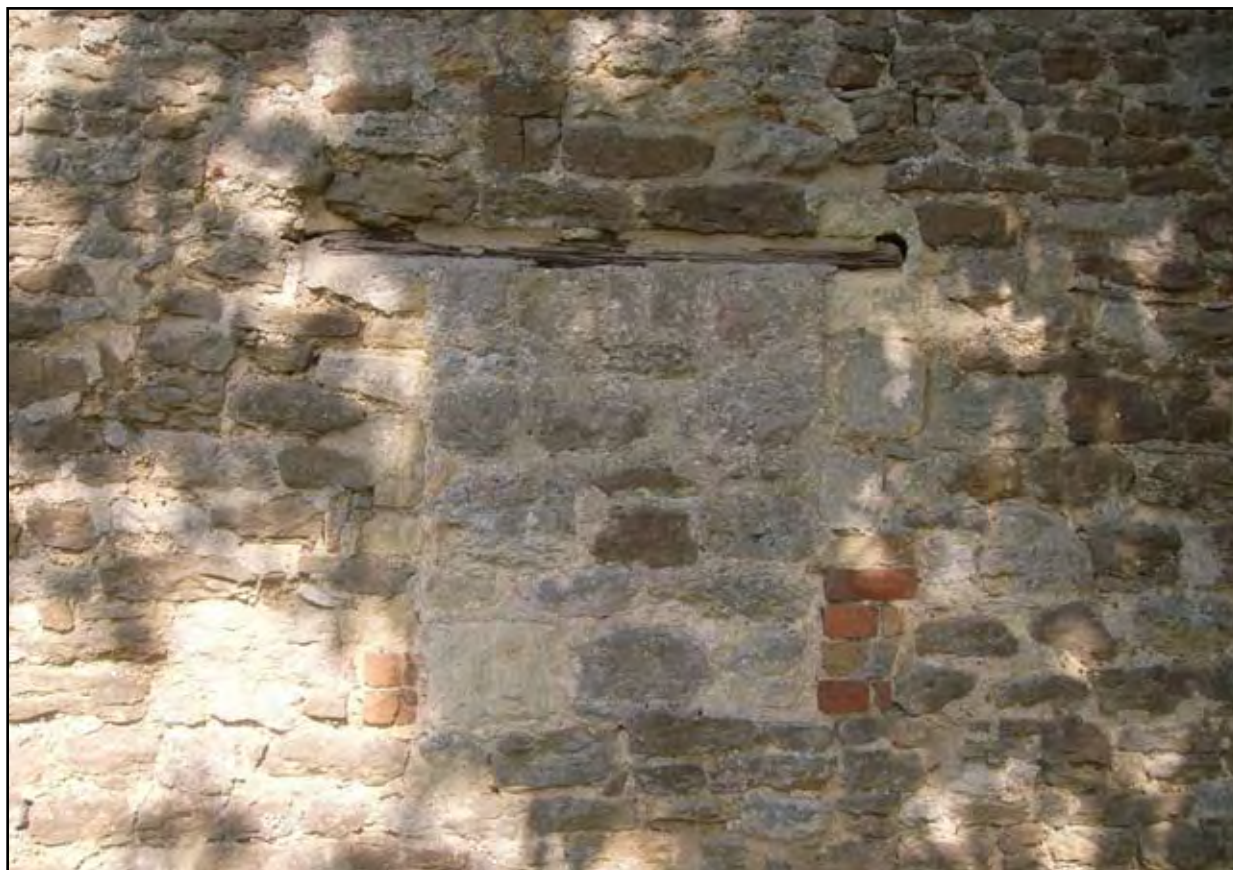
Plate 5: Blocked inserted window in west wall
