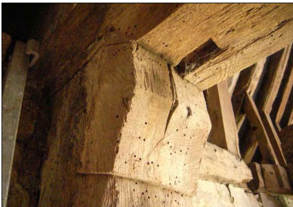
Plate 14: Moulded top of raised arcade post in central truss
