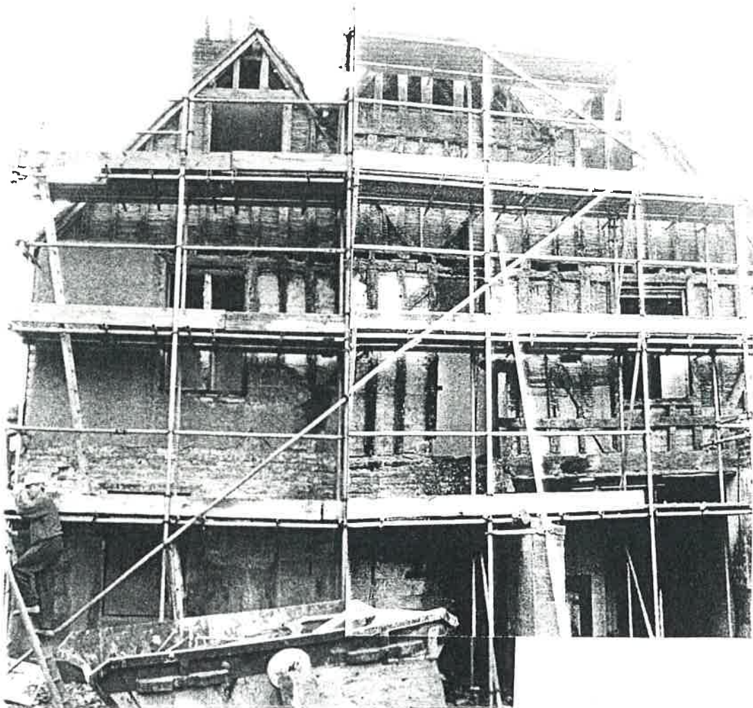
Plate 2: North elevation after removal of brick lean-to
