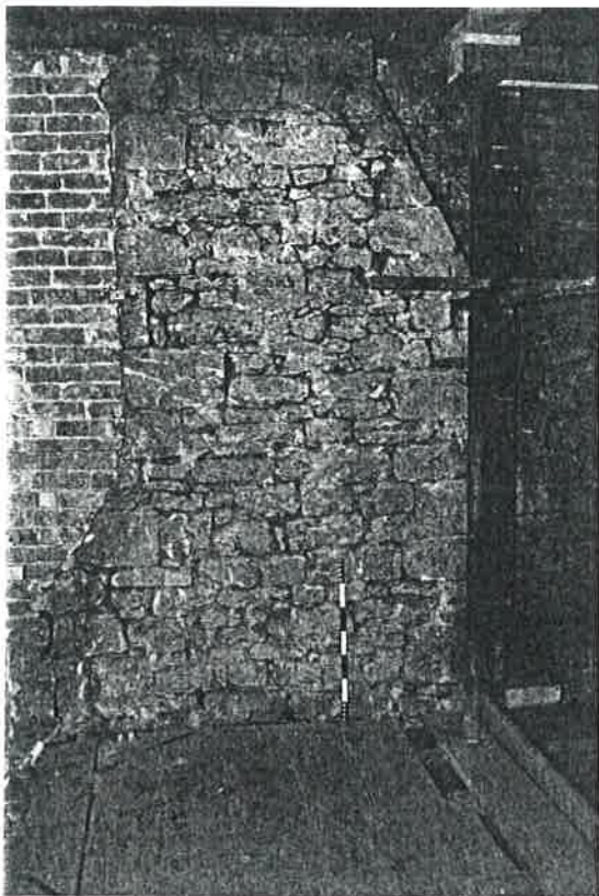
Plate 18: Room 1F/2 west wall - detail of chimney of adjacent property
