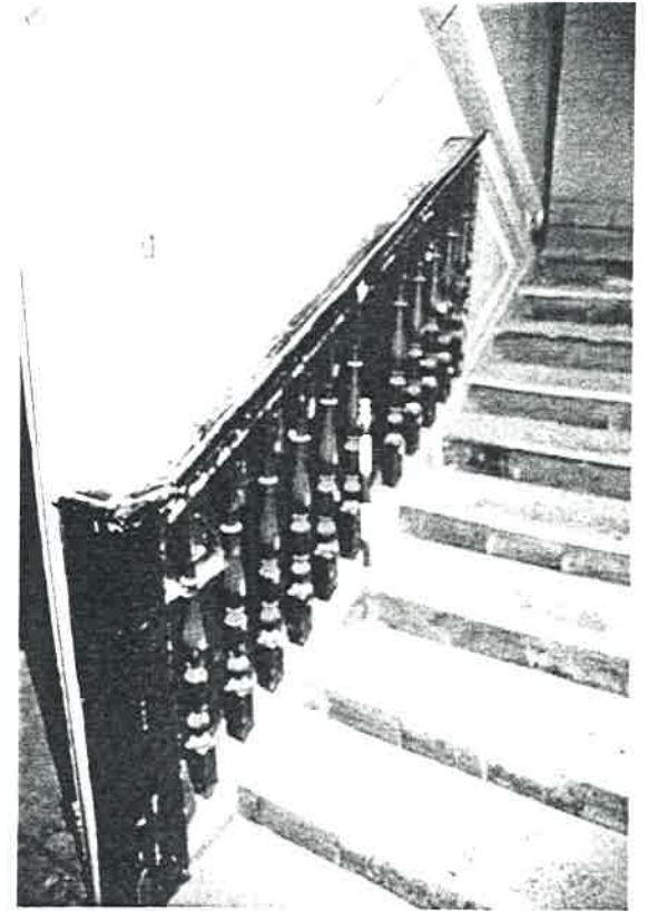
Plate 11: Detail of staircase
