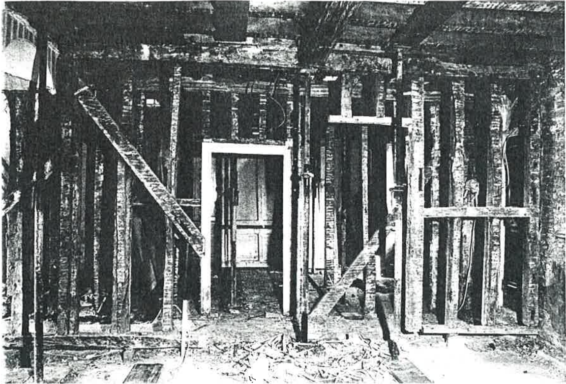
Plate 7: Room GF/2 - partly dismantled passage wall supporting principal joist
