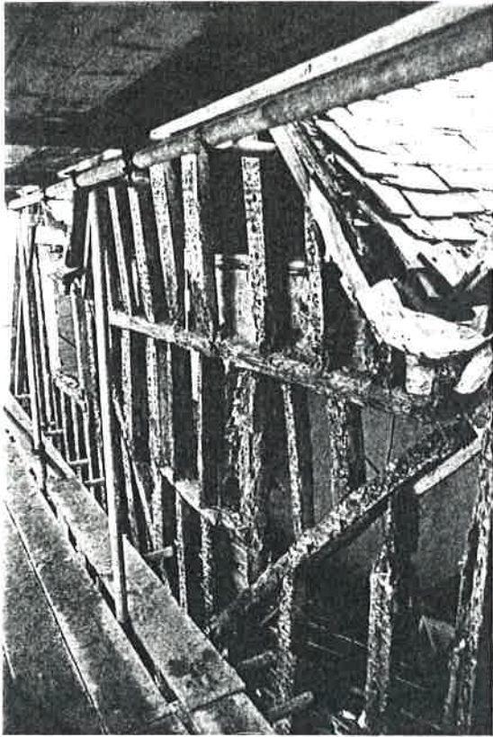
Plate 3: North elevation - second floor, east end
