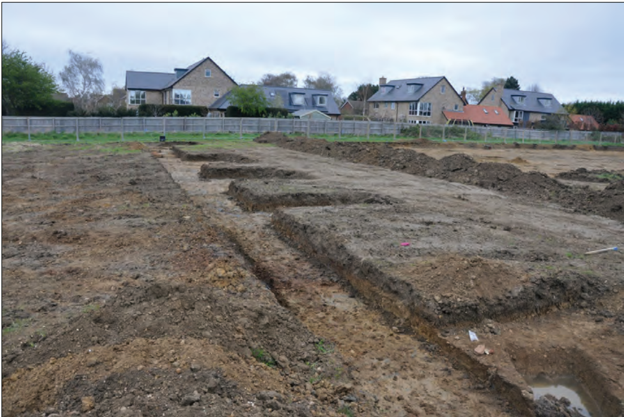
Plate 4: Area 3, looking north-east
