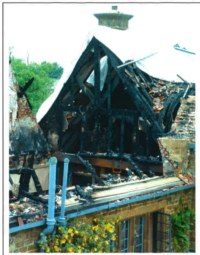
Plate 8: View east - fire damage to roof structure
