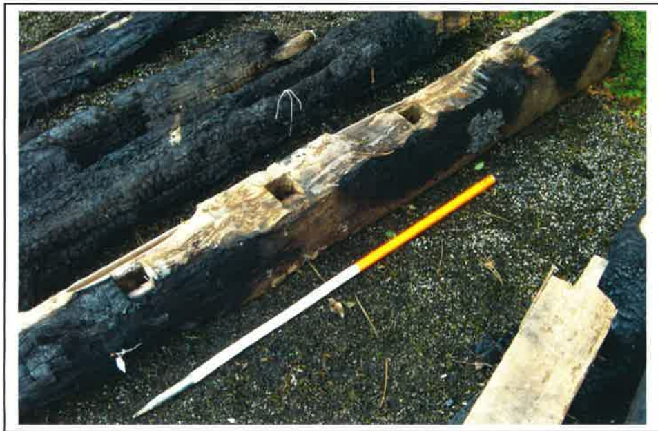
Plate 17: Deatial of charred primary beam - south west wing roof
