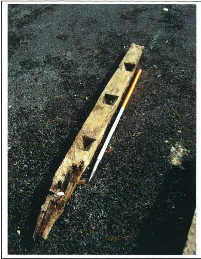
Plate 13 : Damaged ceiling beam - south west wing
