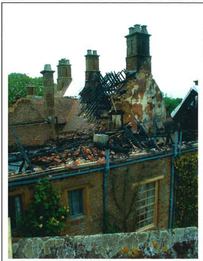
Plate 7: View east - fire damage to roof structure
