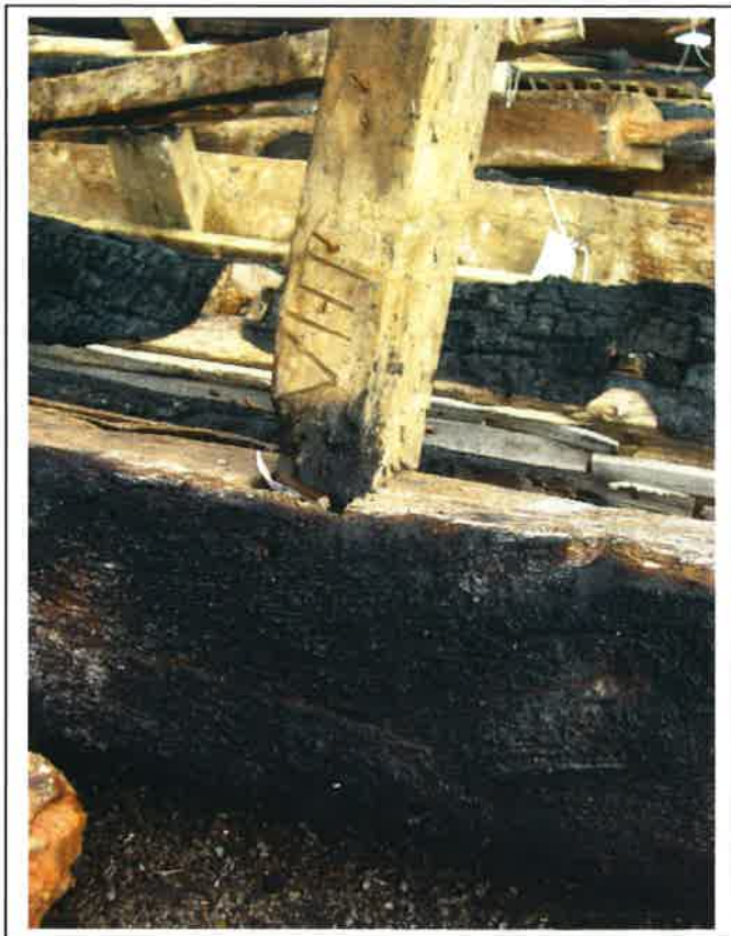
Plate 15 : Construction numbers on ceiling joist
