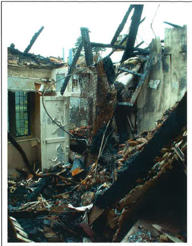
Plate 5: View west - collapsed roof above 1st floor
