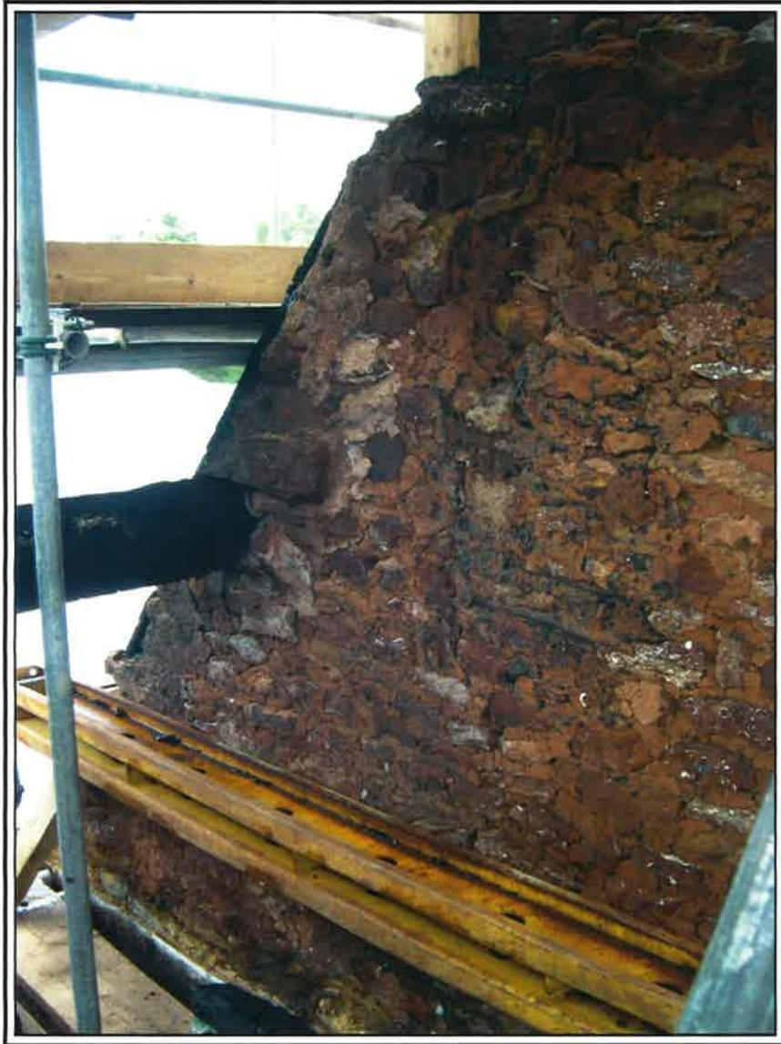
Plate 13 : Charred purling embedded in south east side of elevation
