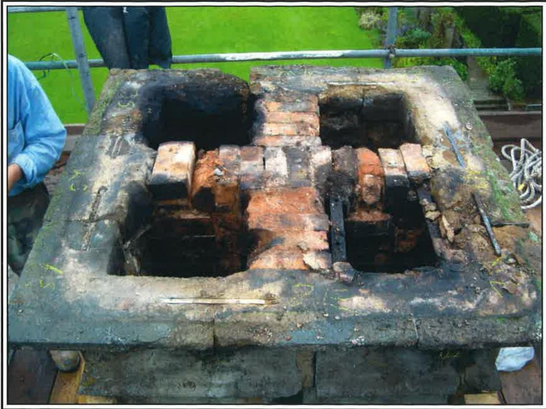
Plate 11 : Detail of chimney with stacks removed - view south west
