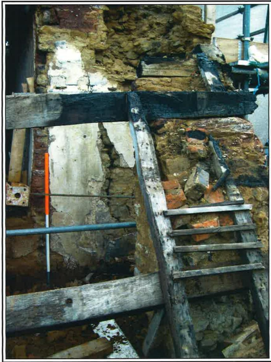
Plate 21: Detail of purlins on north west side of elevation
