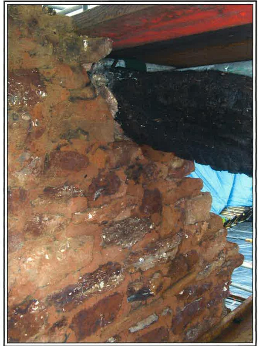
Plate 14 : Charred purlin embedded in north west side of elevation
