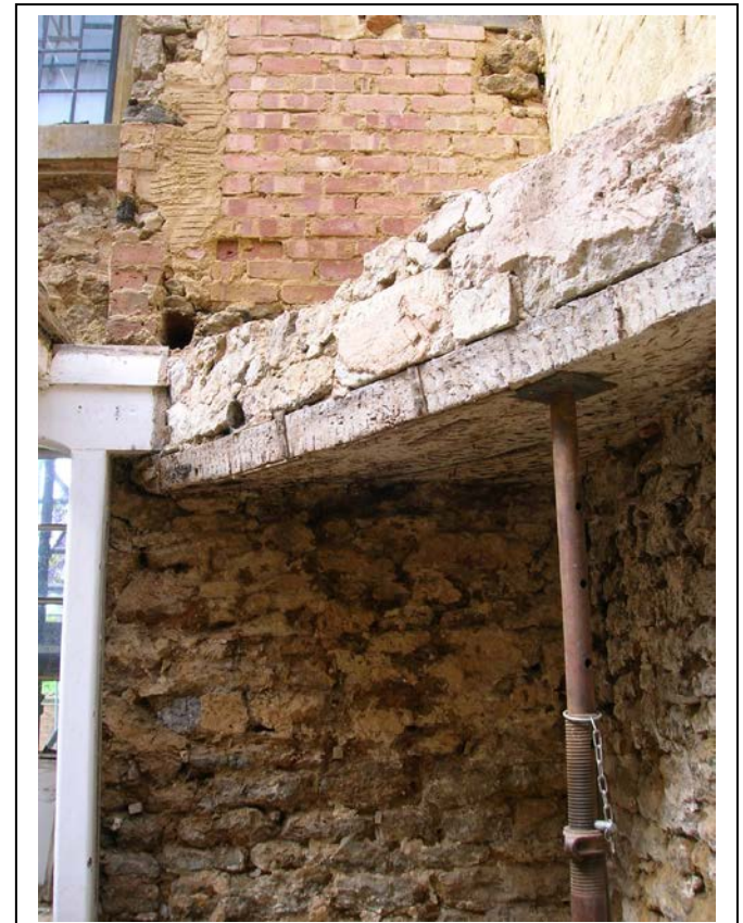
Plate 16: Detail of chimney base and support below.
