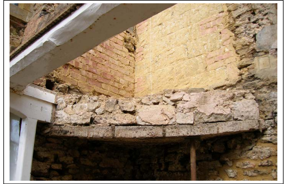
Plate 6: View west - timber and stone elements of the chimney base.
