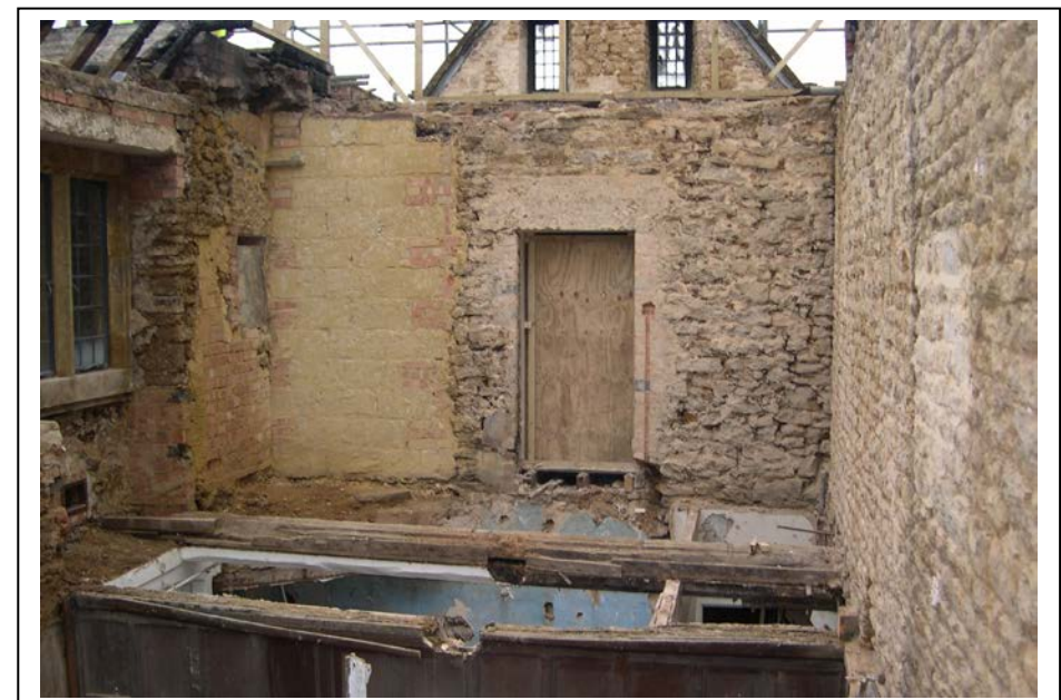
Plate 12: View north west -first floor with base location to the left.
