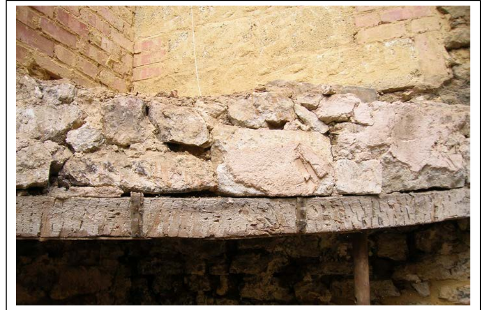
Plate 10: View west - detail of chimney base structure.
