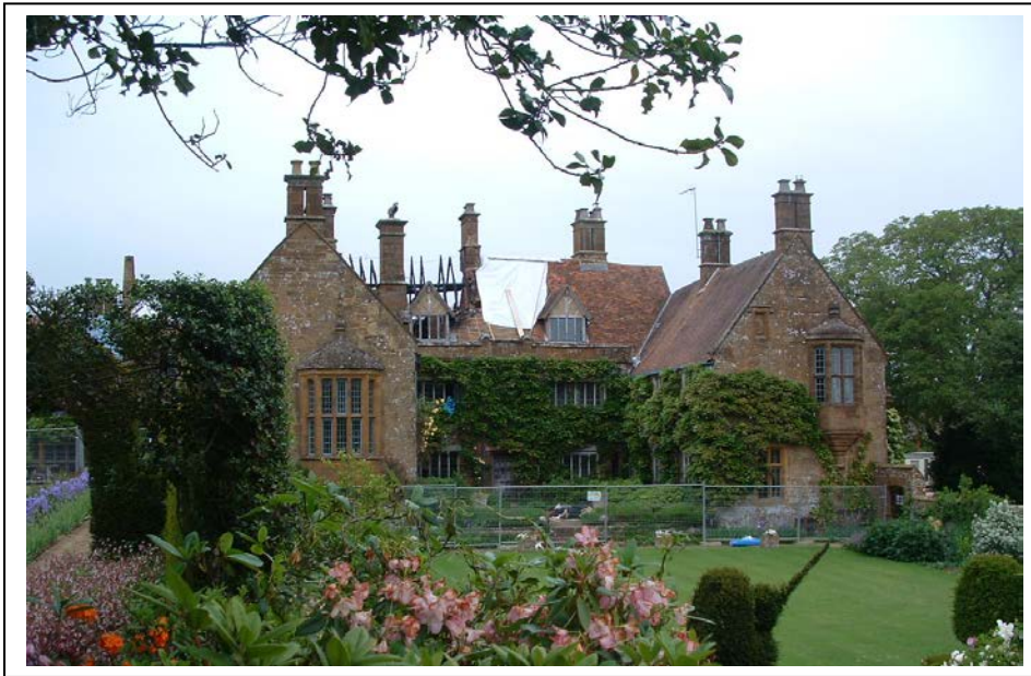
Plate 1: View north west - general view of house.
