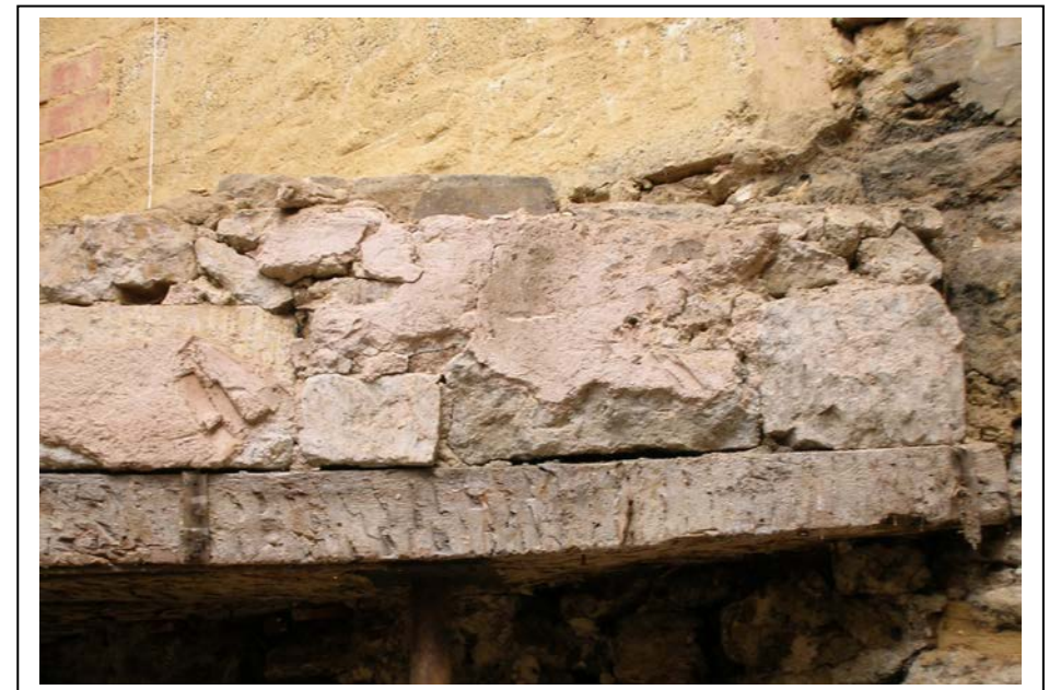
Plate 8: Right side of base showing timber and rubble construction.
