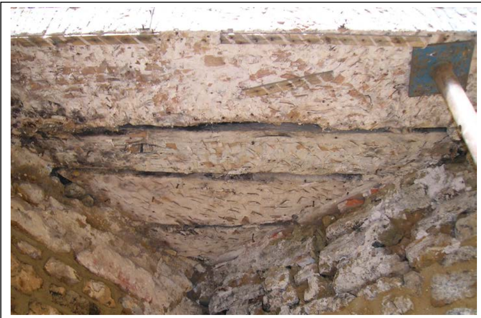
Plate 11: Underside of the four timbers forming bottom element of the base.
