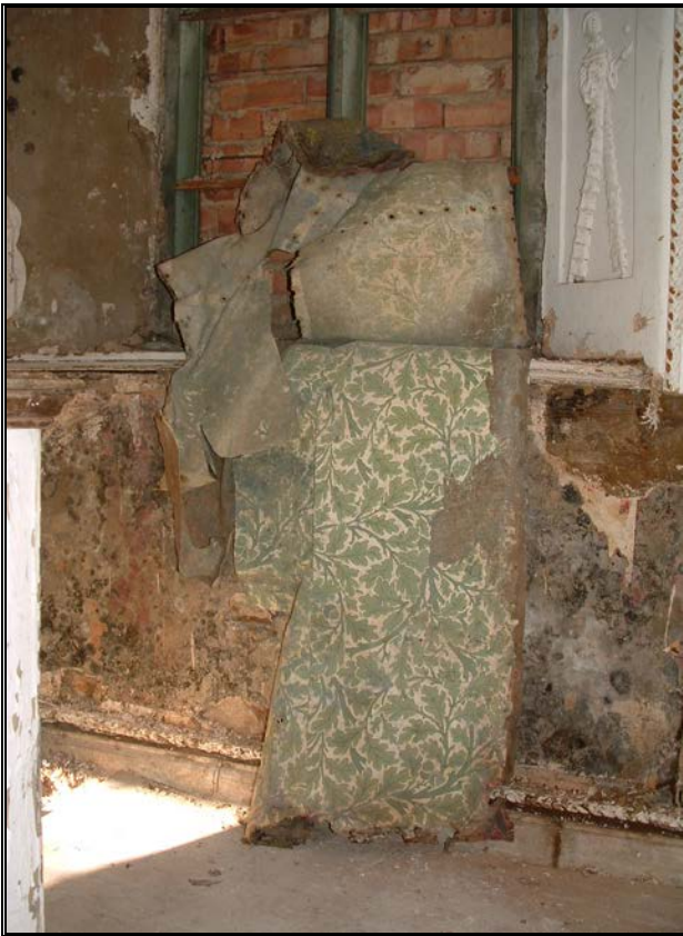
Plate 6: View north - Green oak leaf wallpaper revealed under the fibrous plasterwork.
