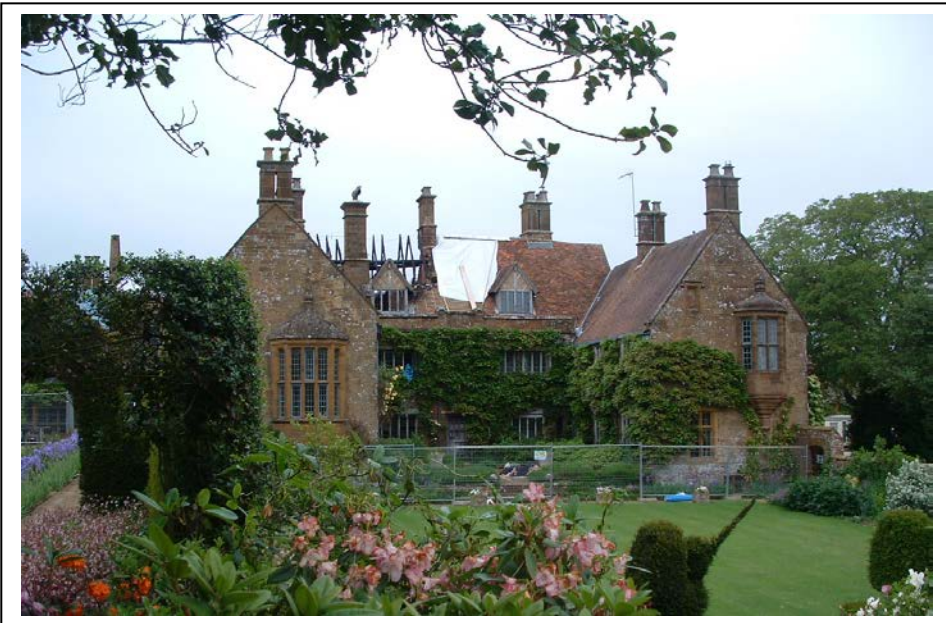
Plate 1: View north west - general view of house.
