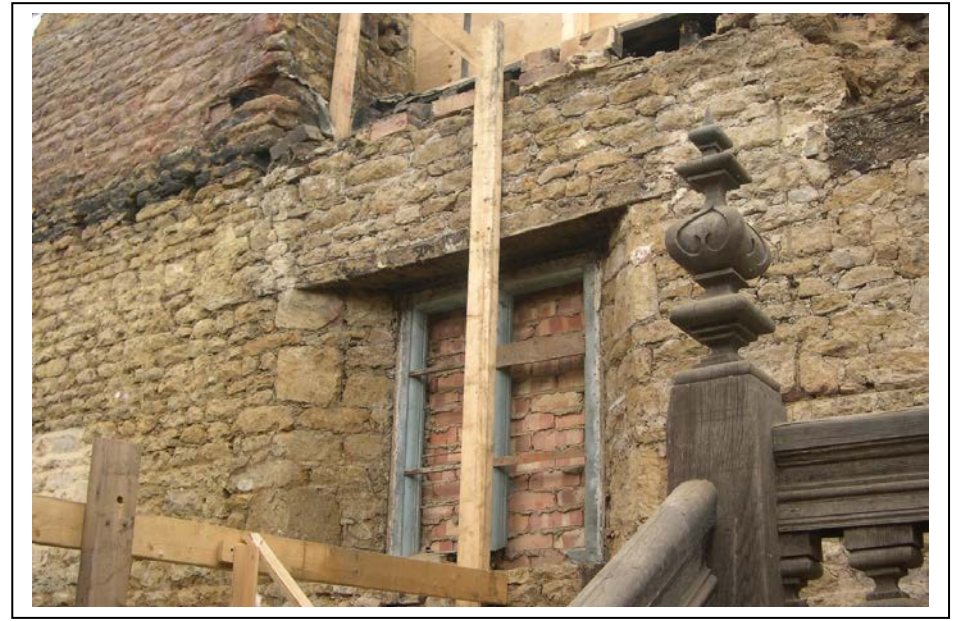
Plate 9: Location of window (after stripping) at the top of landing.
