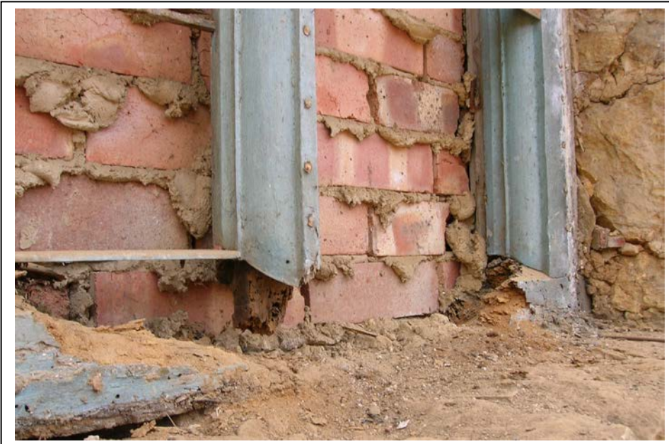
Plate 10: View east - detail of decay in lower element of window frame.
