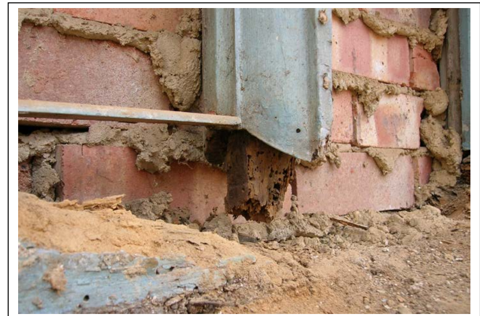
Plate 11: Detail of decay in lower element of window frame.
