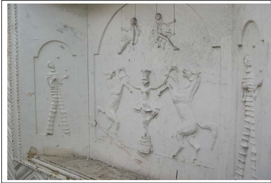
Plate 5: View north - Fibrous decorative plaster within the bay on Landing 2.6.
