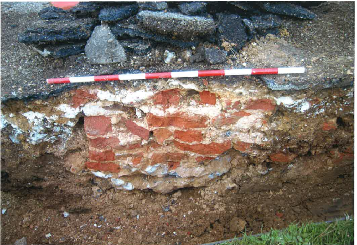
Plate 10: Trench 4; wall 127 in section after breaking through, looking west
