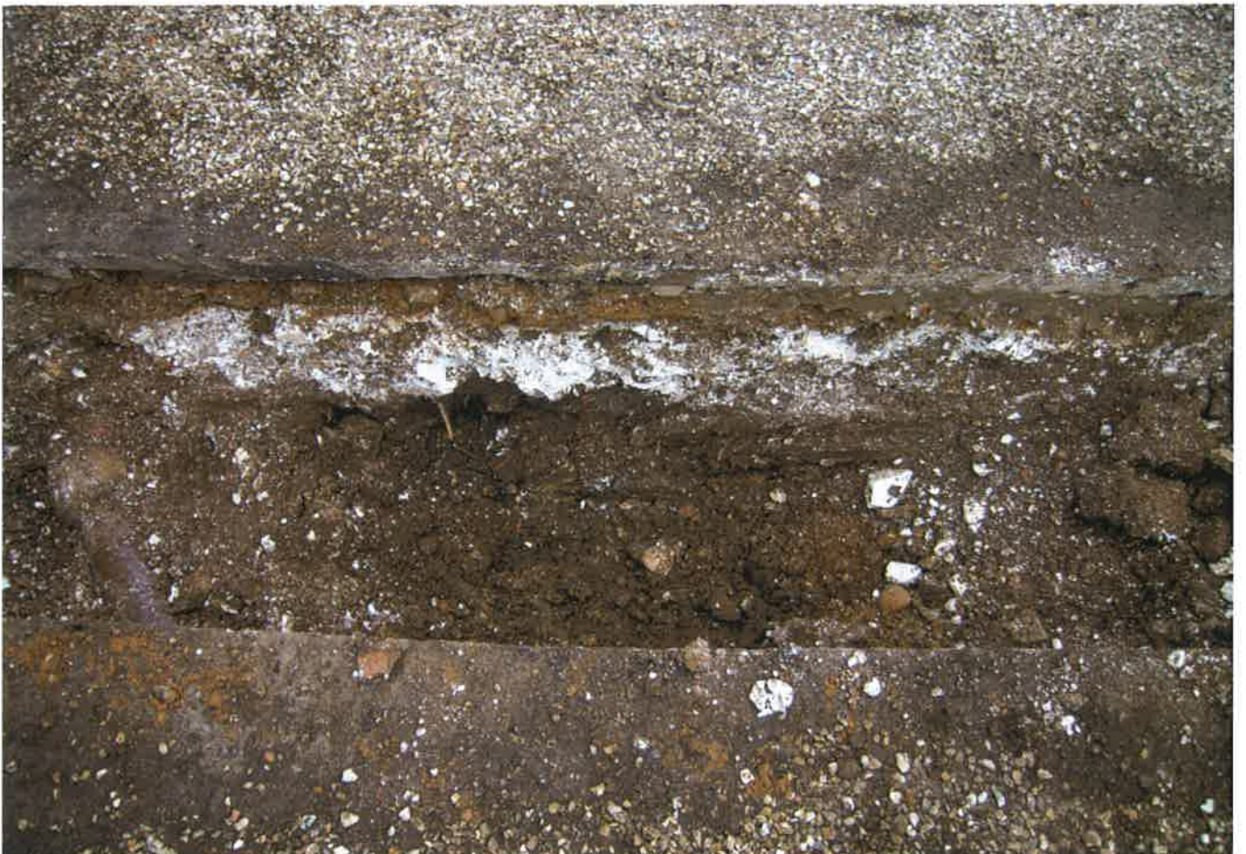
Plate 4: Trench 3; looking north-east
