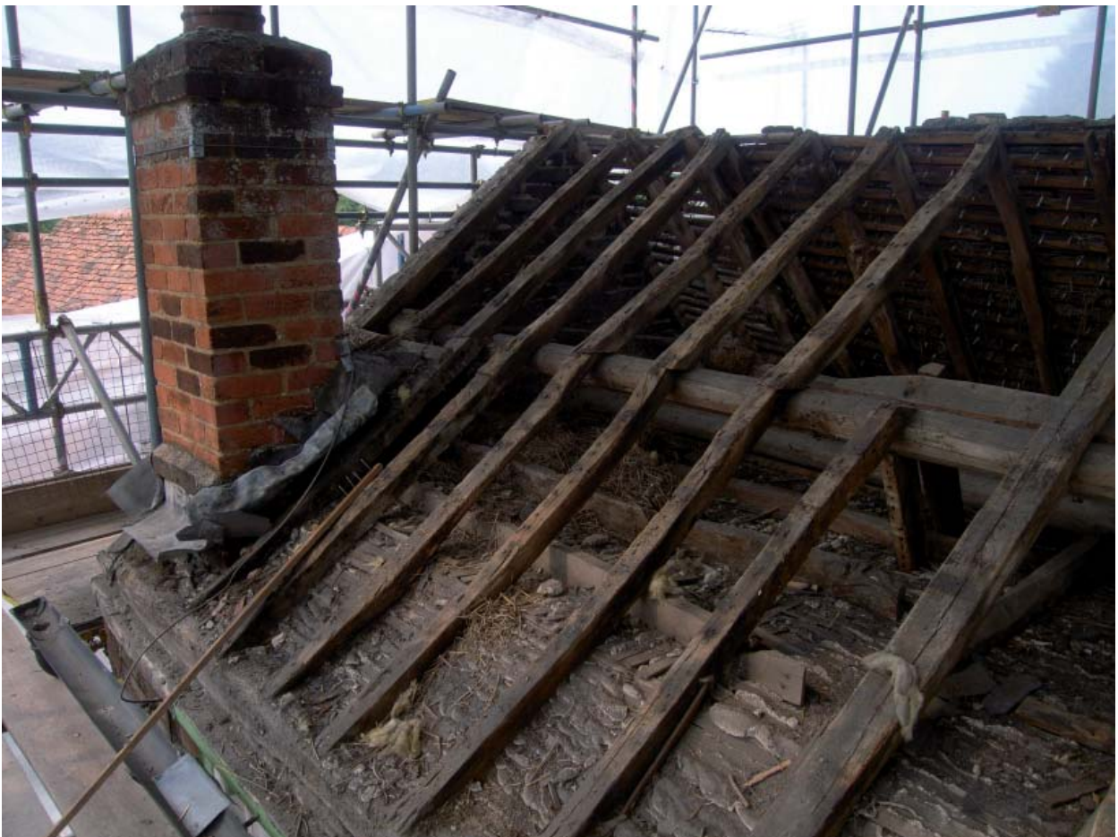
Plate 12: Re-profiled east slope of Bay 1 at south end of building
