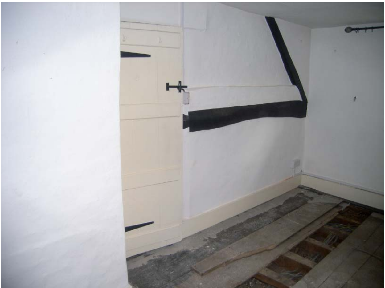
Plate 36: Truss at original north end of cottage (between Bays 3 and 4)
