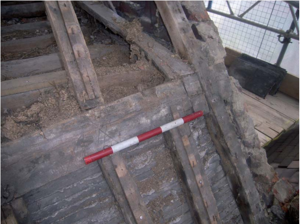
Plate 11: Purlin/butt rafter in west slope of Bay 1 at south end of building
