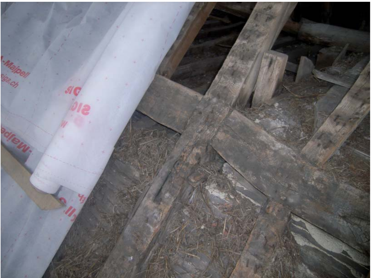
Plate 26: Butt purlin in west slope
