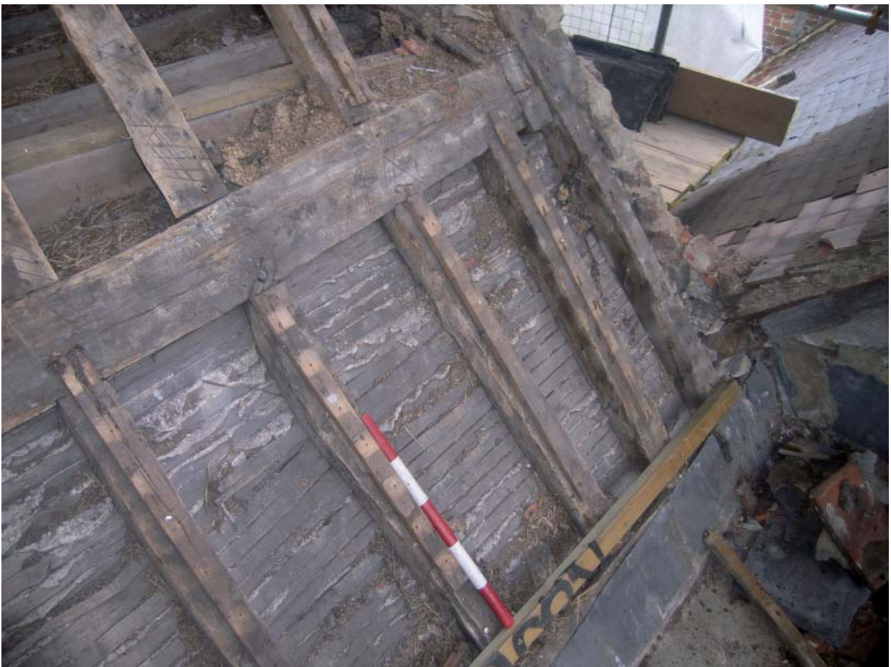
Plate 10: West slope of Bay 1 at south end of building
