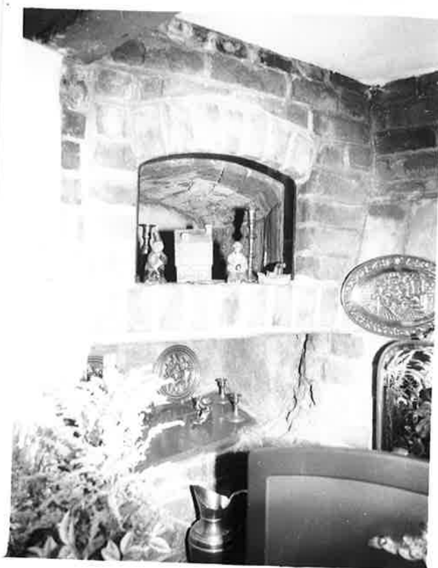
FIREPLACE, LIVING ROOM D. NO. 40. DETAIL OF BREAD OVEN. R 212 N 15.
