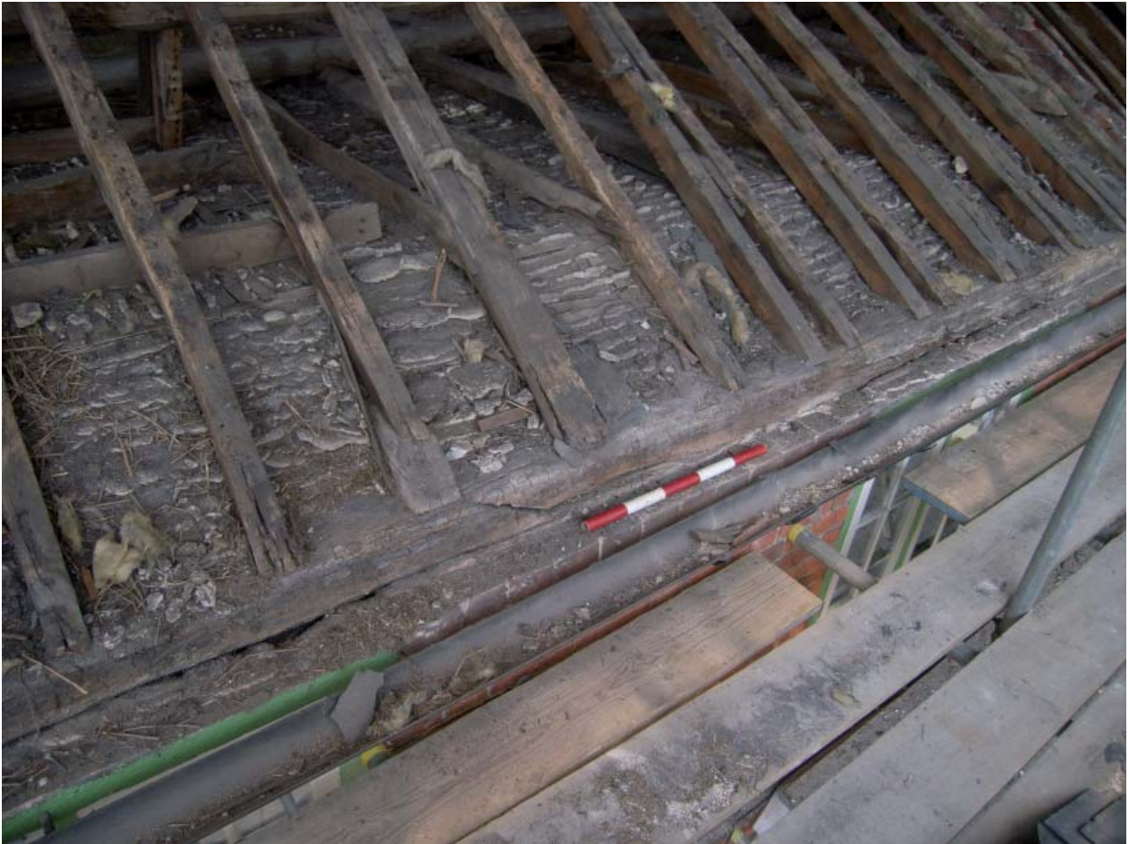
Plate 17: Wall plate detail in Bay 2
