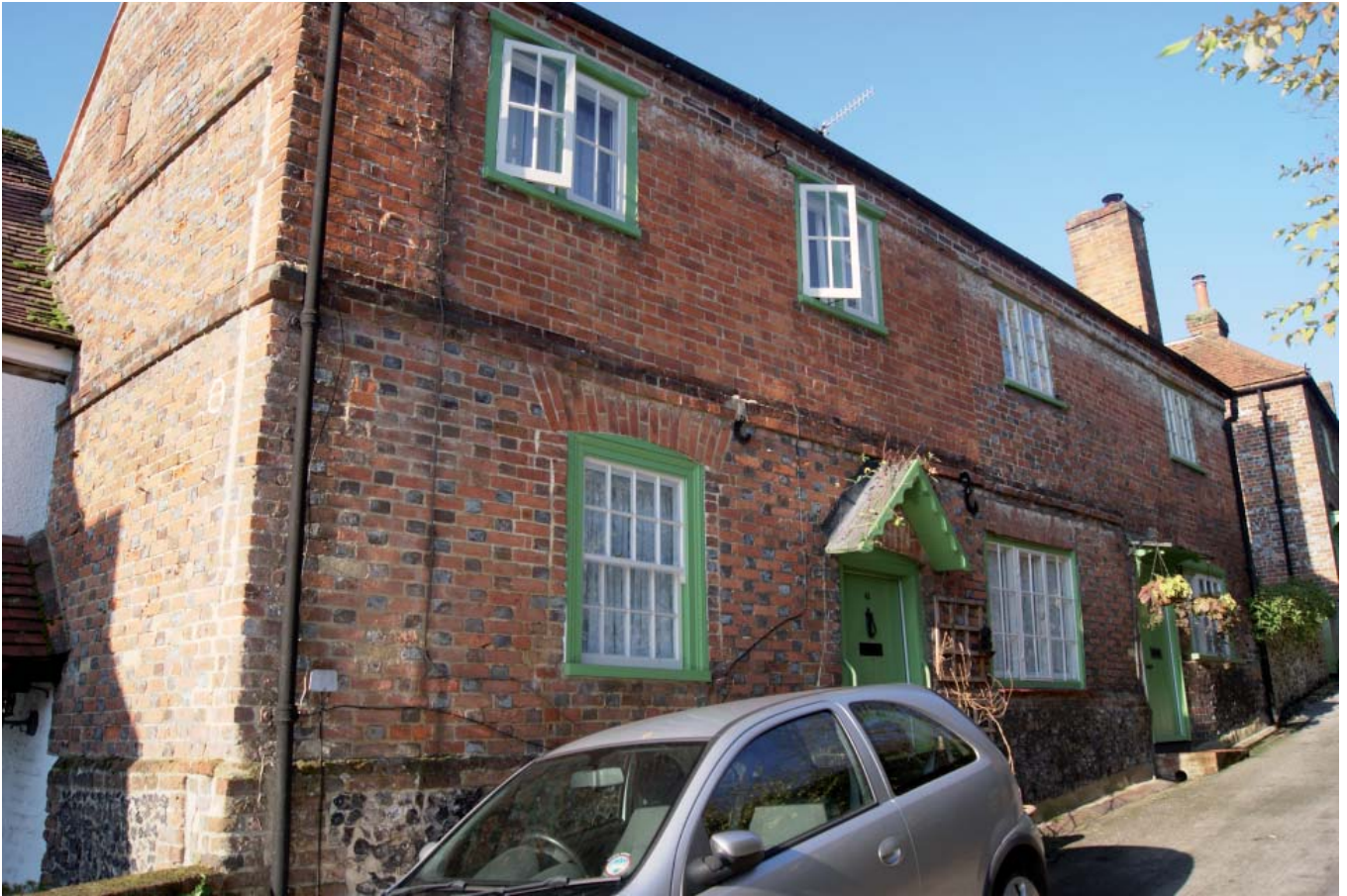
Plate 1: East elevation facing Church Lane (after conservation work)
