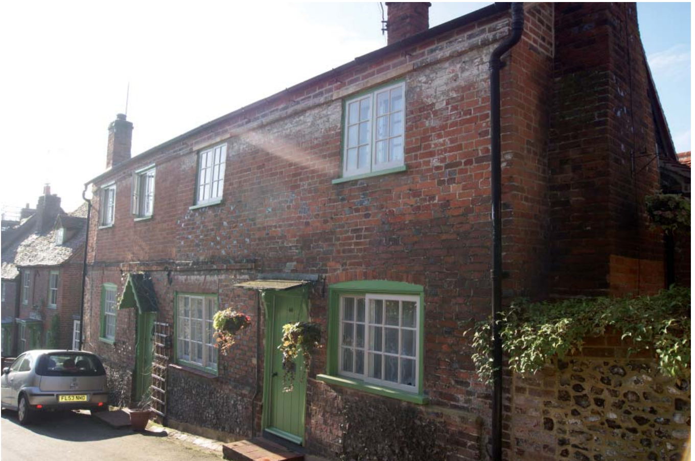
Plate 2: East elevation from north-east (after conservation work)
