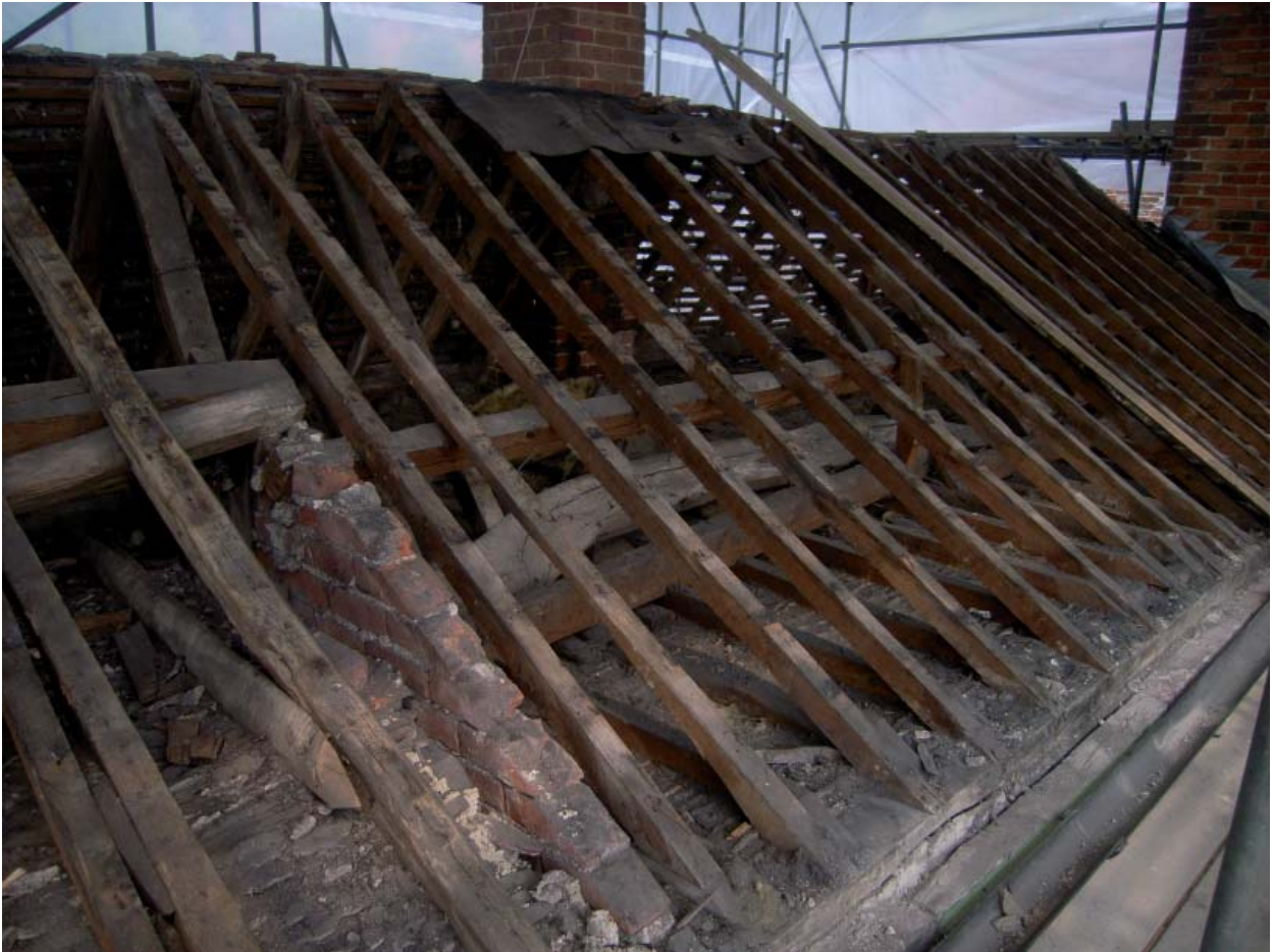
Plate 19: East slope of Bay 3 to north of central line of building
