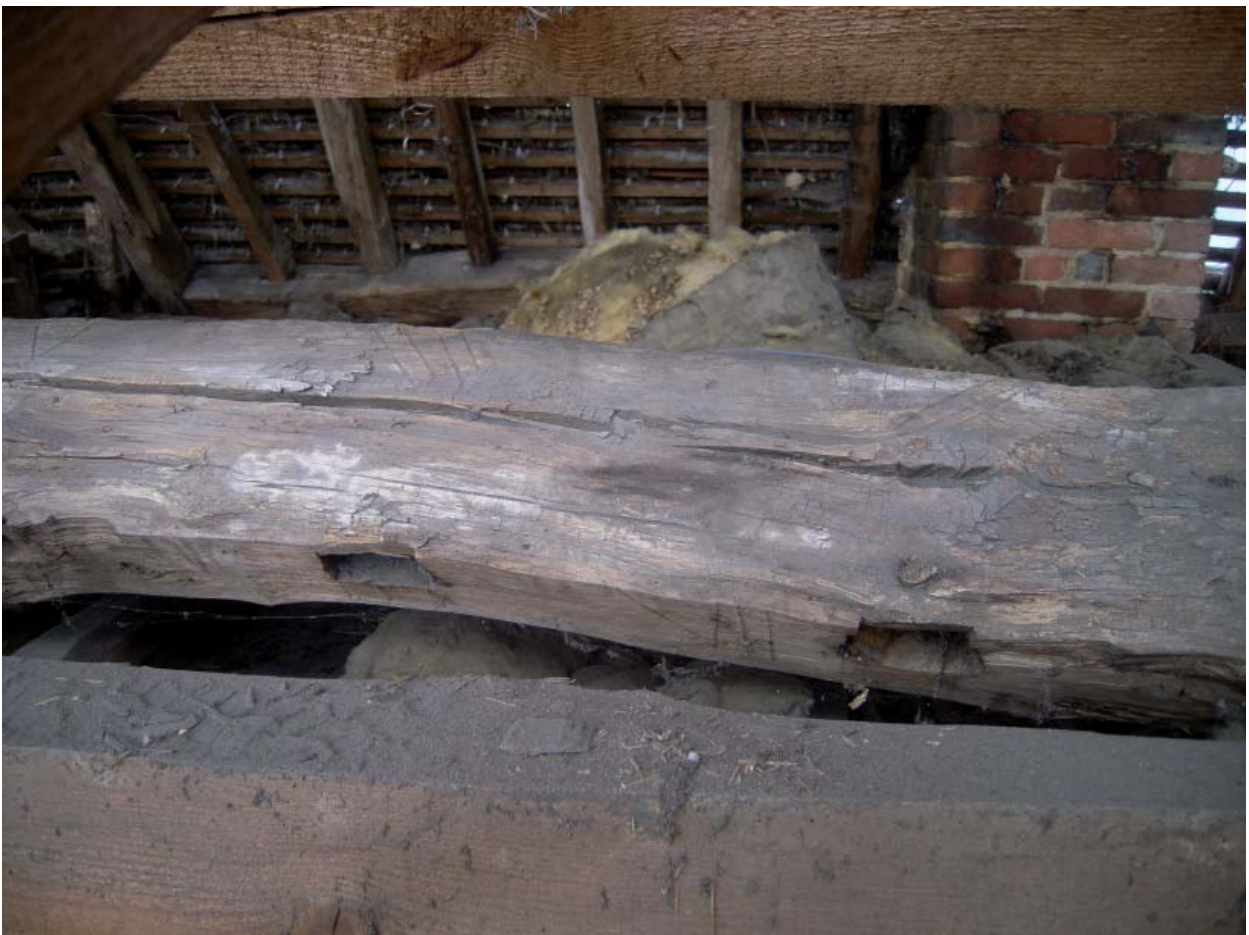
Plate 24: Empty mortises in purlin from former abutting rafters (Bay 3 from south)
