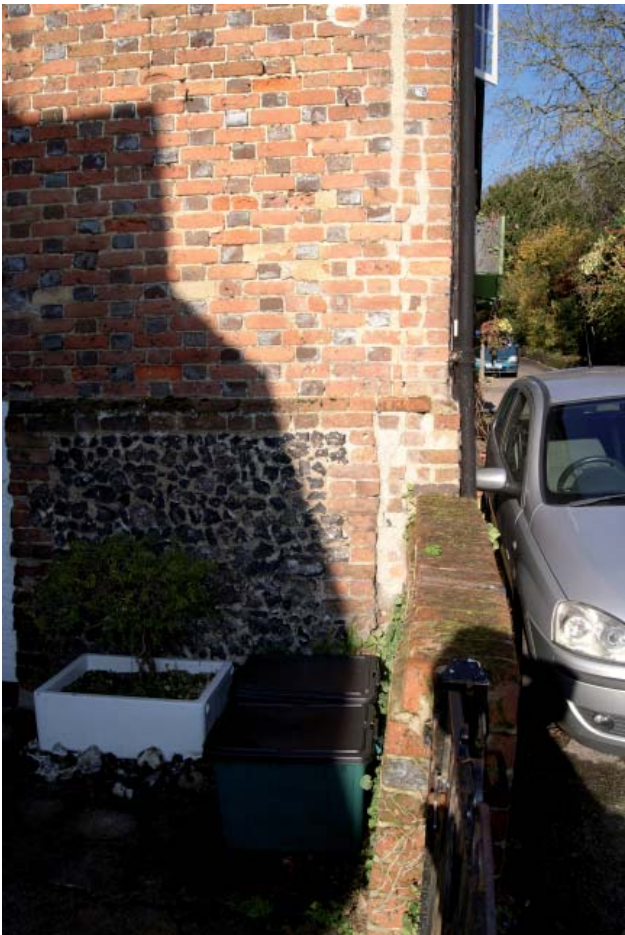
Plate 4: Lower part of south elevation
