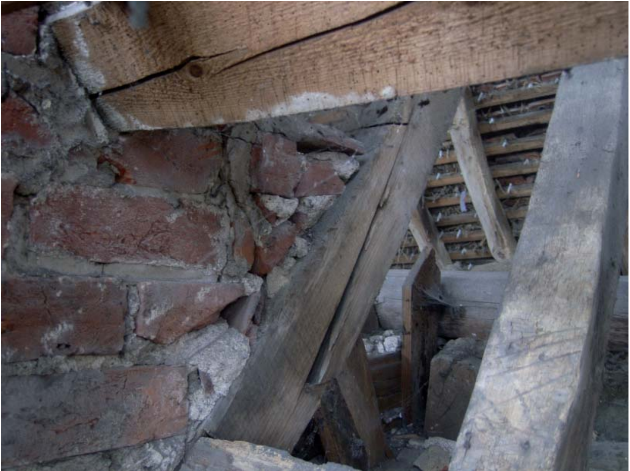
Plate 21: Cruck blade detail in east slope at centre of building
