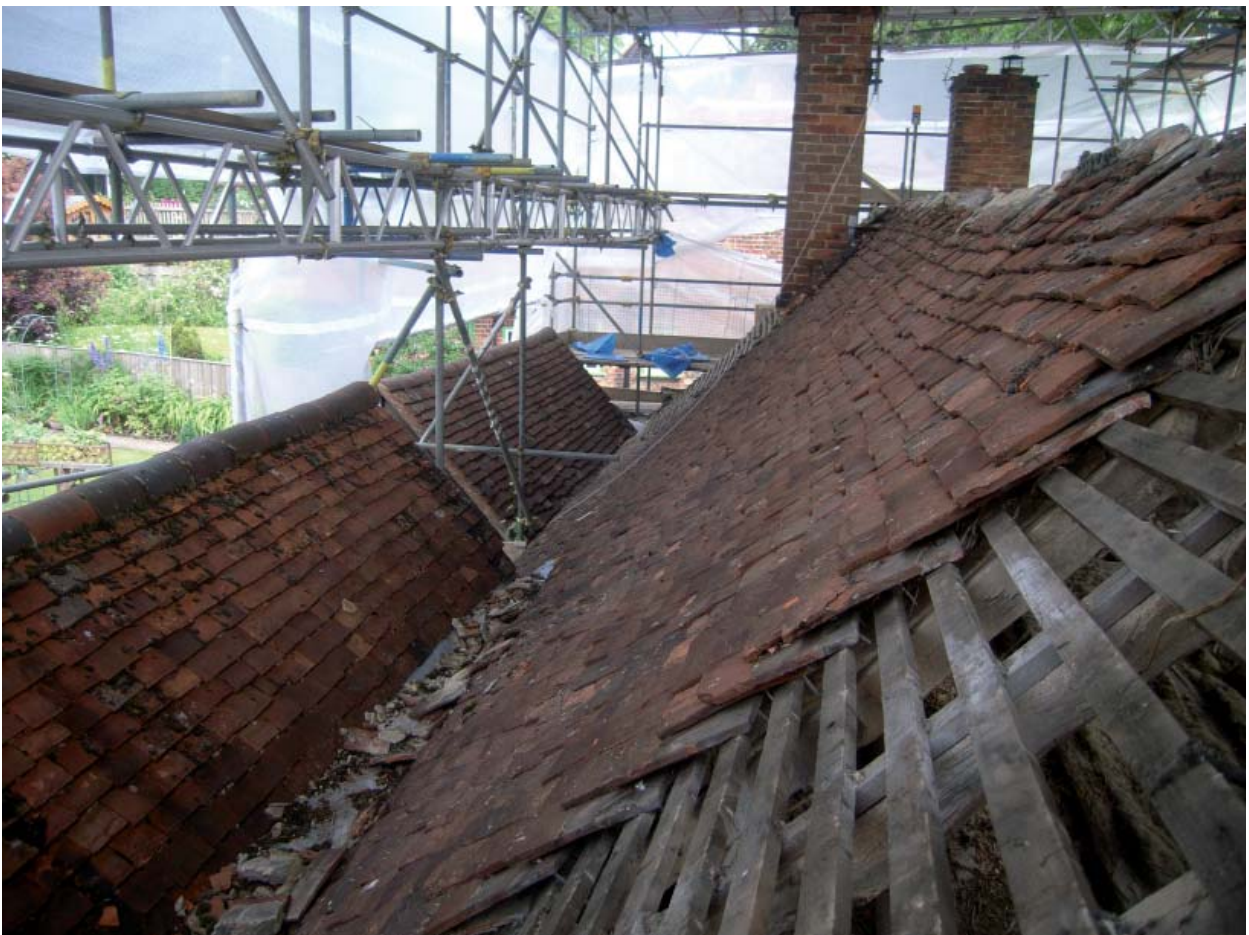
Plate 32: General view of west slope looking north
