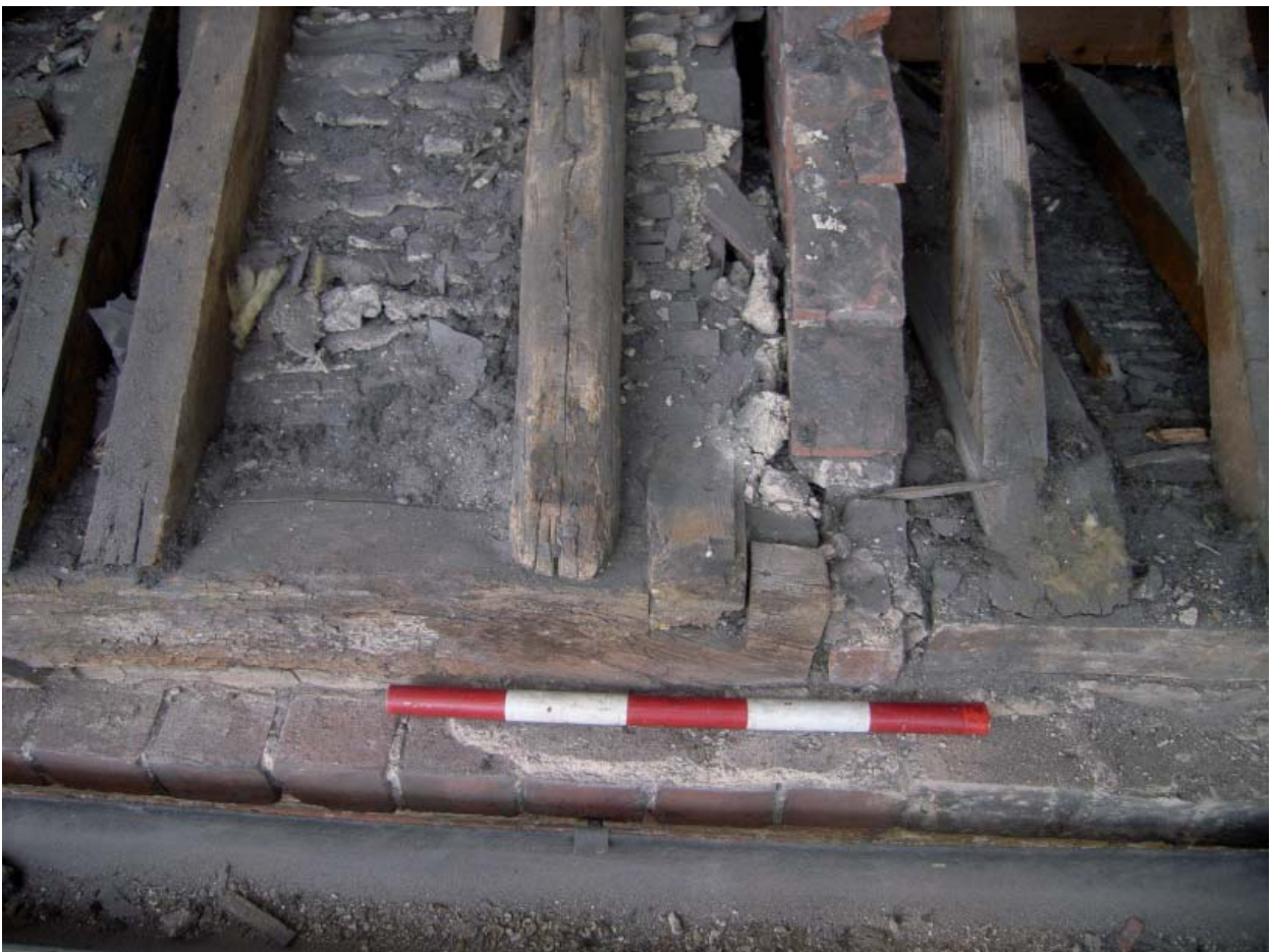
Plate 18: Detail of east slope at centre of building
