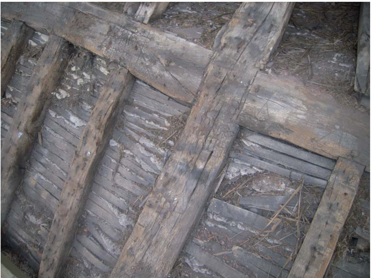
Plate 14: Detail in west slope
