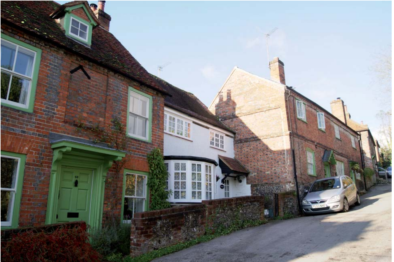
Plate 3: View up Church Lane towards No.40-41
