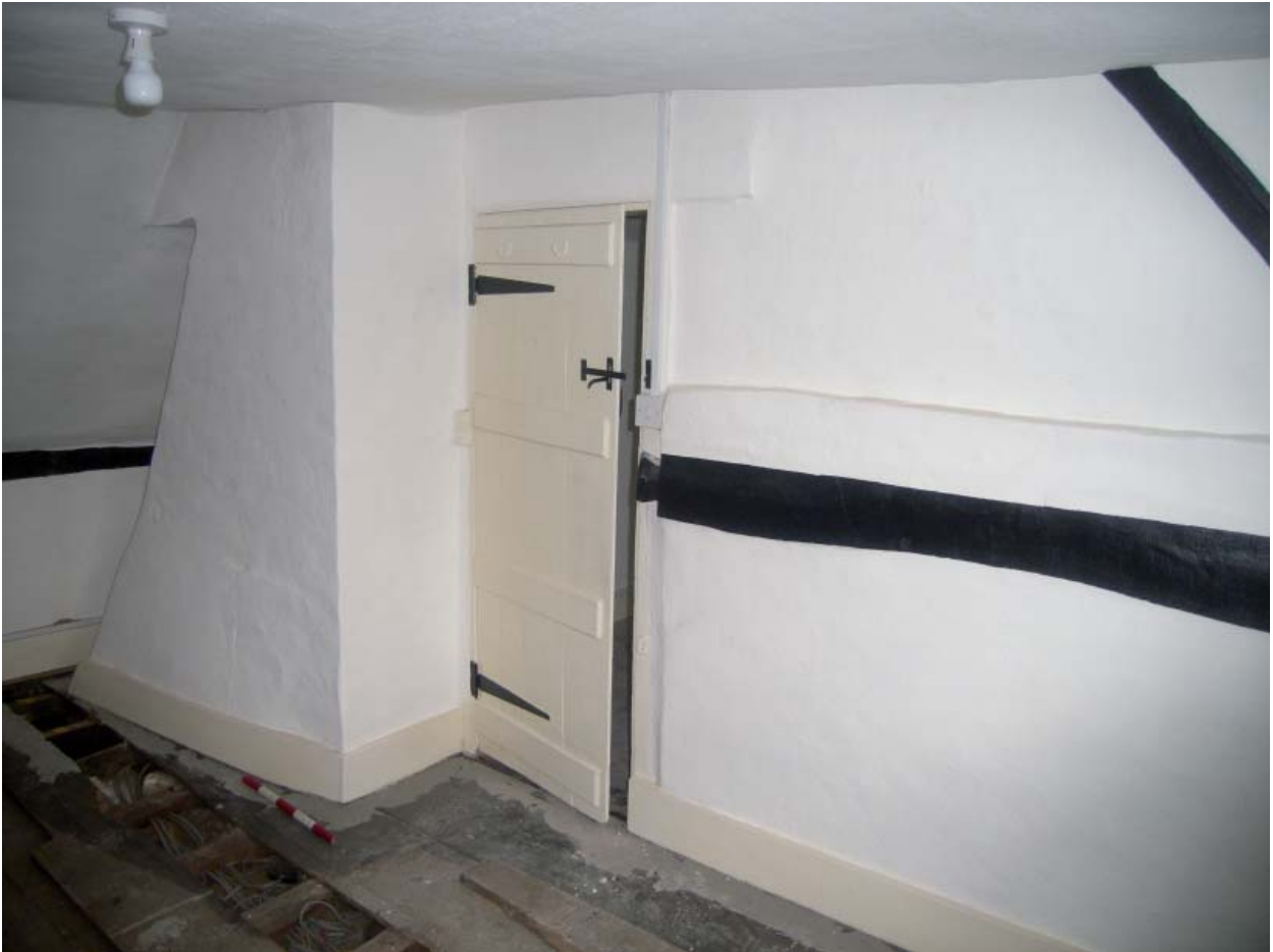
Plate 35: Truss at original north end of cottage (between Bays 3 and 4)
