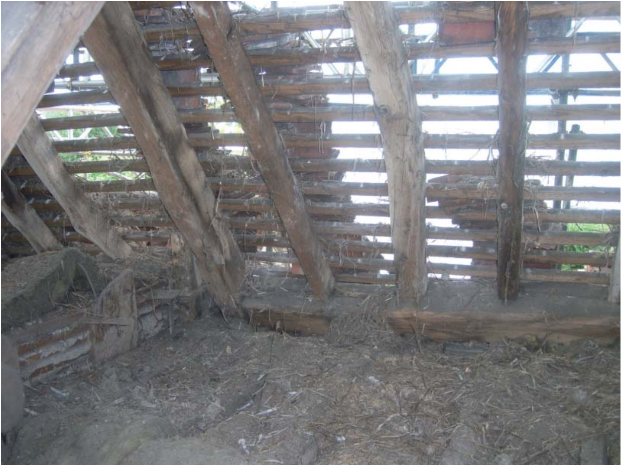
Plate 25: West slope of Bay 3 from inside roof space
