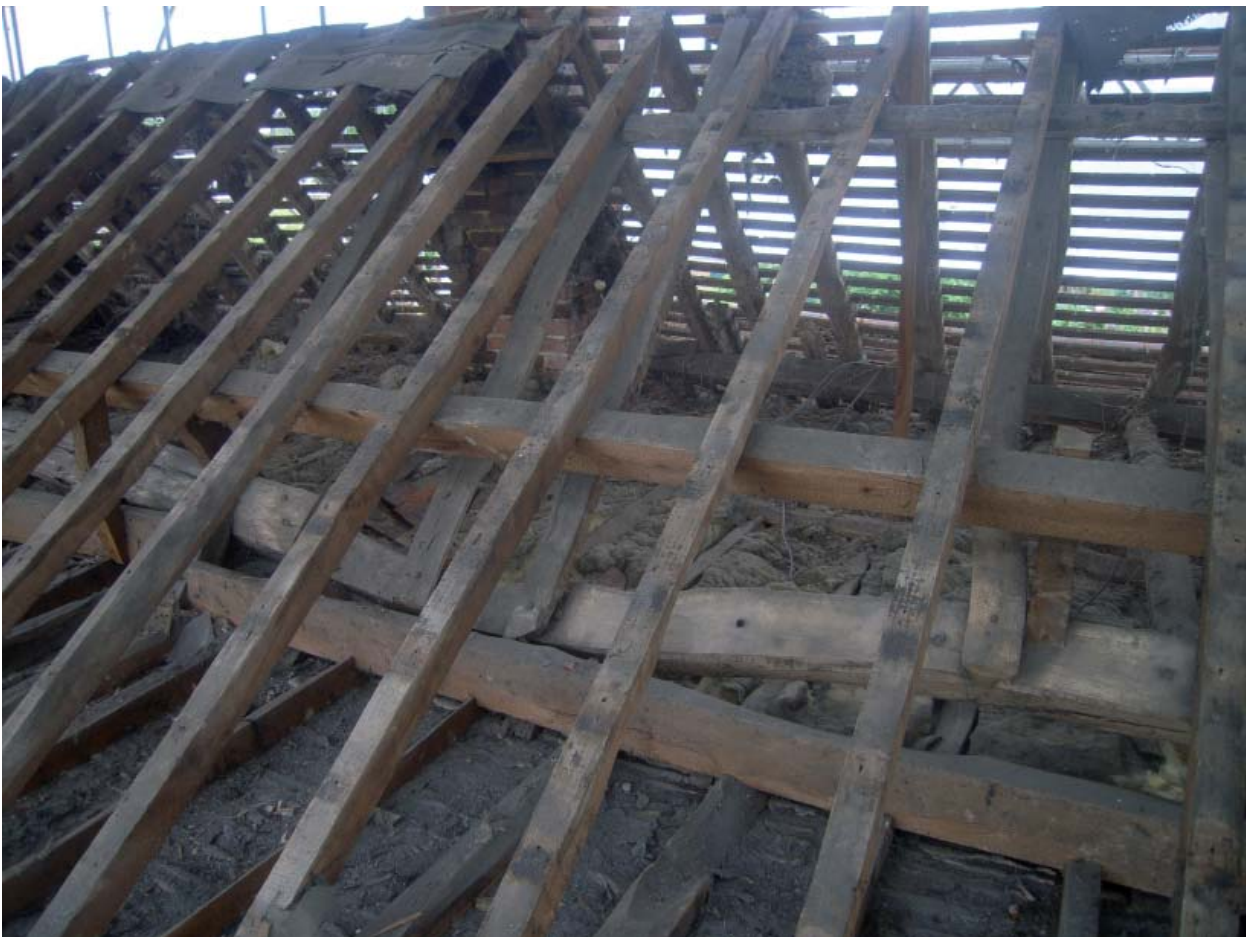
Plate 28: East slope of northernmost bay with earlier purlin below secondary rafters
