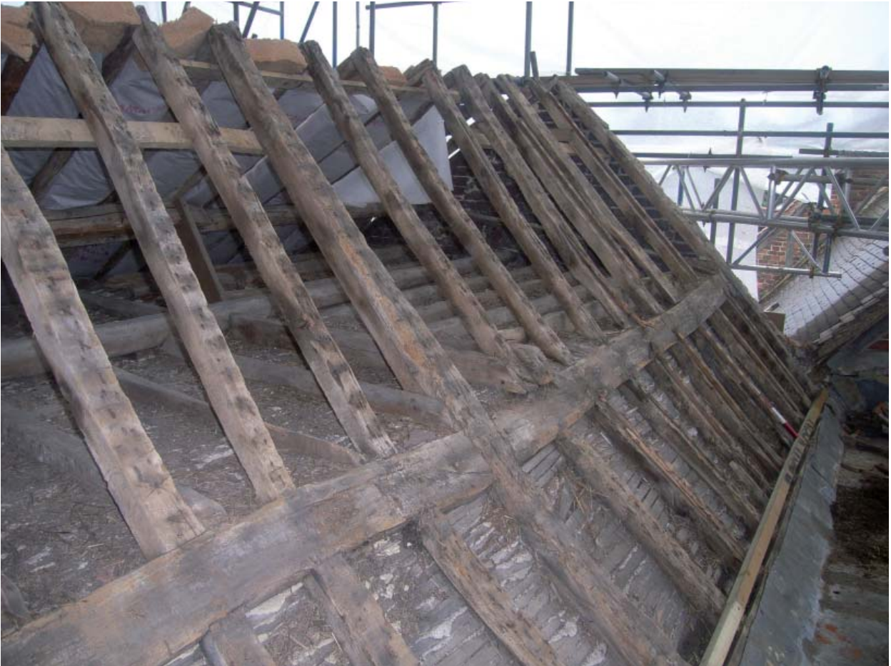
Plate 9: West slope of Bay 1 at south end of building
