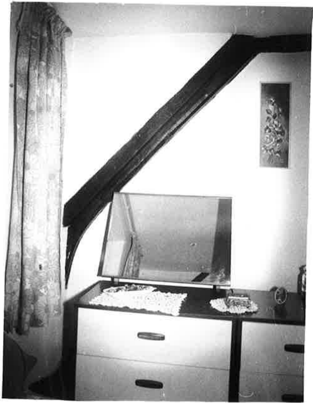
DETAIL OF CRUCK TRUSS, BEDROOM F, NO. 40 LOOKING SOUTH-EAST R212 N18
