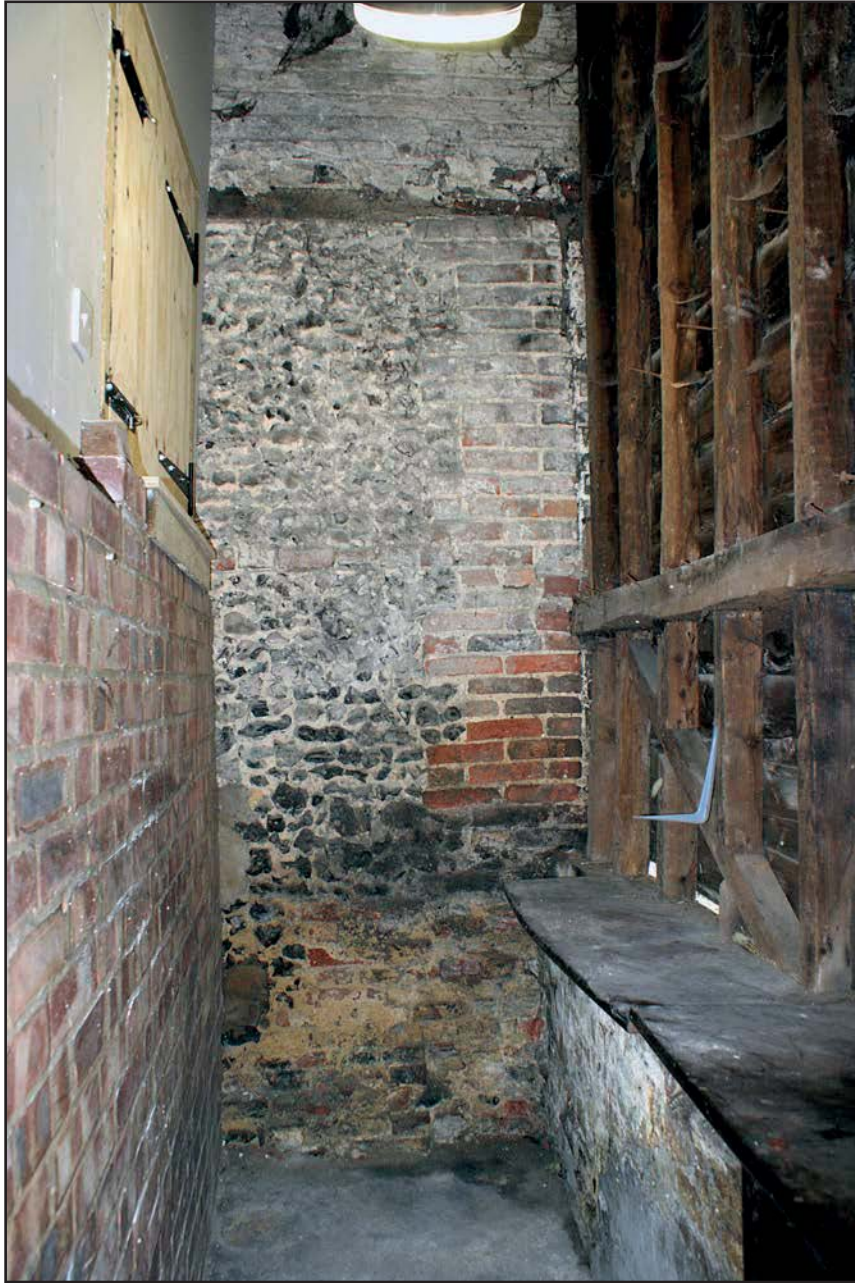
Plate 25: View of flint party wall between no 50 and the extension of no 49
