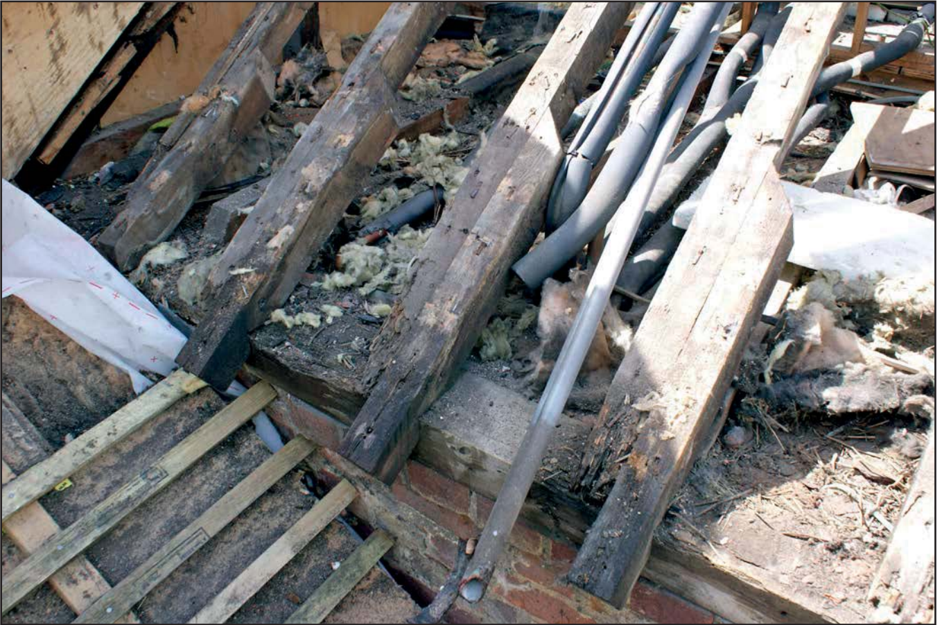
Plate 23: Detail of rear extension roof no. 49
