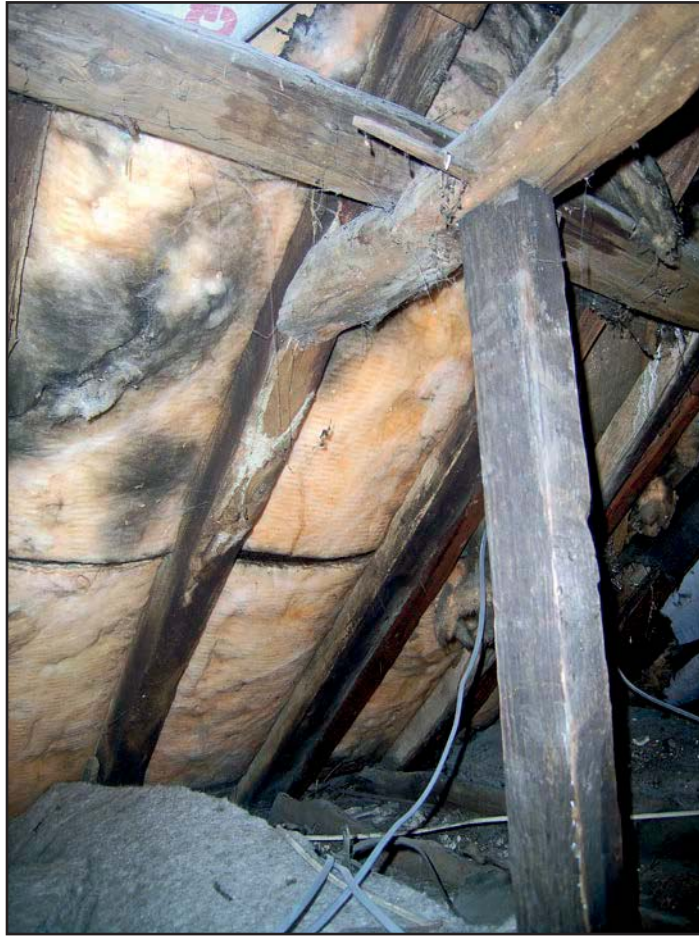
Plate 21: Detail of pegged truss no. 49
