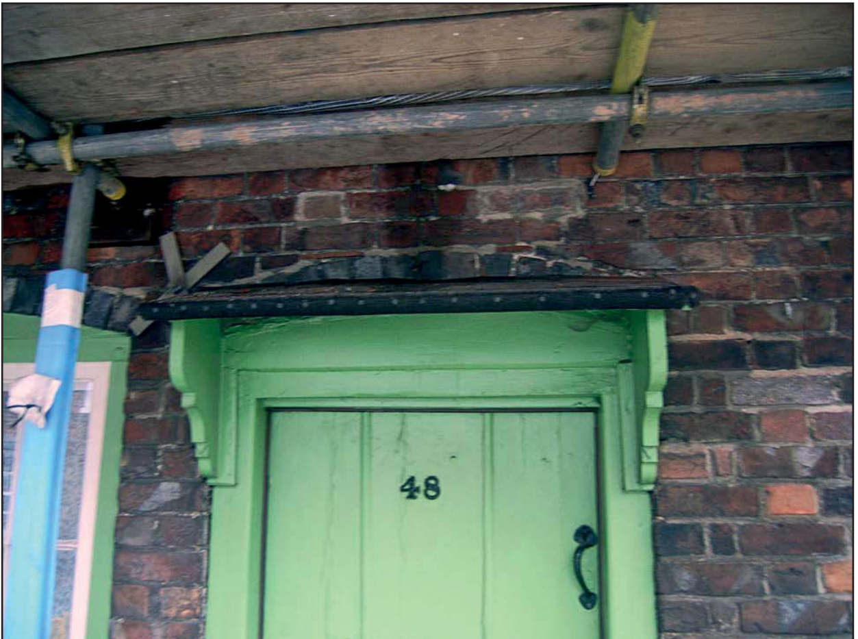
Plate 2: Detail of arch lintel no. 48
