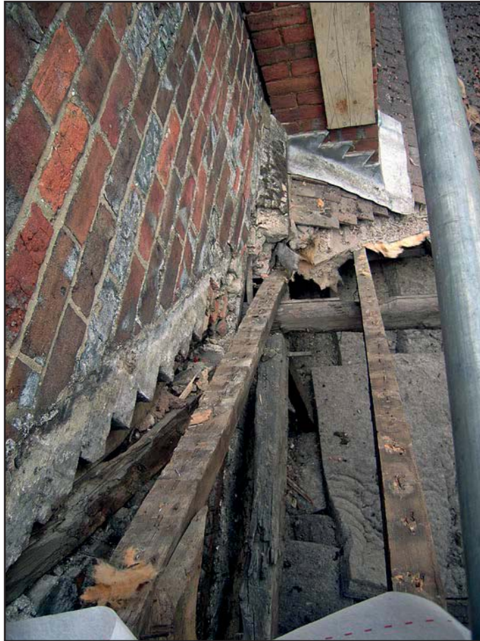
Plate 13: Detail of truss adjacent to gable wall between 49 and 50 (looking north)
