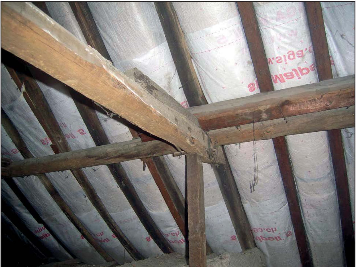
Plate 20: Detail of double purlin no. 49
