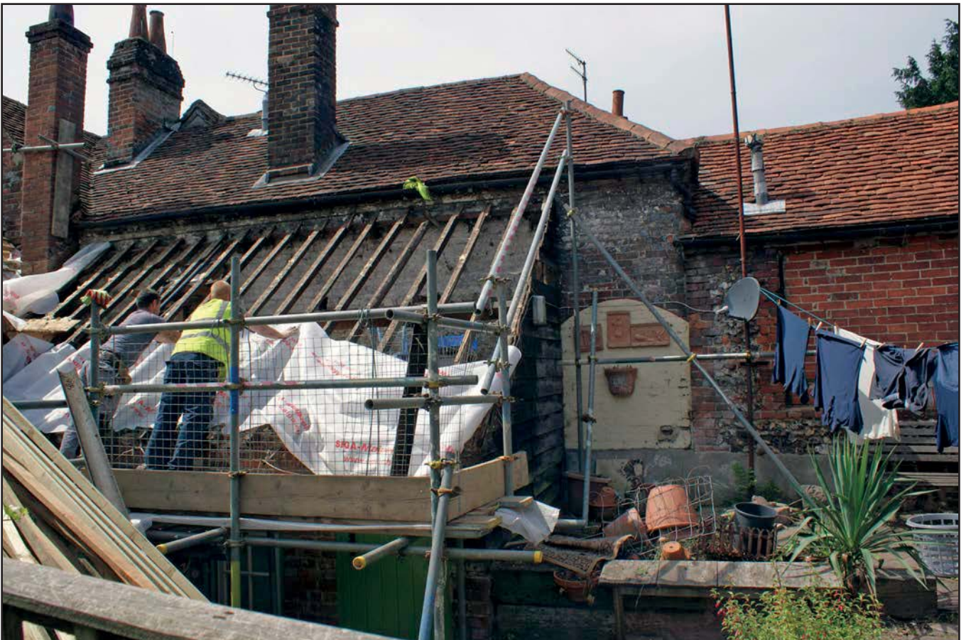
Plate 24: View of rear extension roof no. 49
