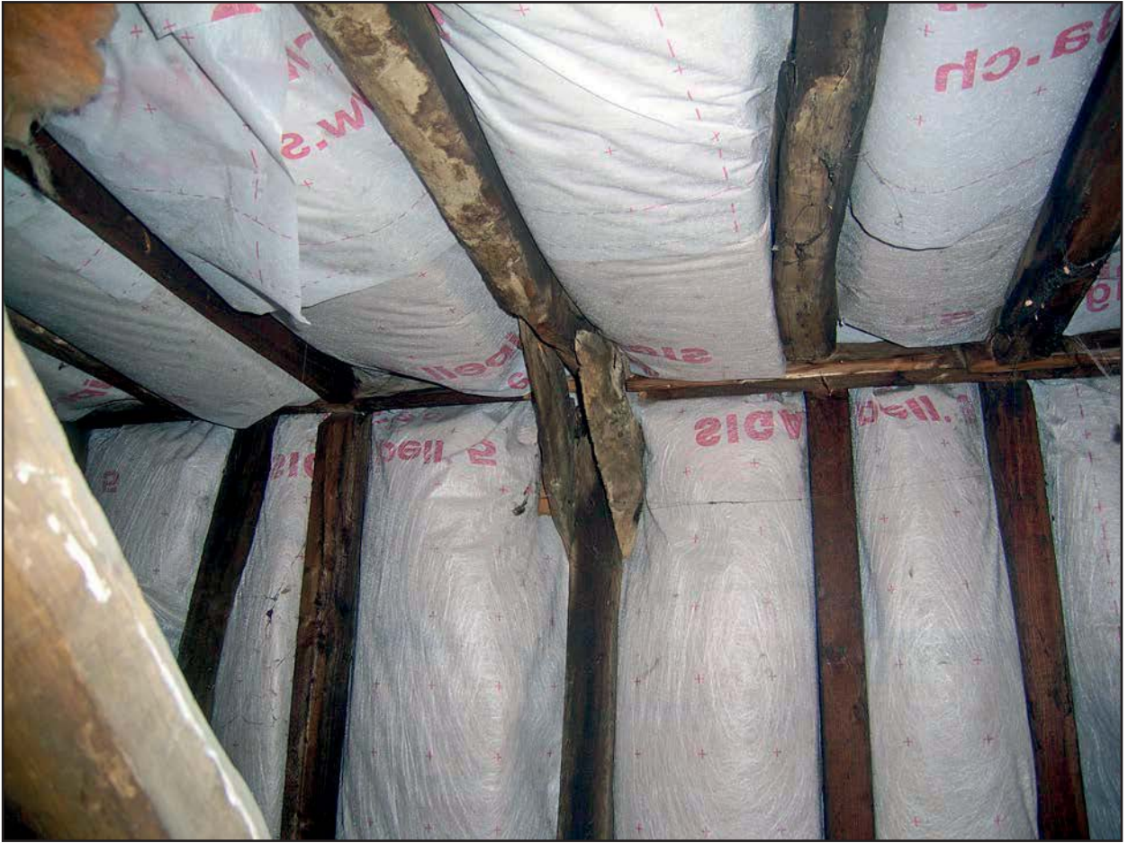
Plate 19: Detail of roof no 49
