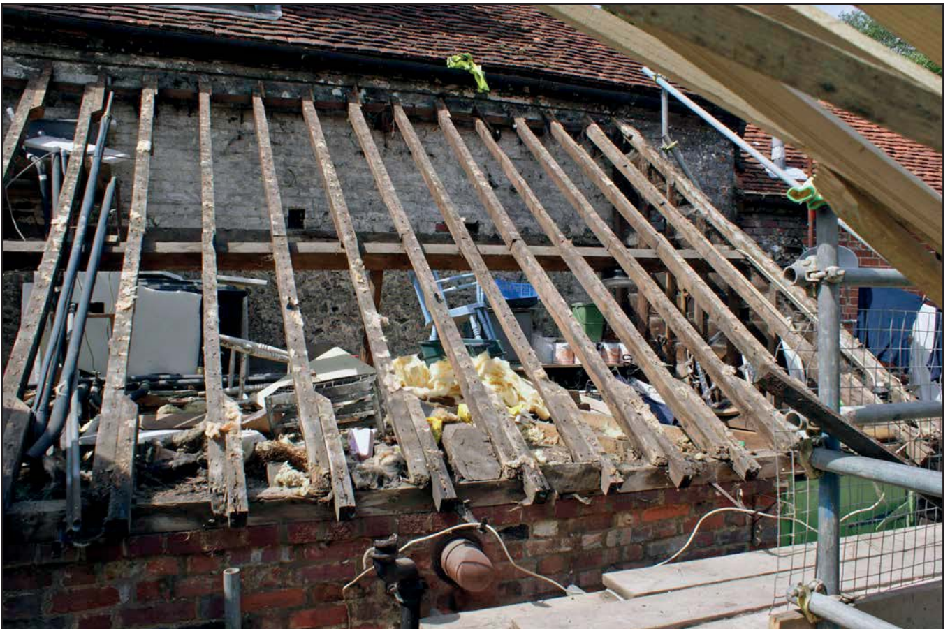
Plate 22: View of rear extension roof no. 49
