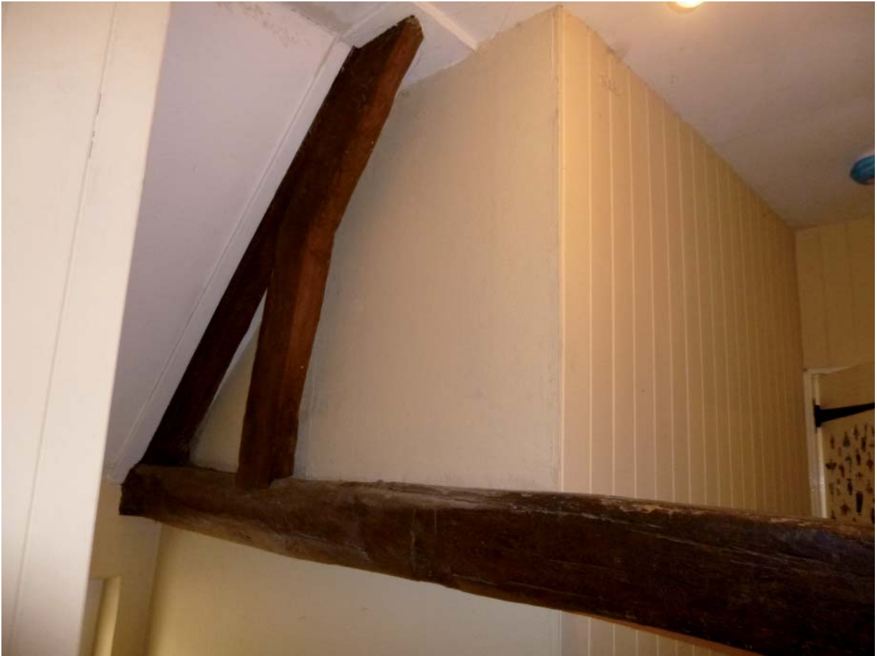
Plate 3: Cranked principal of the central truss seen from the landing
