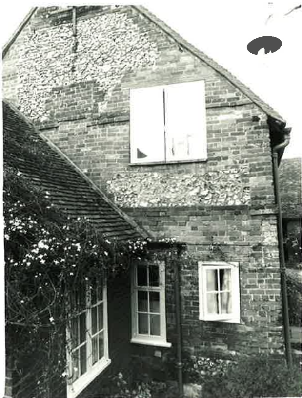
EAST GABLE, VIEWED FROM NORTH-EAST R 216 N 34.
