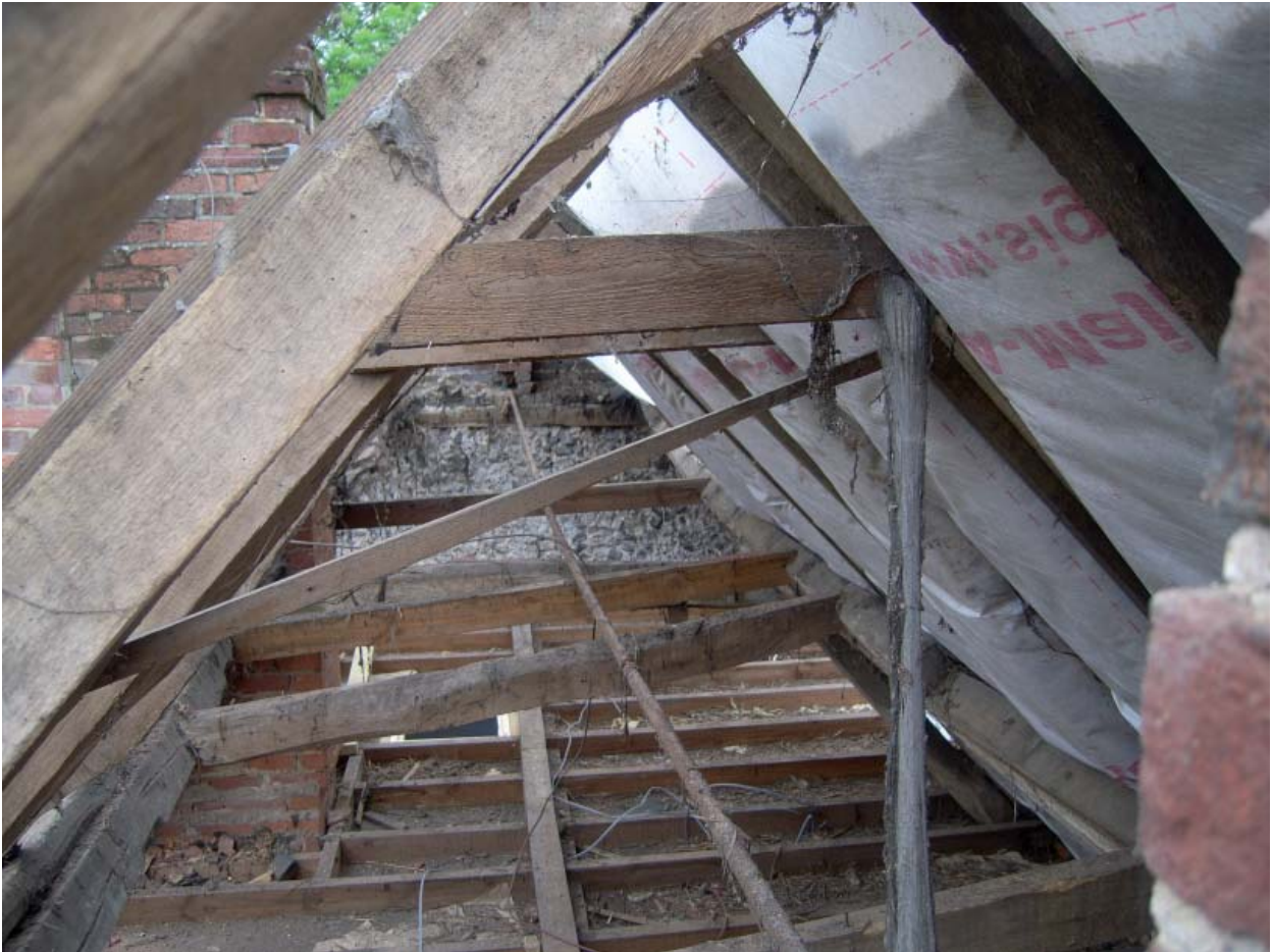
Plate 19: Braces between upper purlins
