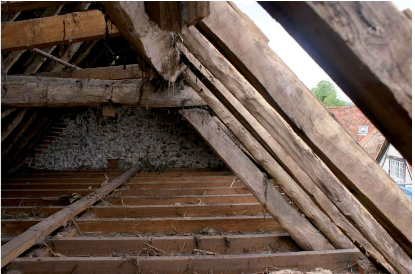
Plate 4: Collar and cranked principal of central truss (courtesy of Gary Marshall)
