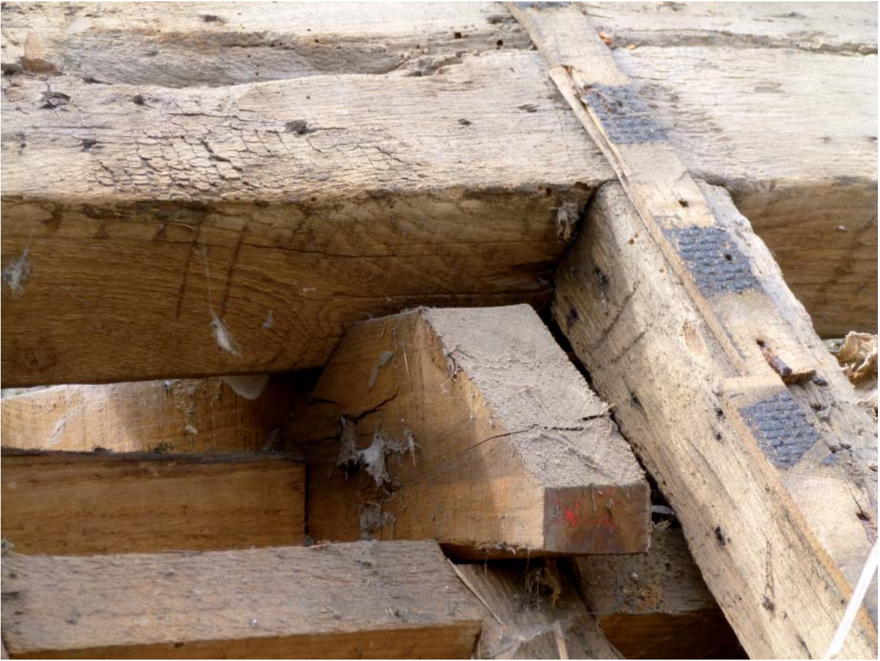
Plate 21: Carpenter's Marks on north slope
