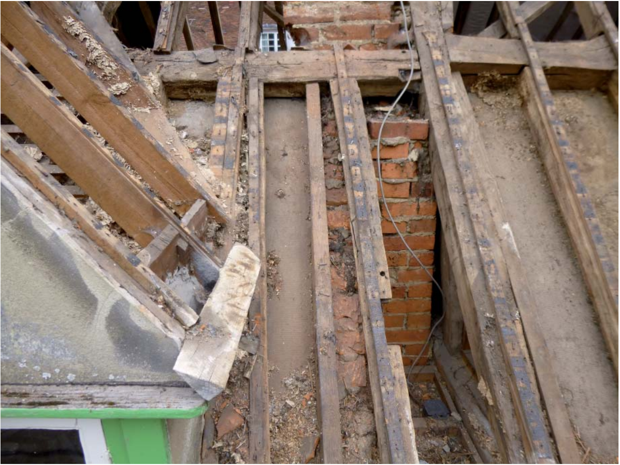
Plate 9: One of the few reused portions of rafter
