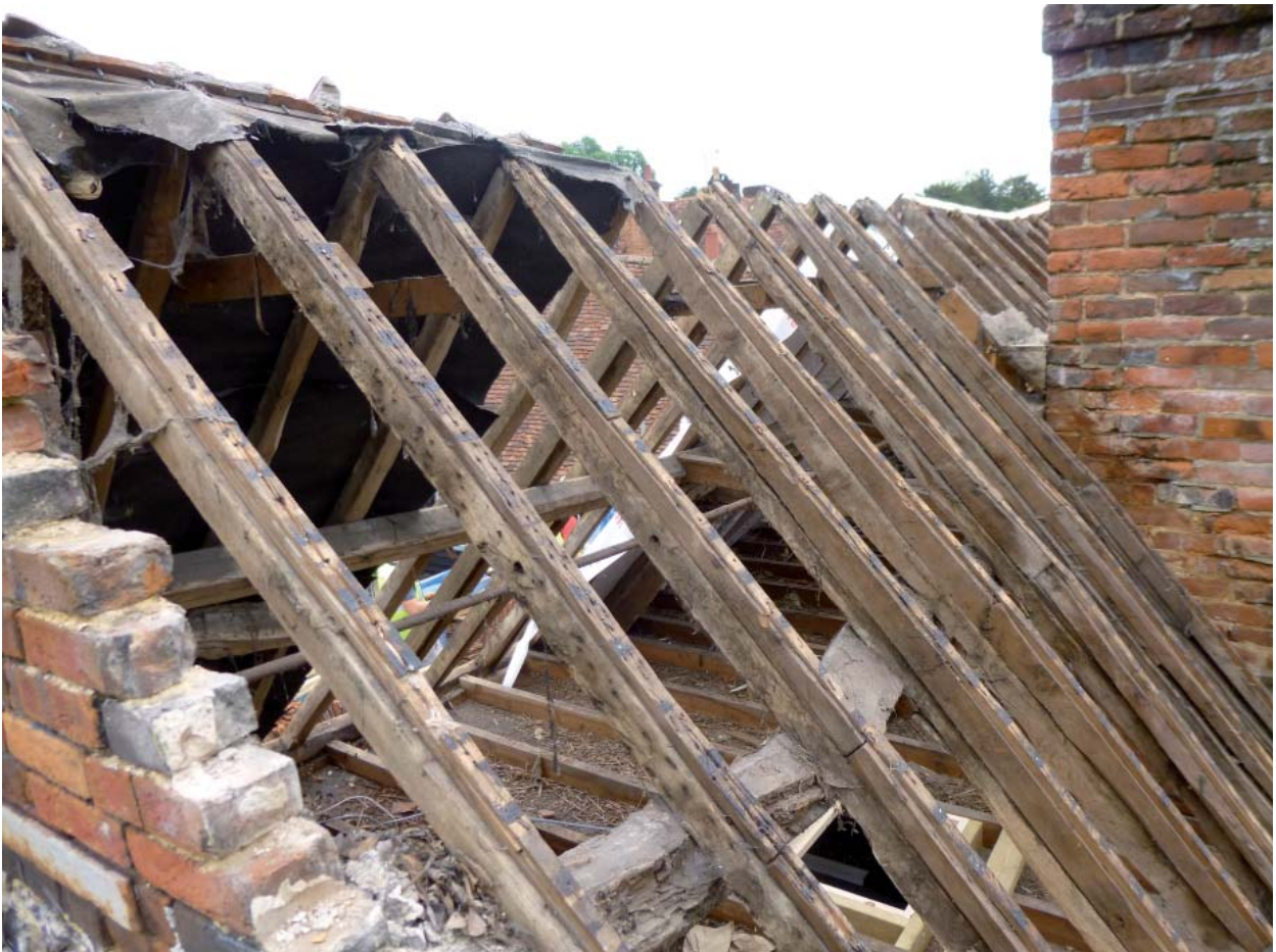
Plate 8: Packing to rafters on the south slope
