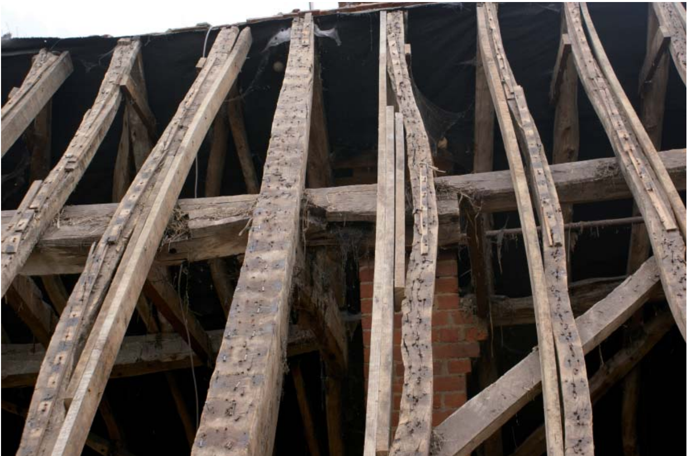
Plate 12: Scarf of north slope upper purlin (courtesy of Gary Marshall)
