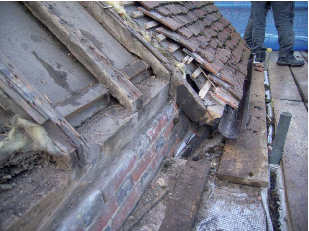
Plate 6: Rafter ends, wall plate and sprockets
