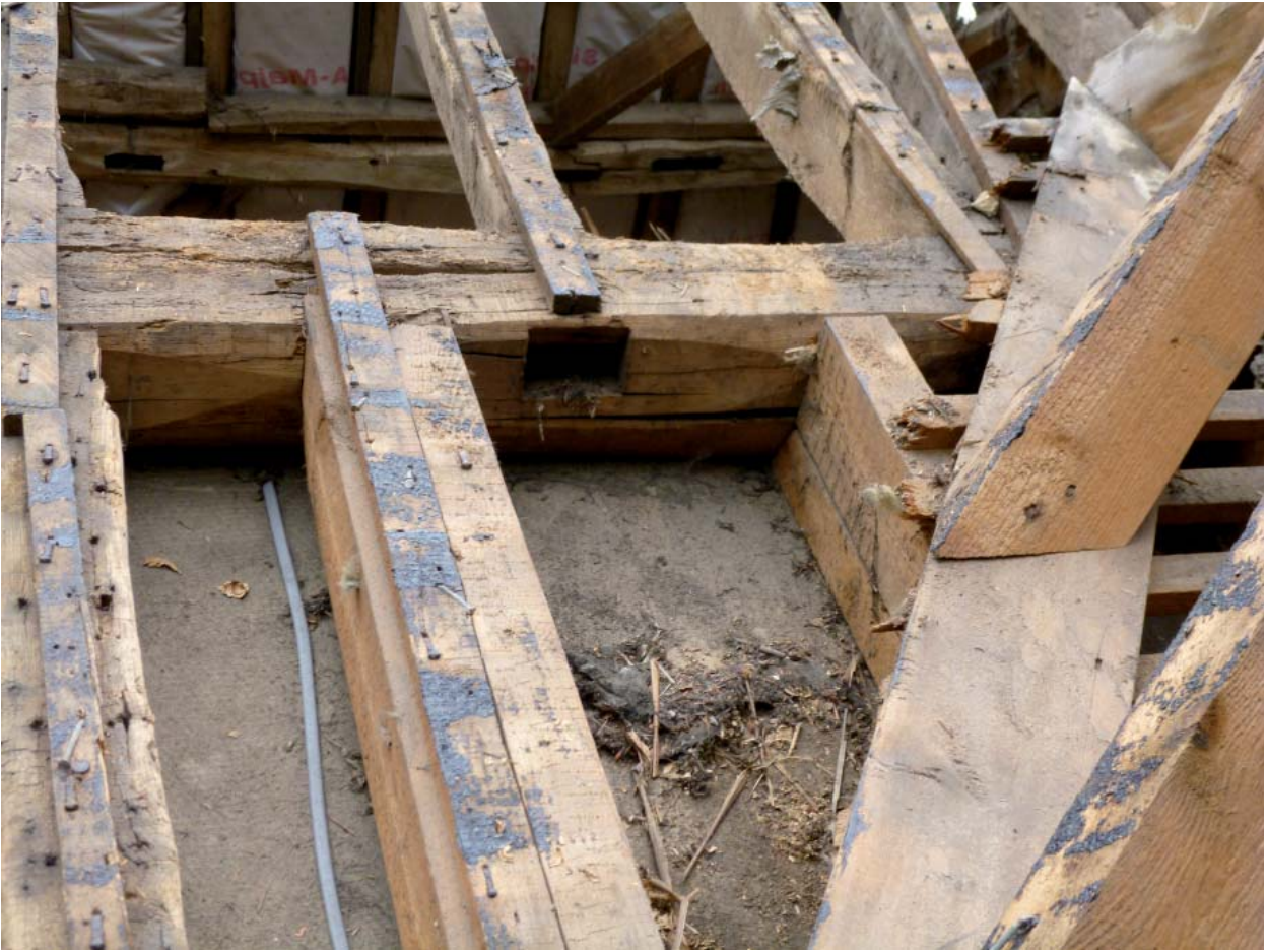
Plate 7: Empty mortise behind easternmost dormer
