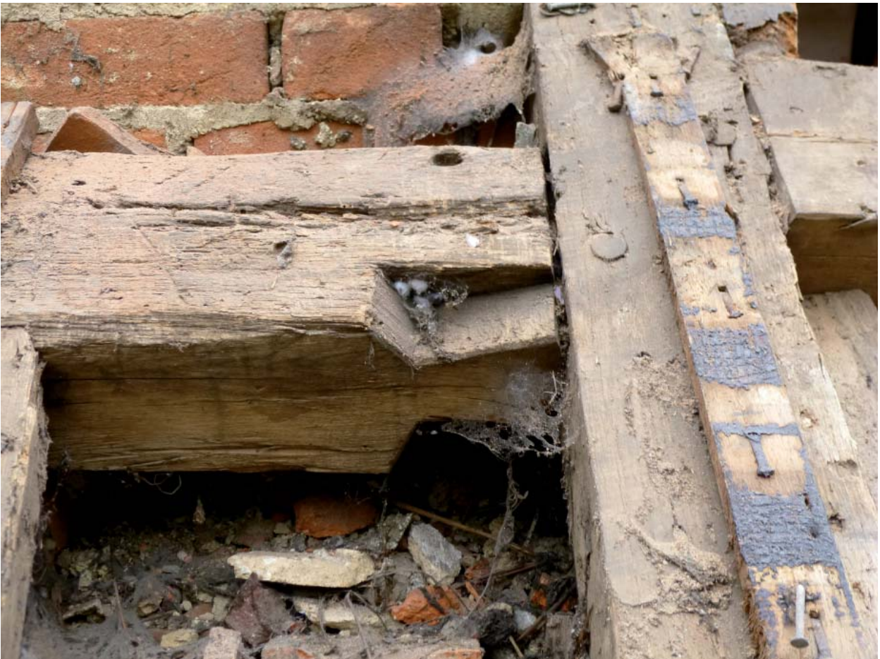
Plate 16: Dovetail from a former use of the south slope lower purlin
