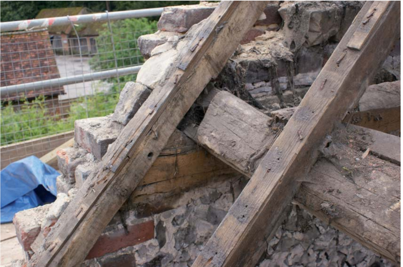
Plate 17: Dovetail from a former use of the north slope upper purlin (courtesy of Gary Marshall)
