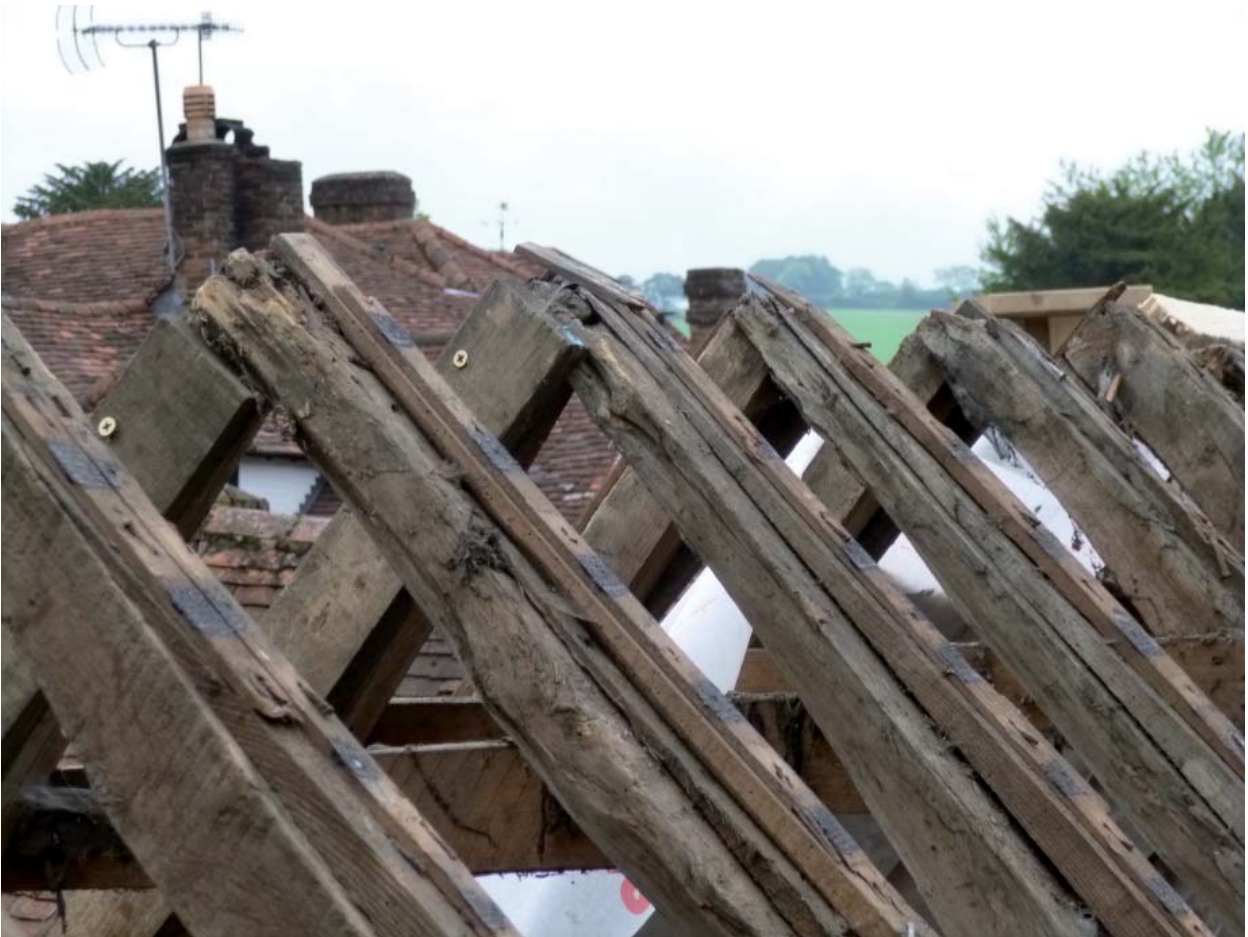
Plate 5: Apex joints and repairs
