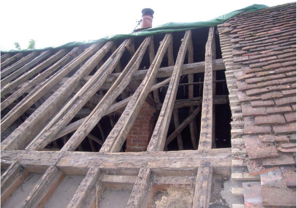
Plate 18: Windbraces
