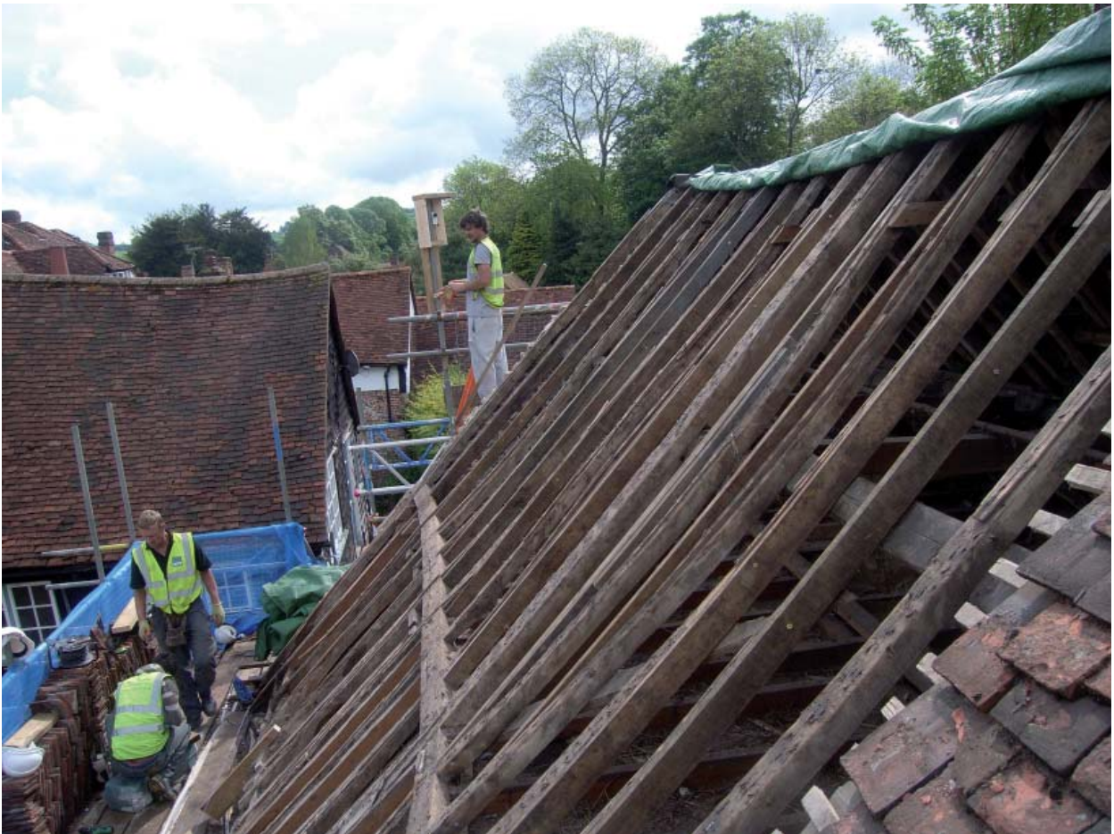
Plate 2: North slope of roof with unstripped area to the west
