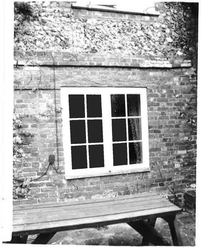
DETAIL OF BRICK INFILLING AROUND WINDOW F. R 216 N 33.
