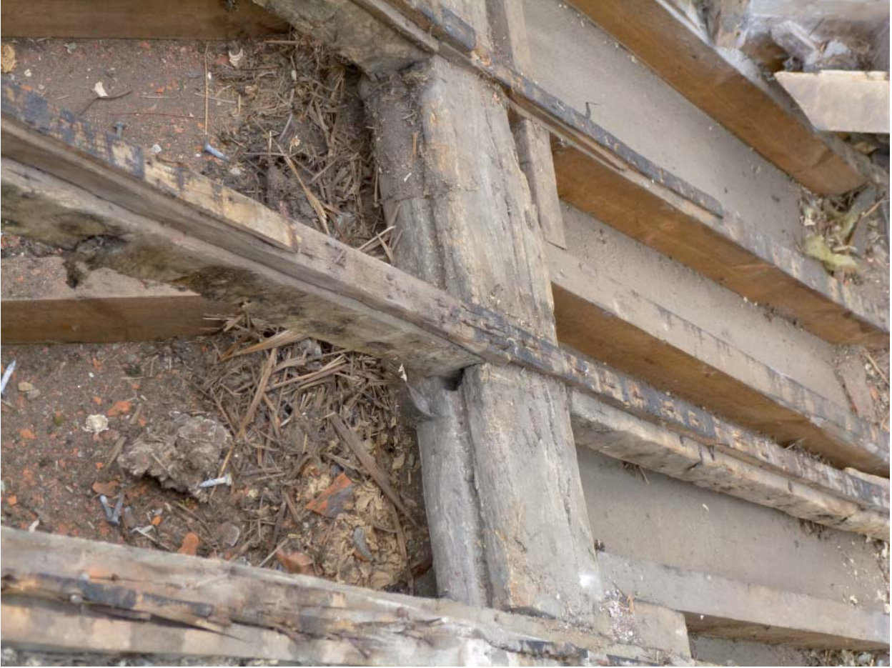
Plate 15: Stave slot in south slope lower purlin
