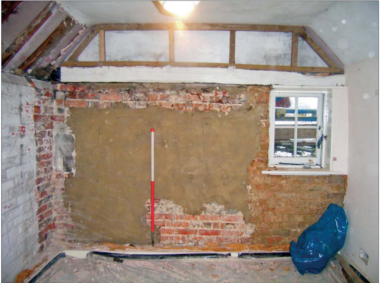
Plate 7: View of east elevation room 11/N
