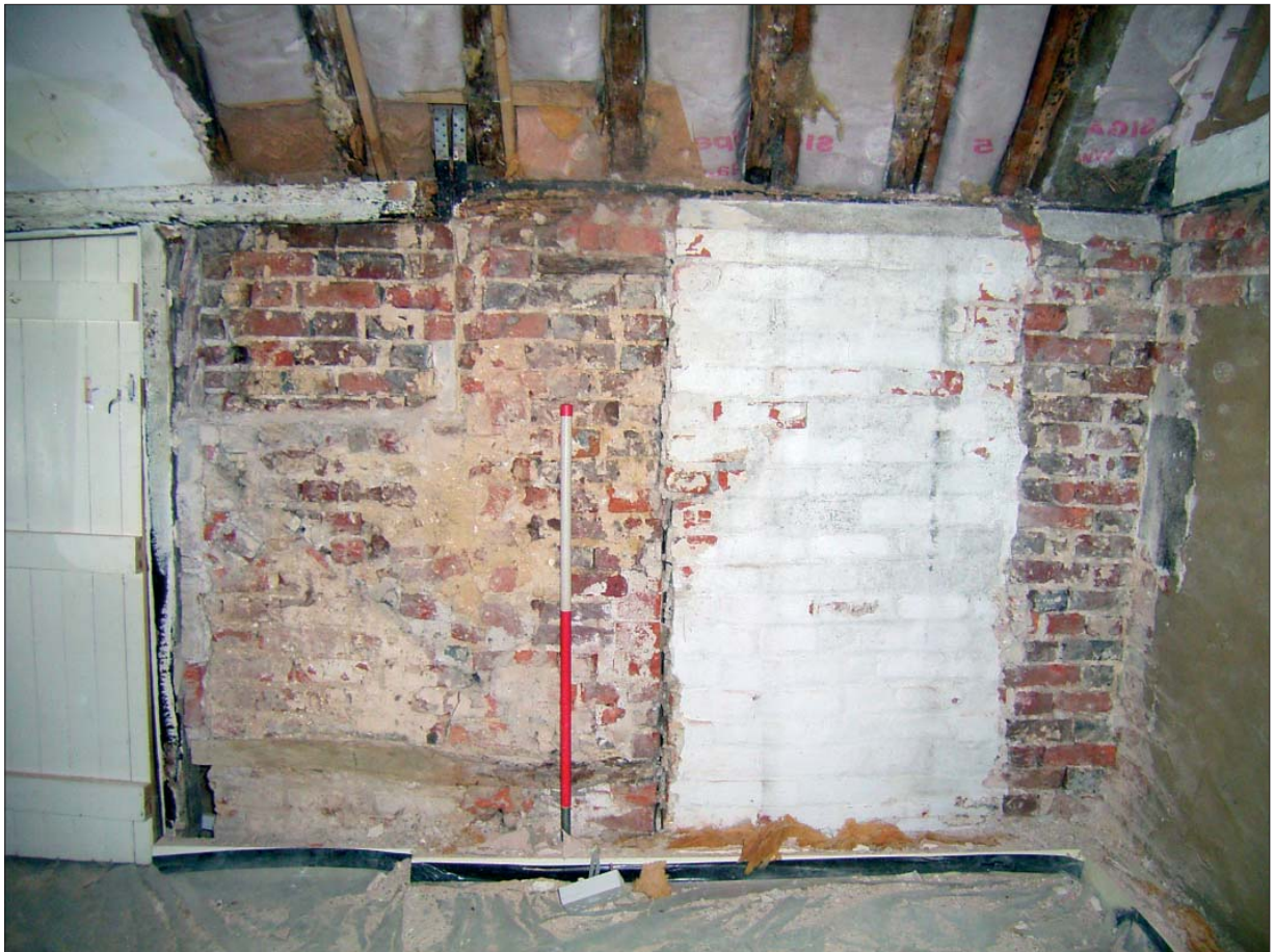
Plate 8: View of north elevation room 11/N
