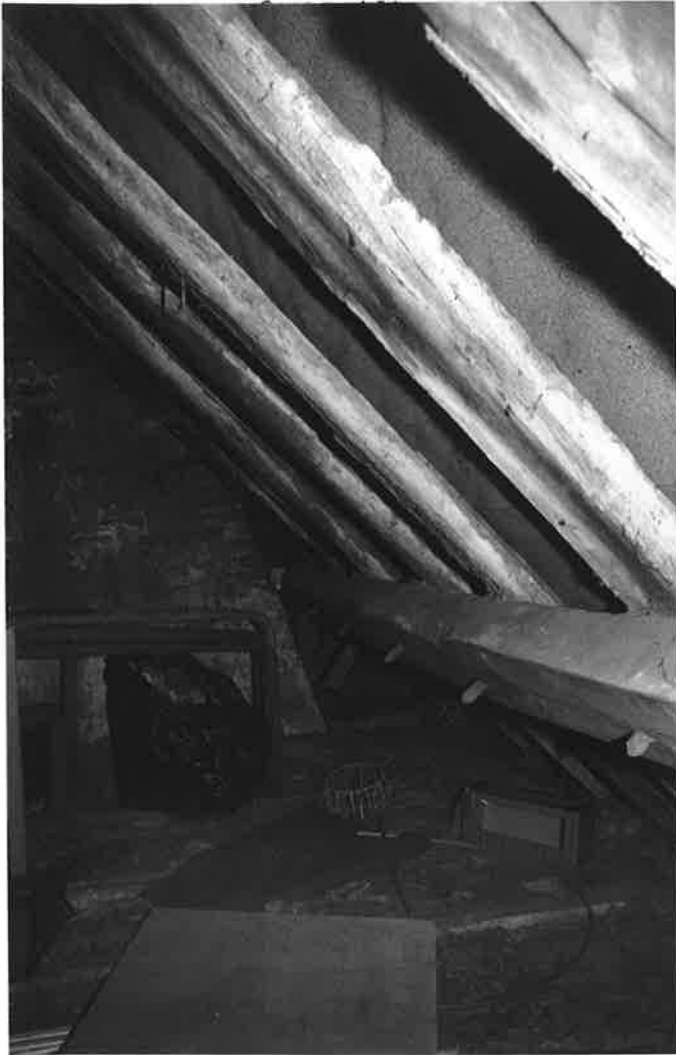
INTERNAL ROOF STRUCTURE , NO.12, LOOKING WEST. R174 N27A.
