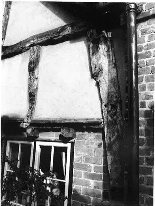
DETAIL OF MAIN POST, SOUTH GABLE, NO. 13. R228 N1.
