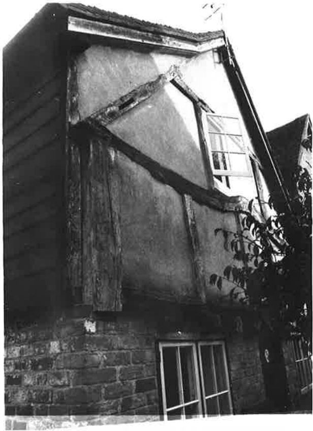
SOUTH GABLE, NO. 13, VIEWED FROM SOUTH - WEST. R228 N2.
