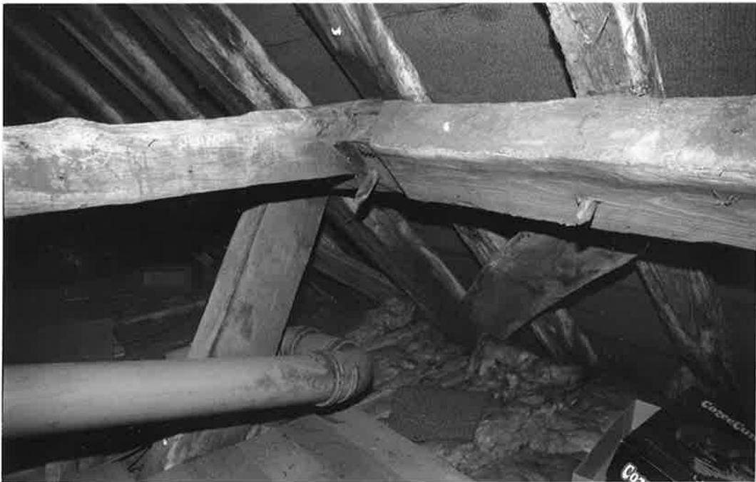
DETAIL OF WINDBRACING, INTERNAL ROOF STRUCTURE NO. 12, LOOKING NORTH-WEST R 174 N28A.
