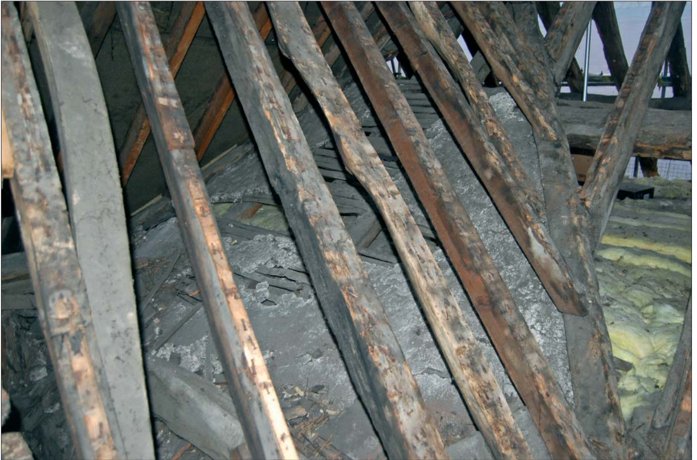
Plate 5: Detail of lath and plaster sloping partition
