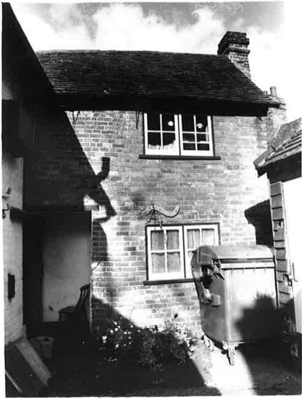
SOUTH ELEVATION OF REAR WING NO. 11. R228 N6.
