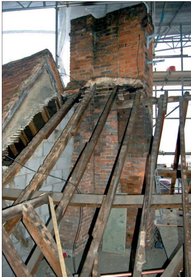
Plate 10: Stack at south-west corner of No.11
