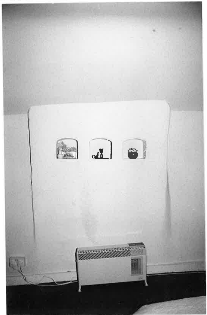
CHIMNEY BREAST, ROOM E, NO. 12. R 179 N3.
