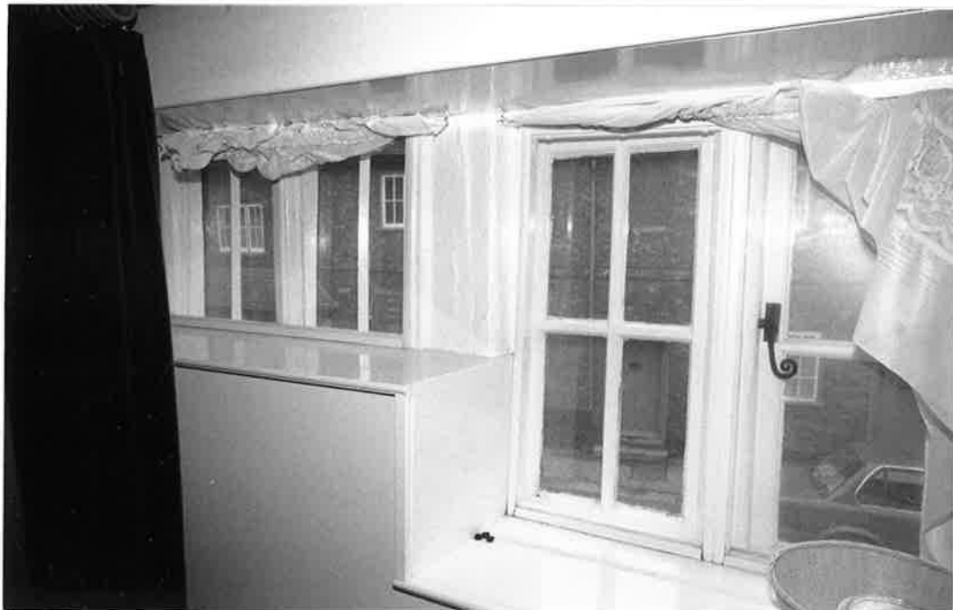
17th CENTURY WINDOW E2, AND MODERN WINDOW E3, NO. 12 R179 N4
