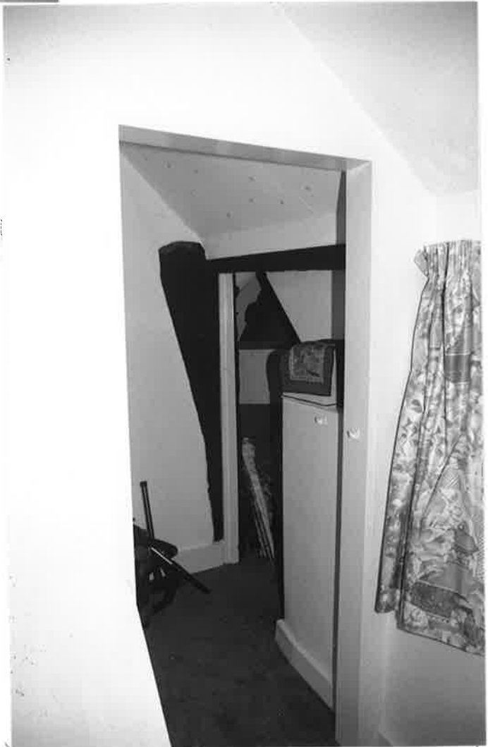
ROOM C, NO. 12, LOOKING SOUTH-EAST. R174 N35A
