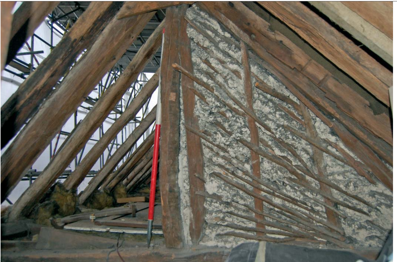
Plate 4: Detail of wattle and daub partition walling (Truss 4)
