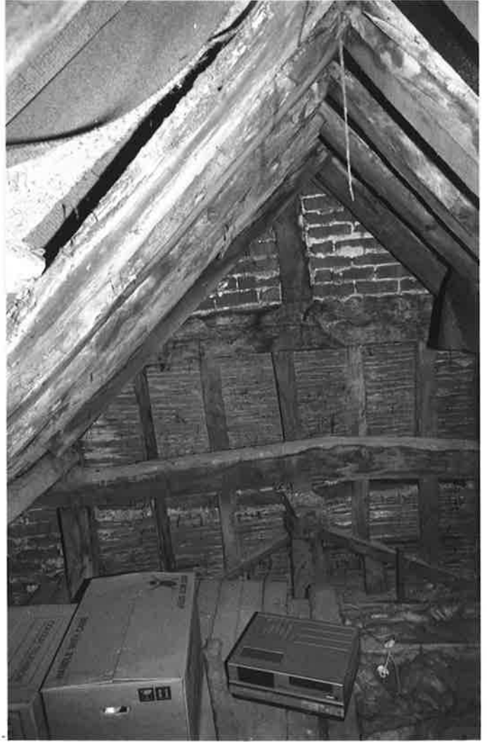
INTERNAL ROOF STRUCTURE , LOOKING EAST. R174 N29A.
