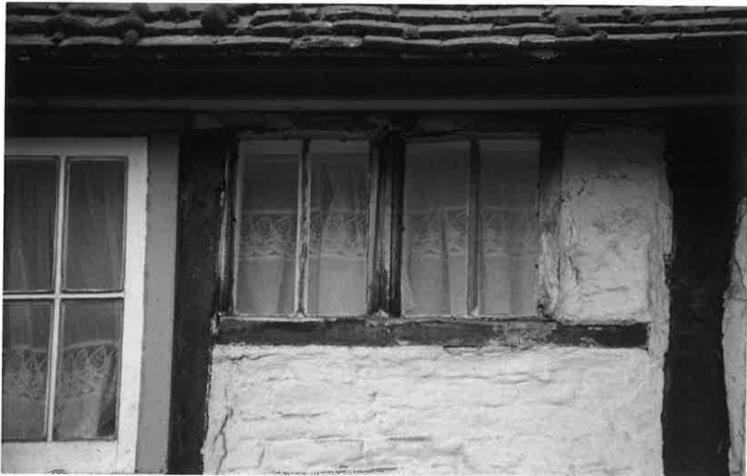
DETAIL OF 17th CENTURY WINDOW E2 NO. 12 R179 N17.
