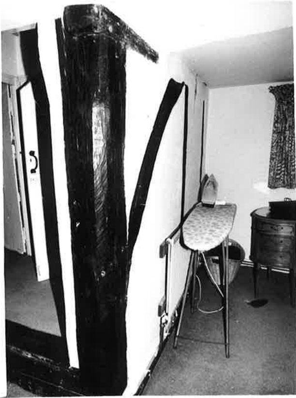
CORNER POST OF ORIGINAL MAIN BLOCK, VIEWED FROM LANDING ROOM K, NO. 11. R 228 N 16.
