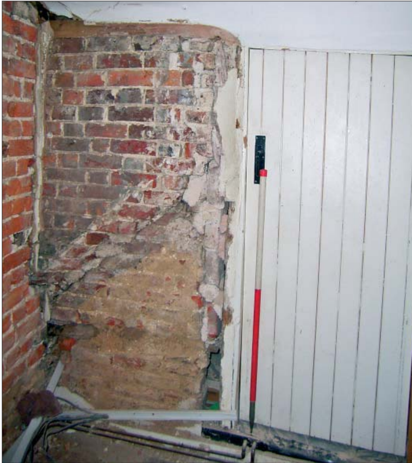
Plate 9: View of south elevation within lobby 11/K
