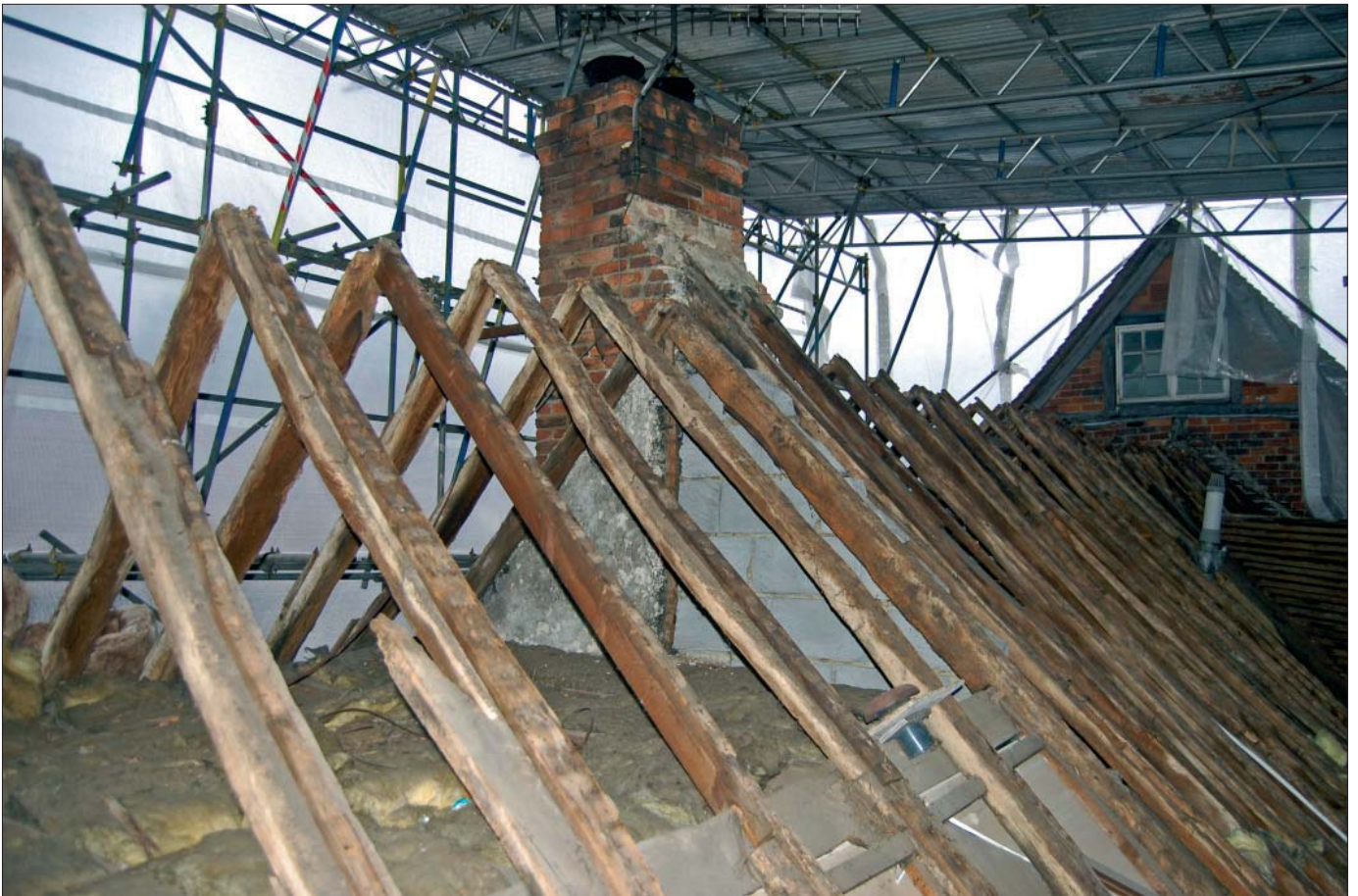
Plate 6: View of rear elevation of roof for no. 11 and 12
