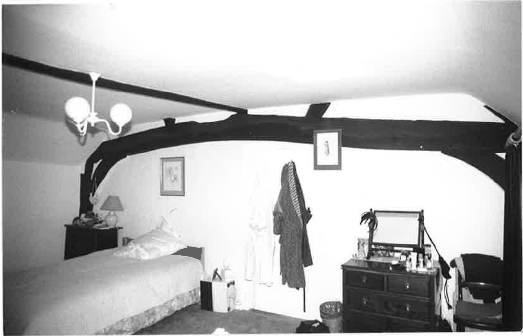
BEDROOM E, NO. 12, LOOKING SOUTH - WEST. R179 N1.
