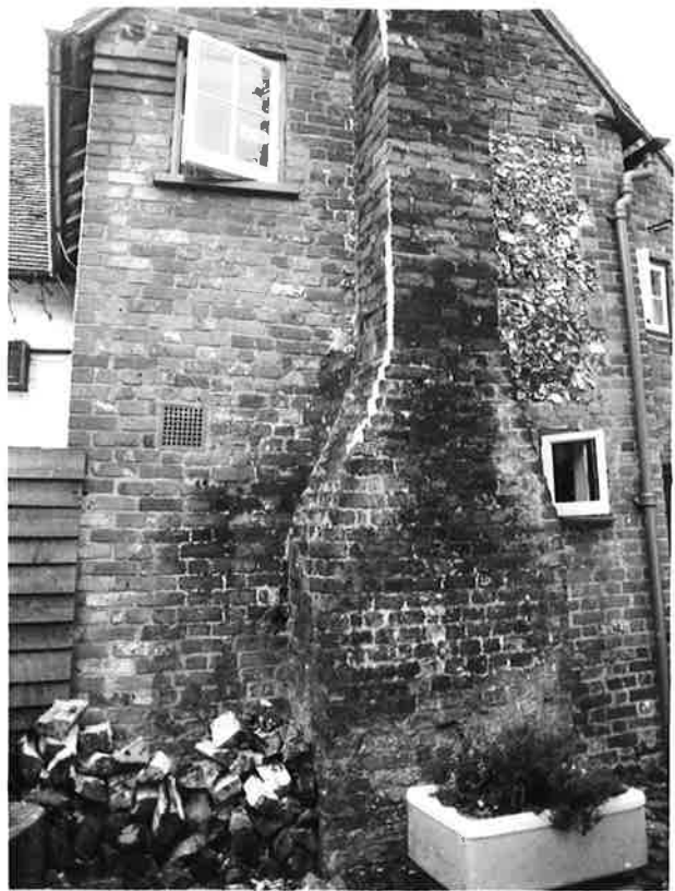
EAST ELEVATION OF REAR WING NO. 11. R228 N8.
