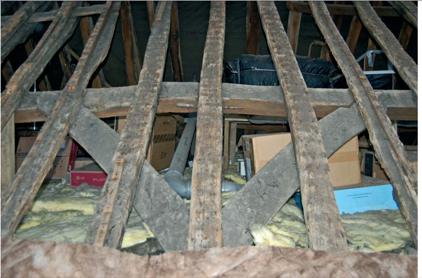
Plate 3: Detail of wind braces on south elevation (Truss 2)
