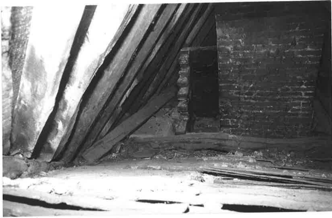
CHIMNEY STACK NO. 12 , VIEWED FROM ROOF SPACE.
