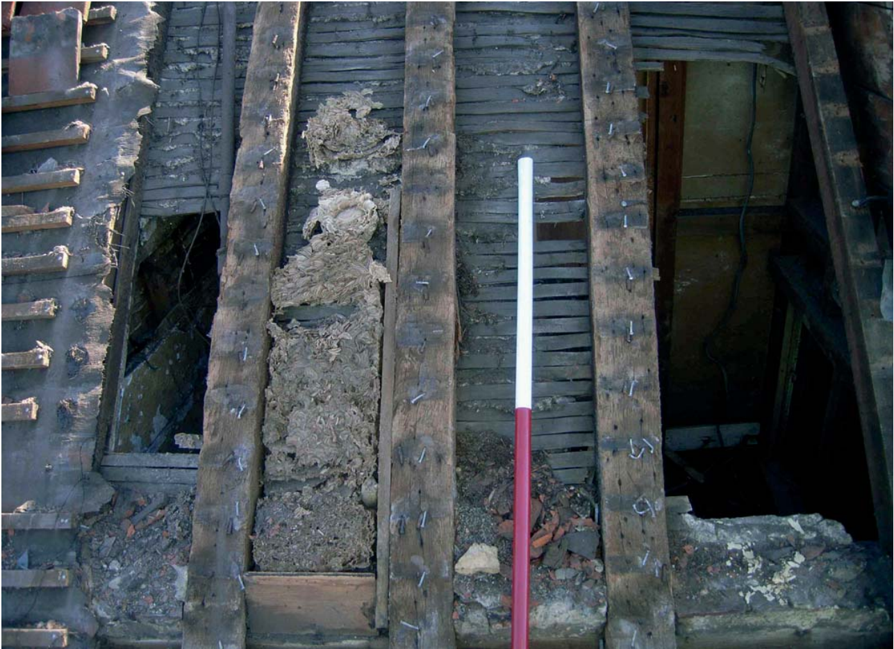
Plate 19: Original lath and plaster wall and ceiling and the RSA boxing-in of the eaves, west slope of the west wing
