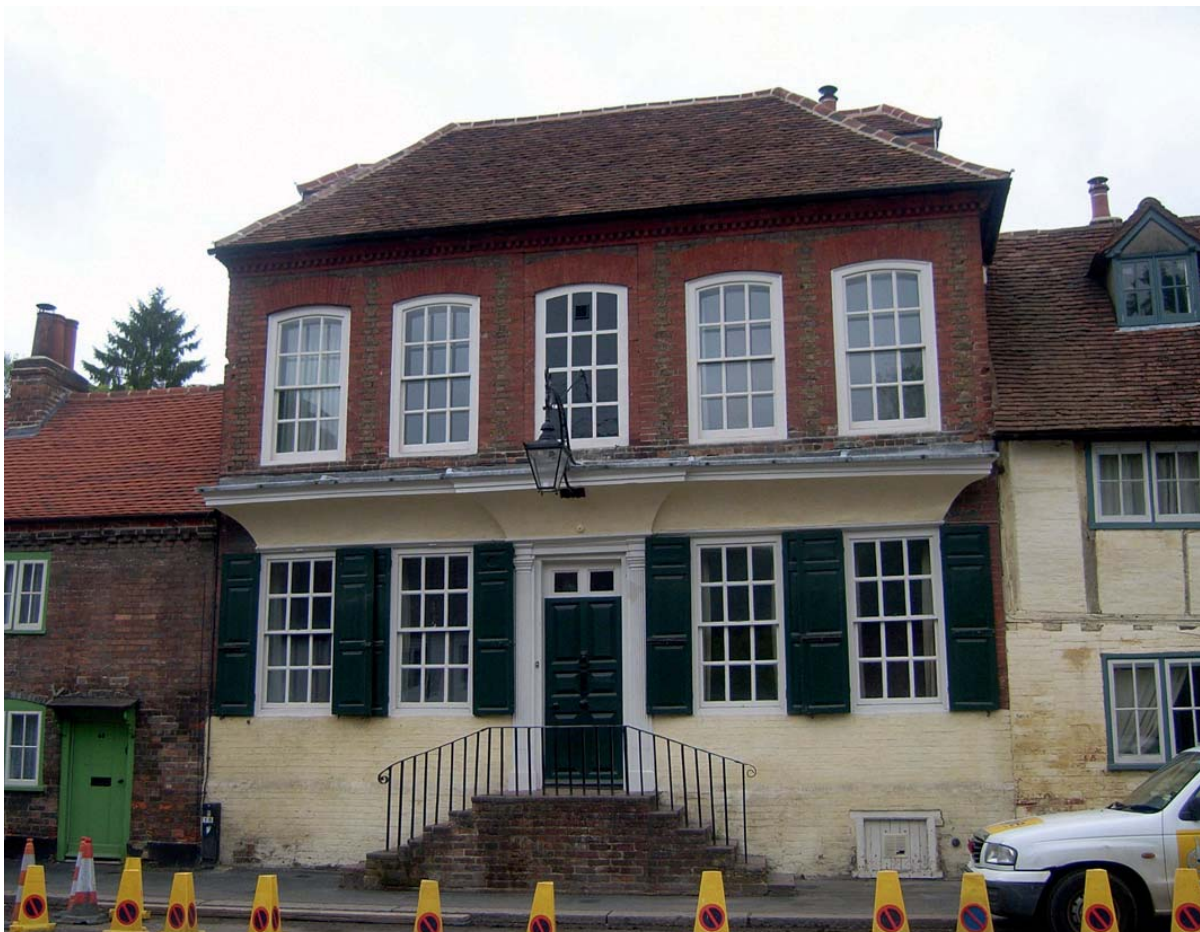
Plate 2: Steps House following re-covering of the roof, south elevation
