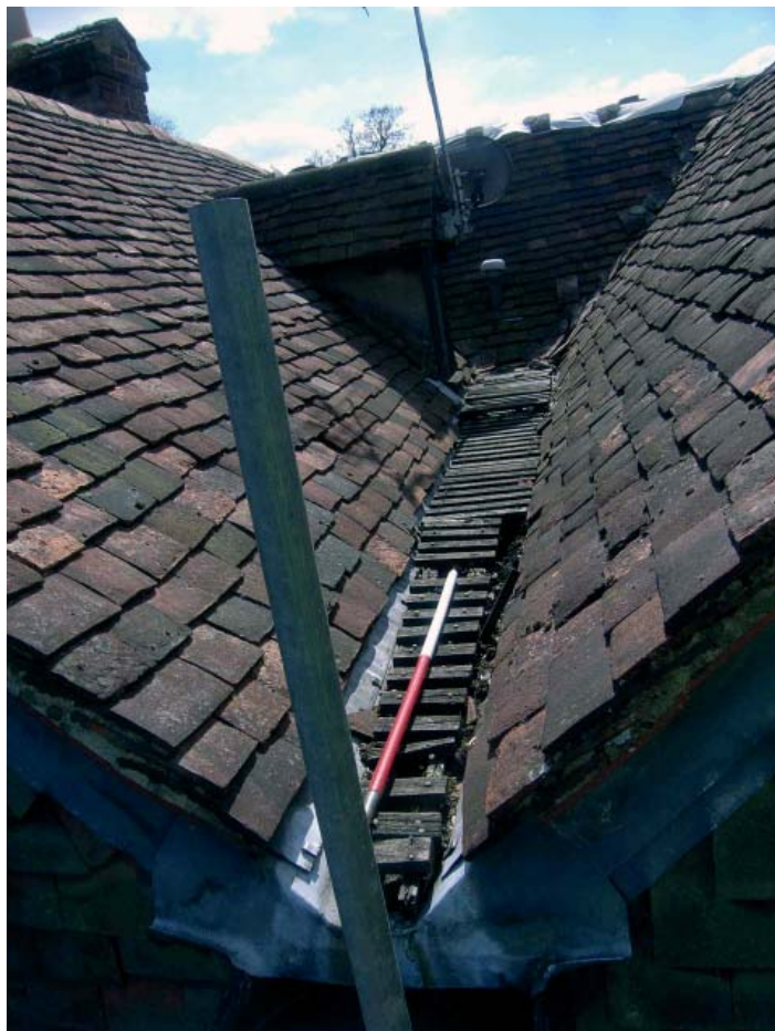
Plate 4: Dormer window/roof access in the valley between the wings
