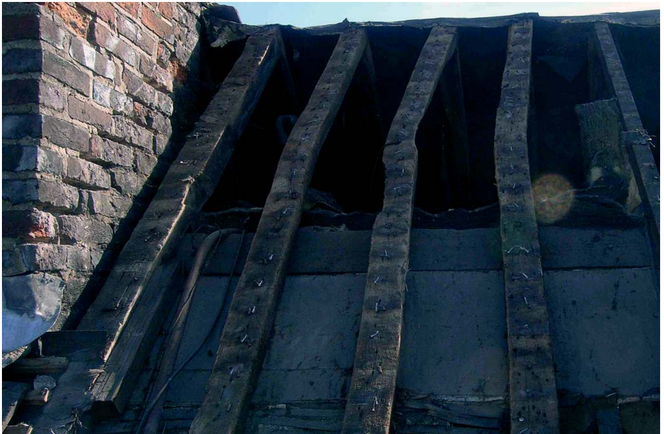
Plate 13: Tenon of collar visible but the collar obscured, west slope of the west wing
