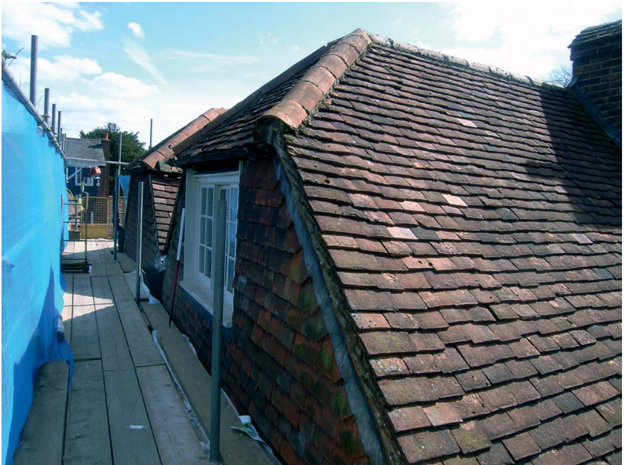
Plate 8: Half-hipped wings prior to stripping
