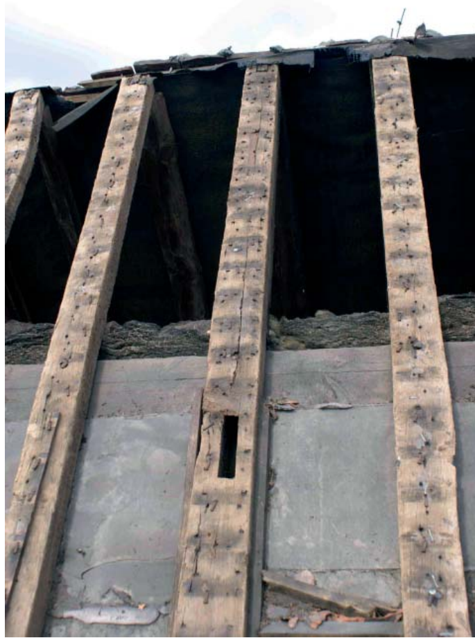
Plate 5: Empty mortice in the principal rafter in the south slope of the south range (courtesy of Gary Marshall)
