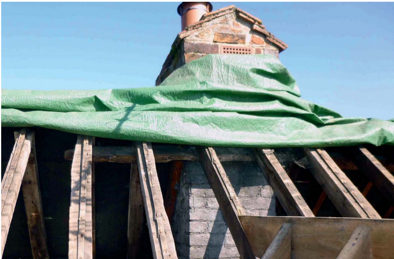
Plate10: Later support of the rafters at the apex next to the east wing chimney stack, west slope
