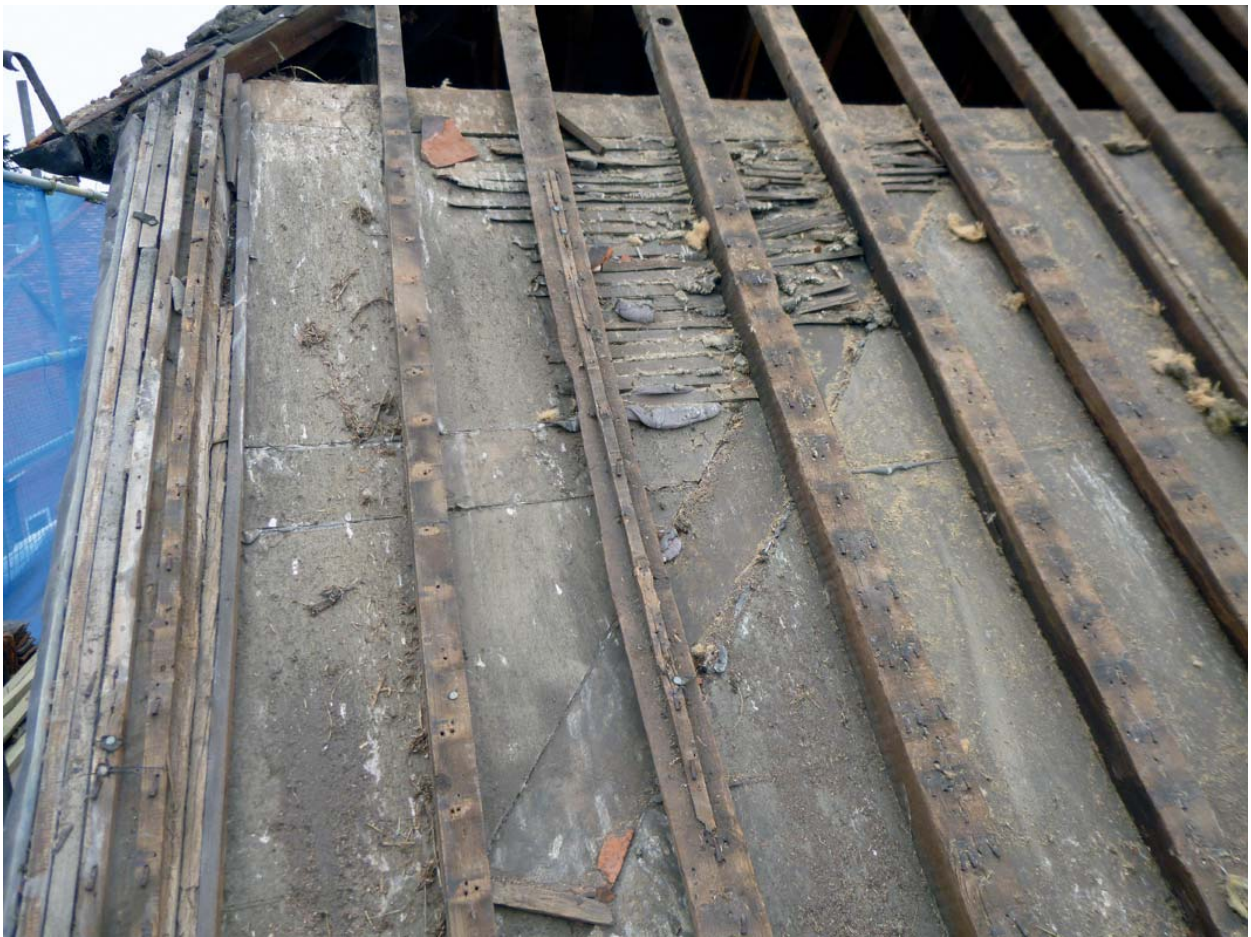
Plate 15: Windbrace in the west slope of the west wing
