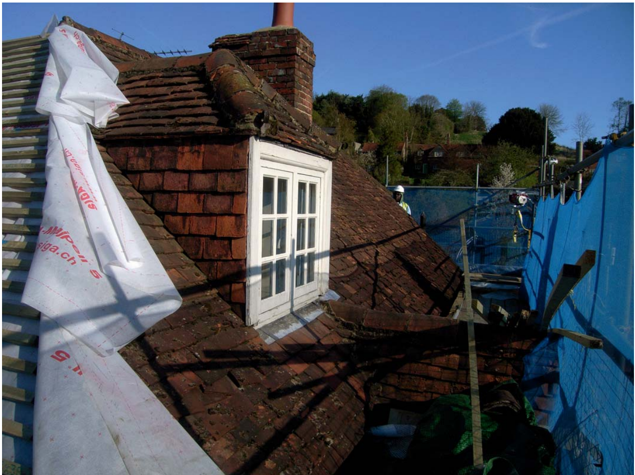
Plate 3: Dormer window in the east slope of the east wing
