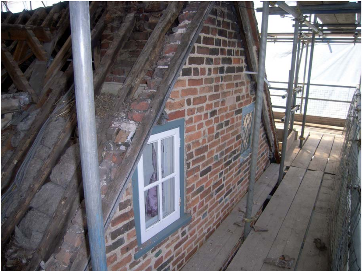
Plate 18: Gable at west end of building (No 29)
