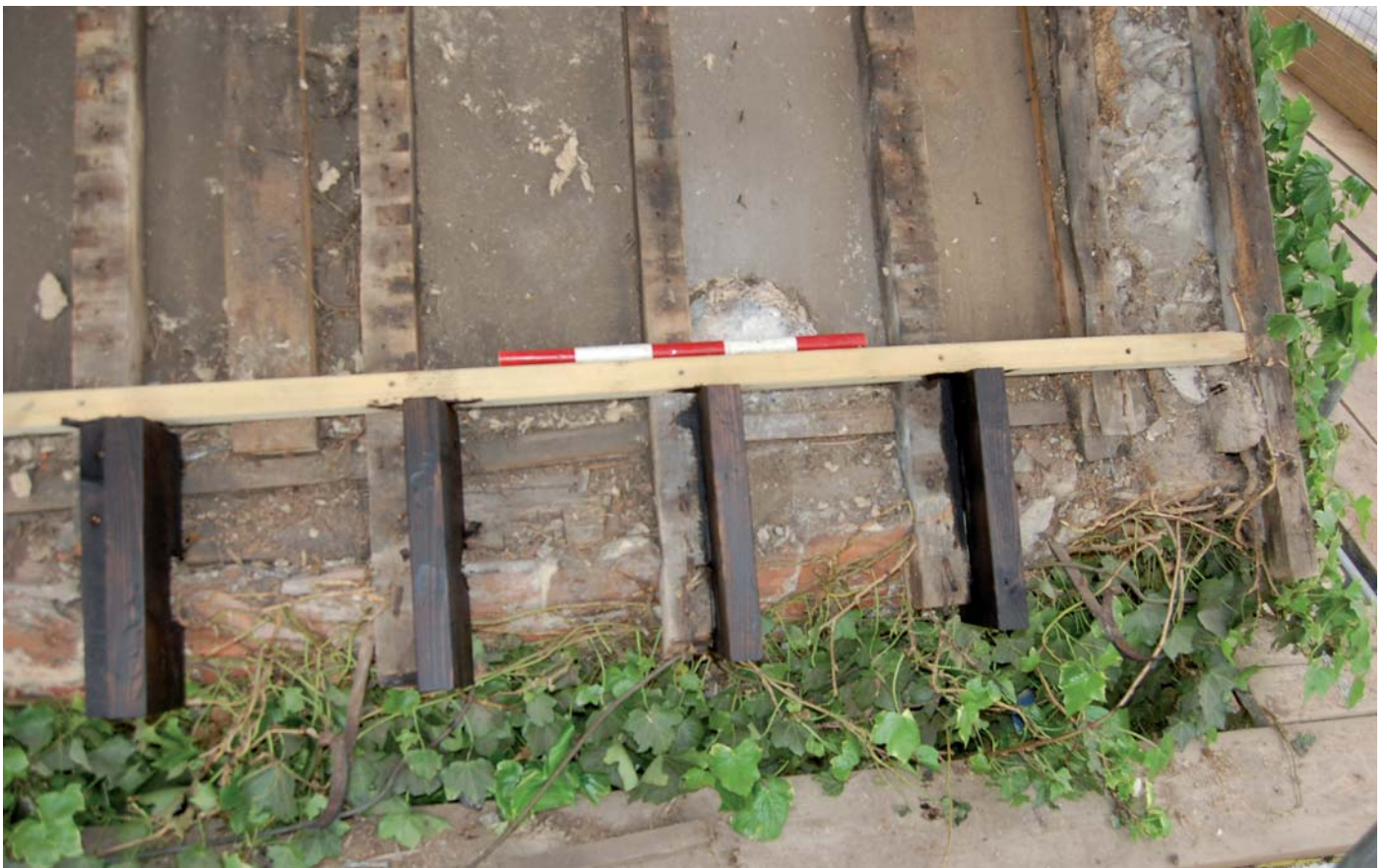
Plate 22: Detail at south-east corner of building
