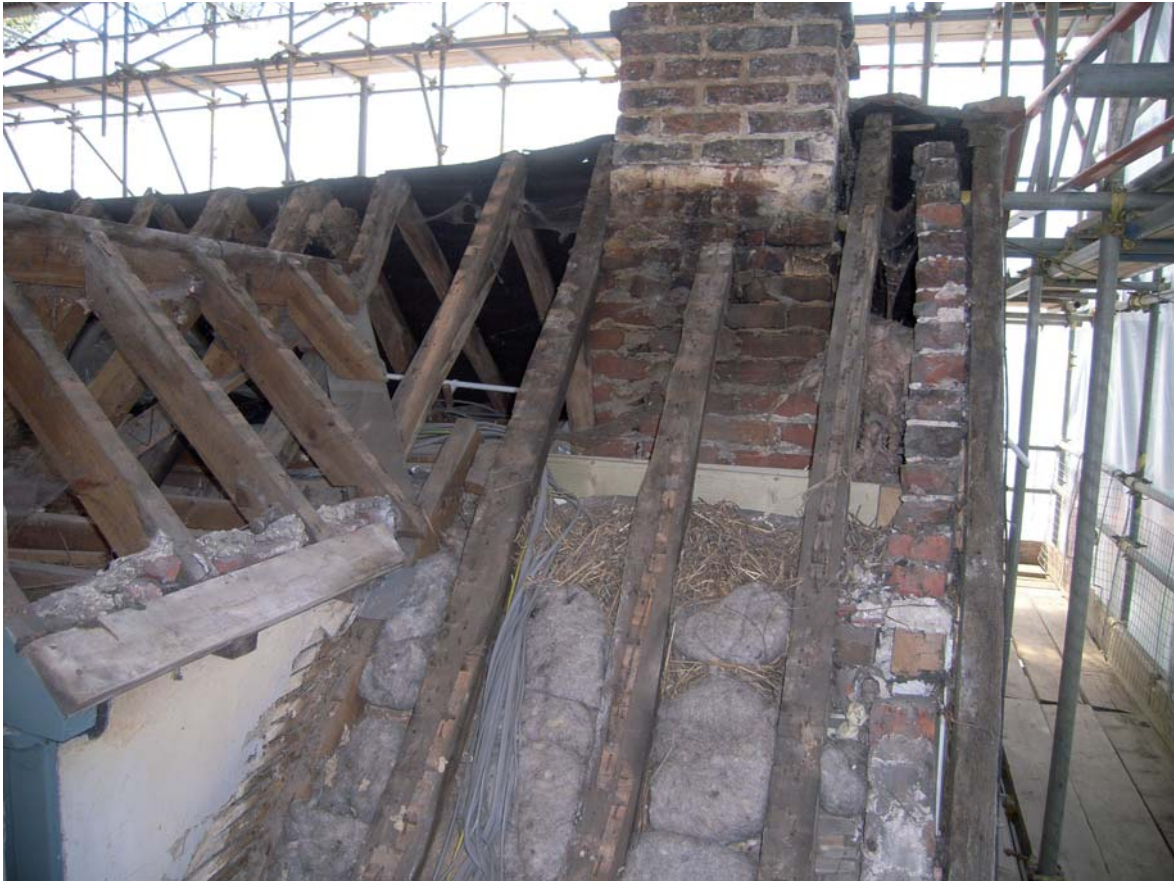
Plate 17: West end of north slope
