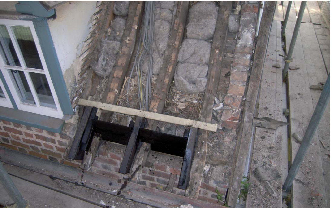
Plate 16: West end of north slope
