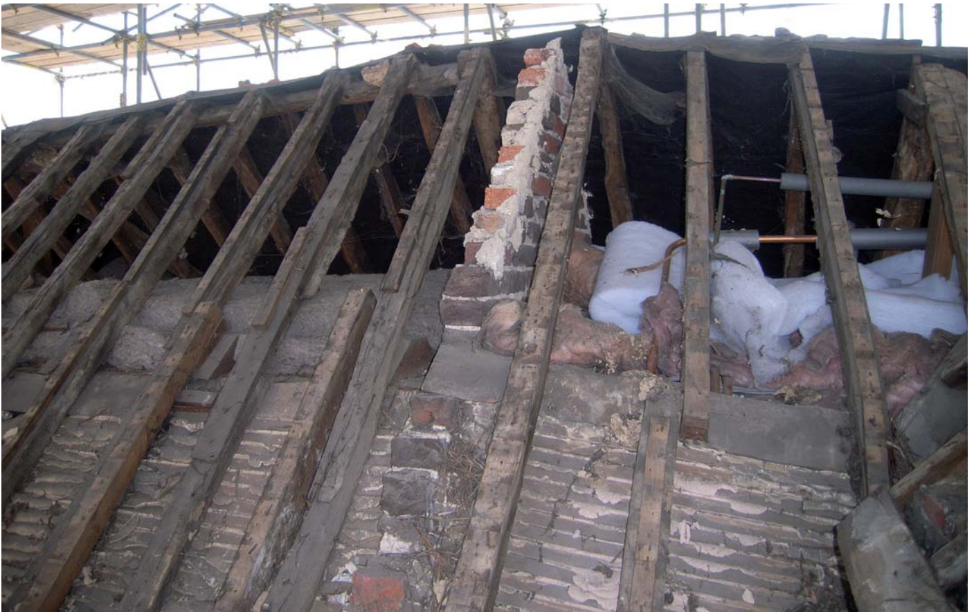
Plate 11: Brick wall (formerly external gable) between No 29 and No 30
