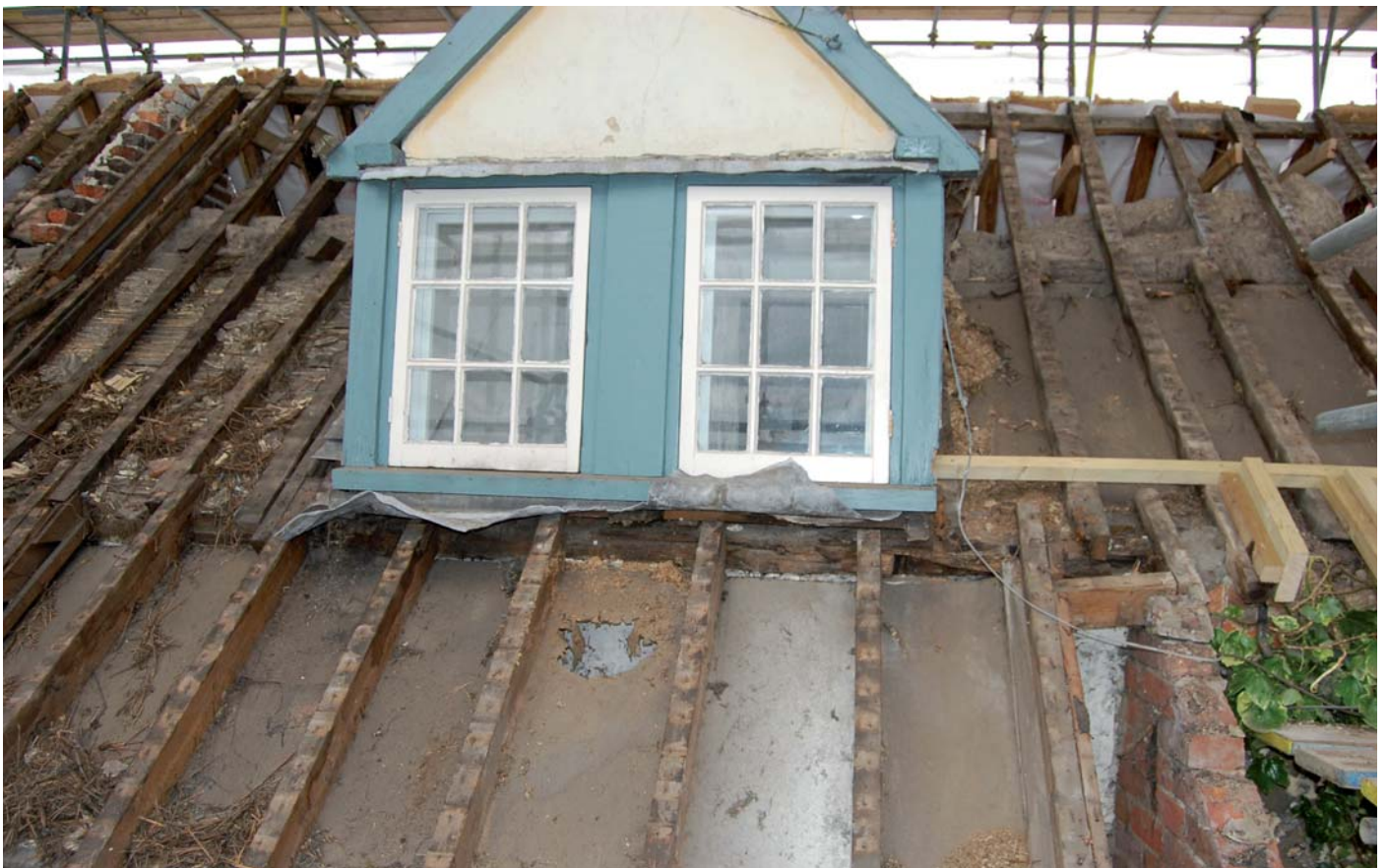
Plate 24: Dormer in south slope of No 30
