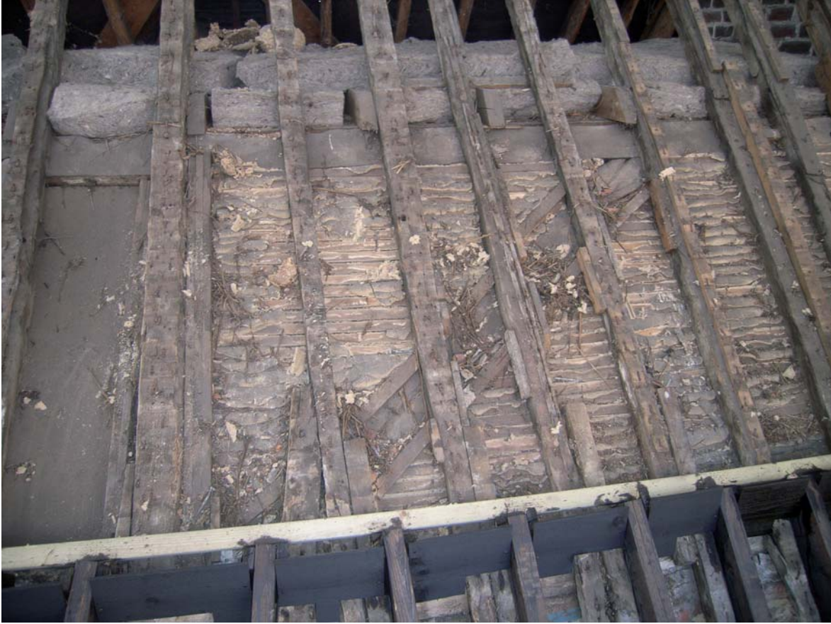
Plate 9: Wind brace in north slope of No 30
