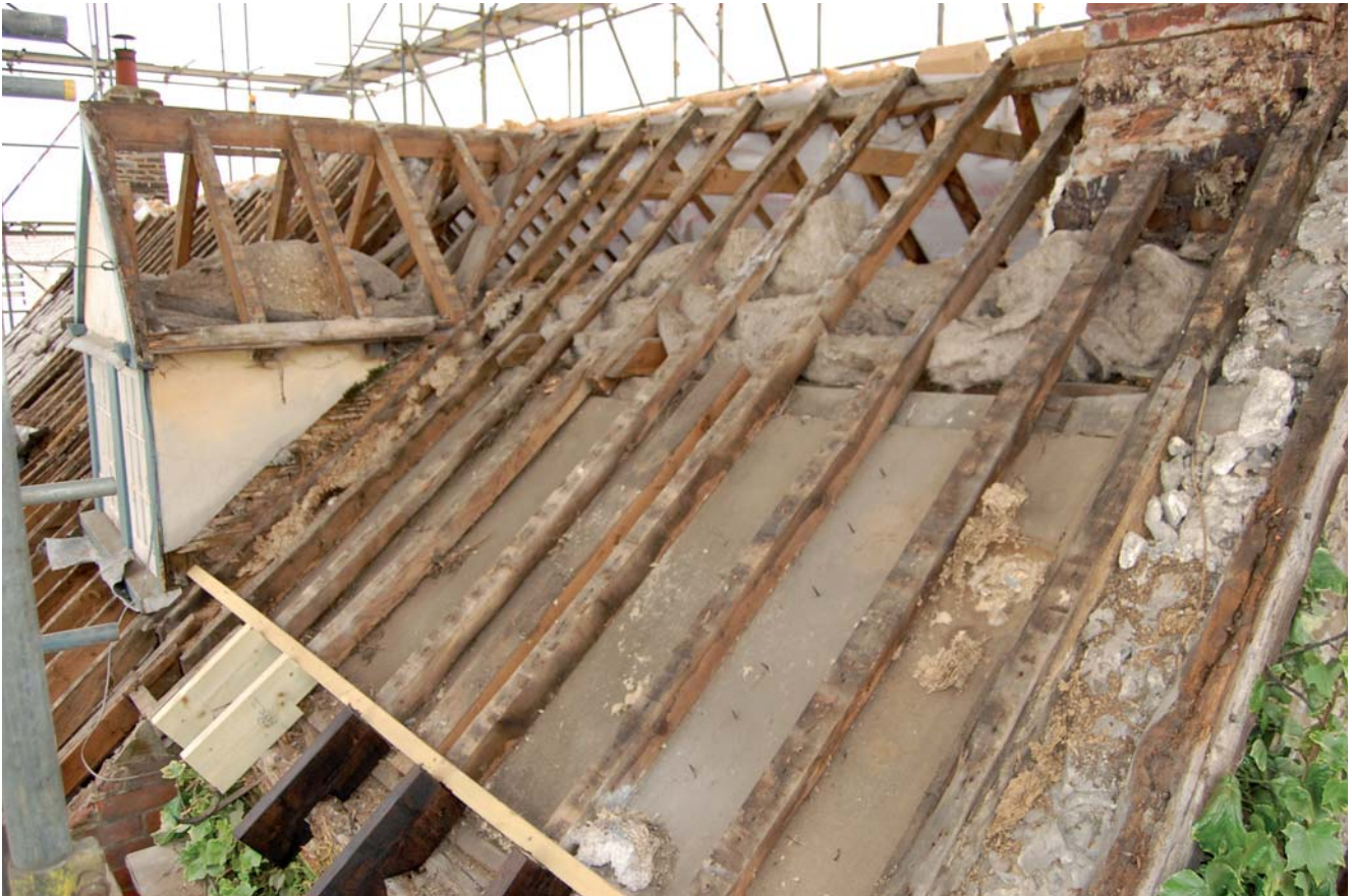
Plate 20: South slope of No 30
