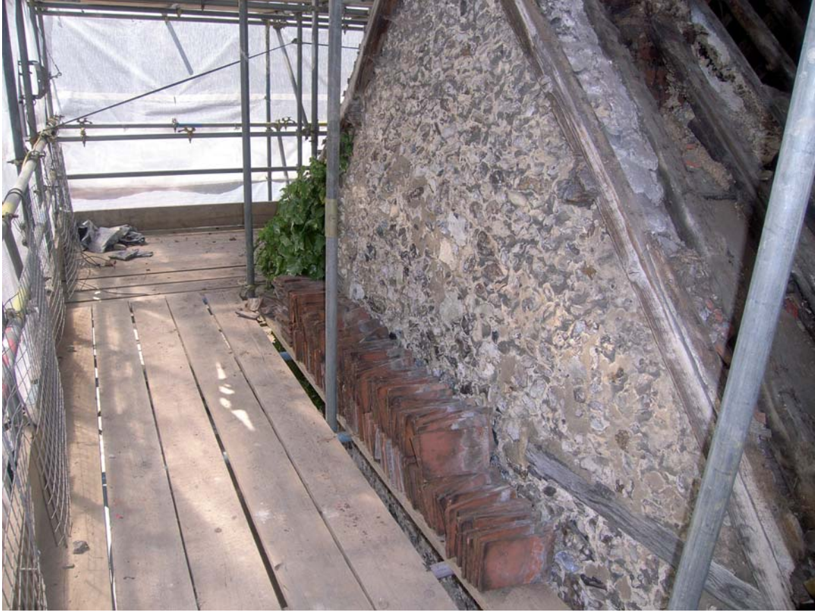
Plate 19: Flint gable at east end of building (No 30)
