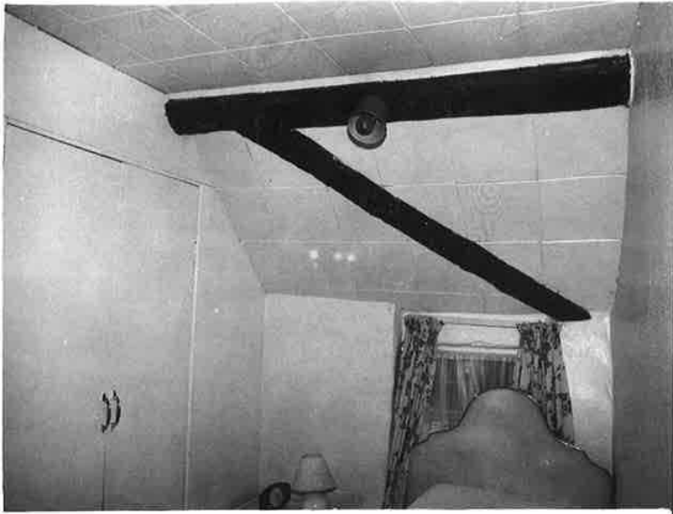
ROOM E, NO. 30, LOOKING NORTH. R221 N25.
