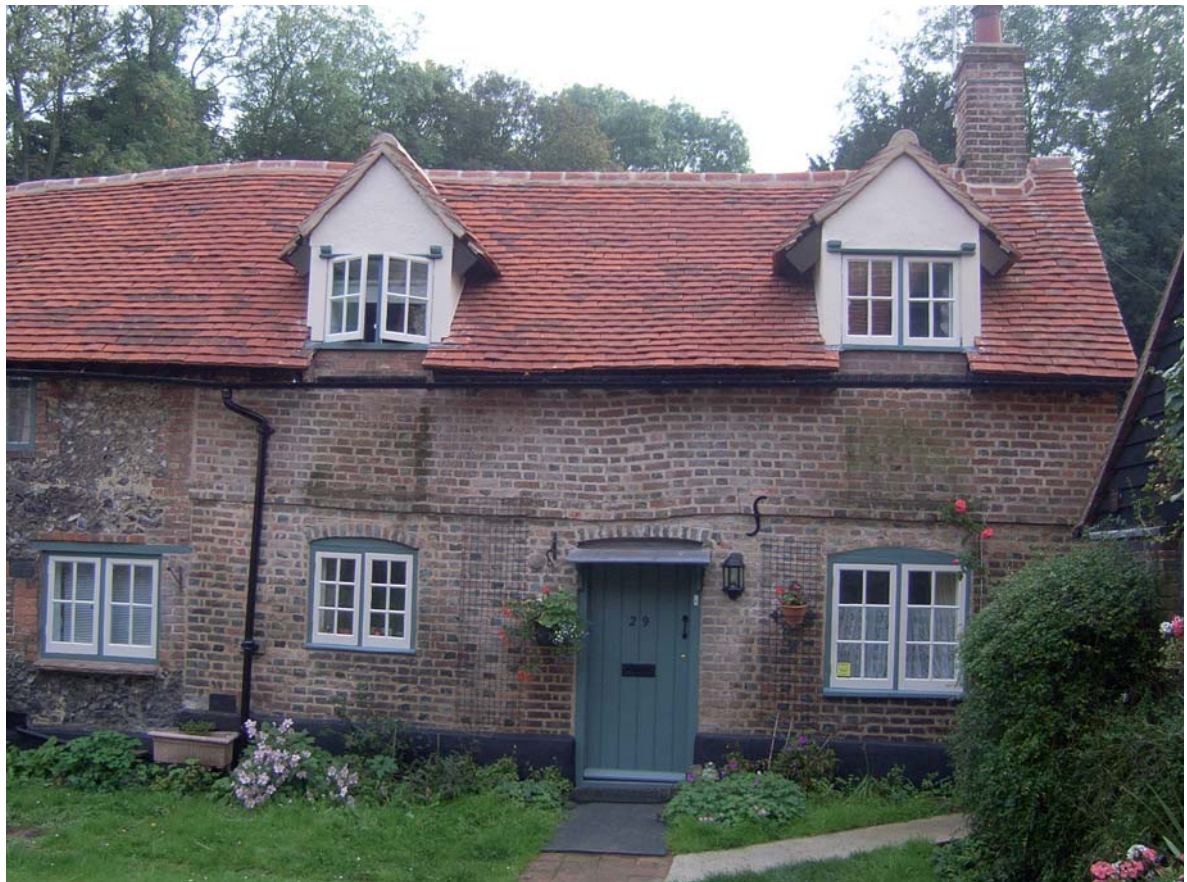
Plate 2: North elevation of No 29 facing Crown Court
