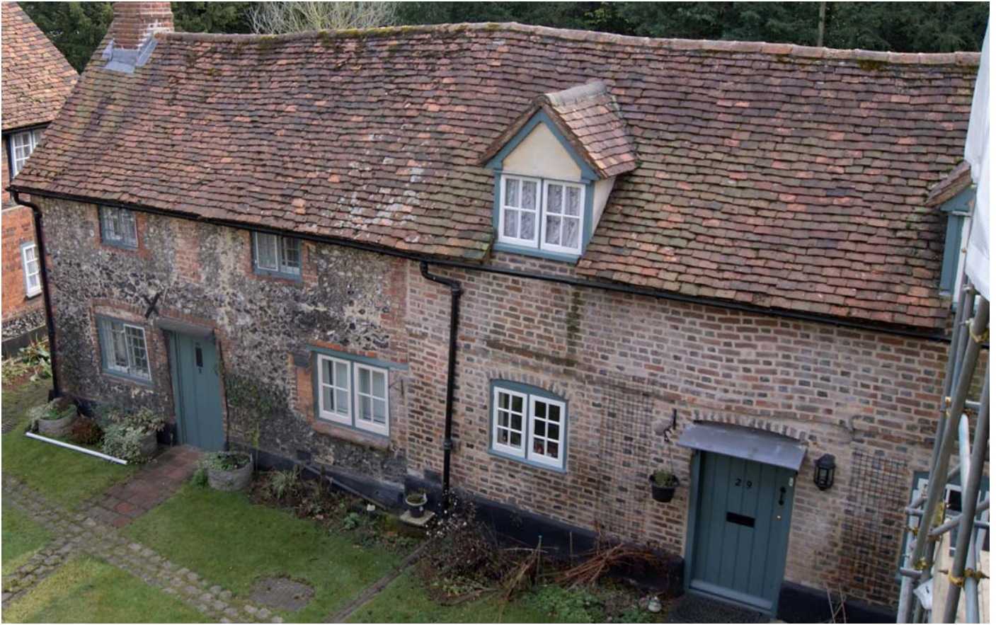
Plate 1: General view of north elevation (taken from scaffolding of adjacent range)
