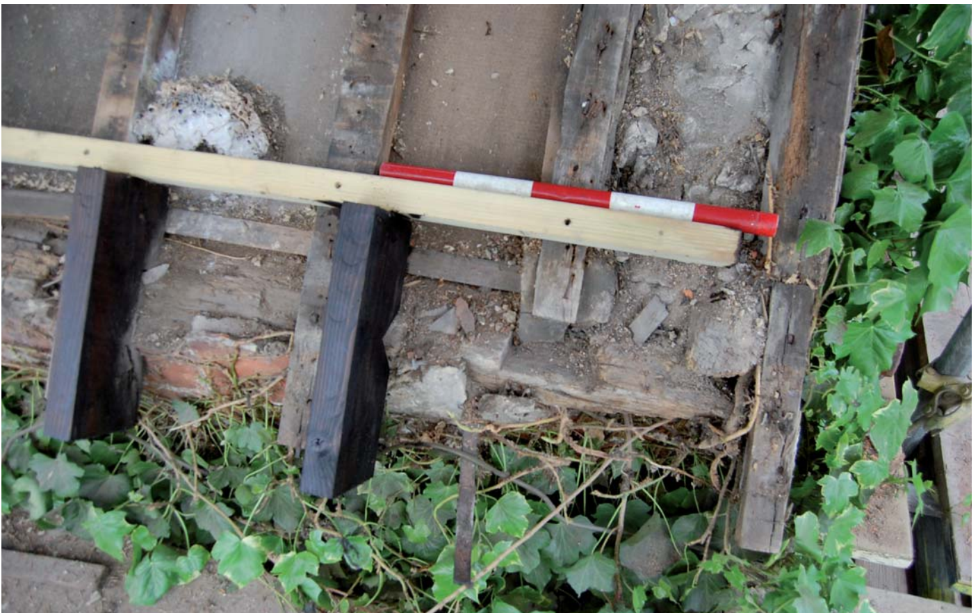
Plate 32: Detail at south-east corner of building
