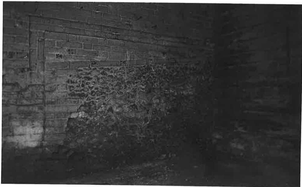
DETAIL OF REAR WALL, BUILDING NO 2, NO 58A. R. 192 N. 27
