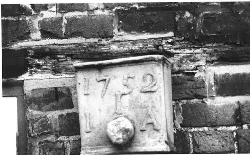
LEAD RAINWATER HEAD, TO REAR WING. NO 58A R. 192 N. 24
