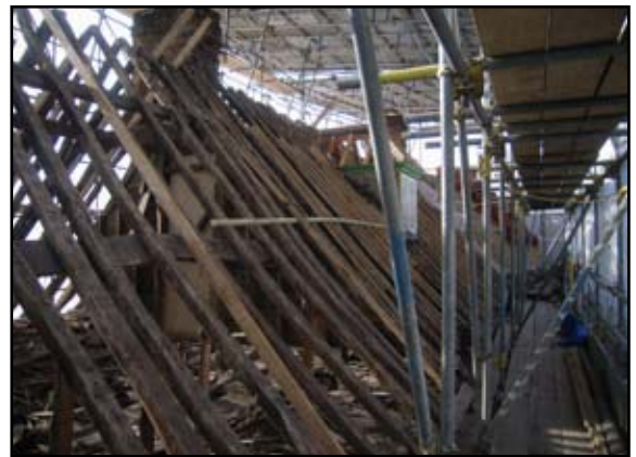
Plate 8: Main block south elevation of roof timbers, view towards west
