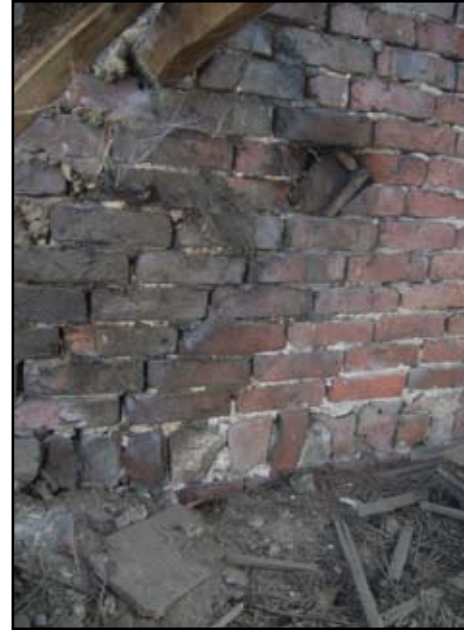
Plate 10: Detail of main block north east east gable wall
