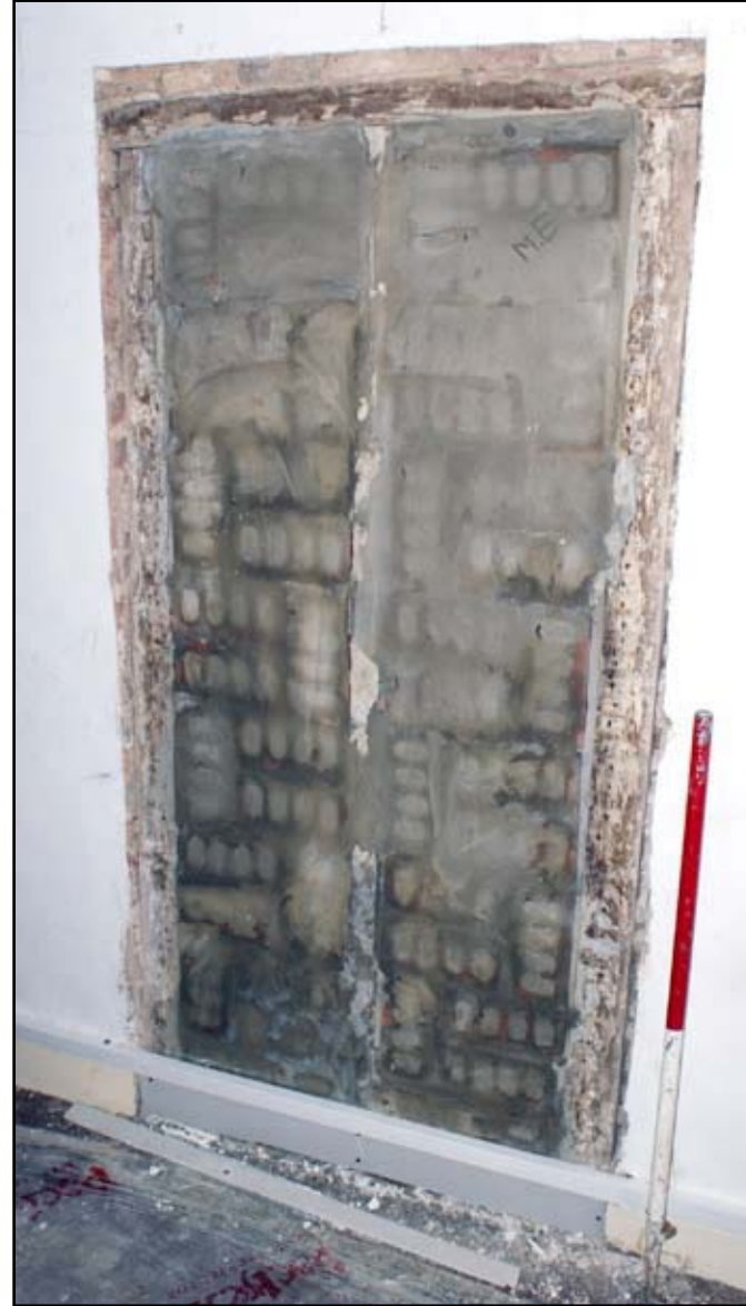
Plate 18: Blocked opening in room 57/1 (photo: National Trust)
