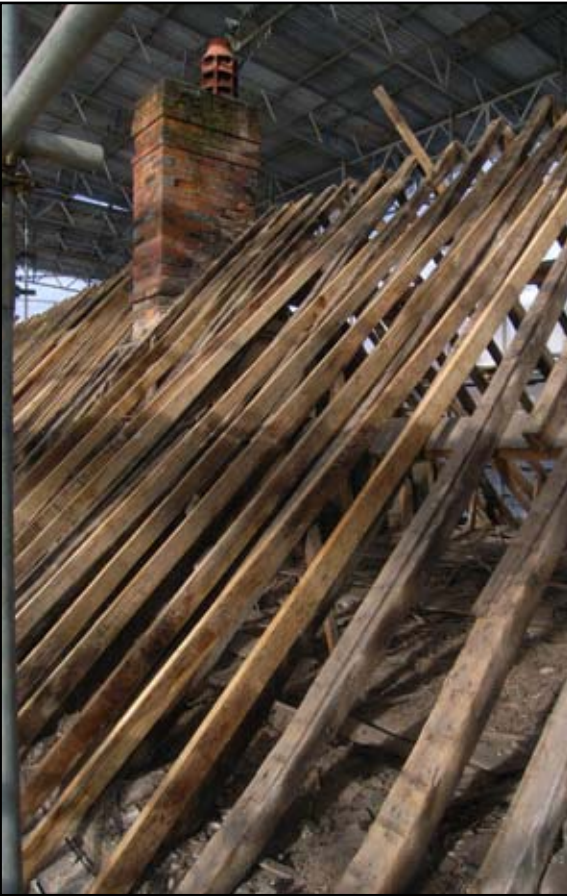
Plate 1: Main block north elevation roof timbers following removal of tiles
