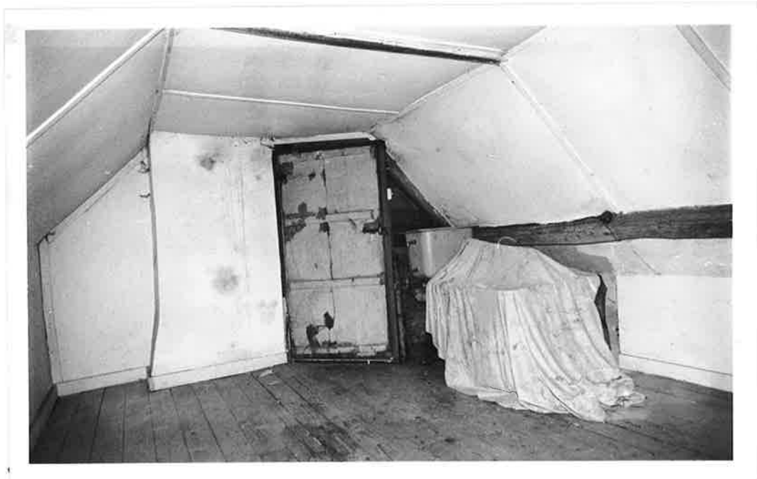
ATTIC ROOM M, NO 58A LOOKING WEST. R.191 N.35A.
