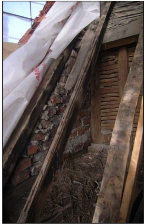
Plate 6: Detail of gable wall between main and west blocks
