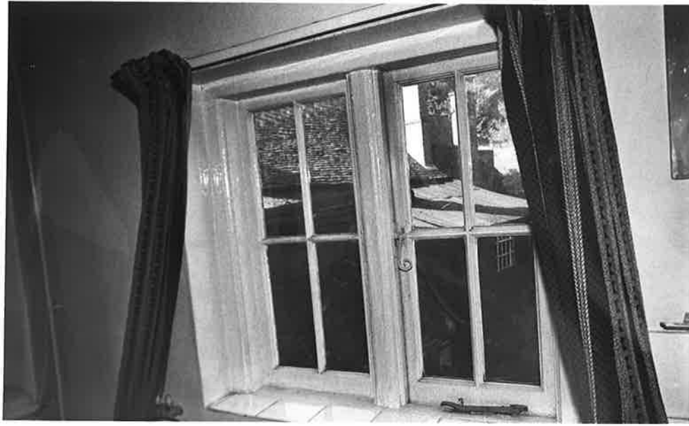
ROOM I, LOOKING NORTH-WEST. NO 58A. R.192 N.3
