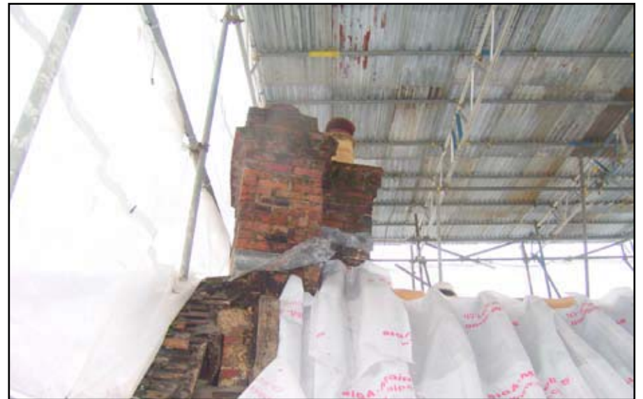
Plate 12: Detail of central chimney stacks south elevation
