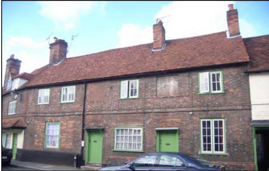
Plate 19: High street elevation prior to works
