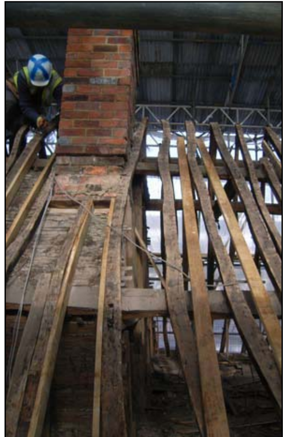
Plate 4: Northern elevation of main block roof timbers with central chimney and attic rooms lath and plasterwork
