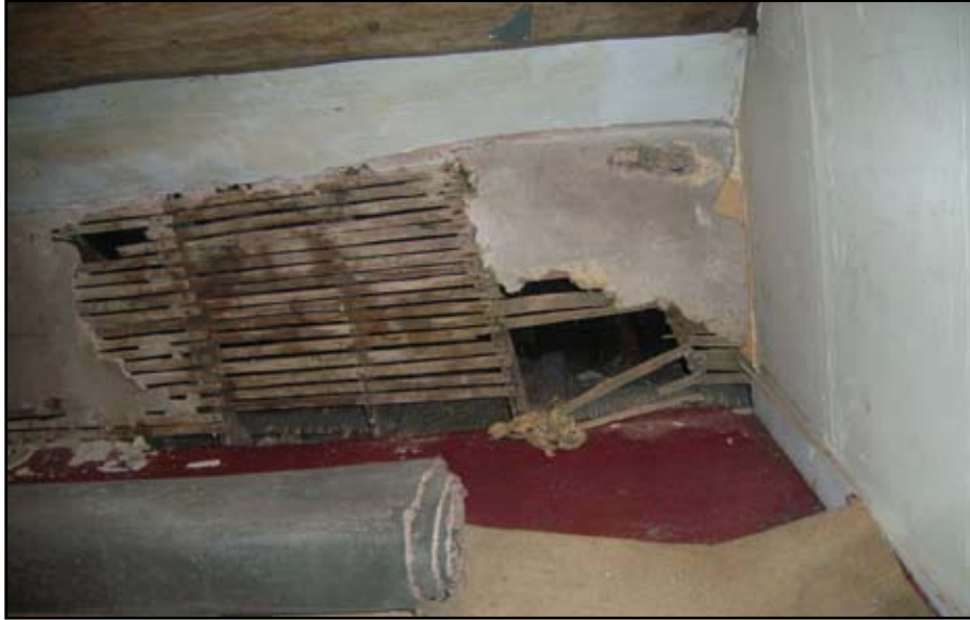
Plate 17: Room 58/M interior view, lath and plaster detail on north elevation
