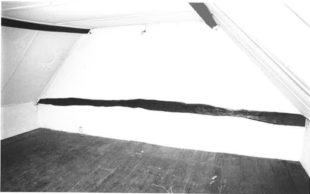
ATTIC ROOM K, NO 58A, LOOKING WEST. R.191 N.36
