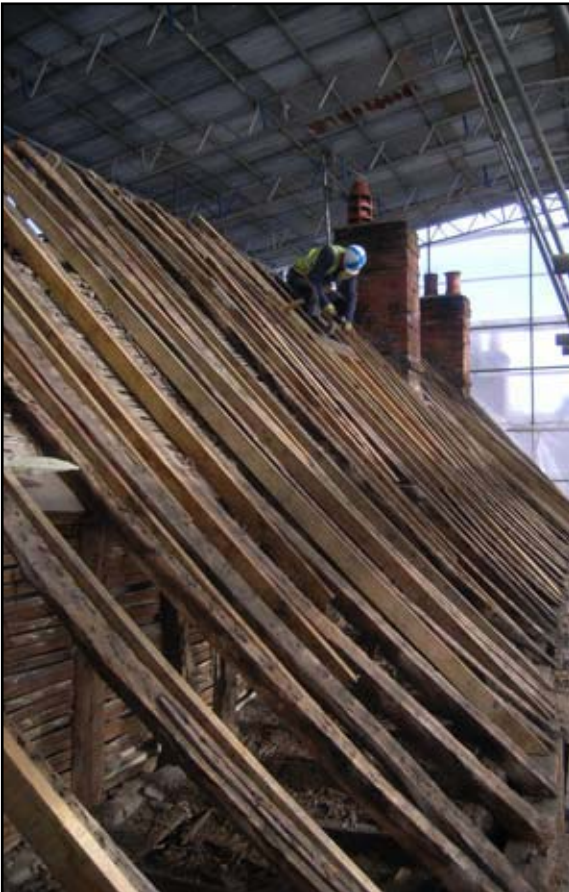
Plate 7: Main block roof timbers north elevation viewed towards east
