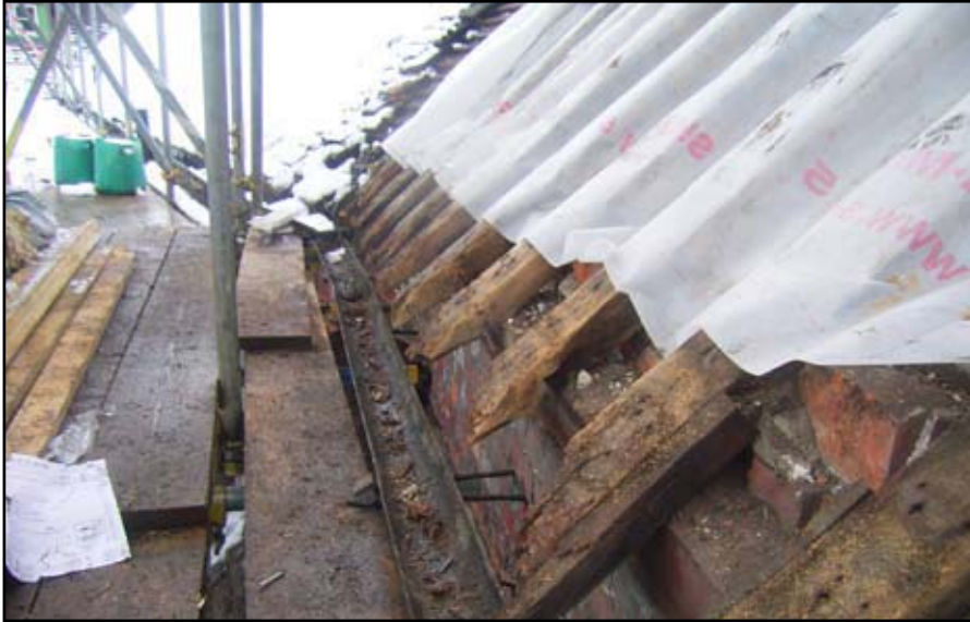
Plate 13: No. 58a notched rafter detail on north elevation
