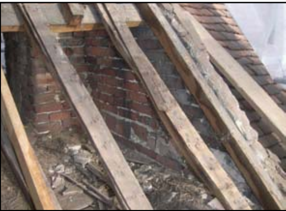
Plate 3: Gable wall between 57 and 56 detail showing tile infill
