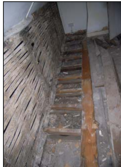
Plate 16: Room 58/M interior view, exposed joists on south side of room
