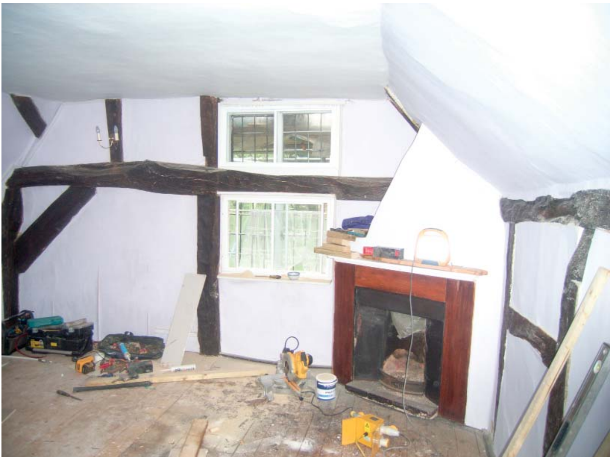
Plate 96: No. 4. First floor rear projection looking south
