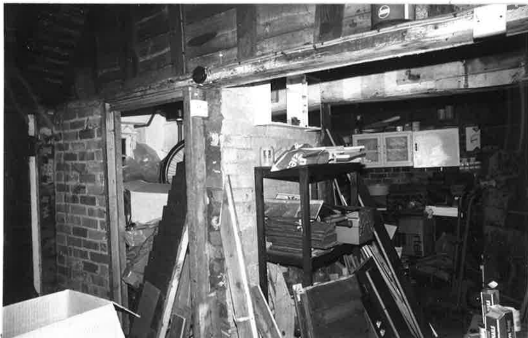
ROOM B, BUILDING Nº5, LOOKING SOUTH-WEST. R173 N22A.
