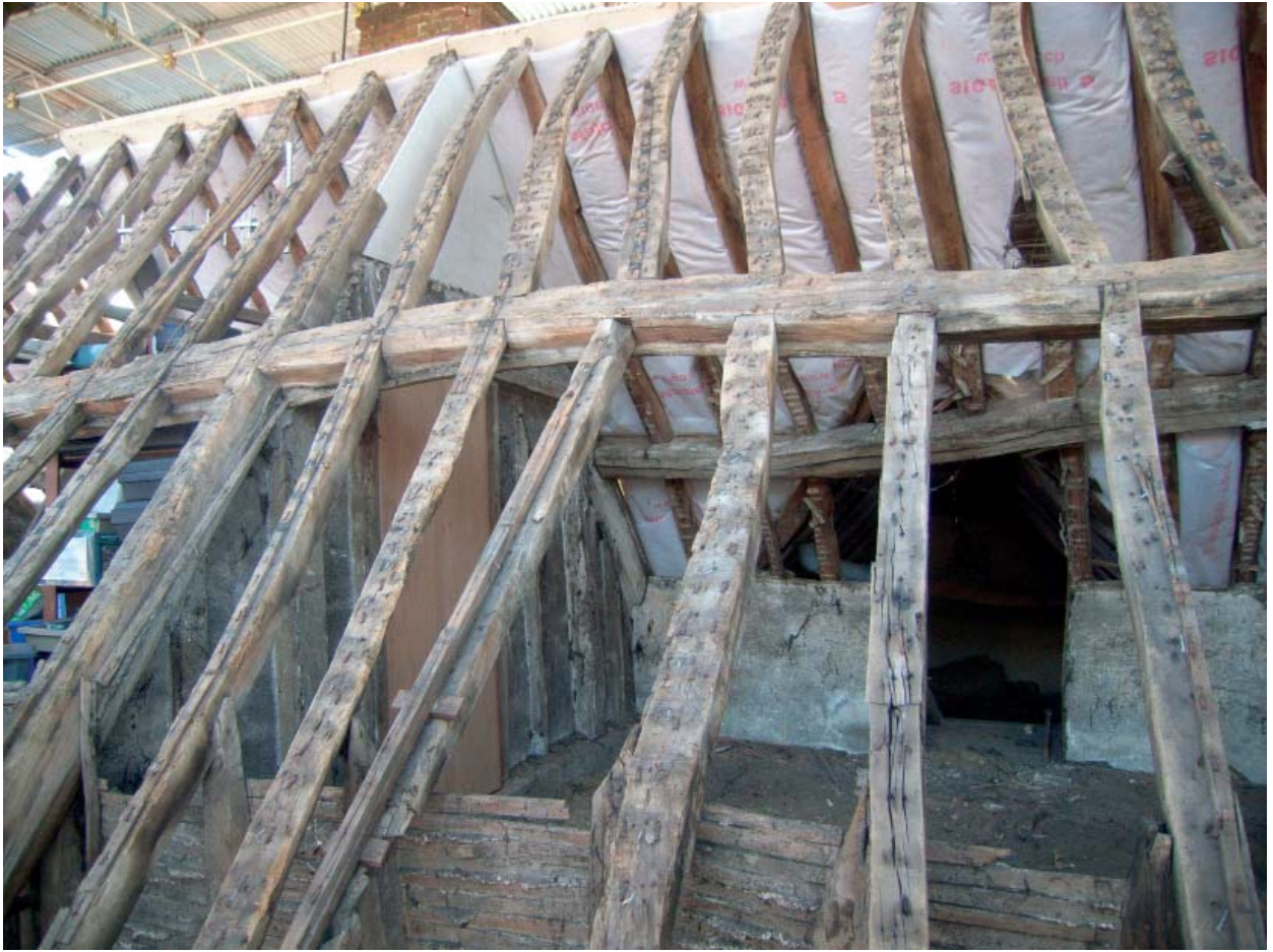
Plate 37: Roof of No.5-7
