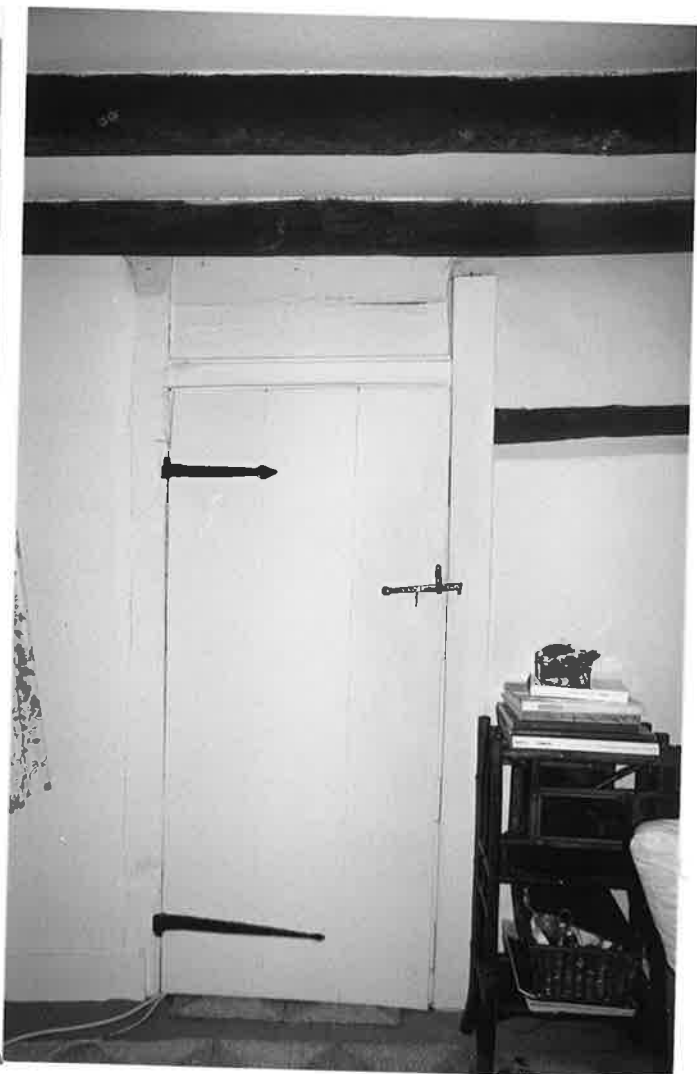
EARLY LEDGED AND BRACED DOOR,
