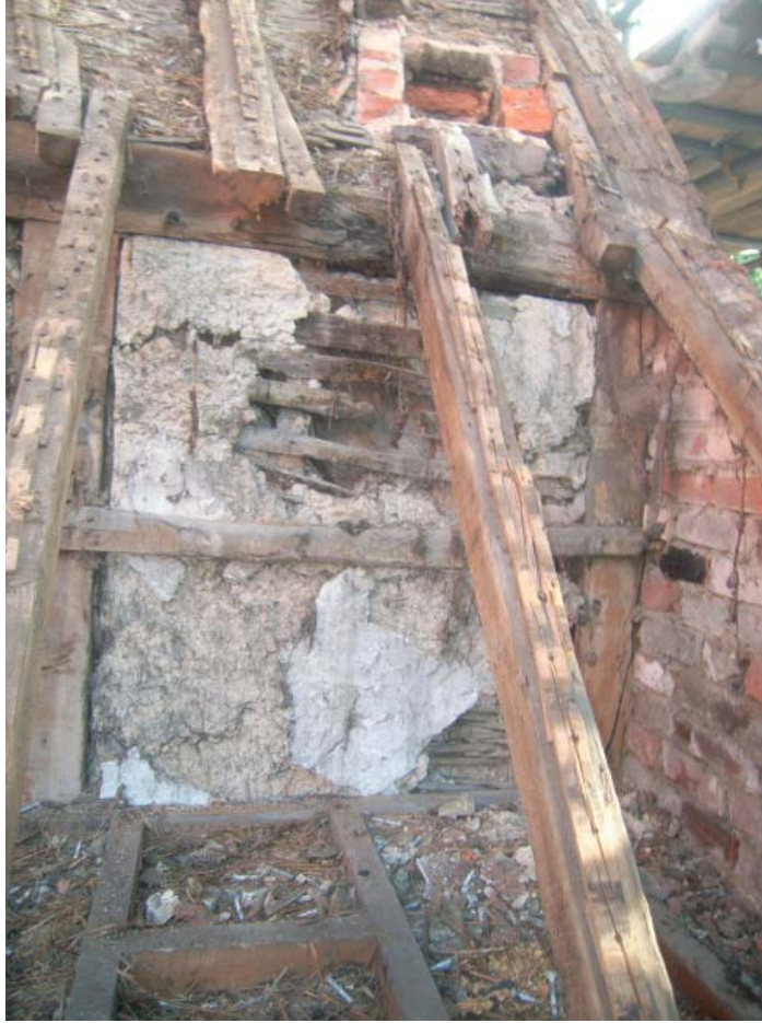
Plate 21: Rear of No.4, old laths (Block N)
