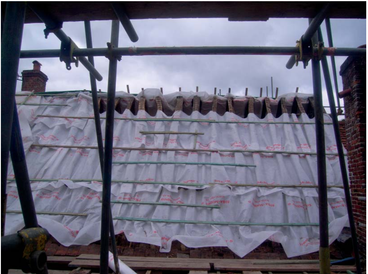
Plate 72: Rear slope general of No.3
