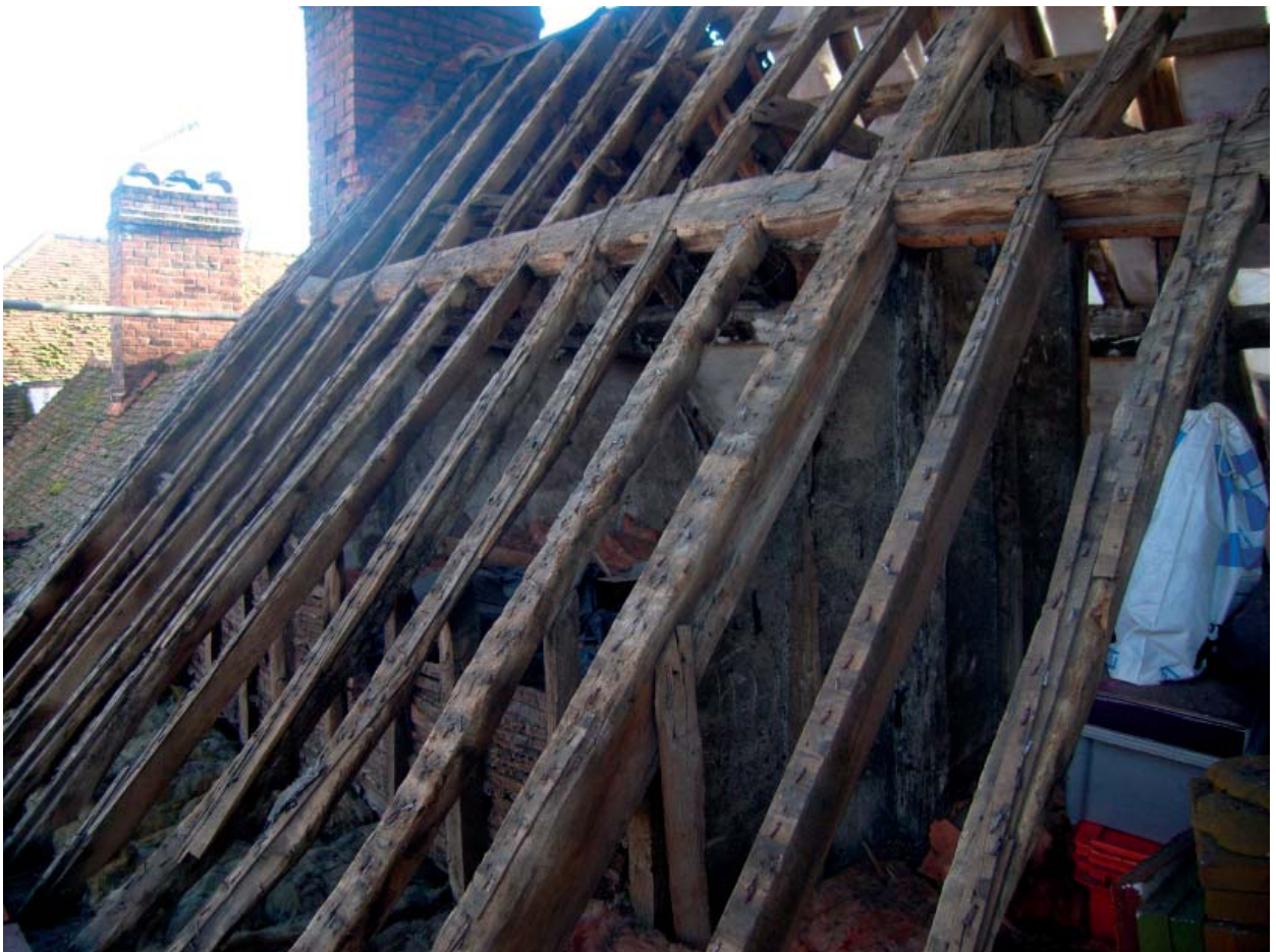
Plate 30: Roof of No.5-7 looking east towards the Swan Inn
