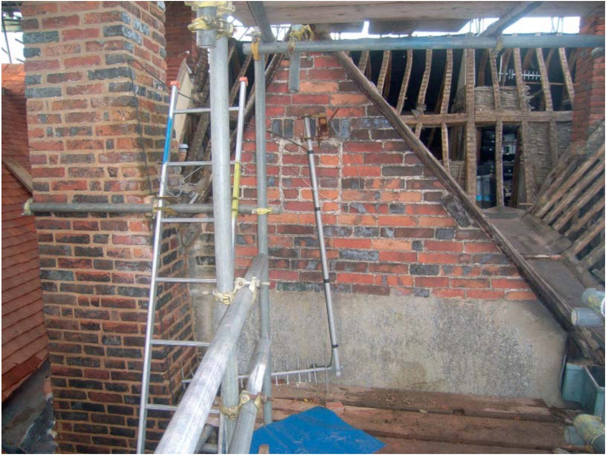
Plate 49: End of rear range of No.5-7 (Block K)
