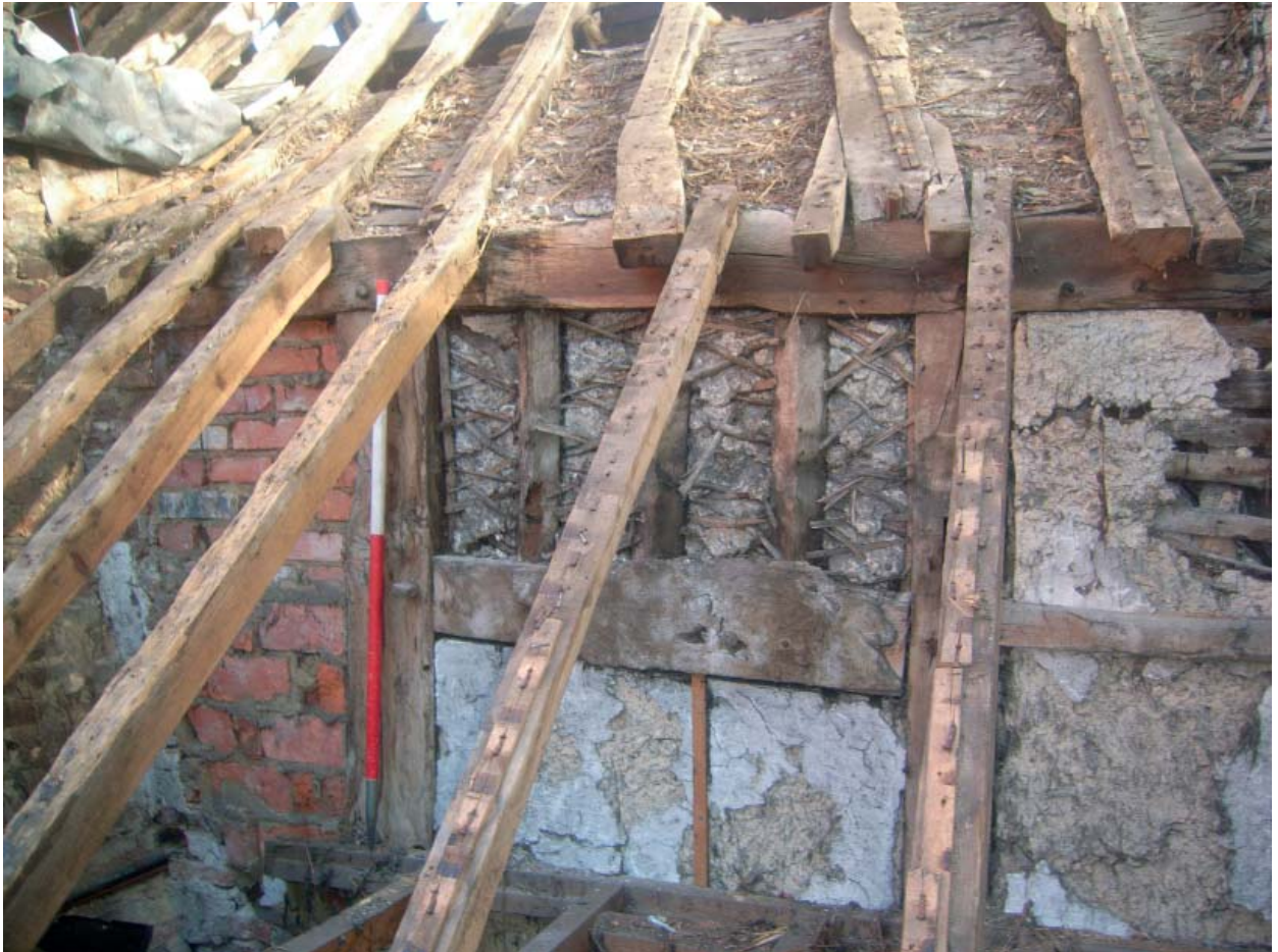
Plate 19: Side of wall of rear range (Block N)
