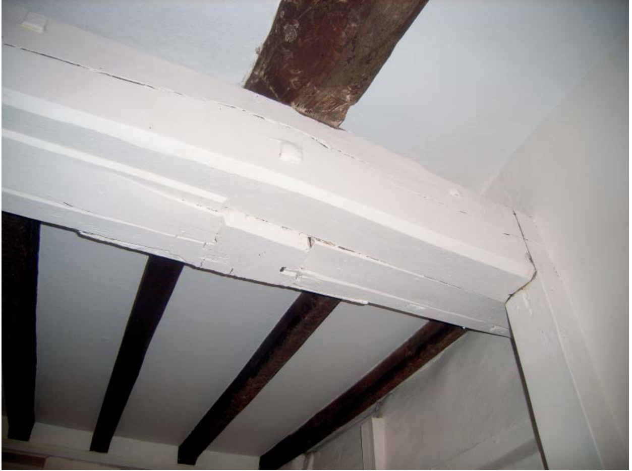
Plate 89: No 4. Underside of truncated post. Rear wall
