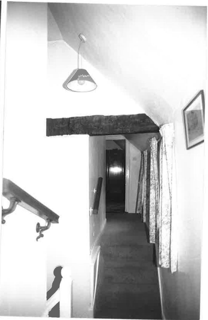
ORIGINAL TIE BEAM VIEWED FROM LANDING G. R173 N33 A.
