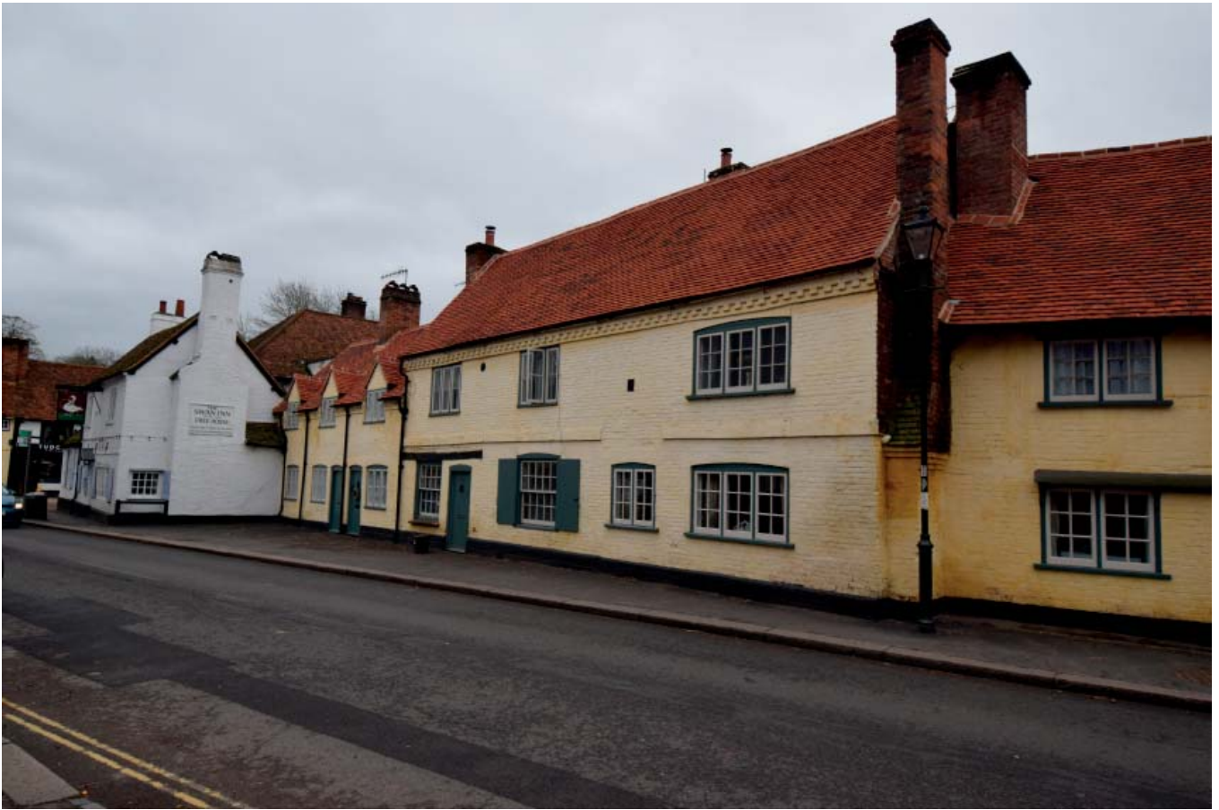
Plate 3: North elevation of No's 5-8
