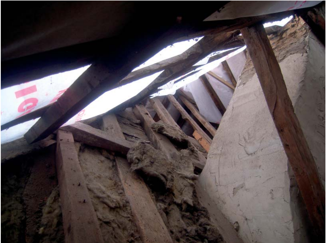
Plate 57: Roof space of No.2-3 (Front range – Block T)
