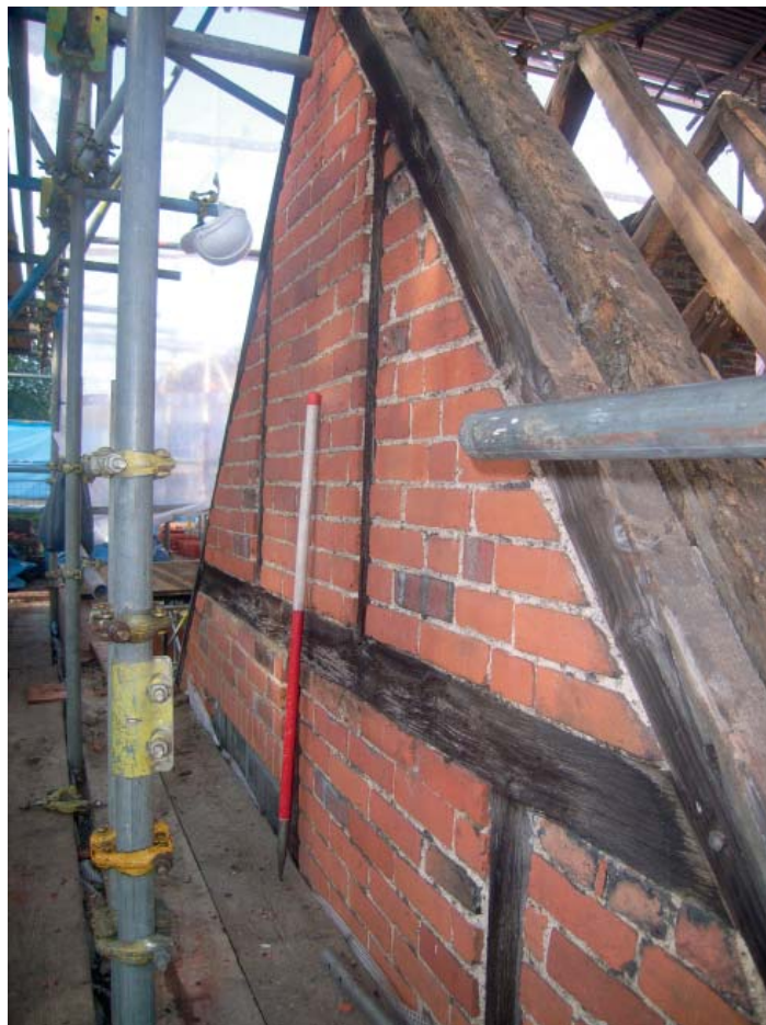
Plate 14: End of south projection of No.4 (Block N)
