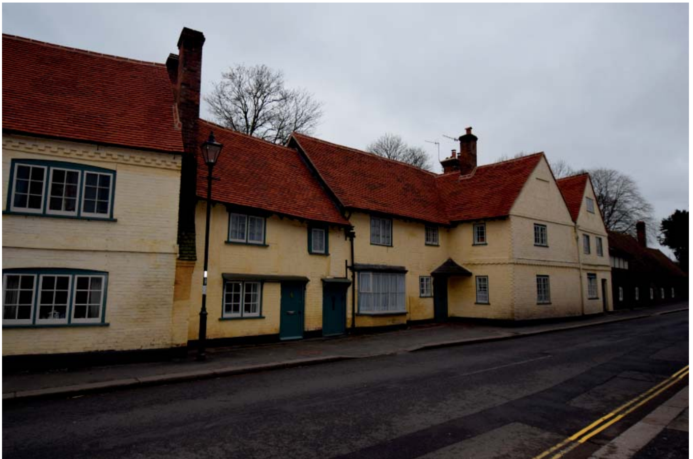
Plate 2: North elevation of No's 2-5
