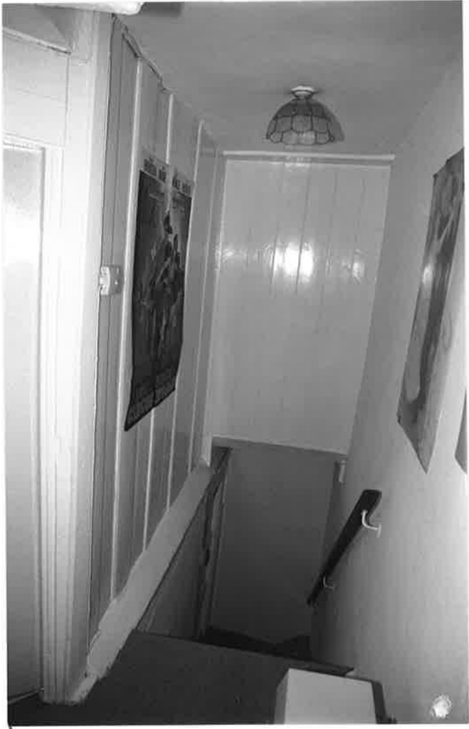
STAIRS, VIEWED FROM LANDING, ROOM H. R177 N18.
