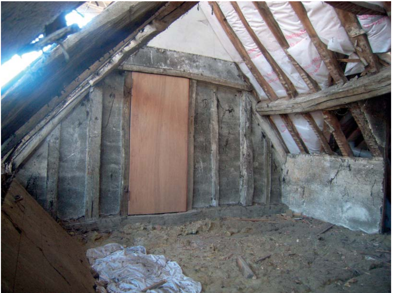
Plate 40: Roof space of No.5-7 looking east
