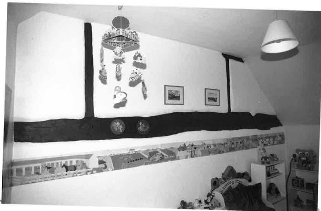
PART OF ORIGINAL TRUSS, ROOM H. R173 N32 A.
