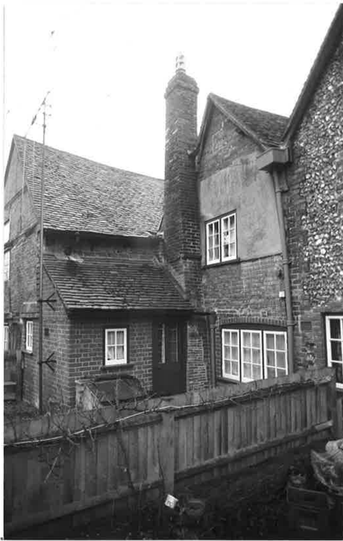
No 5, REAR ELEVATION, VIEWED FROM SOUTH- EAST, WINGS K AND N R.175 N 18
