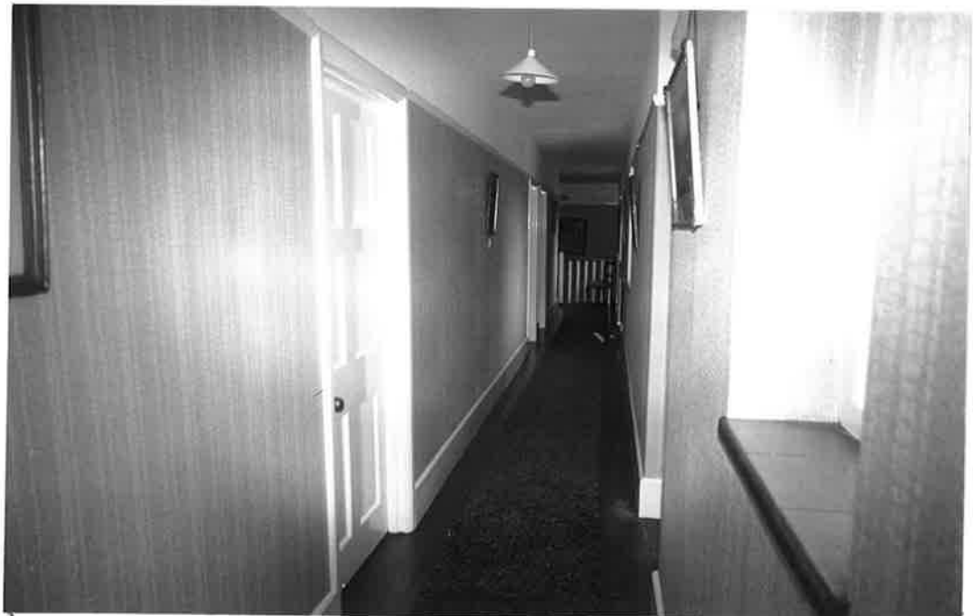
LANDING, ROOM 0, LOOKING SOUTH-WEST.
