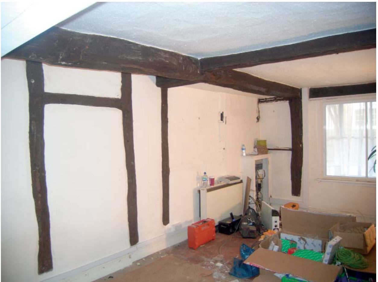
Plate 82: No 4. Ground floor front room looking north
