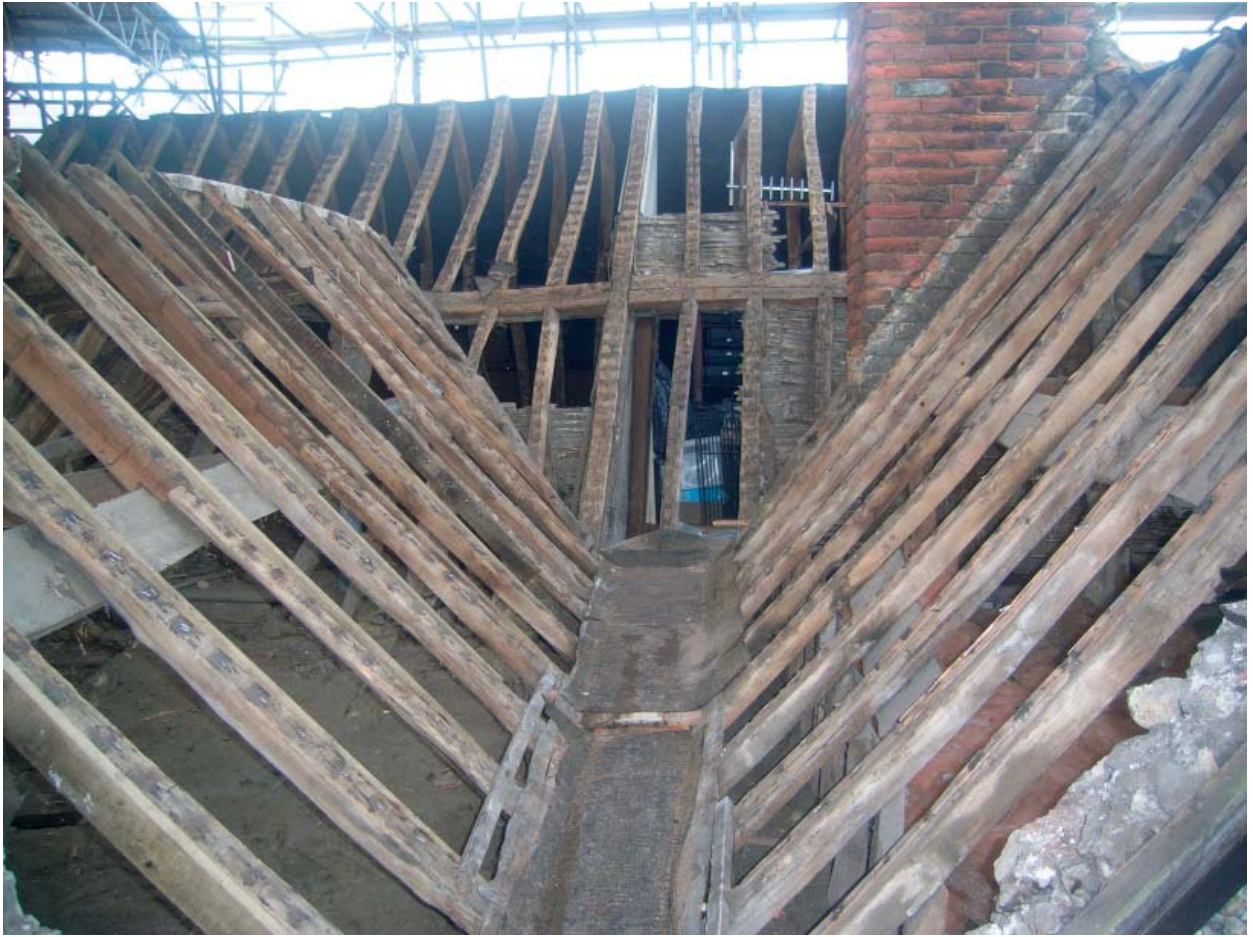
Plate 51: Rear slope of No.5-7
