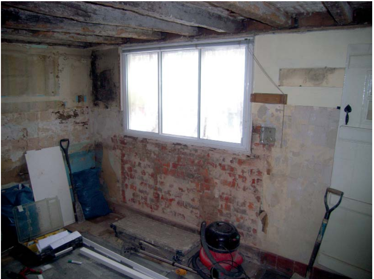
Plate 74: Interior of No 2 front room ground floor
