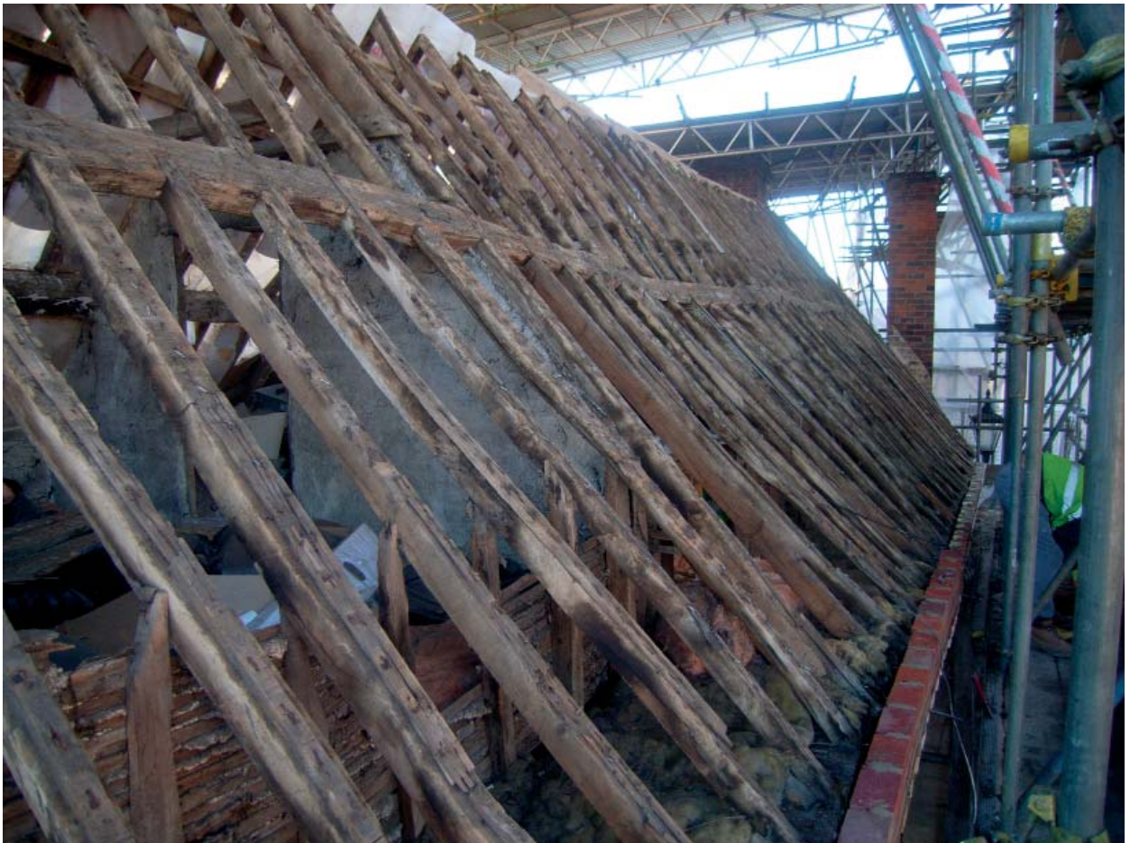
Plate 28: General view of roof of No.5-7 looking west
