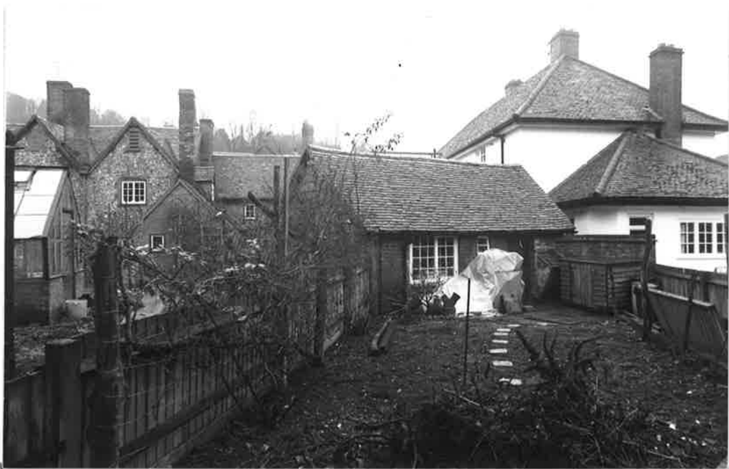
BUILDING Nº5, VIEWED FROM SOUTH-EAST. R173 N23A.
