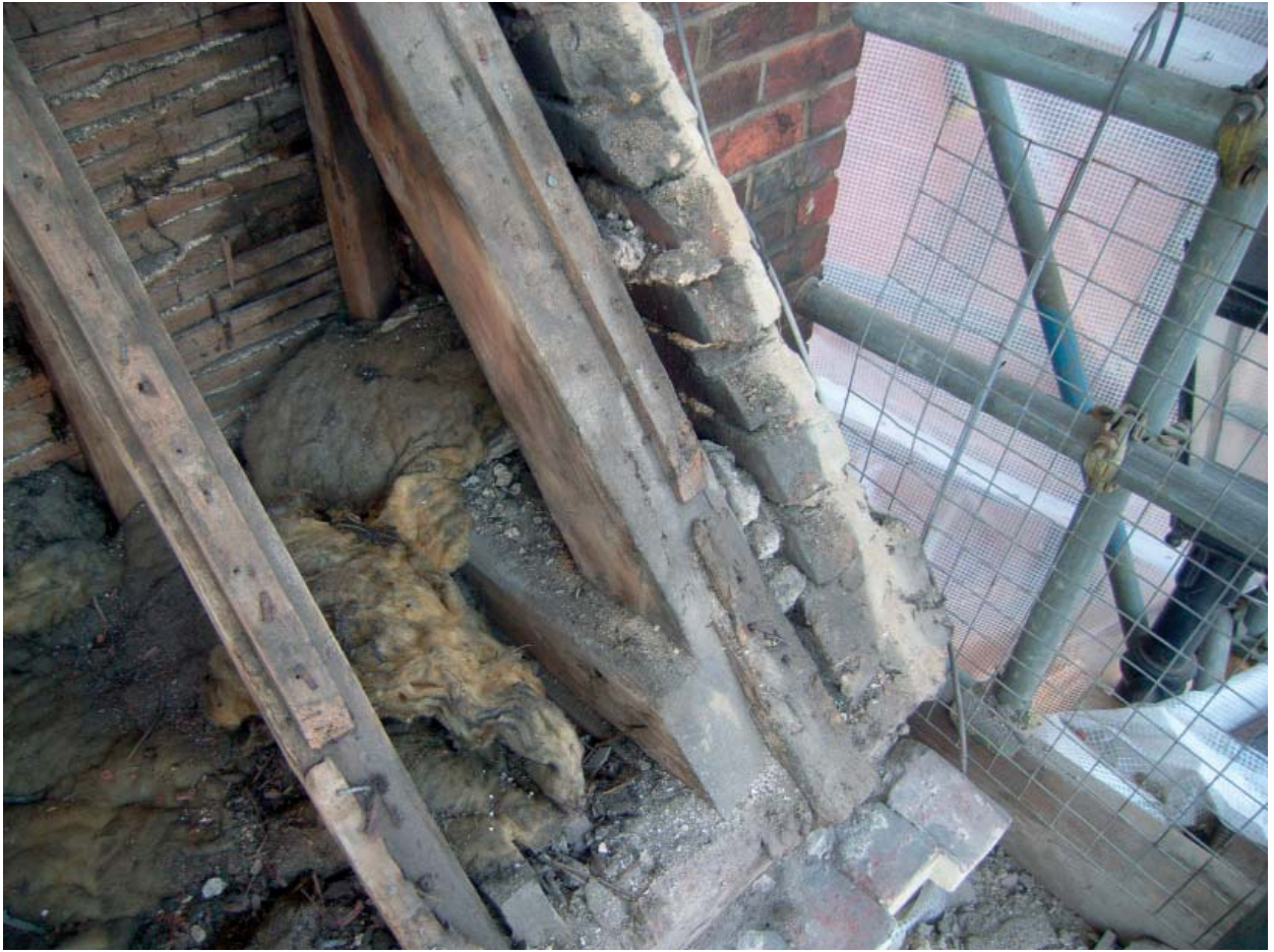
Plate 39: Roof of No.5-7, corner detail
