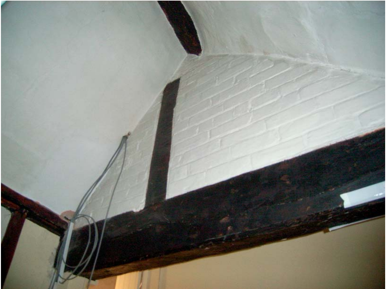
Plate 93: No. 4. Roof at first floor
