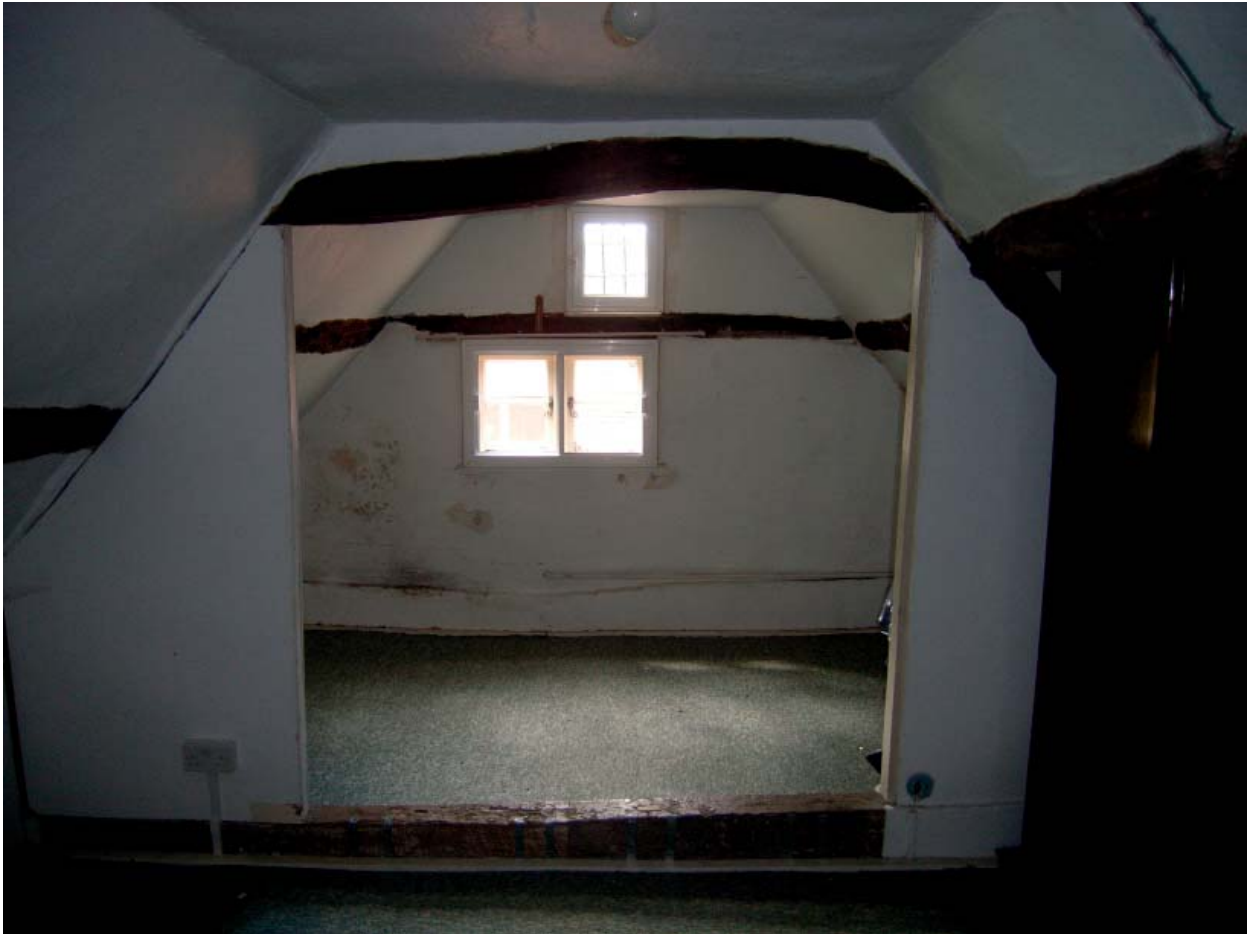
Plate 79: Interior of No 2. Attic looking north
