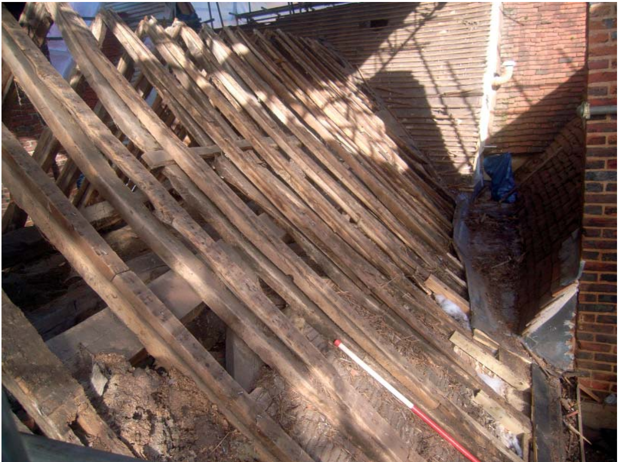
Plate 6: General view of roof of No.4
