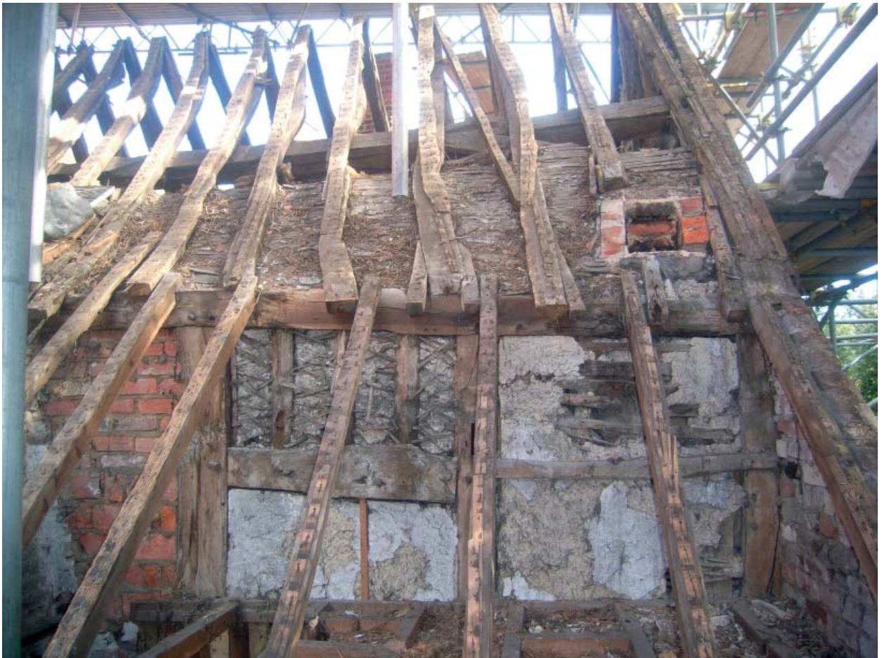
Plate 20: Rear of No 4 showing exposed old features (Block N)
