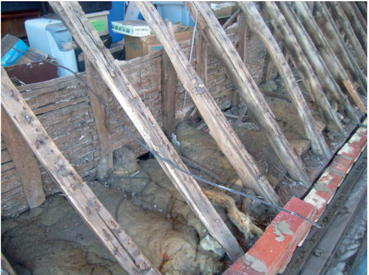
Plate 32: Rafters and purlin of roof of No.5-7
