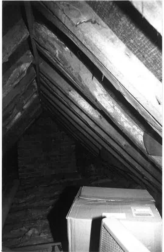
NO 8 HIGH STREET - INTERNAL ROOF SPACE LOOKING EAST. R173 N19A.
