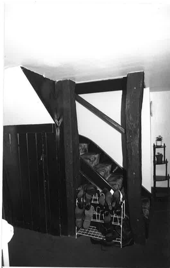
STAIRS, VIEWED FROM ENTRANCE HALLWAY, ROOM F. R176 N7A.
