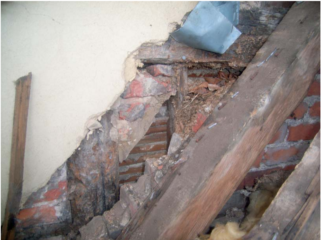
Plate 24: Blocked window at east end of No.4 (Block P)
