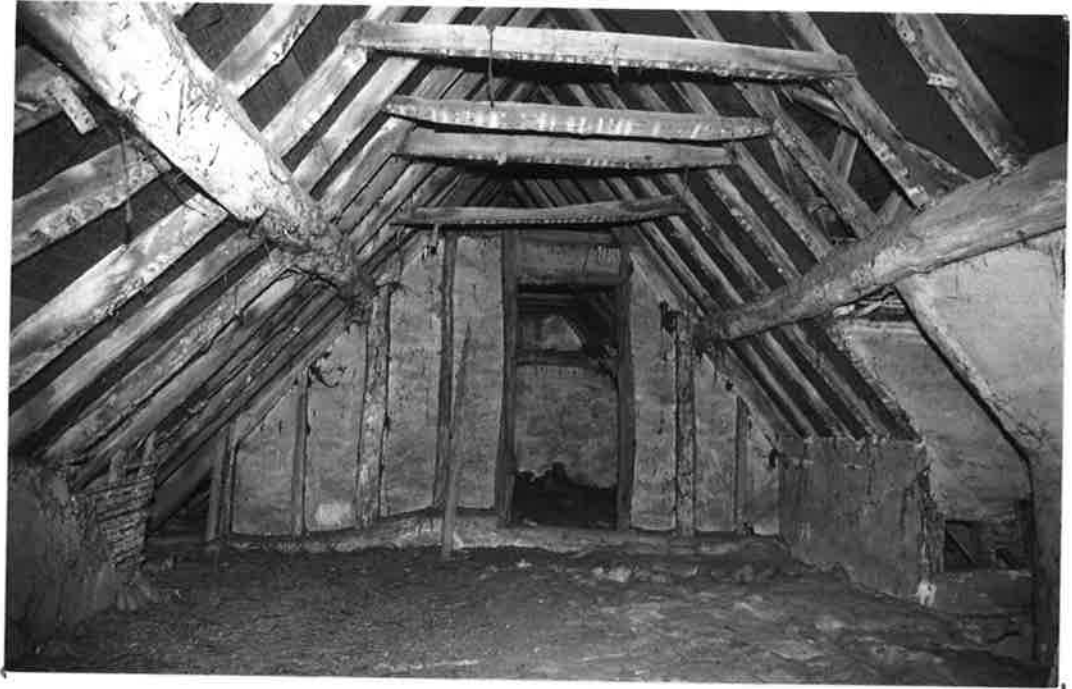
Nº7 HIGH STREET - ROOF STRUCTURE, MAIN BLOCK LOOKING EAST. R175 NO.
