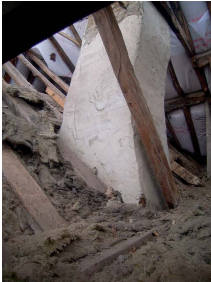
Plate 58: Roof space of No.2-3 (Front range – Block T)
