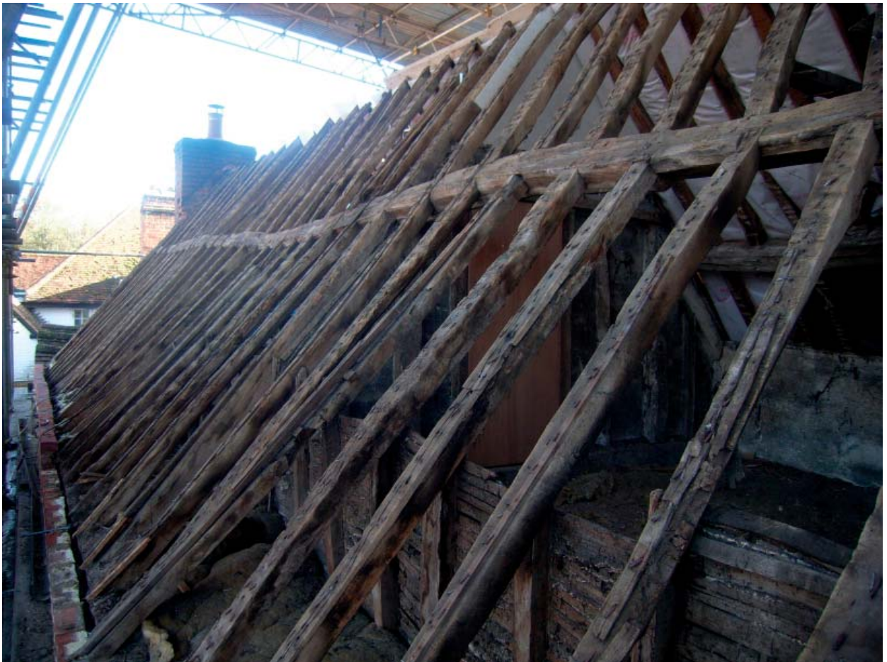
Plate 38: Roof of No.5-7 looking east
