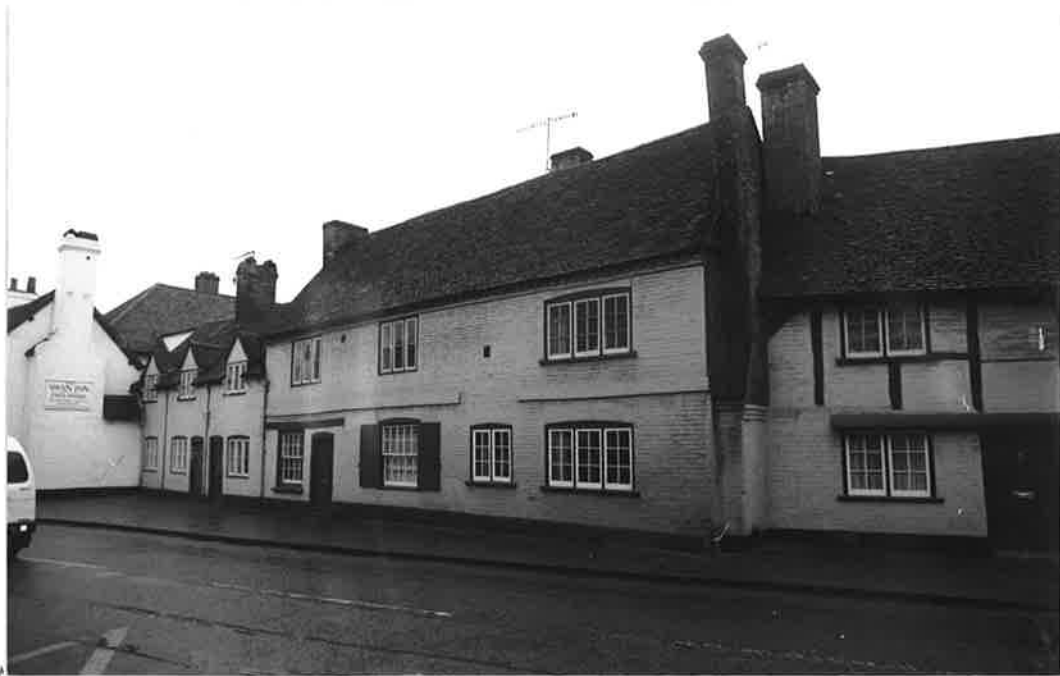
NOS 5 AND 7, BLOCK L, VIEWED FROM NORTH-WEST R. 175 N 10
