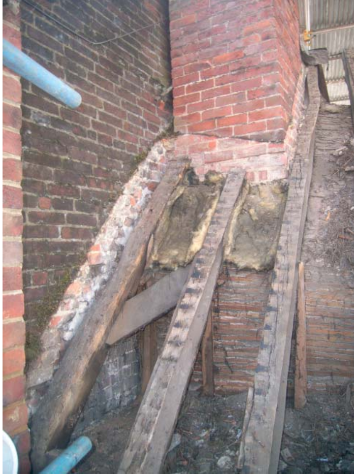
Plate 25: Front slope of No.4 at junction with No.5
