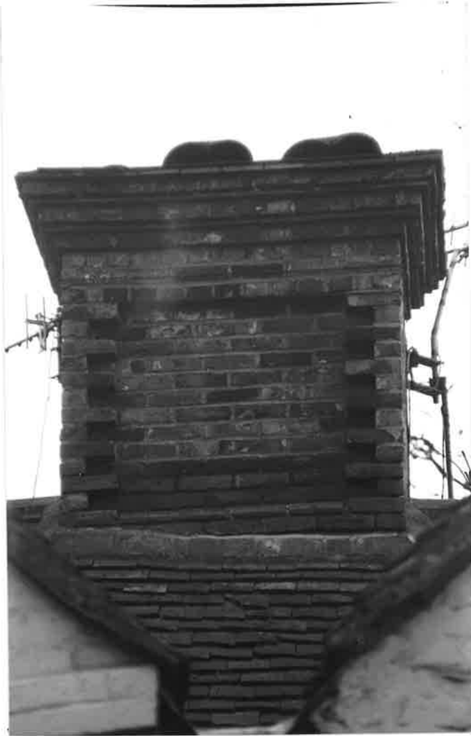
DECORATIVE CHIMNEY STACK, NOS 2 AND 3, BLOCK 5, VIEWED FROM NORTH.
