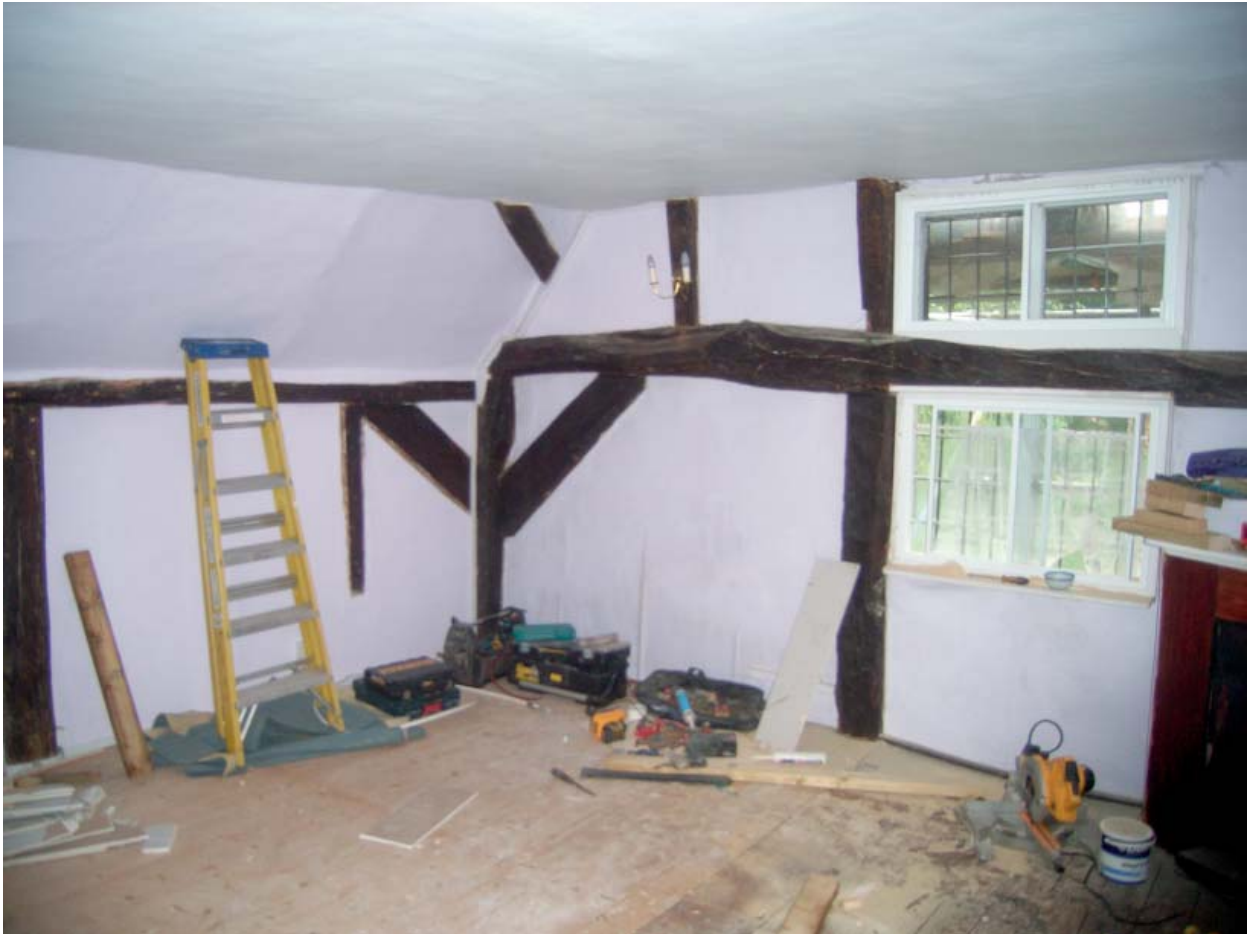
Plate 95: No. 4. First floor rear projection looking south
