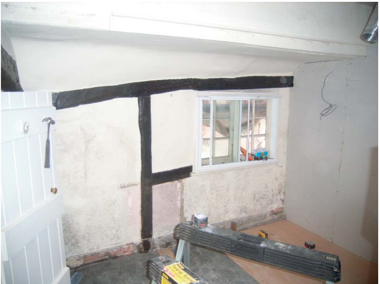
Plate 94: No. 4. First floor rear wall
