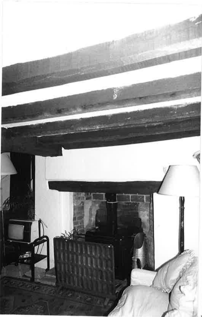
FIREPLACE, ROOM D. R178 N15A.
