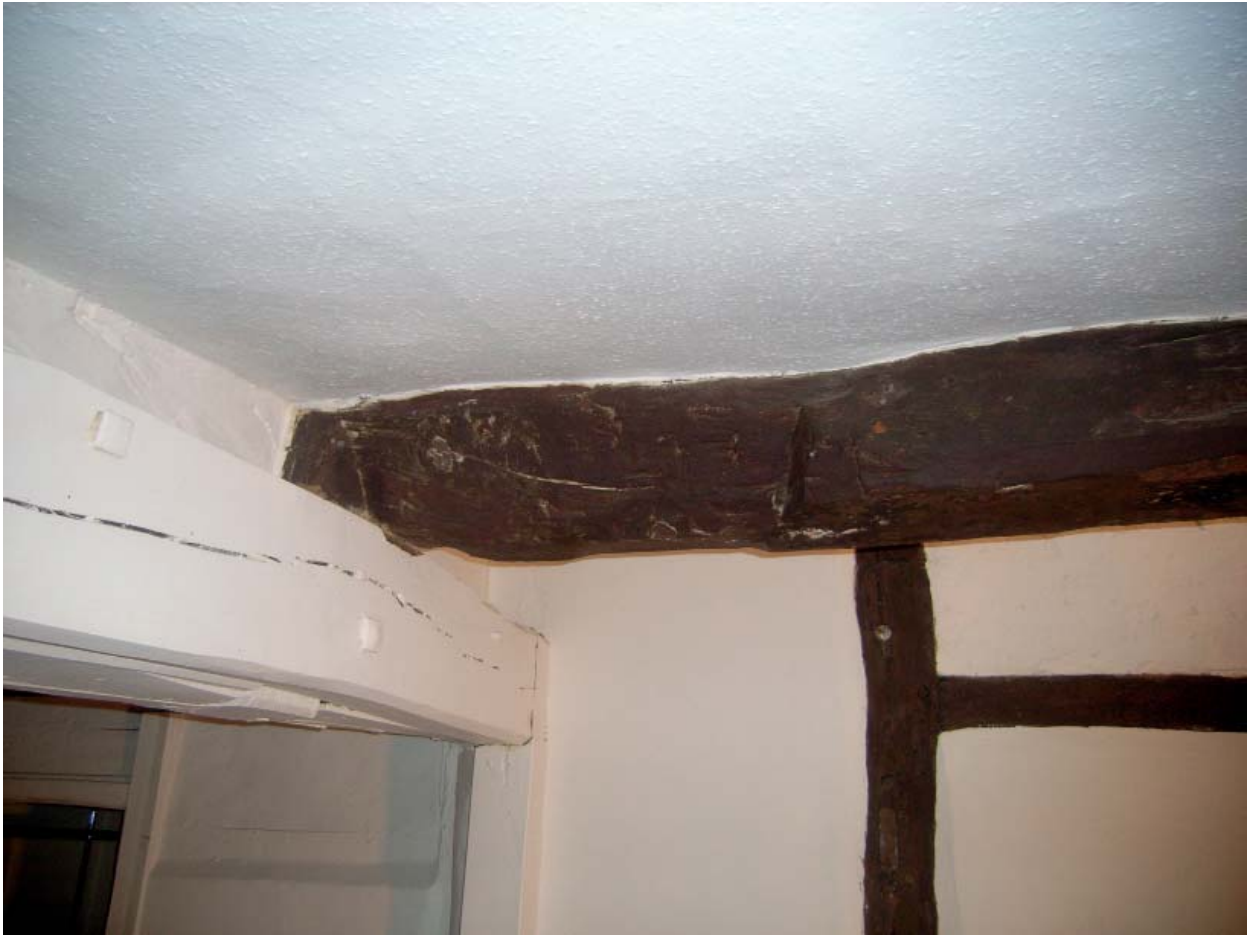
Plate 83: No 4. Ground floor front room looking west
