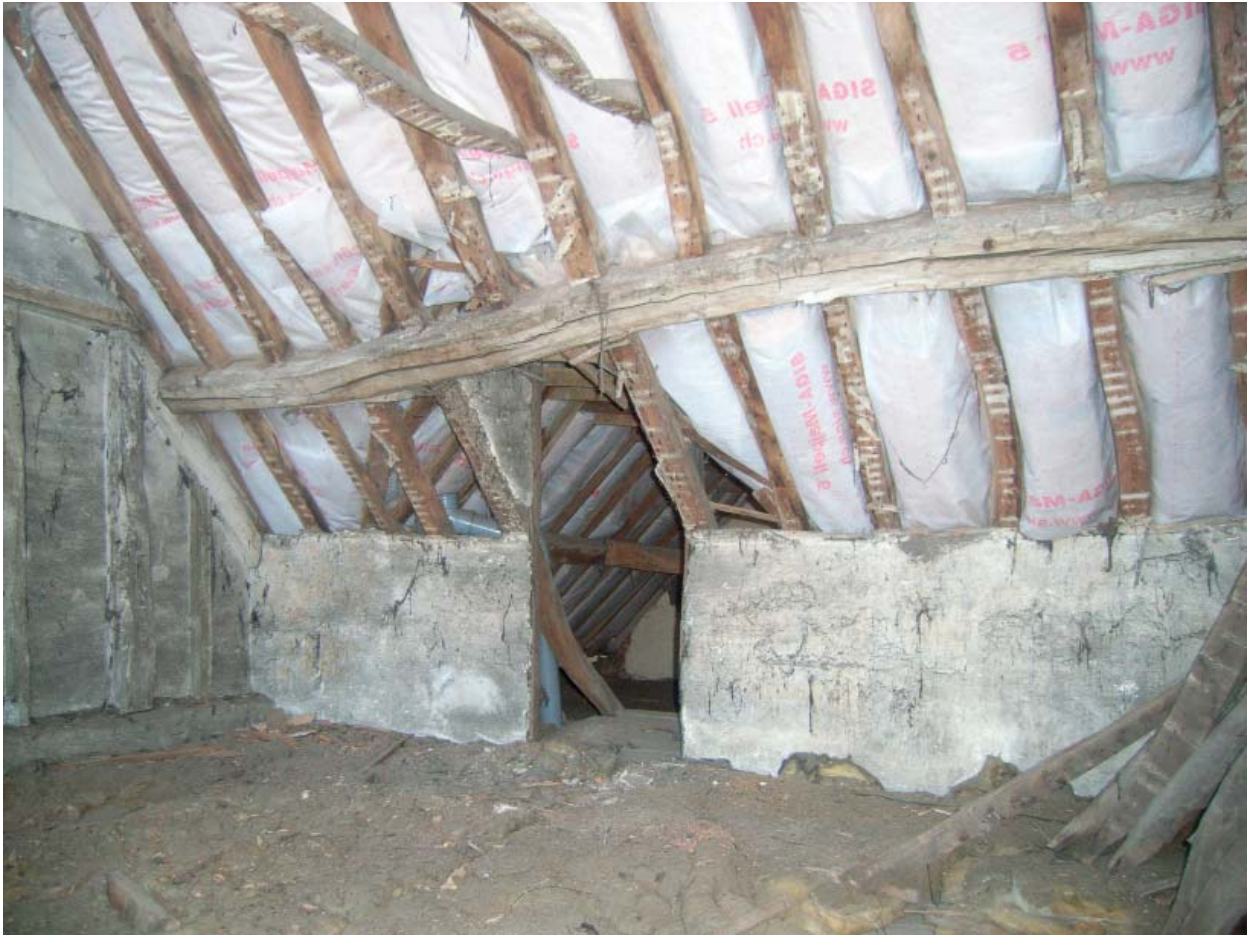
Plate 41: Roof space of No.5-7 towards rear range
