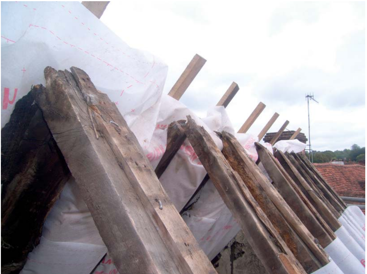
Plate 70: Apex of rafters in No. 3
