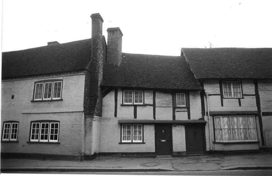
No. 3. 4 AND 5 FRONT ELEVATION (BLOCK P TO CENTRE OF PHOTOGRAPH.) R 176 N 4A
