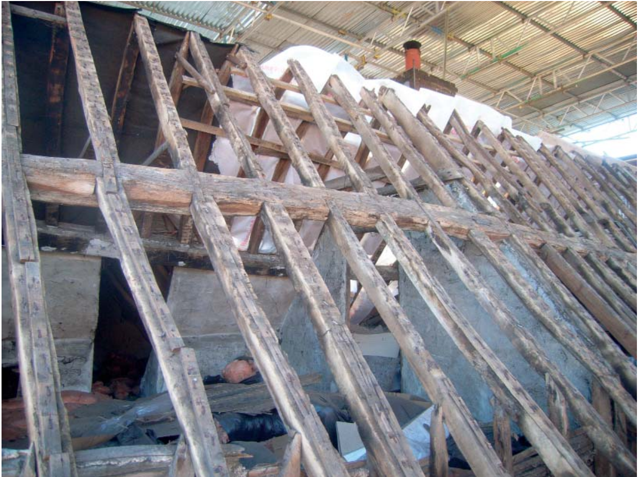
Plate 29: General view of roof of No.5-7. Butt purlins
