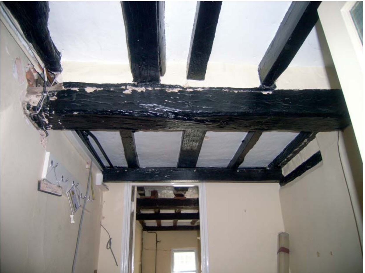
Plate 76: Interior of No 2. Former passage
