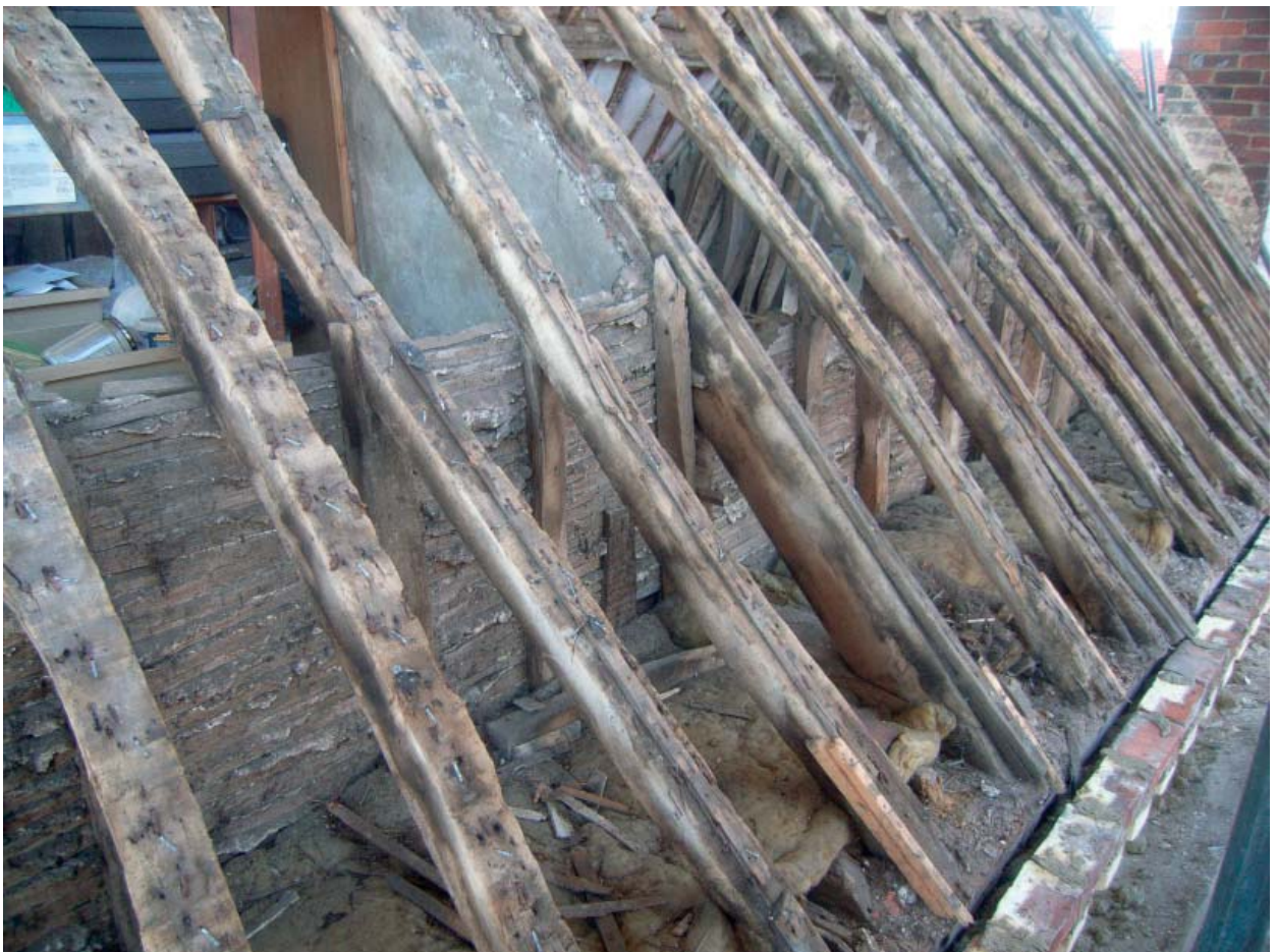
Plate 34: General view of roof of No.5-7
