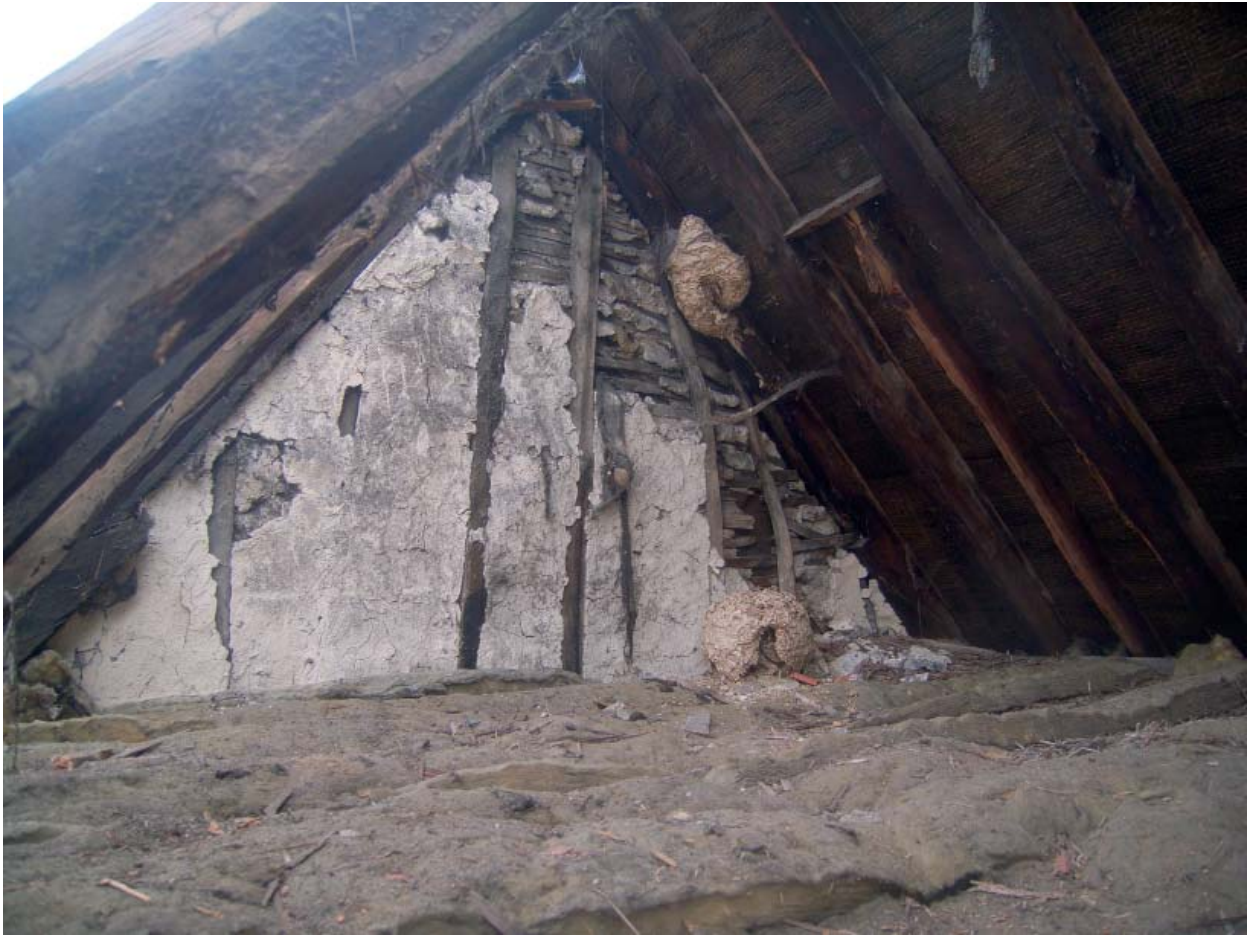
Plate 61: Old plaster, looking east in roof space of No.2-3
