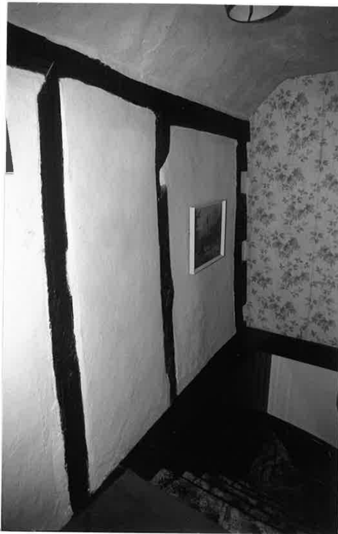
SOUTH WALL, LANDING ROOM H. SHOWING RE-USED TIMBERS. R.176 N10A
