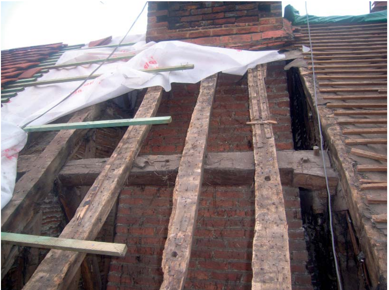
Plate 64: Rear slope of No.2
