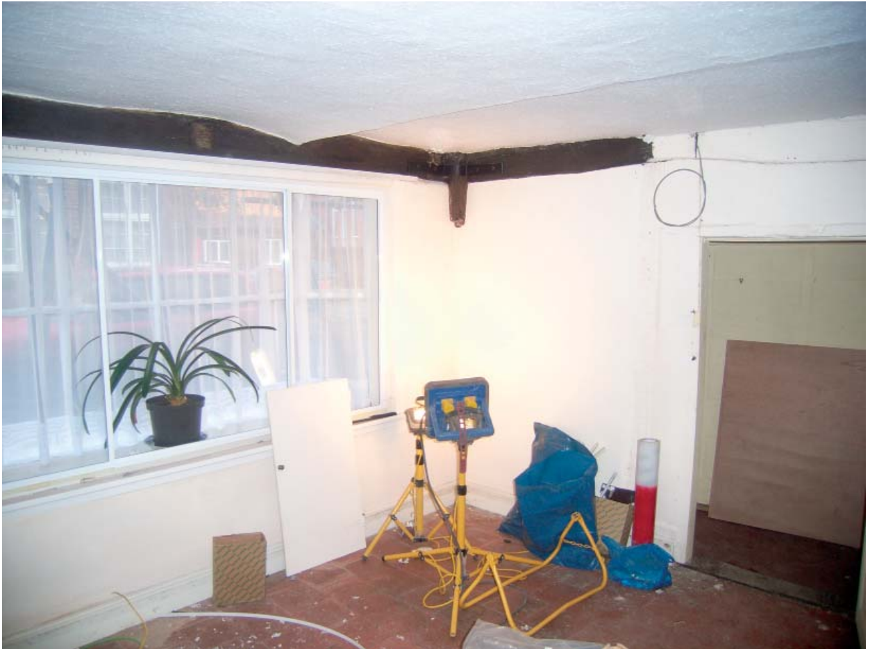
Plate 85: No 4. Ground floor front room, north-east corner
