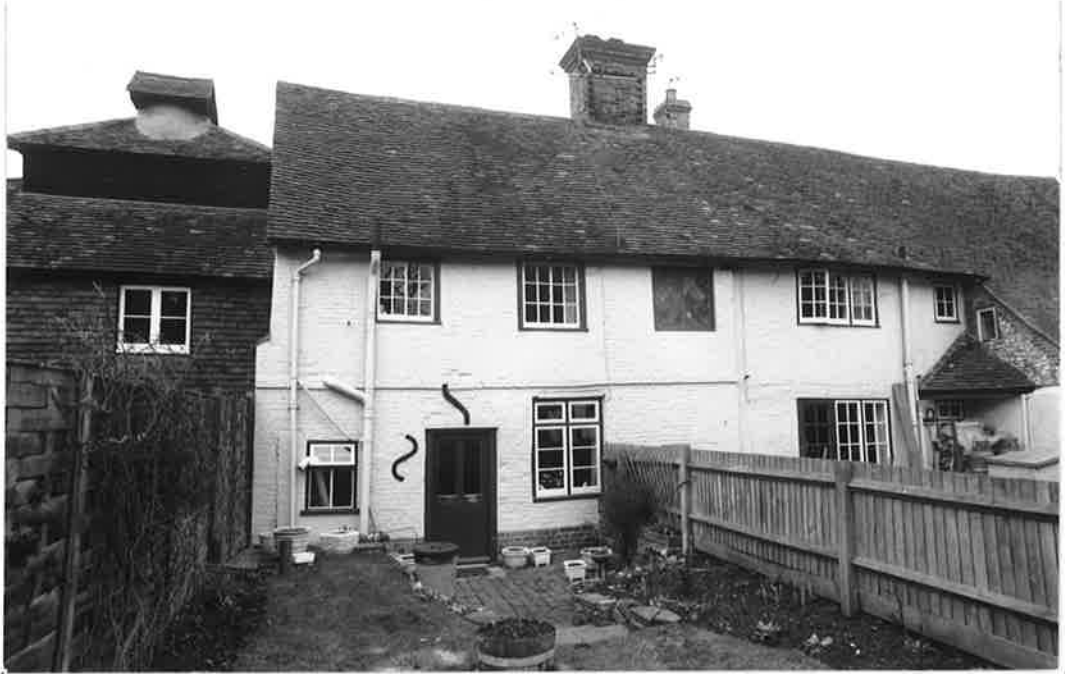
NOS 2 AND 3, BLOCKS S AND R, VIEWED FROM SOUTH-WEST. R. 177 N 28
