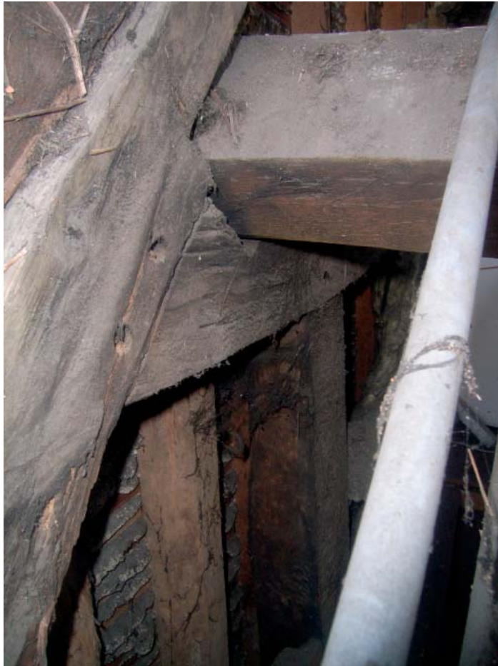
Plate 22: Clasped purlin in No.4 (Block R)
