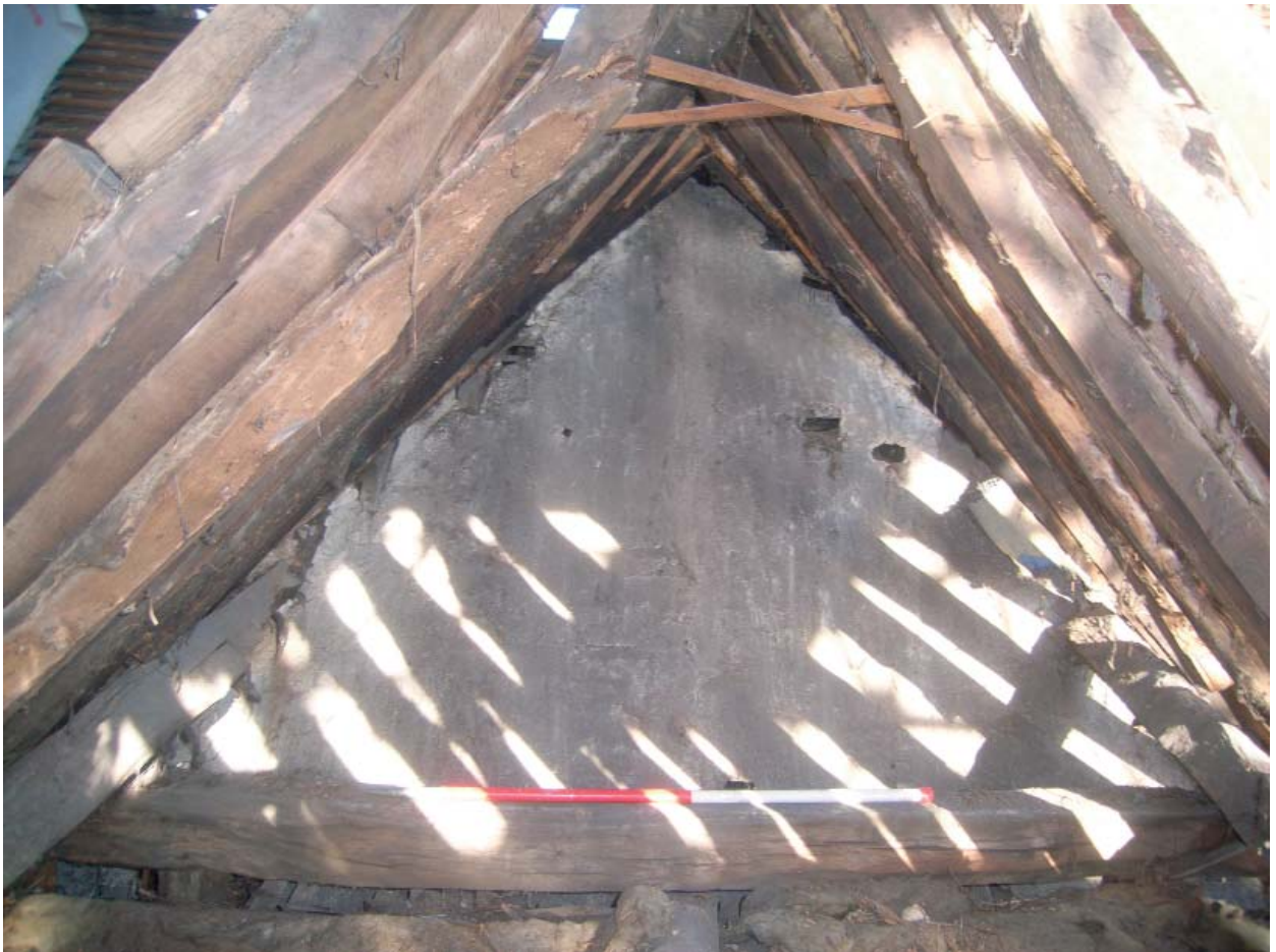
Plate 12: Loft space of No.4 (N end of Block N)
