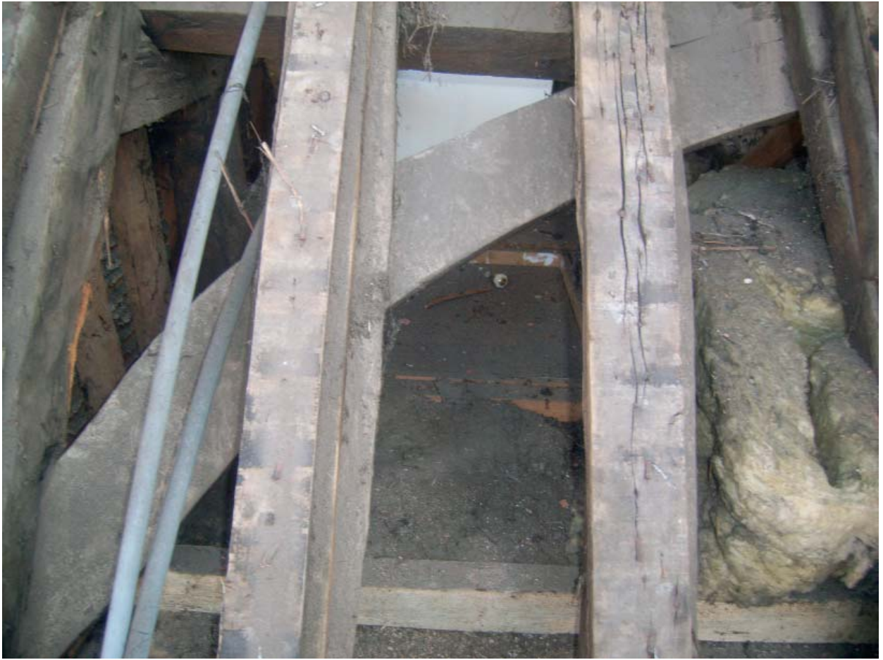
Plate 11: Curved wind brace in street-front range of No.4 (Block R)
