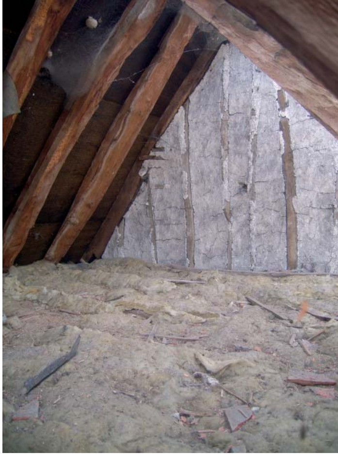
Plate 59: Roof space of No.4 (east end of Block R)
