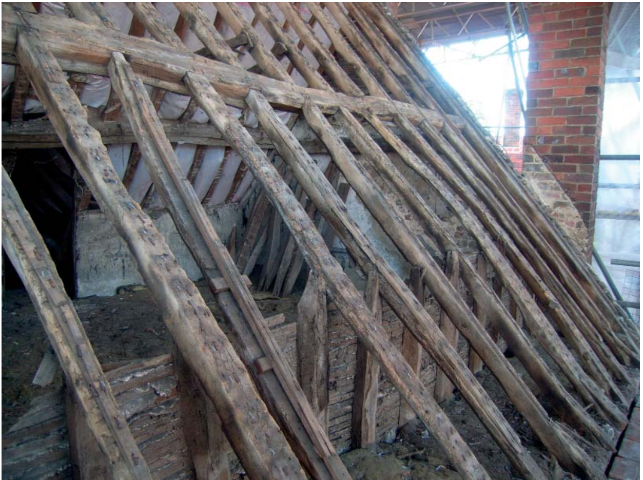
Plate 36: Roof of No.5-7 looking west
