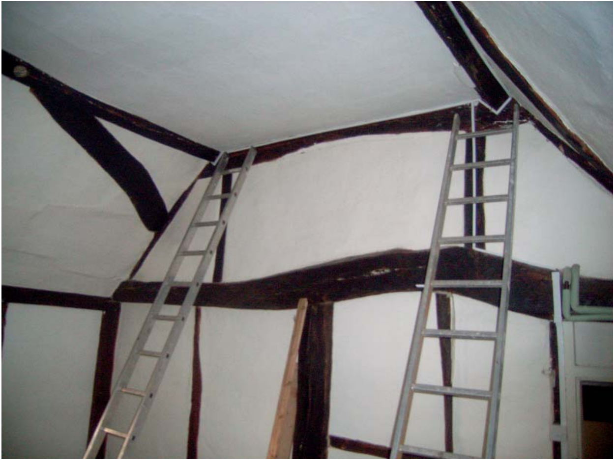
Plate 99: No. 4. First floor main range roof
