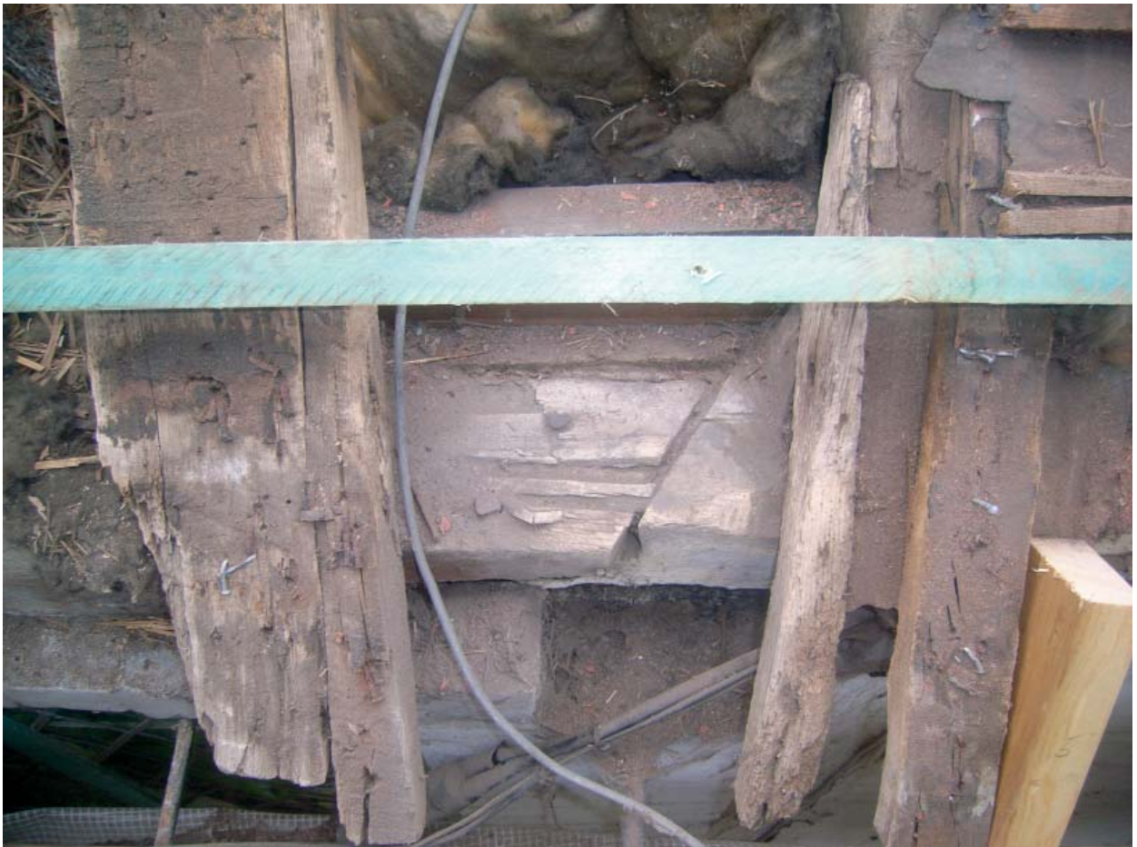
Plate 66: Scarfed purlin in roof of No.2-3
