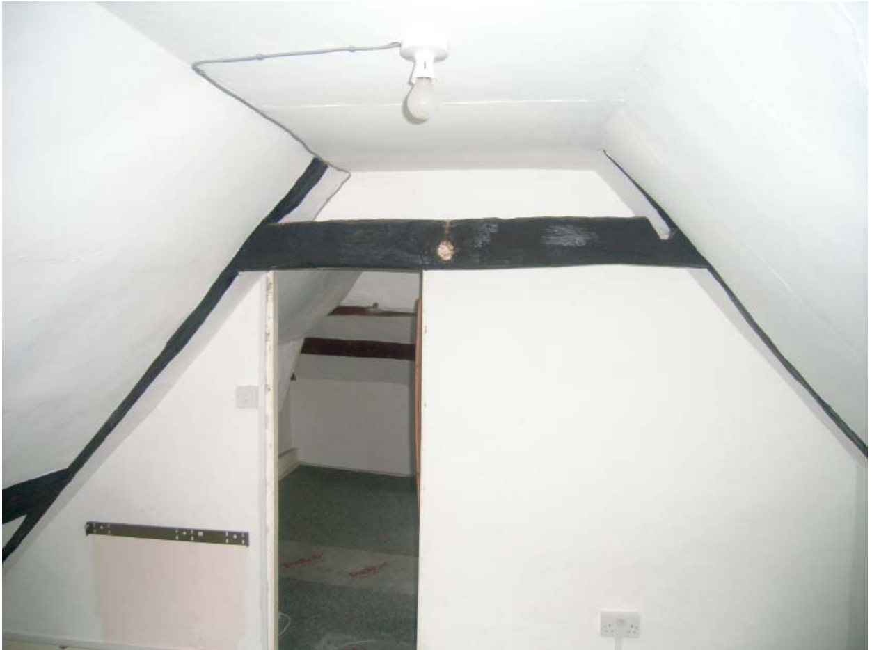
Plate 81: Interior of No 2. Attic looking west
