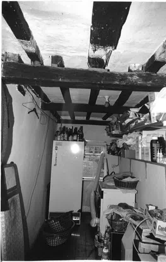
ROOM B, LOOKING SOUTH. R177 N11.
