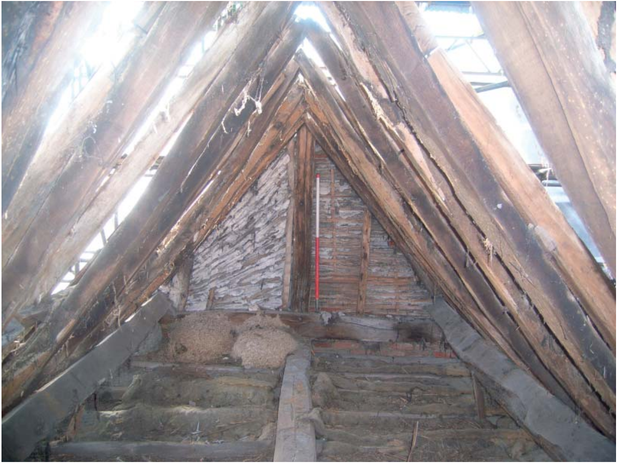
Plate 17: Plaster and wattle and daub in No.4 looking south (Block N)
