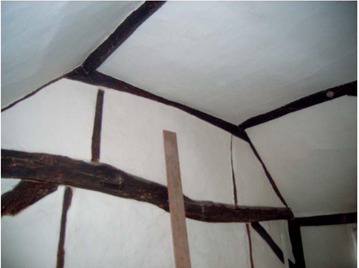
Plate 97: No. 4. First floor main range roof.
