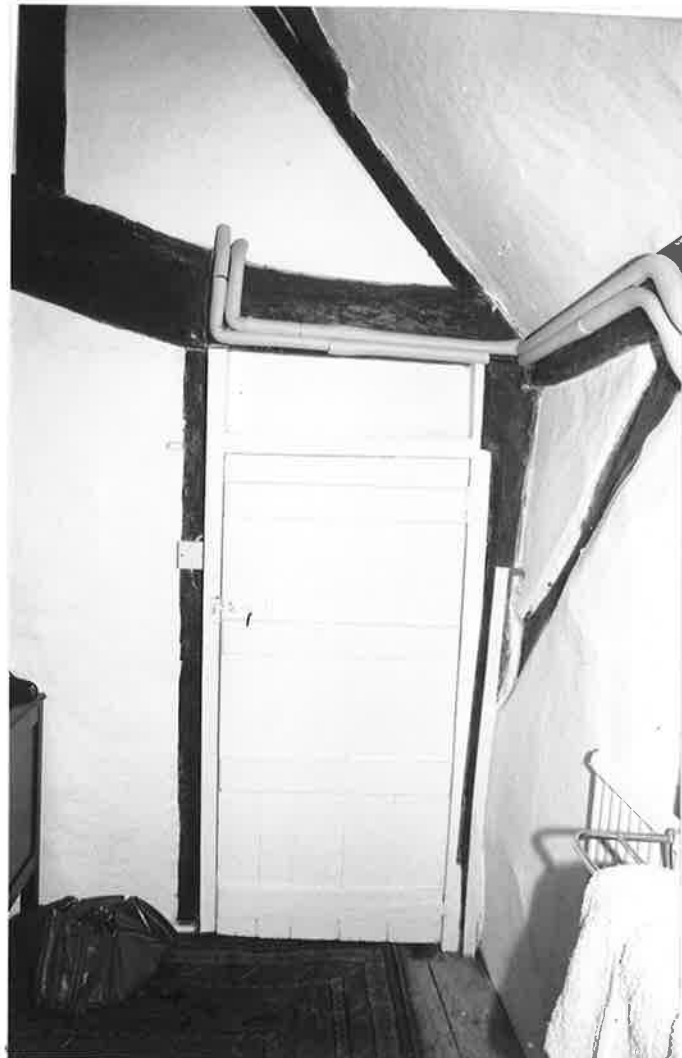
PERIOD FLANK AND BATTEN DOOR,
