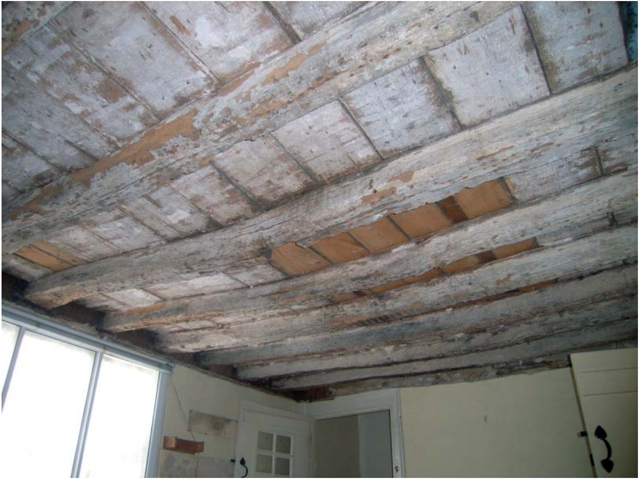
Plate 73: Interior of No 2. Joists in front room looking east
