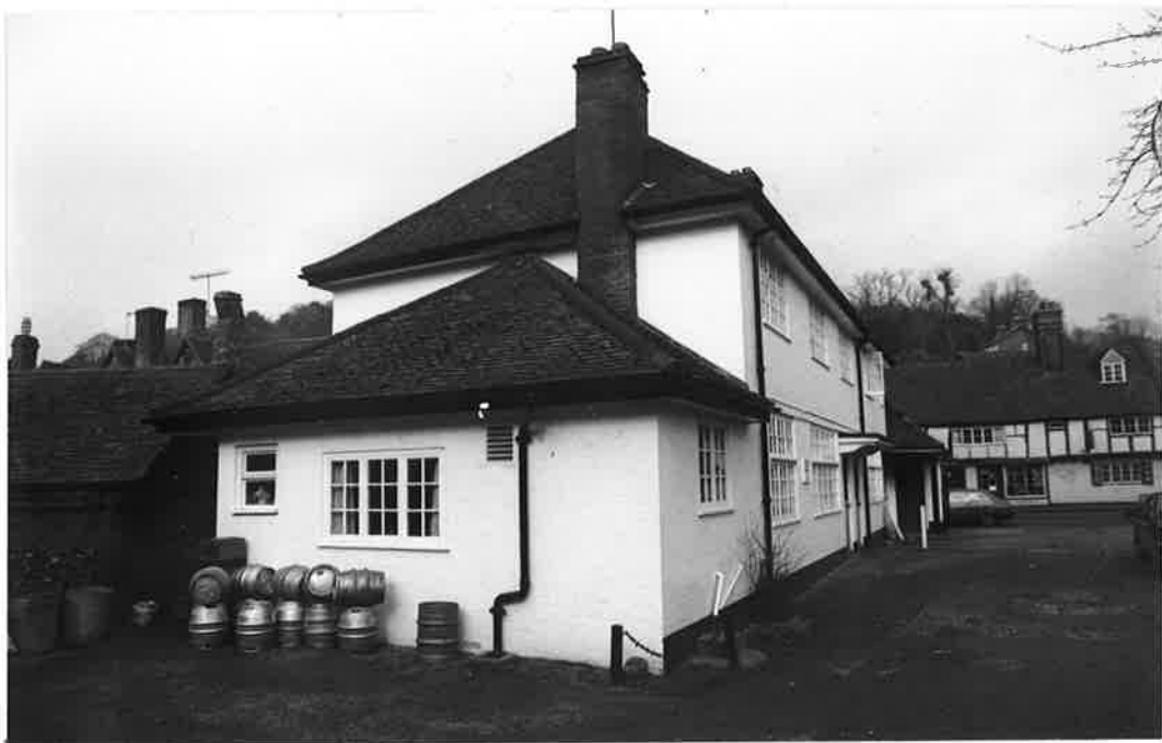
VIEW FROM SOUTH EAST, BLOCKS A AND B. R.176 N 29A
