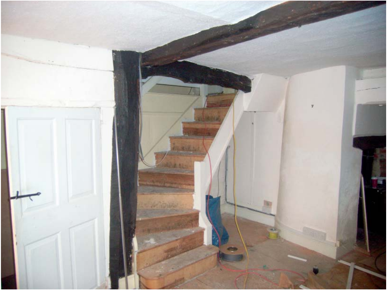
Plate 87: No 4. Ground floor front room looking south-east
