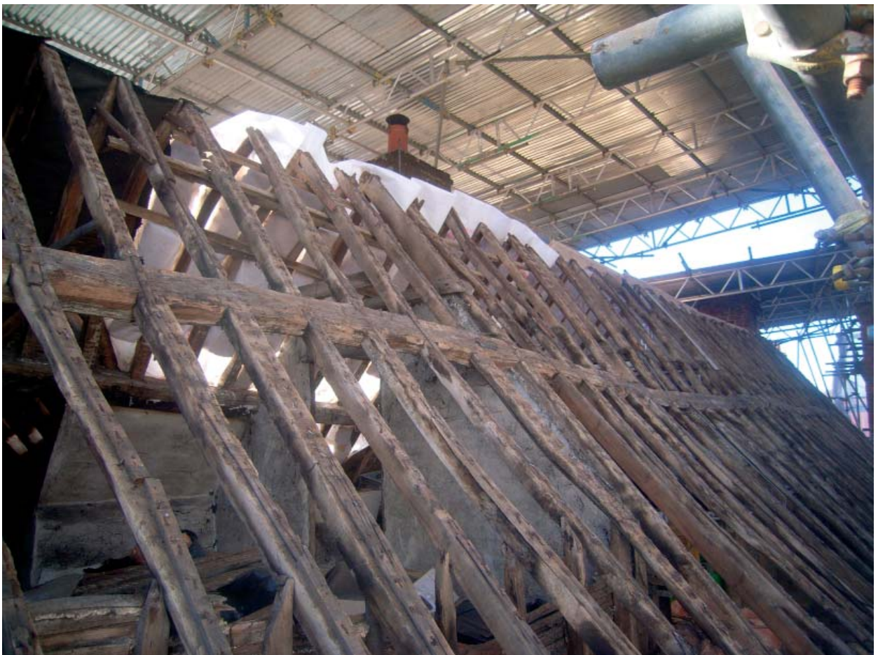
Plate 54: Rear slope of No. 5-7
