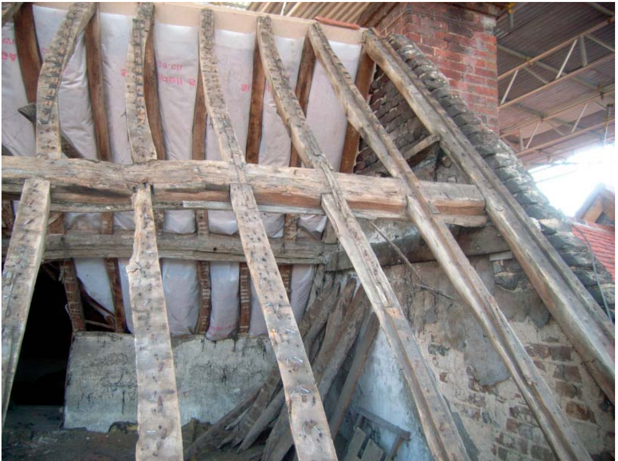
Plate 42: West end of roof of No.5-7
