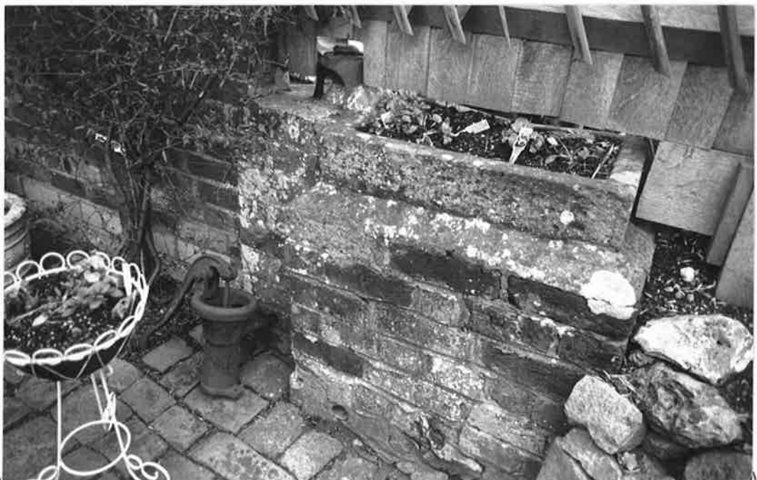
BASE OF WATER PUMP AND REMAINS OF CAST-IRON HAND PUMP SHARED BETWEEN COTTAGES NO 2 AND 3 R. 177 N 30
