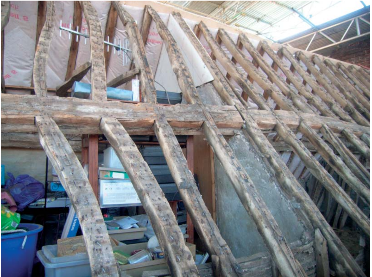
Plate 33: Roof of No.5-7
