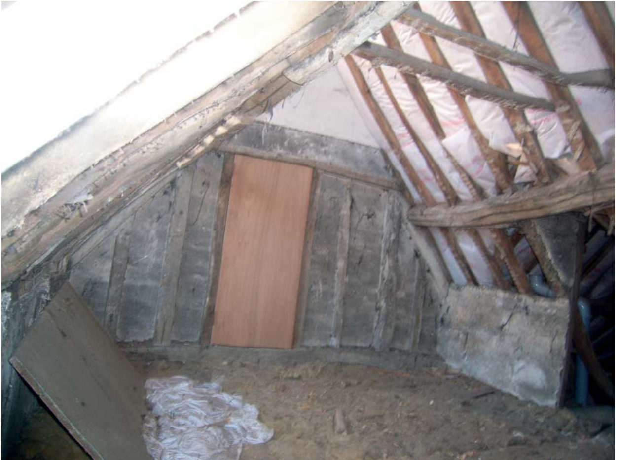
Plate 53: Roof space of No.5-7 looking east
