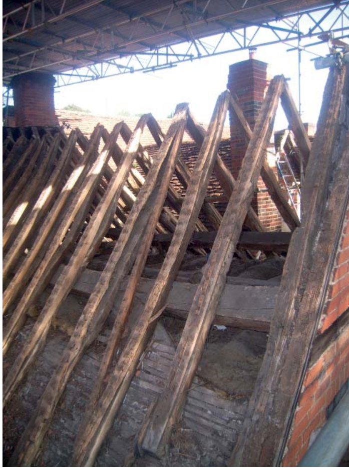
Plate 15: Roof of rear projection of No.4 looking east (Block N)
