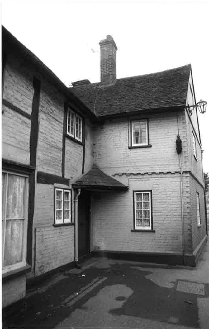
NO 3, VIEWED FROM EAST. PROJECTING FRONT WING T. R. 179 N 31
