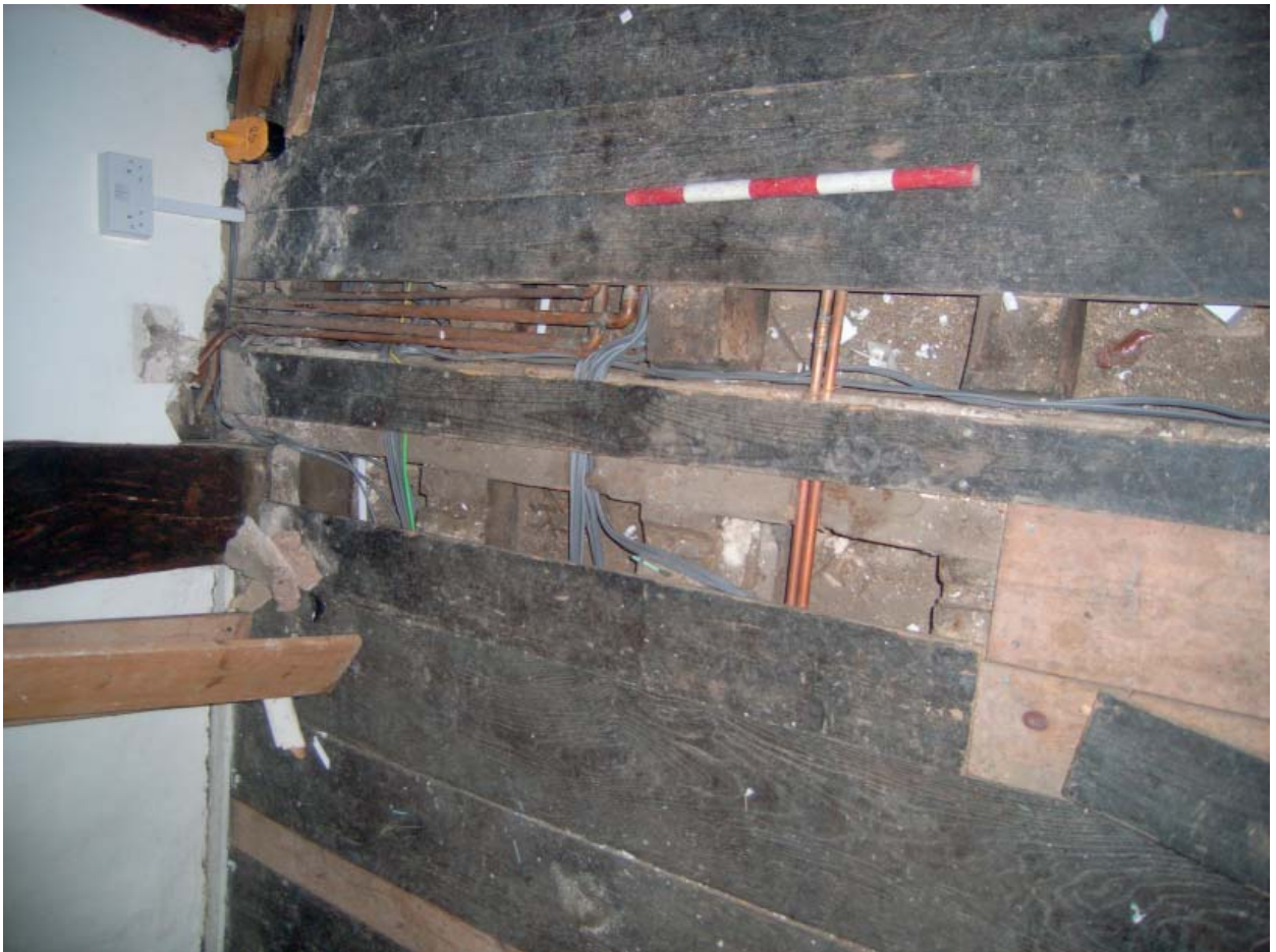
Plate 100: No. 4. Floor boards lifted. Main range 1st floor.
