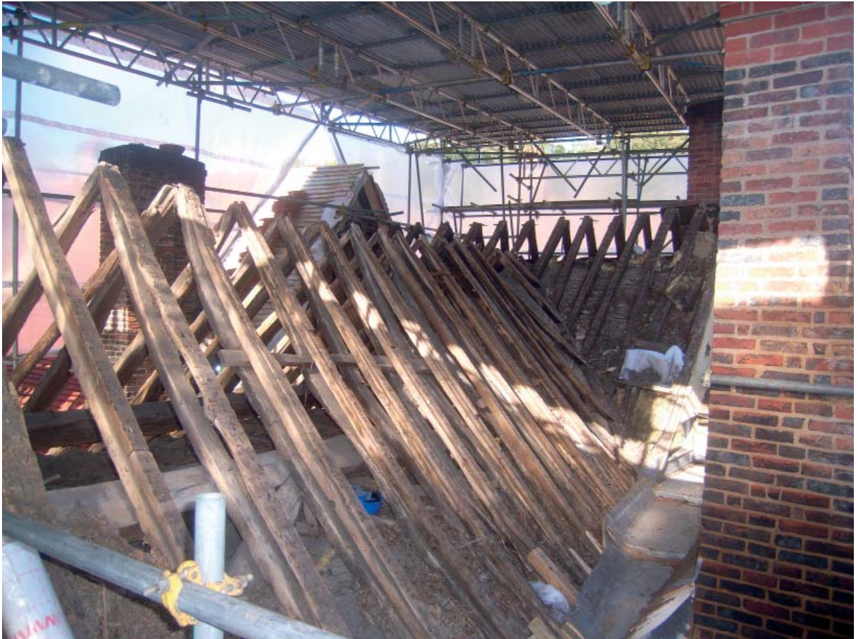
Plate 9: Roof of rear wing of No.4
