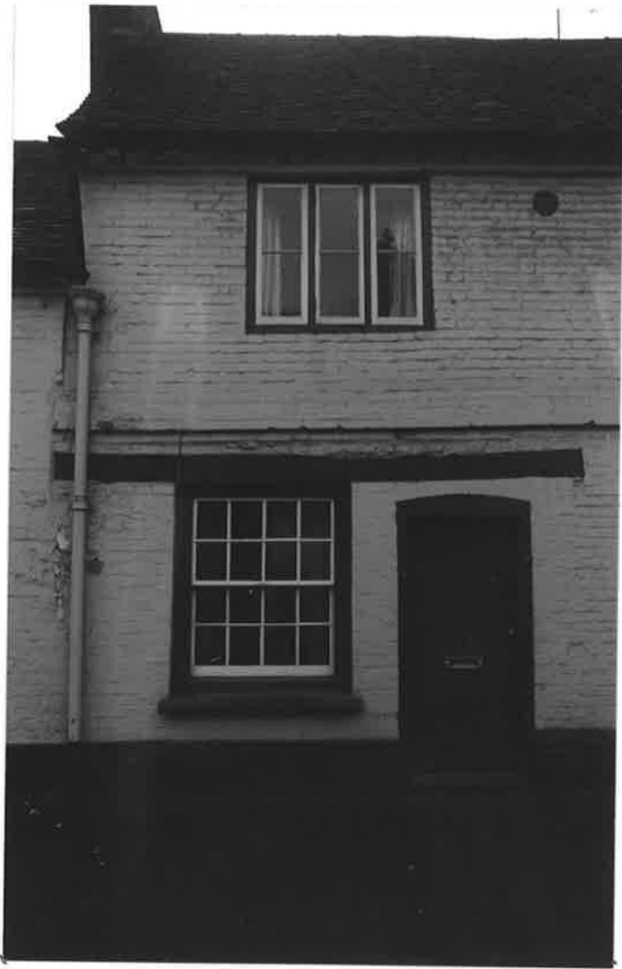
Nº 7 BLOCK L, DOOR AND GROUND FLOOR WINDOW D, FIRST FLOOR WINDOW I R. 175 N12
