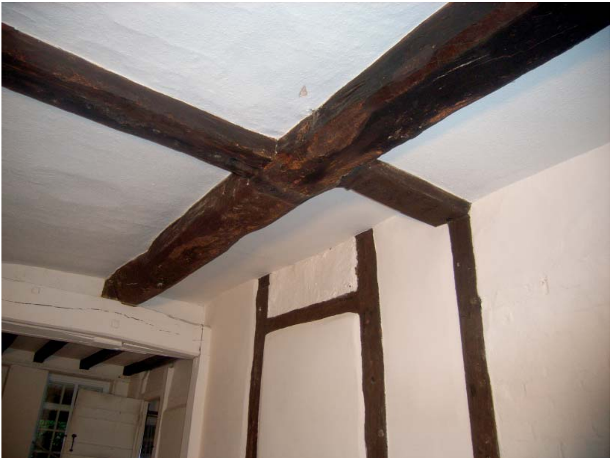
Plate 84: No 4. Ground floor front room looking south-west
