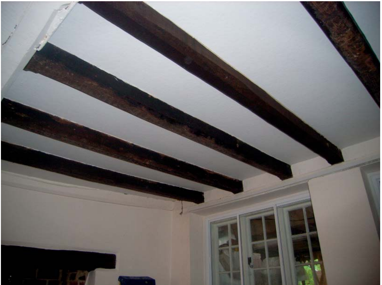
Plate 88: No 4. Joists in rear extension
