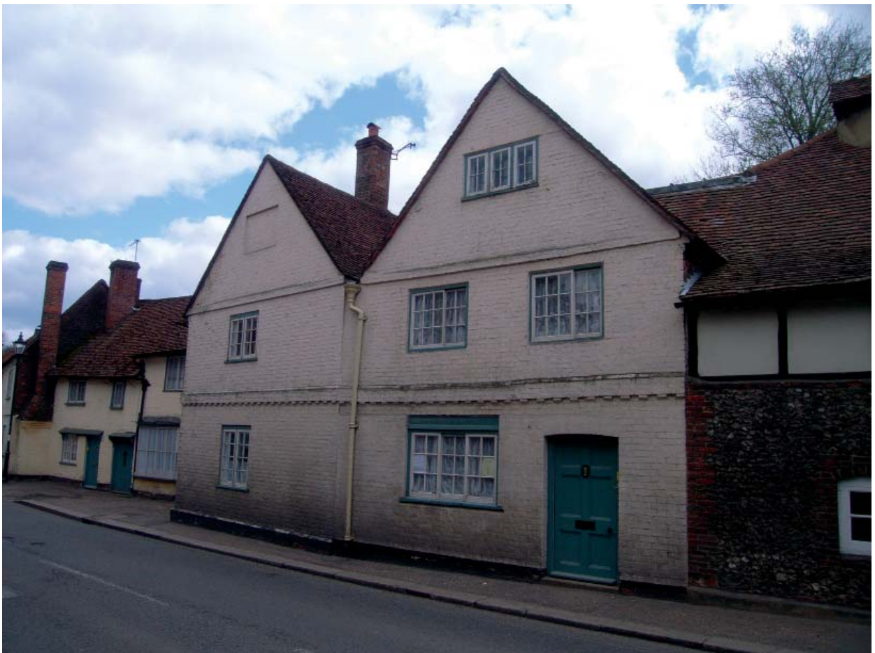
Plate 4: North elevation of No's 2-3
