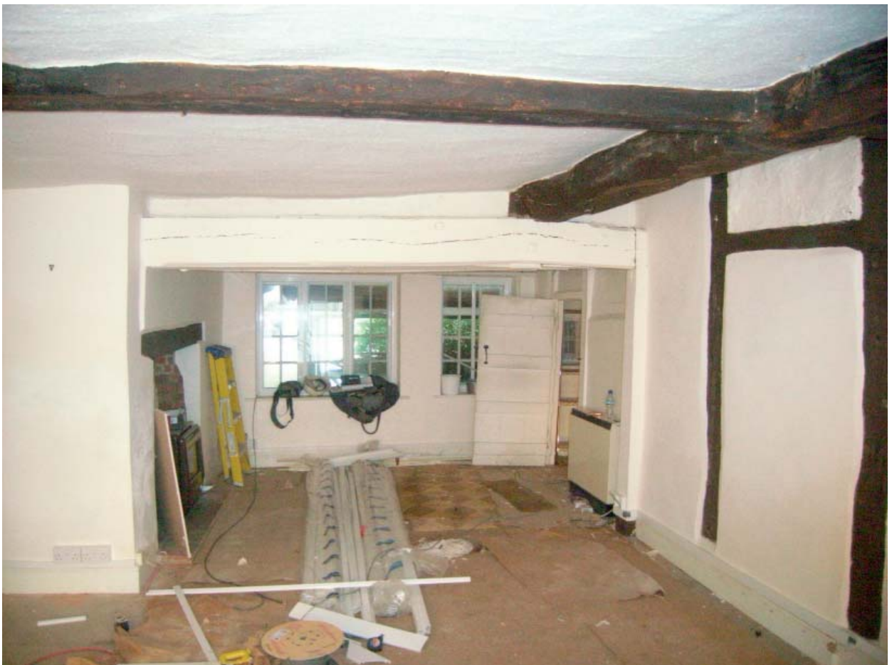
Plate 86: No 4. Ground floor front room looking south
