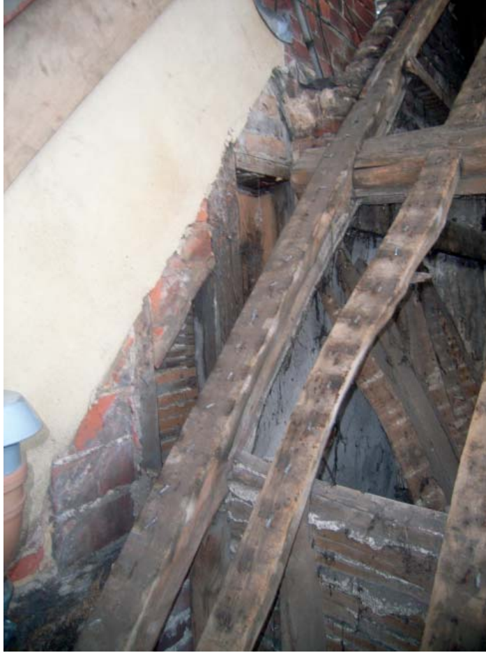
Plate 27: Blocked window at east end of No.4 (Block P)
