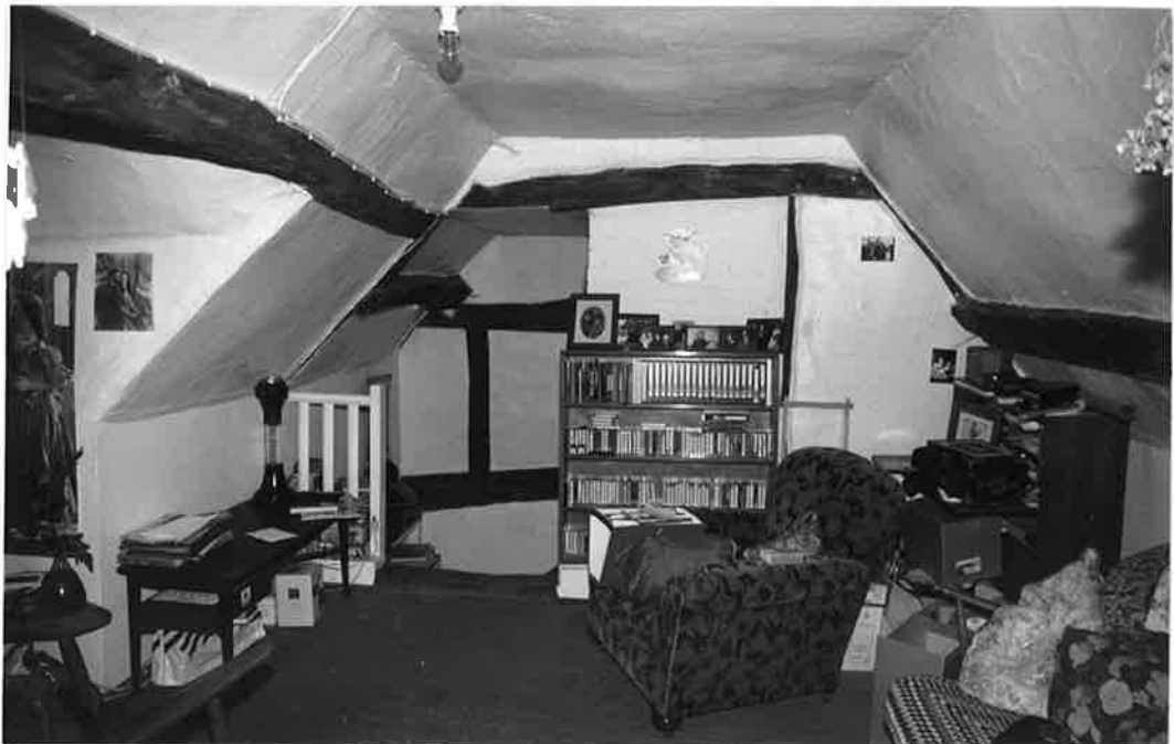
Nº2 HIGH STREET - ATTIC ROOM K, LOOKING EAST.
