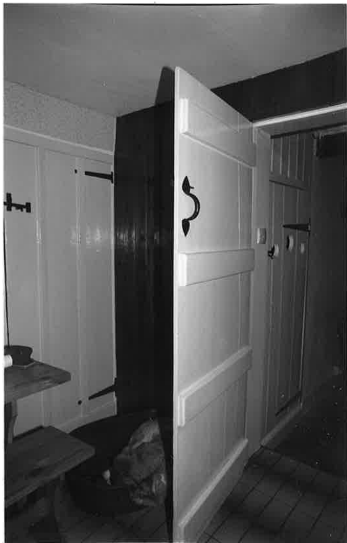
PERIOD PLANK AND BATTEN DOORS
