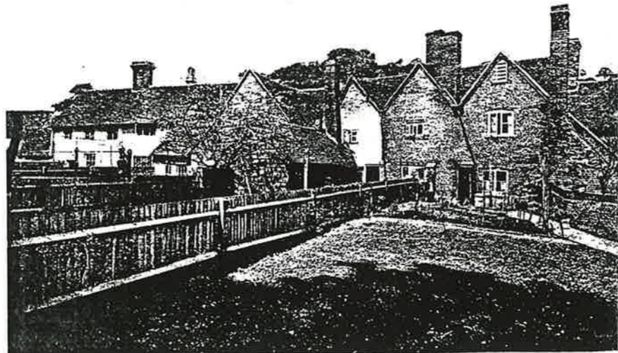
Fig. 5 (b).—The backs of cottages Nos. 1-8 after reconditioning.
