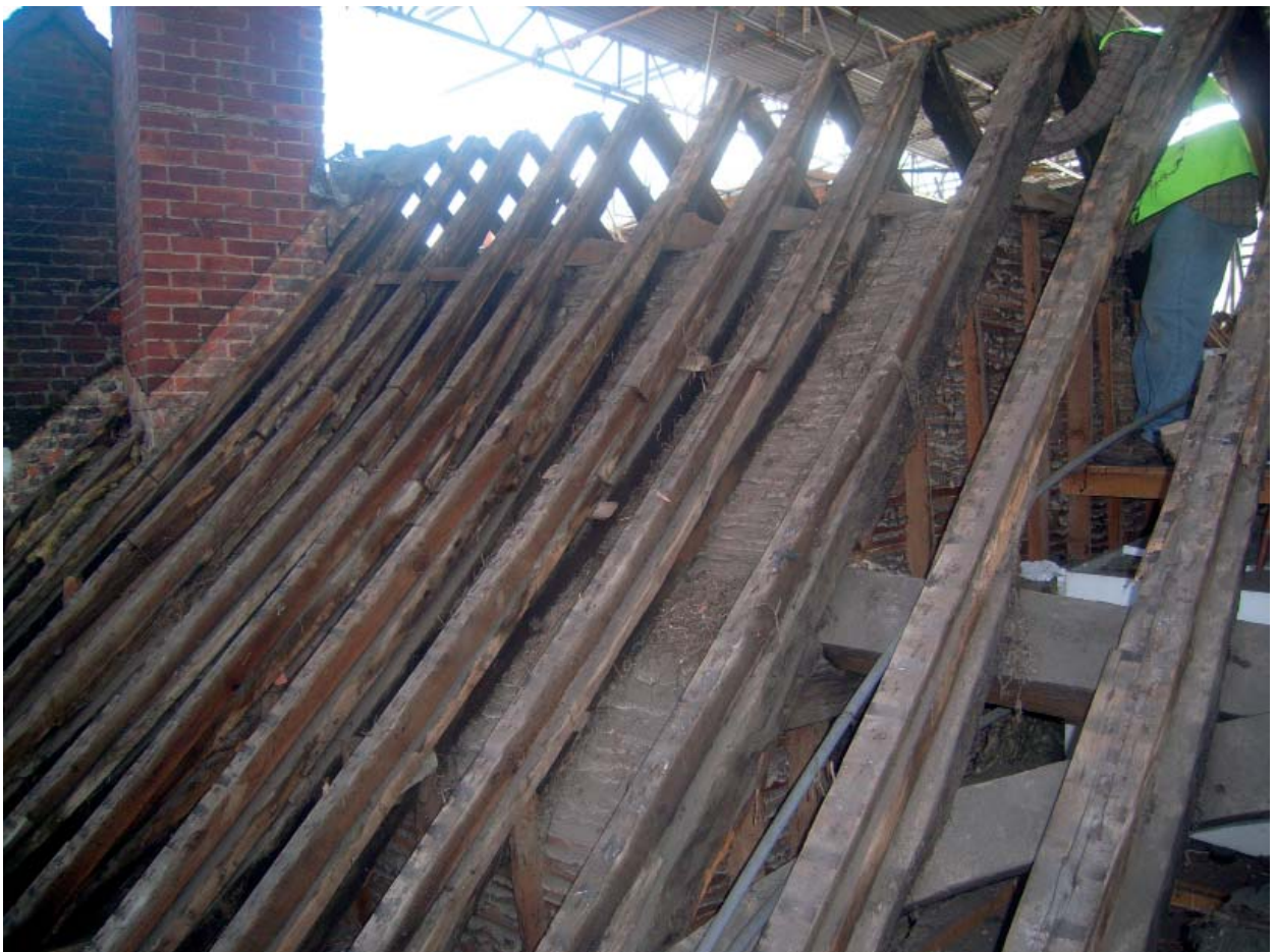
Plate 10: North slope of street front range (No.4) (Blocks P & R)
