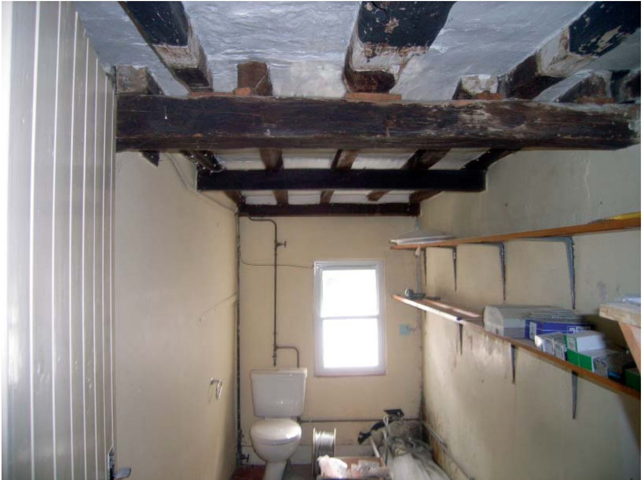
Plate 77: Interior of No 2. Former passage
