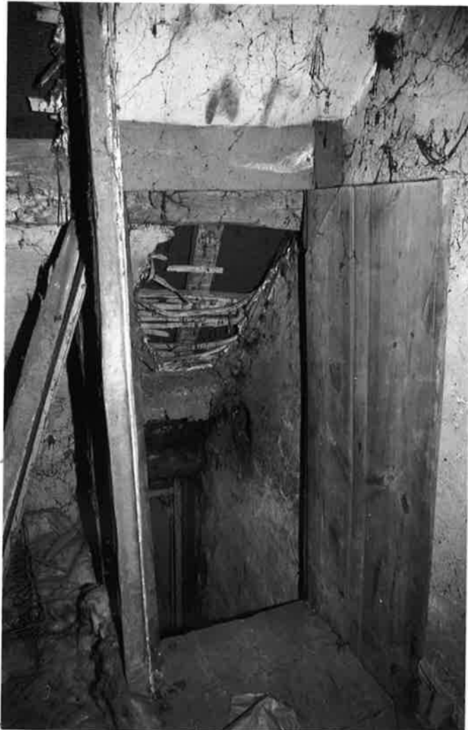
Nº7 HIGH STREET - ATTIC STAIRS VIEWED FROM ROOF SPACE. R175 N3.
