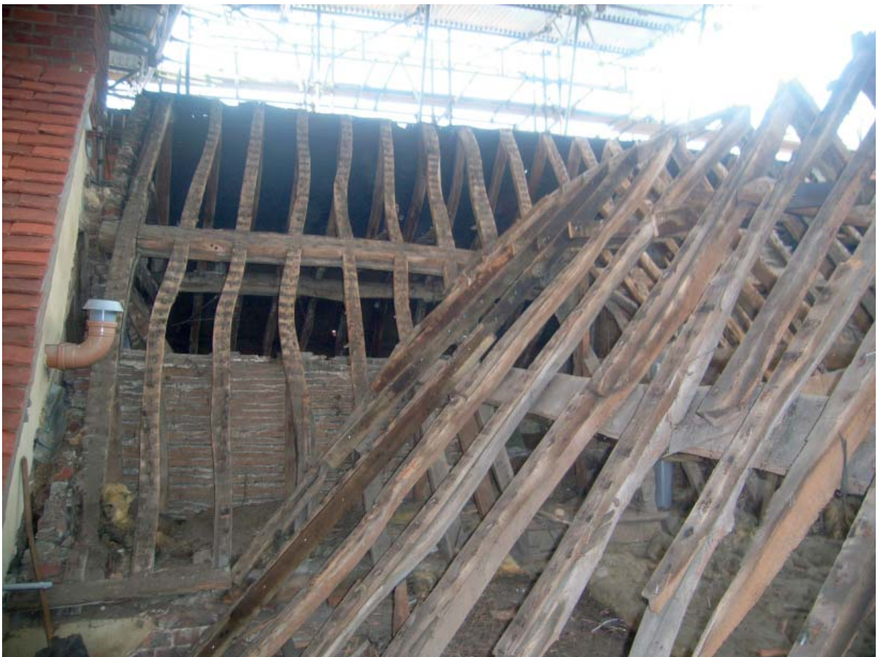
Plate 48: Rear slope of main range of No.5-7
