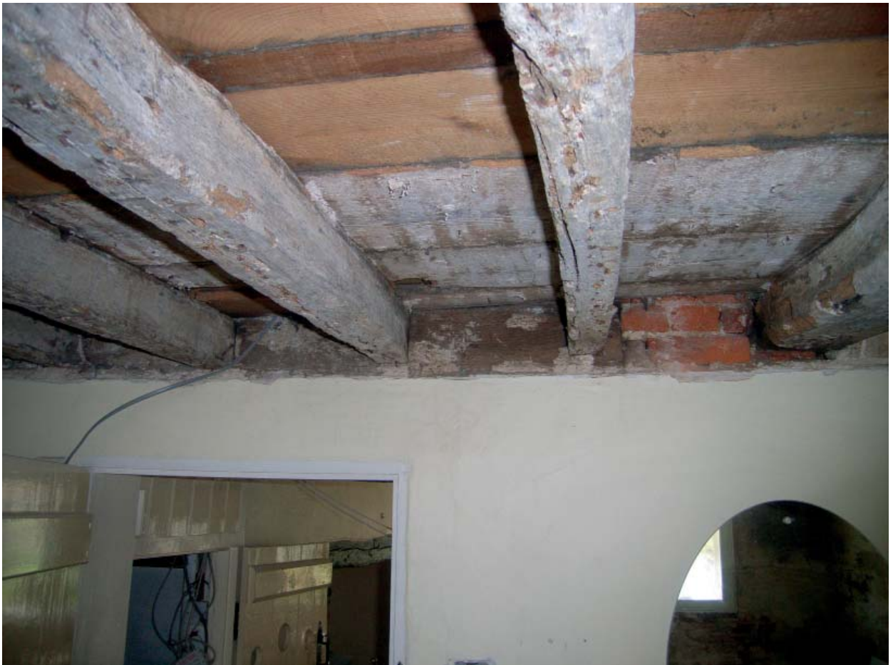
Plate 78: Interior of No 2. Ground floor joists
