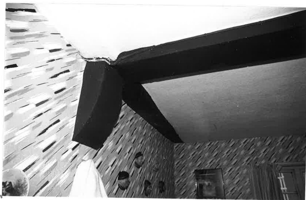
PERIOD LATERAL WOODEN BEAM SUPPORTED BY ROUNDED CORBEL. R176 N11A.
