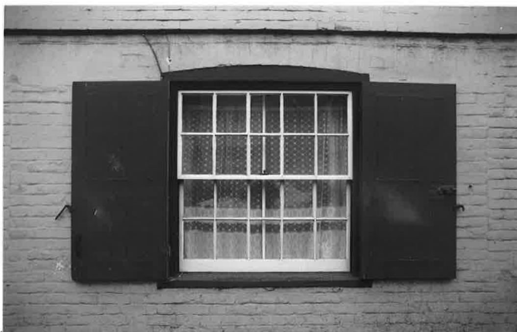
SASH WINDOW E WITH PERIOD SHUTTERS, NO 7, BLOCK L, R 175 N 13
