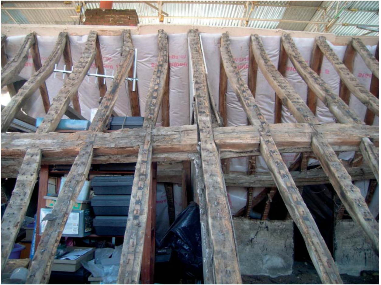
Plate 35: View of roof of No.5-7
