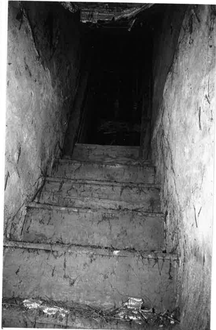
Nº7 HIGH STREET - ATTIC STAIRS, VIEWED FROM ROOM G. R175 N4.
