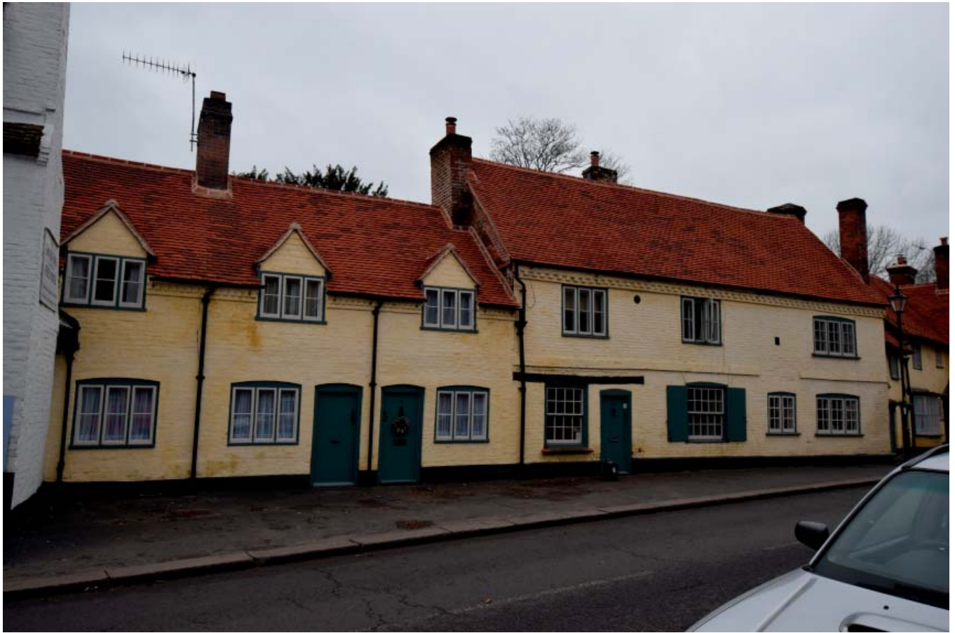
Plate 1: North elevation of No's 5-8
