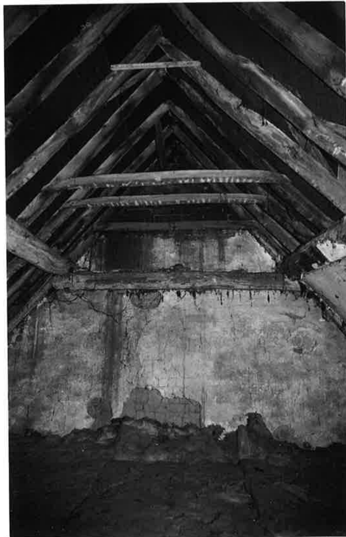
Nº7 HIGH STREET - ROOF STRUCTURE MAIN BLOCK, LOOKING EAST. R175 N1.
