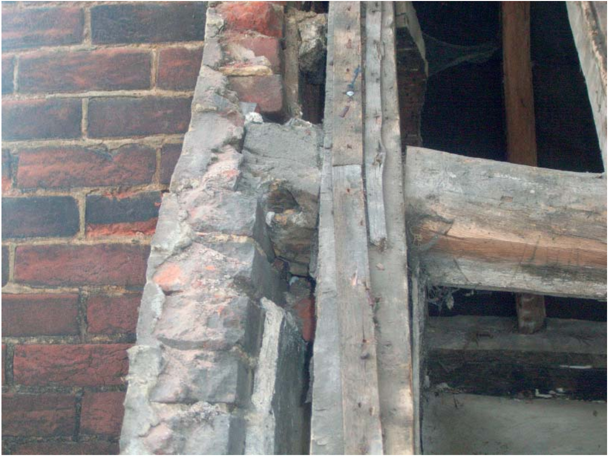
Plate 43: Purlin detail in No. 5-7
