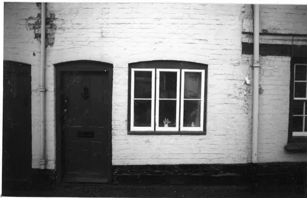
FRONT DOOR D3, AND WINDOW D R.173 N30A
