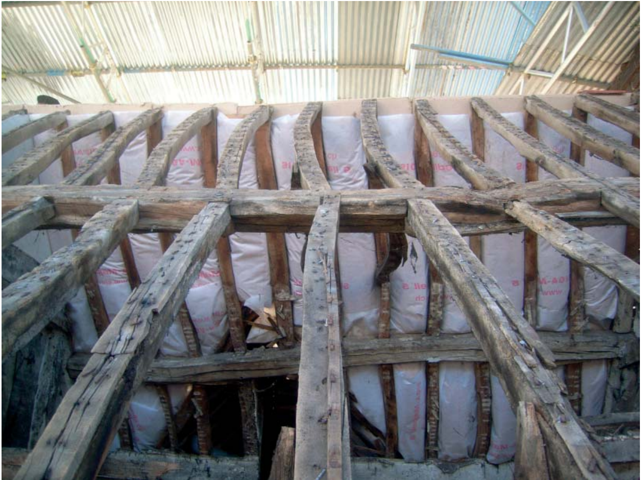
Plate 55: Rafters in rear slope of No.5-7
