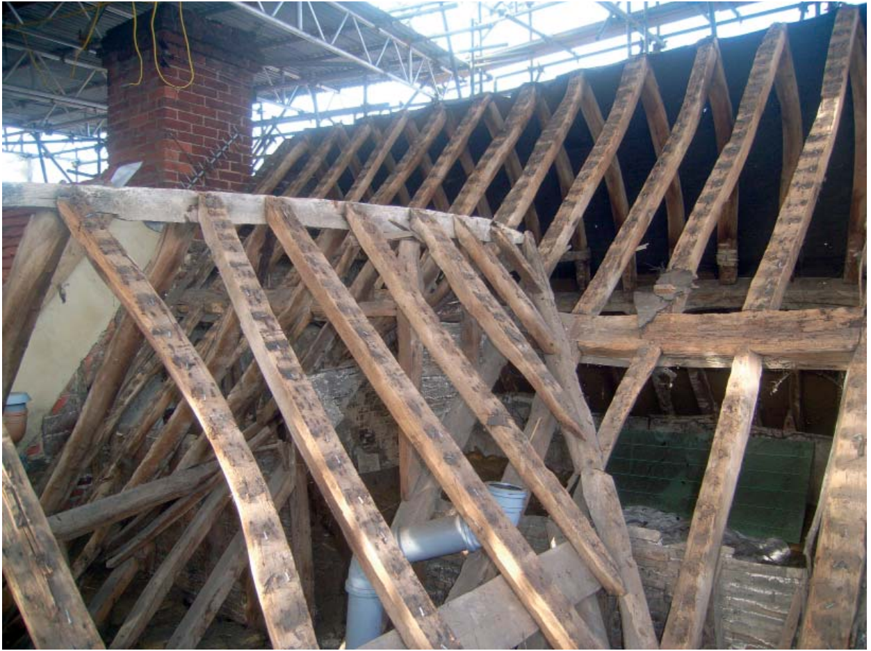
Plate 45: Rear projection and rear of main roof (Block K)
