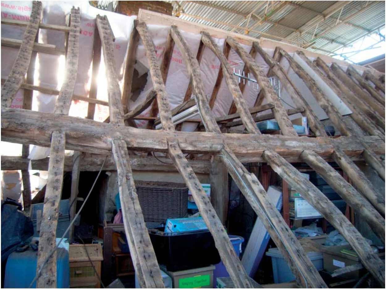
Plate 31: Roof of No.5-7
