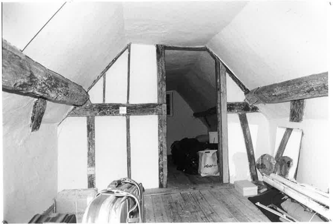
No. 27/28 ATTIC ROOM H , LOOKING SOUTH R251 N6.
