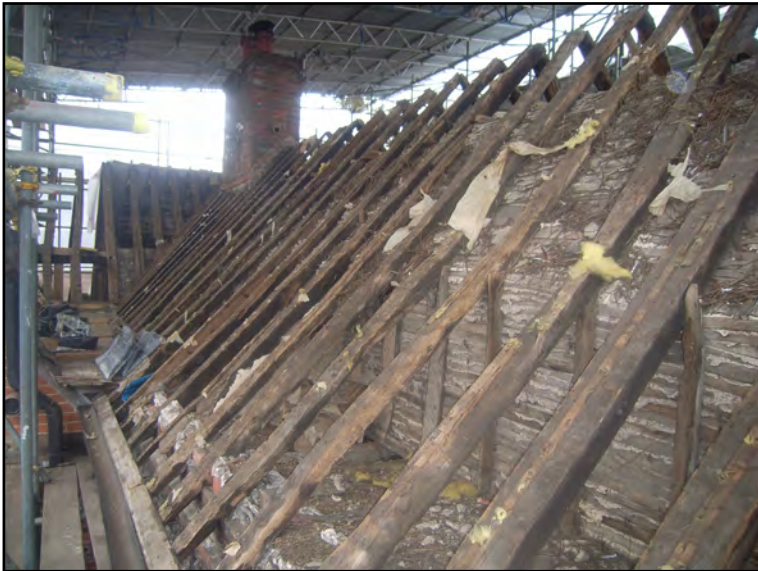
Plate 59: General view of west slope of Building C
