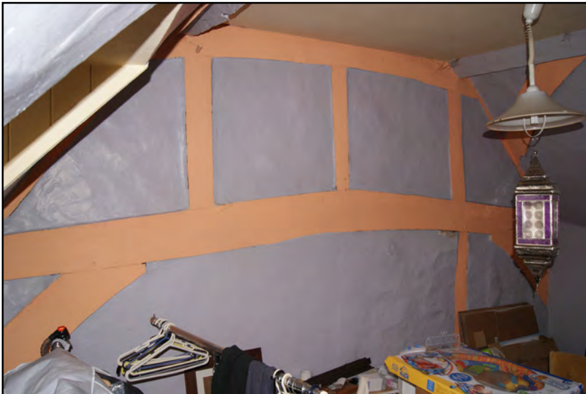
Plate 78: Wind braces in eastern bay of Block B (south slope)
