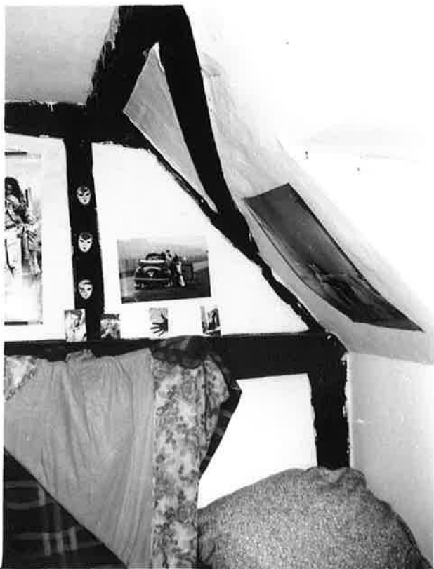
No. 34/35. ATTIC ROOM K, LOOKING EAST R235 N10A.
