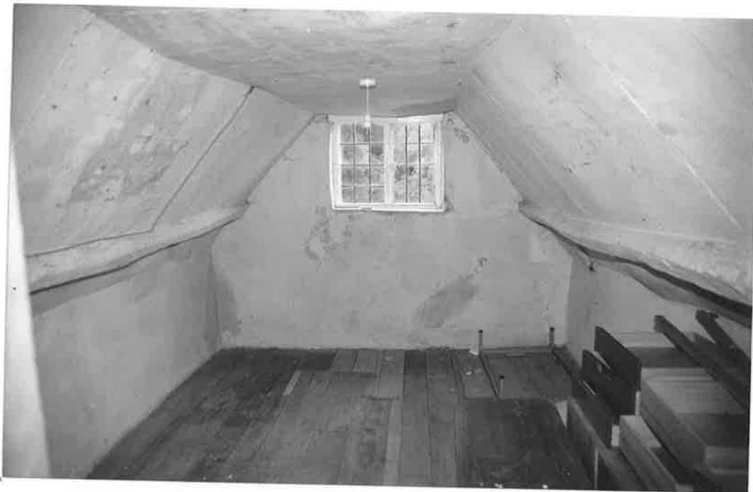
INTERNAL ROOF STRUCTURE, LOOKING NORTH, NO. 27. R70 N12.
