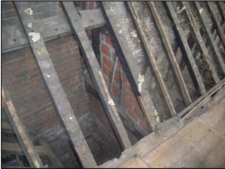
Plate 65: North western corner of Building C
