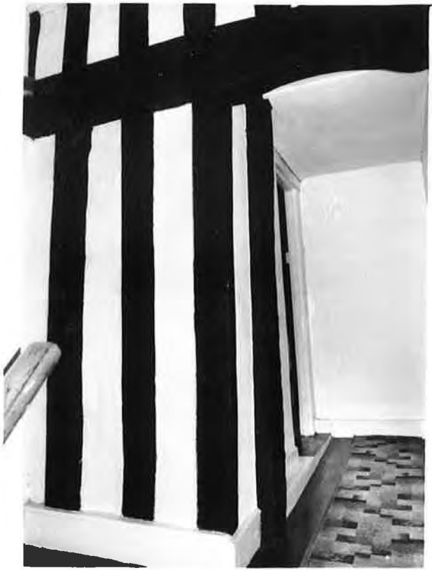
NO. 25. LANDING, ROOM H, LOOKING EAST R229 N 27A.
