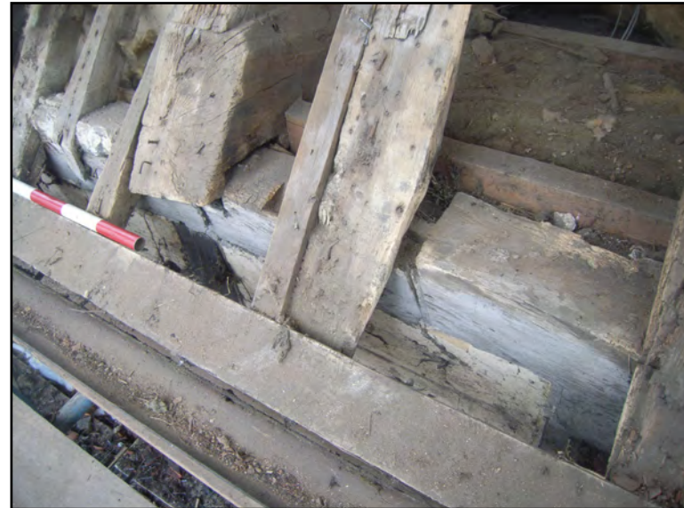
Plate 12: Wall plate scarf detail in N slope of Block A
