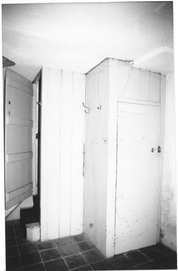
BLOCKED-OFF GROUND FLOOR ROOM WITHIN CROSS WING LOOKING NORTH. R70 N34.
