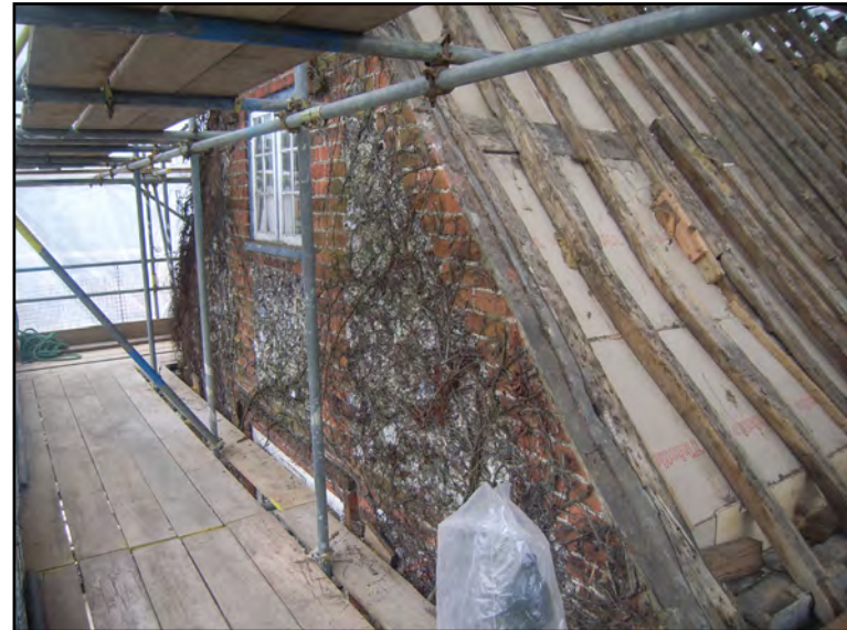
Plate 8: Re-faced east elevation of Block A
