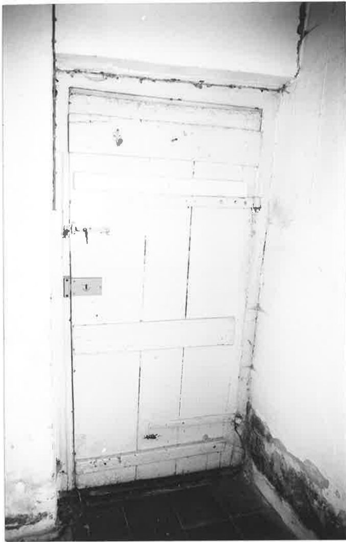
DOOR LEADING FROM CROSS WING TO ROOM C, NO. 27. R70 N36.
