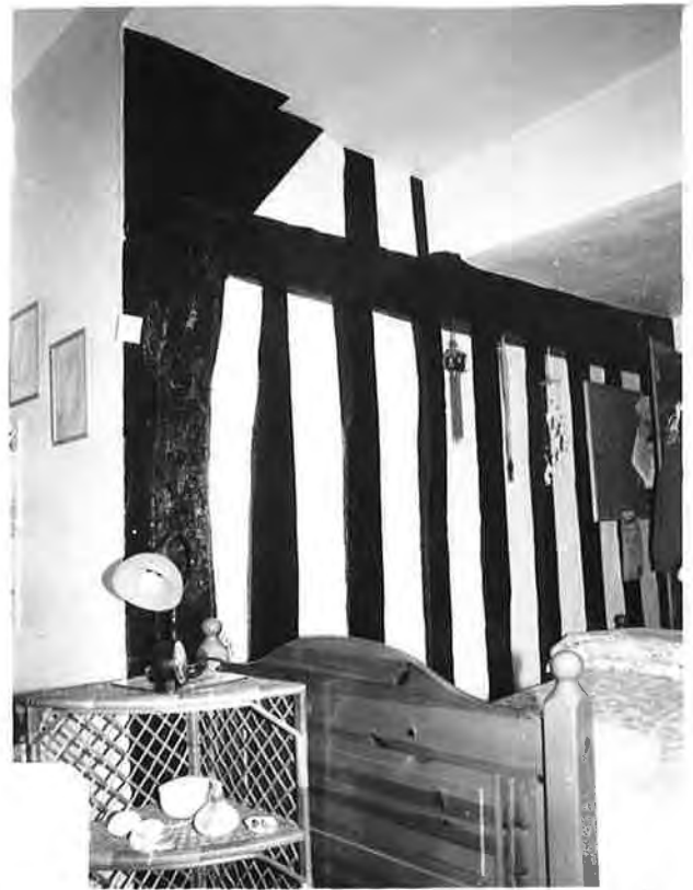
NO. 24. BEDROOM I, LOOKING SOUTH-EAST R227 N20.
