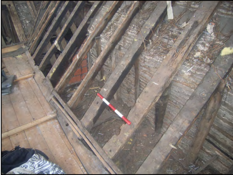
Plate 61: Towards north end of west slope of Building C
