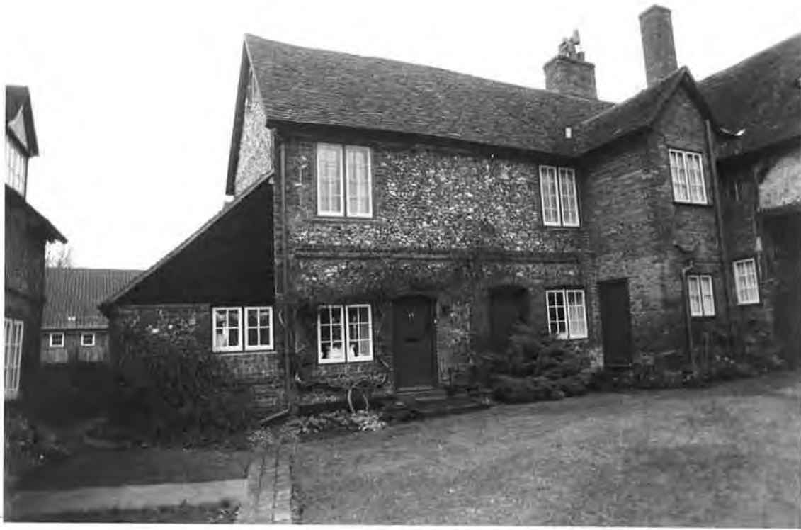
VIEW FROM SOUTH-EAST R251 N4.
