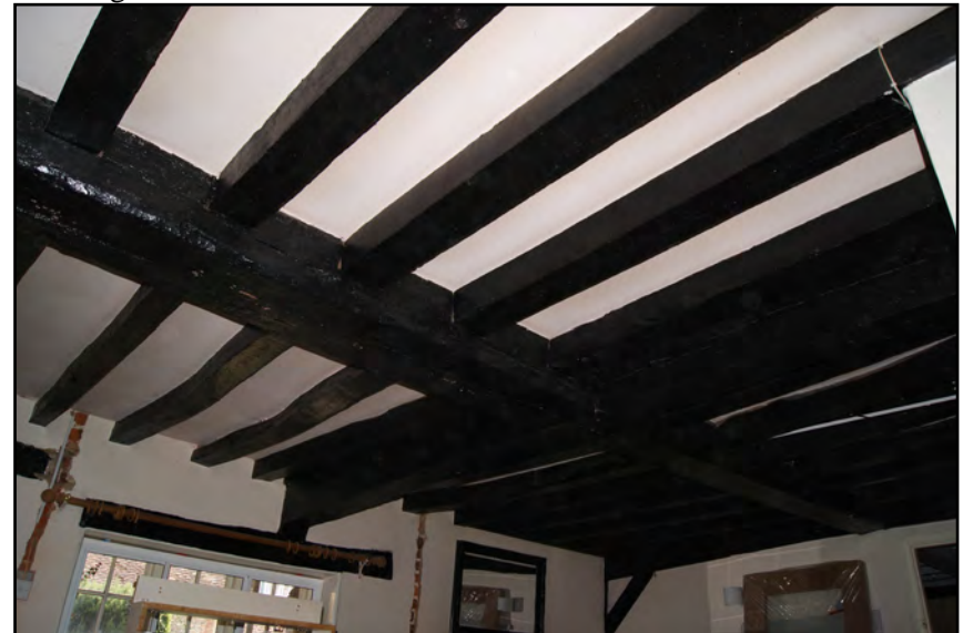
Plate 72: Underside of first floor joists towards east end of Block A
