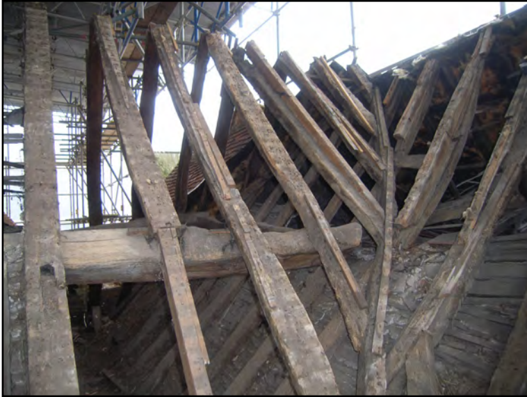
Plate 33: Roof of Block B overlying earlier roof of Block D
