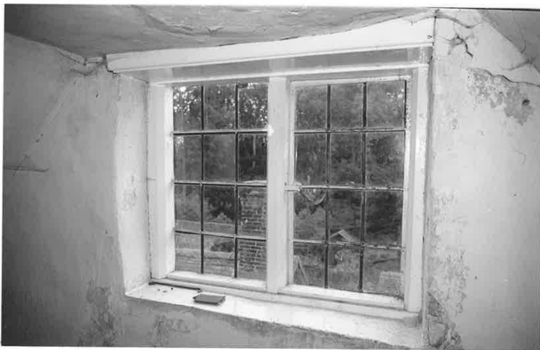
ATTIC WINDOW, NO. 27 R70 N13.
