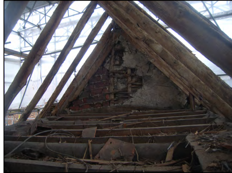
Plate 22: Wattle and daub in formerly external E end of Block B
