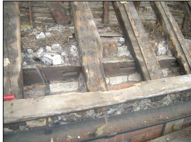
Plate 56: Detail of west wall plate of Building C
