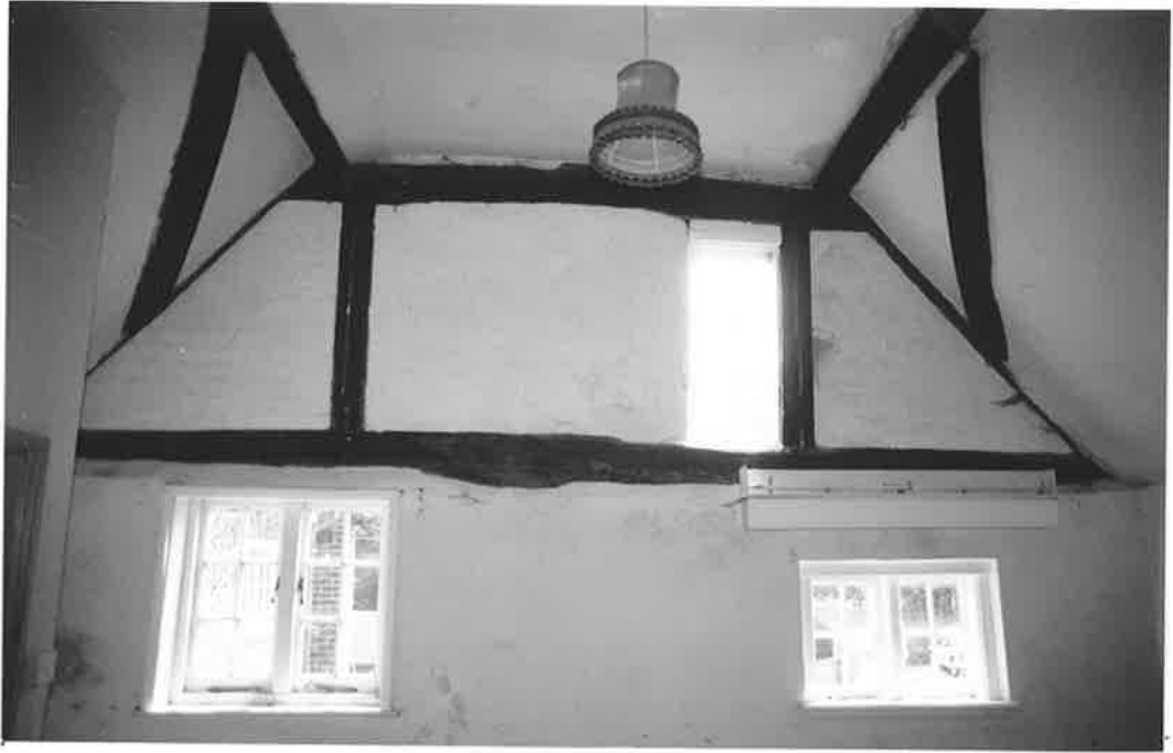
BLOCKED-OFF FIRST FLOOR ROOM WITHIN CROSS WING LOOKING SOUTH R 70 N 28.
