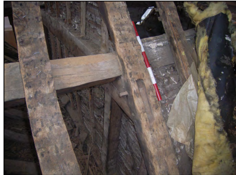
Plate 36: Clasped purlin detail. South end of westernmost truss of Block B
