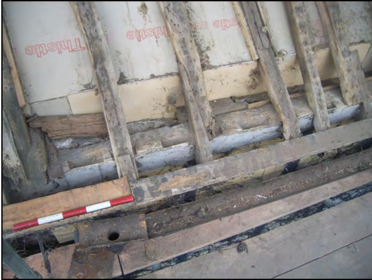
Plate 9: Empty rafter mortices in wall plate.
