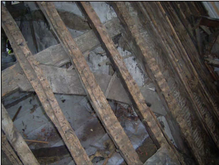
Plate 43: Wind brace to south slope of Block B. Truss B2.
