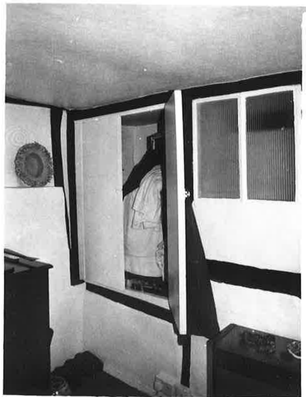
NO. 24. BEDROOM F, LOOKING NORTH-WEST R227 N26.
