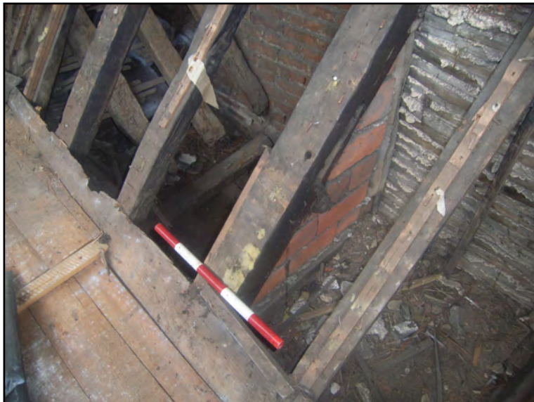
Plate 67: North-western corner of Building C
