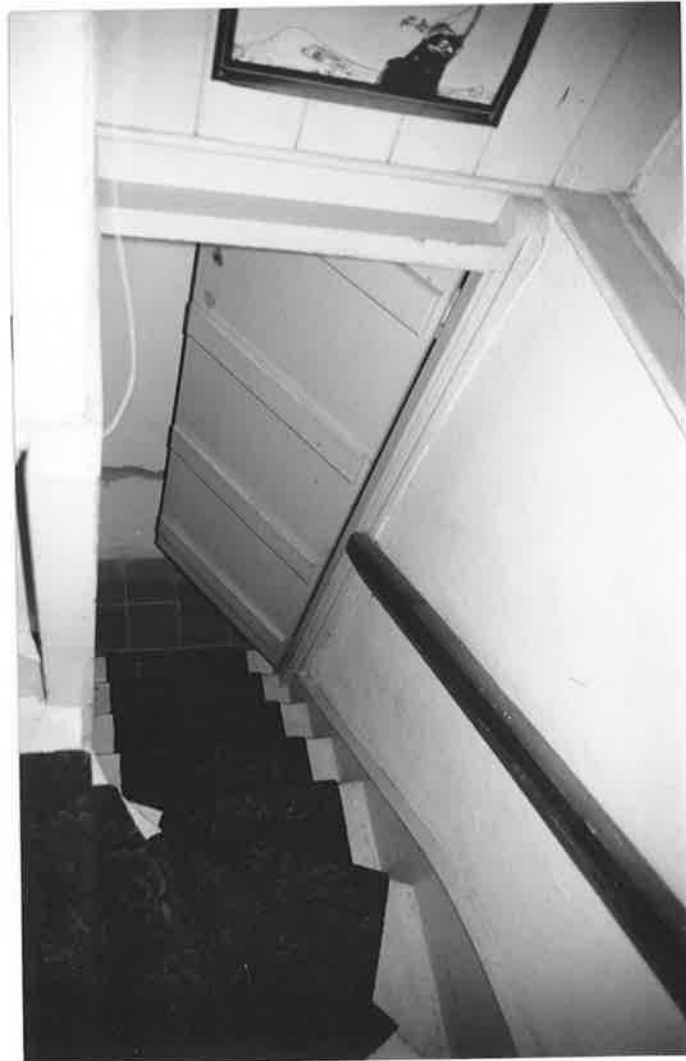
BOTTOM SECTION OF STAIRS WITHIN CROSS WING R70 N31.
