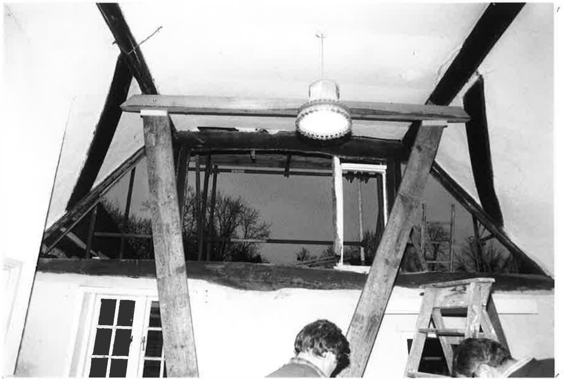
NO. 25, ROOM K, LOOKING SOUTH R251 N8
