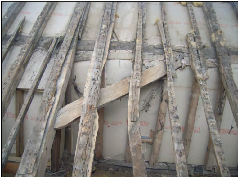
Plate 11: Straight wind brace in north slope of Block A
