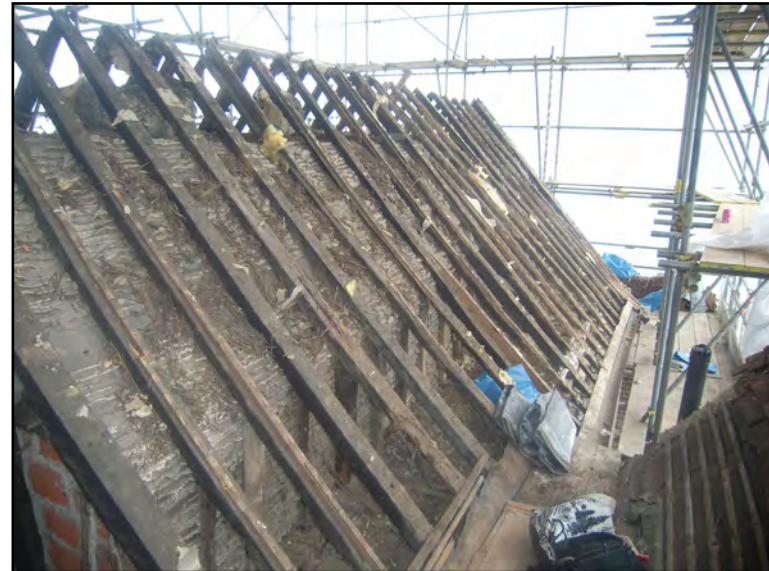
Plate 60: General view of west slope of Building C
