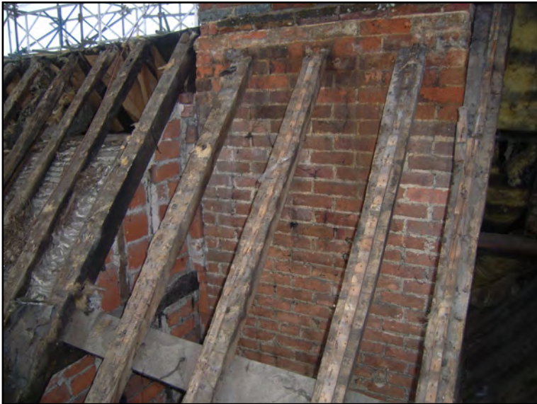
Plate 51: East side of chimney stack at N end of Block C
