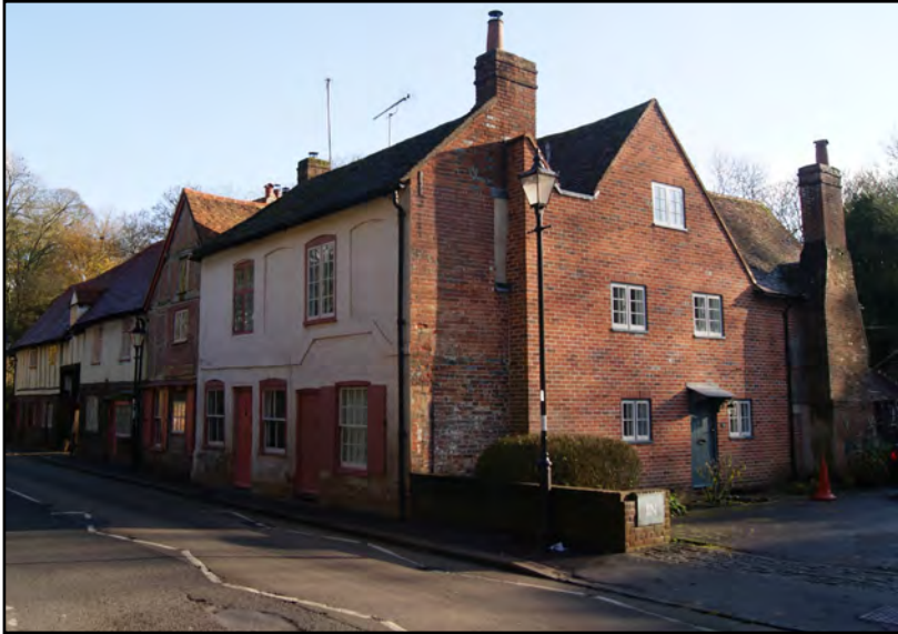
Plate 1: General view of complex from NW
