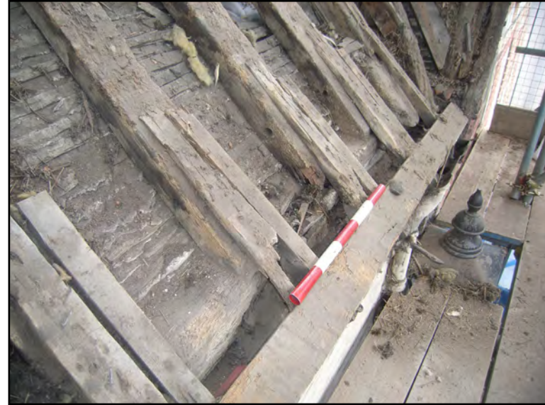
Plate 34: Rafter feet at west end of north slope of Block B.
