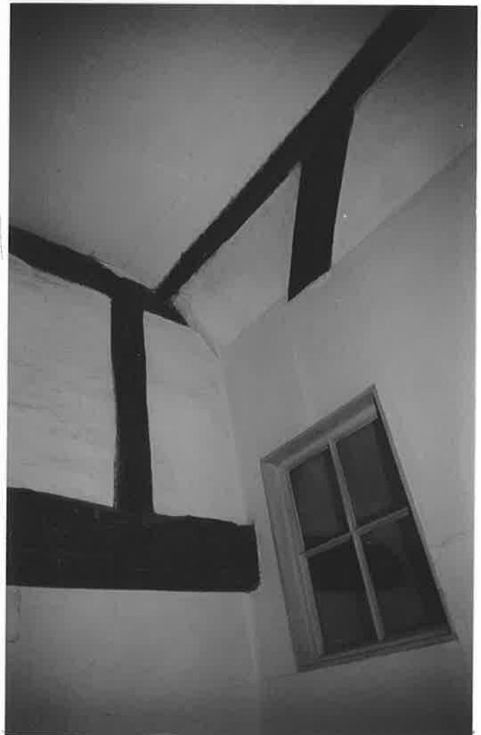
DETAIL OF ROOF STRUCTURE TO CROSS WING, LOOKING NORTH-EAST R70 N33.
