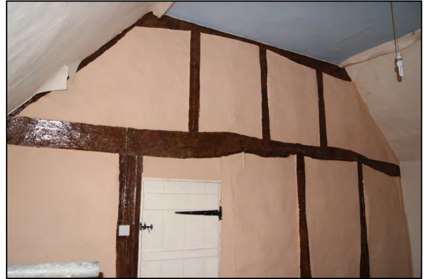
Plate 76: Internal cross frame in Block A
