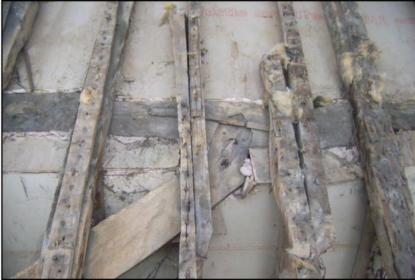
Plate 13: Wind brace detail in N slope of Block A
