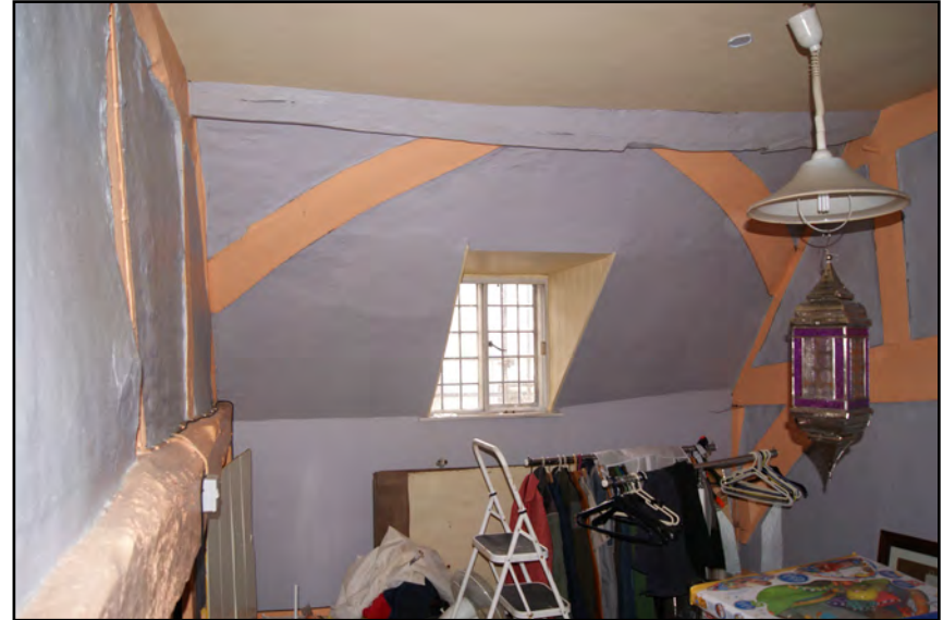
Plate 79: Internal truss on west side of Bay B1 (above carriage entrance)
