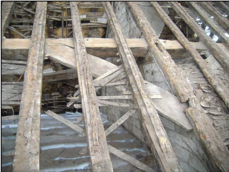
Plate 27: Wind brace in N slope of Block B. Truss B3
