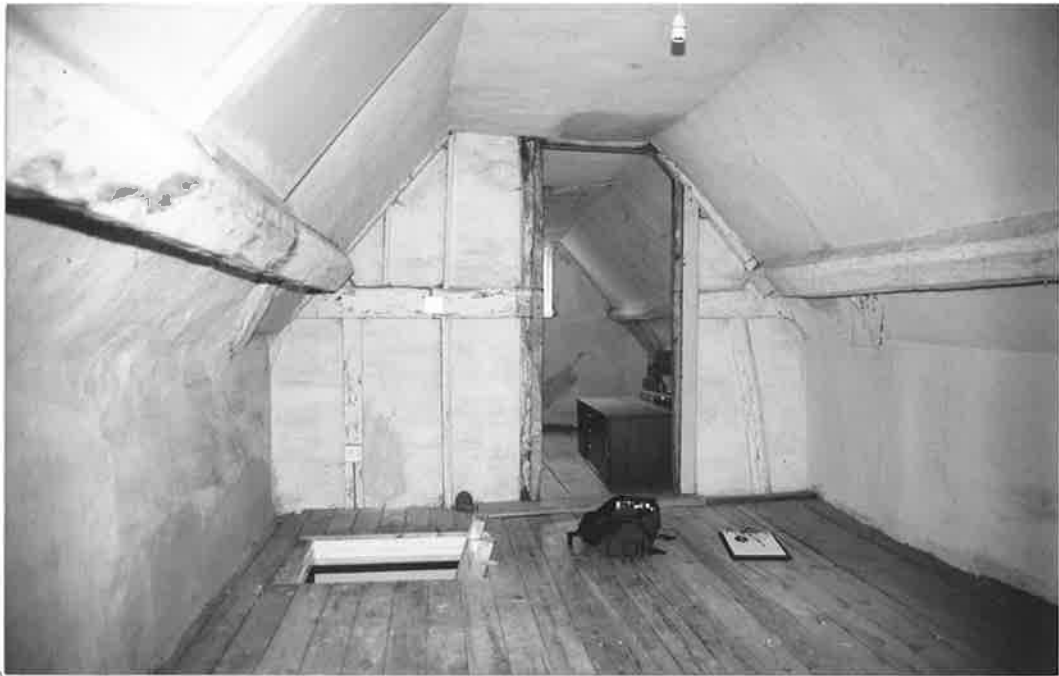
NO.27 INTERNAL ROOF STRUCTURE, LOOKING SOUTH R 70 N 10.
