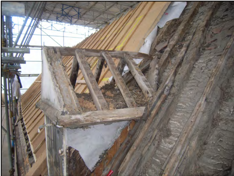
Plate 19: Dormer above carriage entrance. Block B north slope
