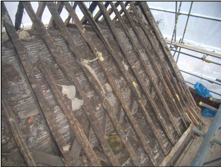
Plate 55: West slope of Building C
