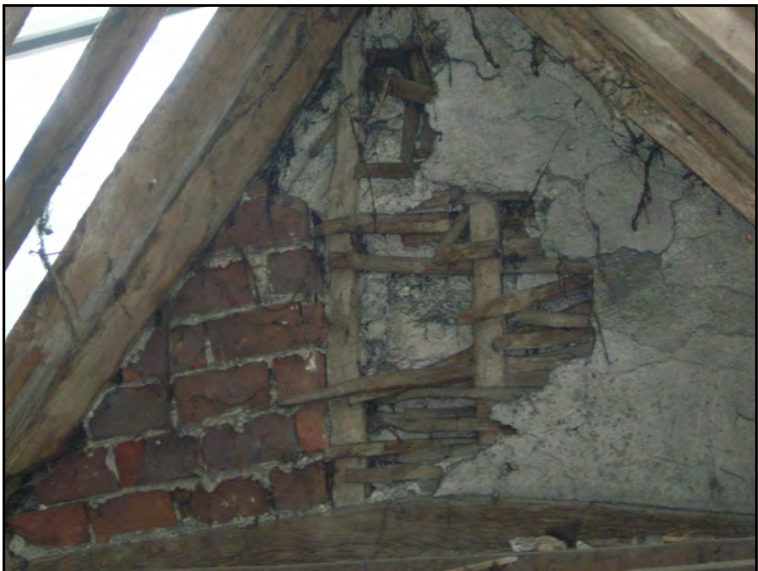
Plate 23: Wattle and daub in formerly external E end of Block B
