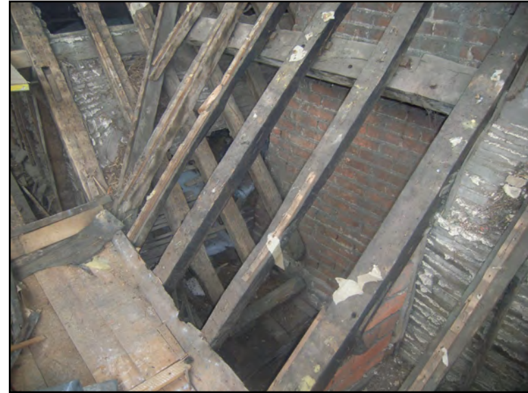
Plate 64: North-western corner of Building C
