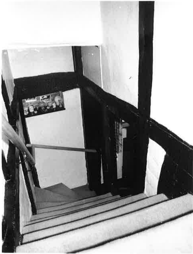
NO. 24. STAIRS, VIEWED FROM LANDING, ROOM C. R227 N19.
