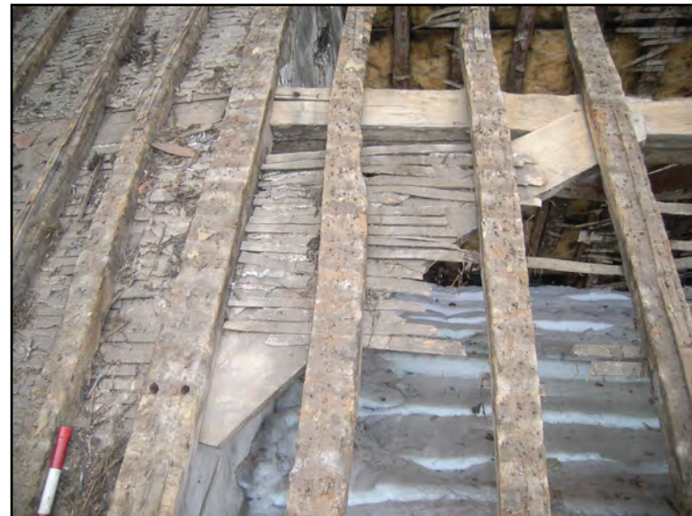
Plate 24: Wind brace in north slope of Block B (Bay B2)
