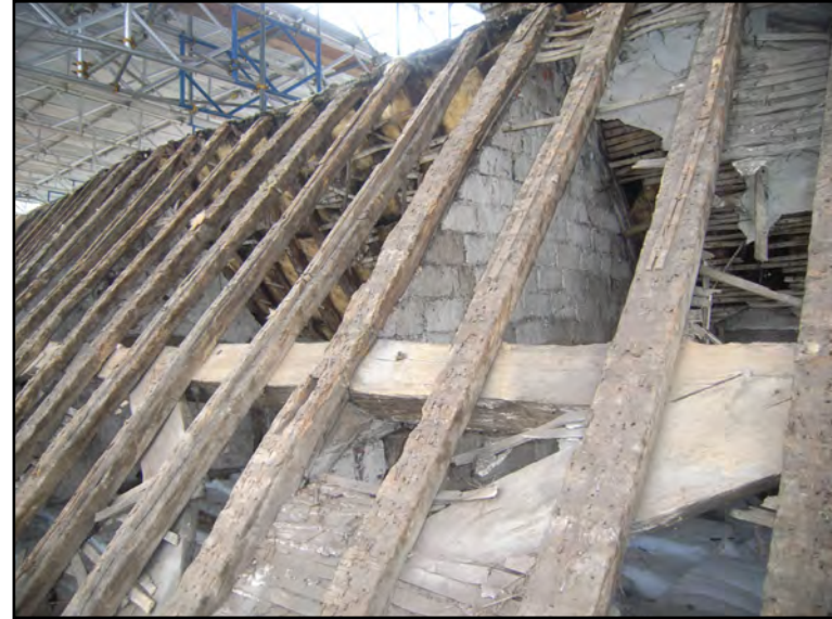
Plate 30: North slope of Block B. Infilled Truss B3
