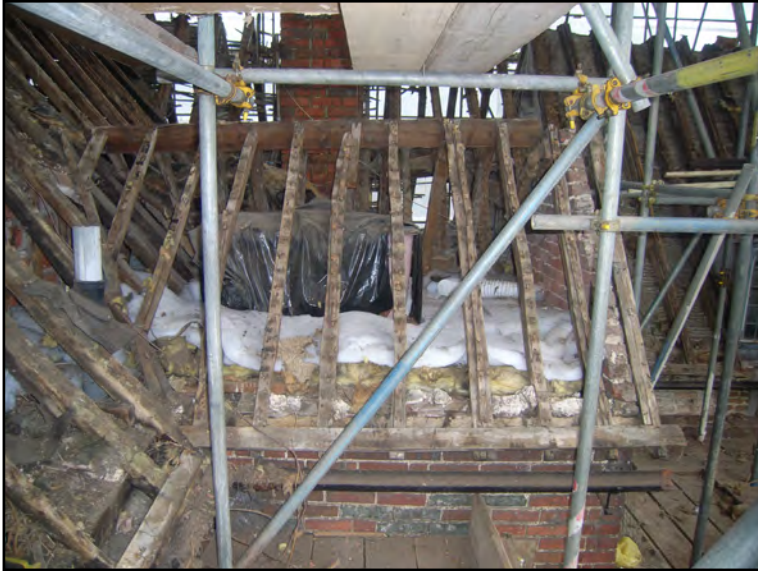
Plate 49: Secondary projection on east side of Block C
