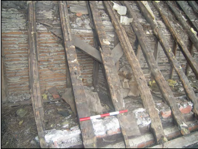
Plate 57: Central section of west slope of Building C
