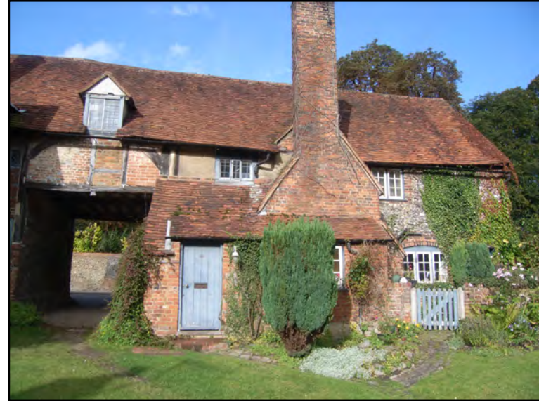
Plate 6: Rear elevation of Block A and part of Block B
