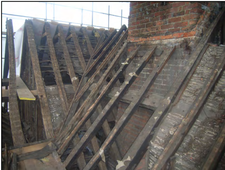
Plate 63: Northern end of Building C at junction with Building B
