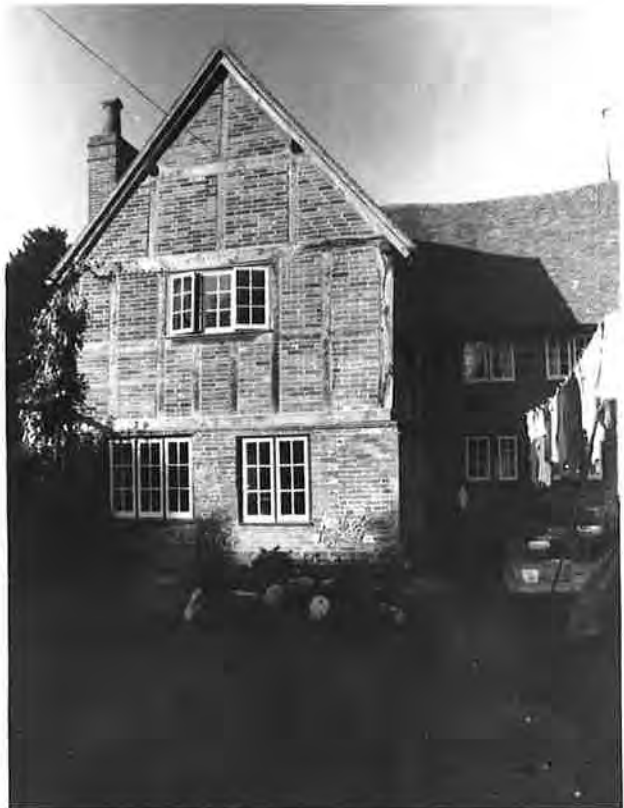
VIEW FROM SOUTH R227 N33.
