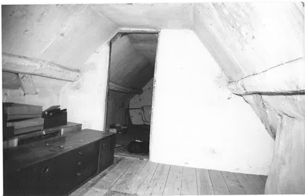
AS ABOVE, LOOKING NORTH, SHOWING PURLINS AND WINDBRACES.
