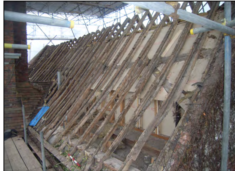
Plate 16: General view of south slope of Block A
