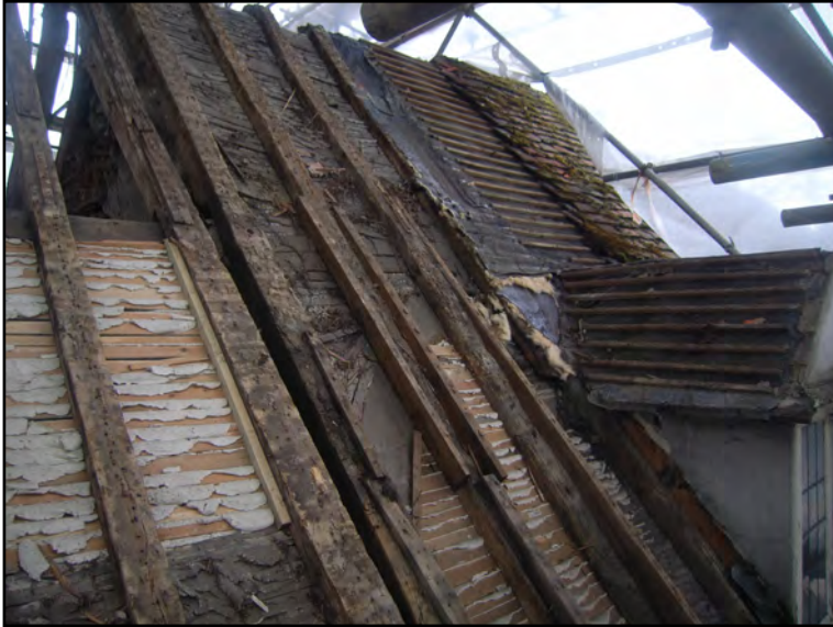
Plate 21: Dormer above carriage entrance. Block B north slope
