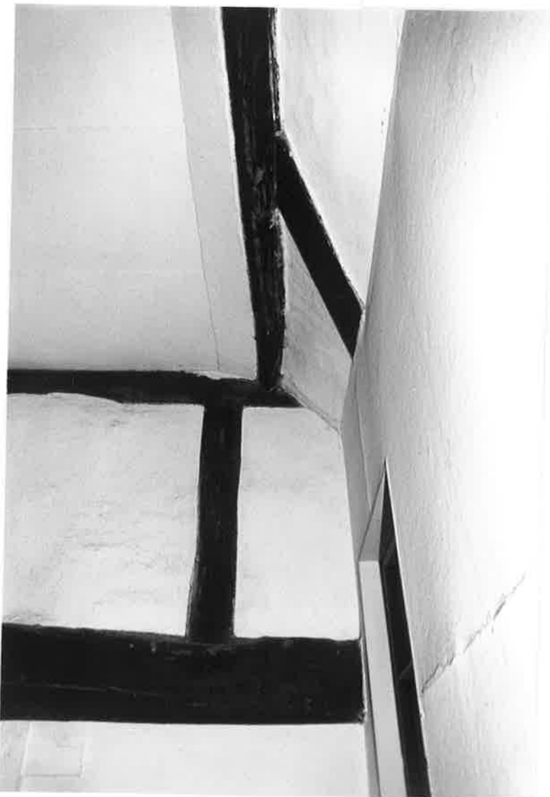
NO. 25 DETAIL OF TRUSS ROOM K, LOOKING SOUTH R251 N10.
