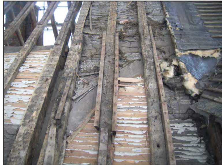
Plate 20: Wind brace at east end of north slope of Block B
