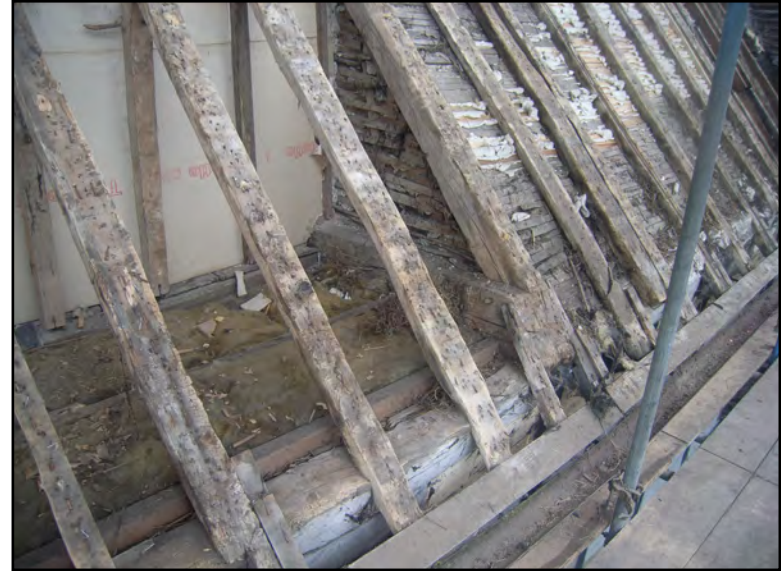
Plate 14: Block A Bays A2 and A3 north slope.
