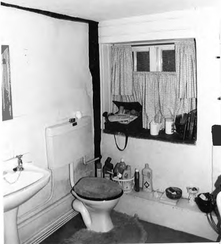
NO. 34/35 BATHROOM H, LOOKING SOUTH-EAST R253 N34.
