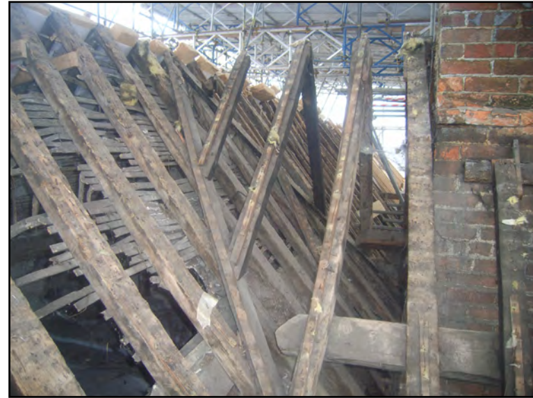
Plate 66: Northern end of Building C, overlying earlier rafters of Building B
