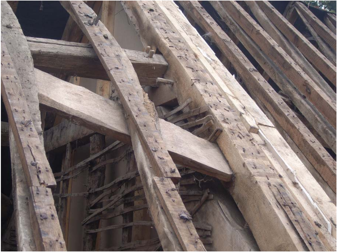
Plate 17: Wind brace in north bay, west slope
