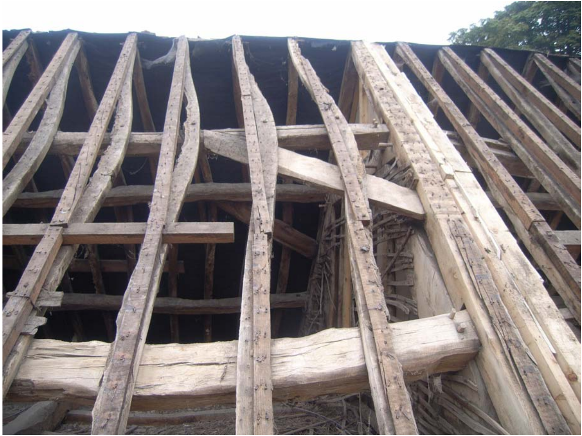
Plate 15: West slope of north bay
