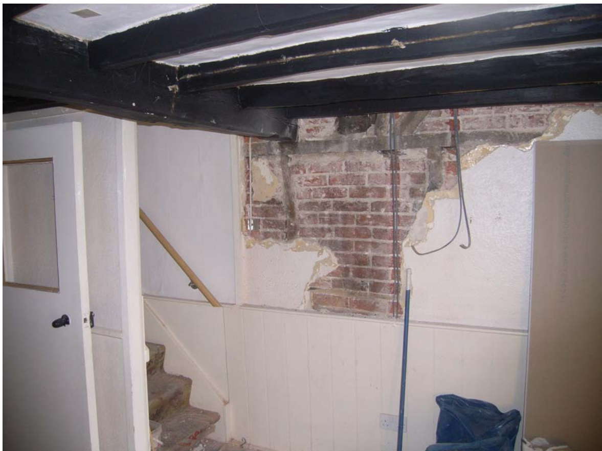
Plate 38: North face of wall dividing No 32 from No 33 (Room 33A)
