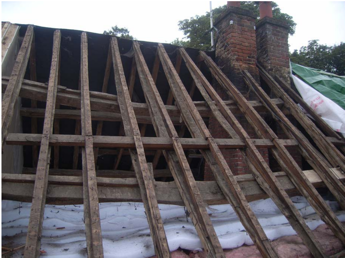
Plate 8: West slope of central bay
