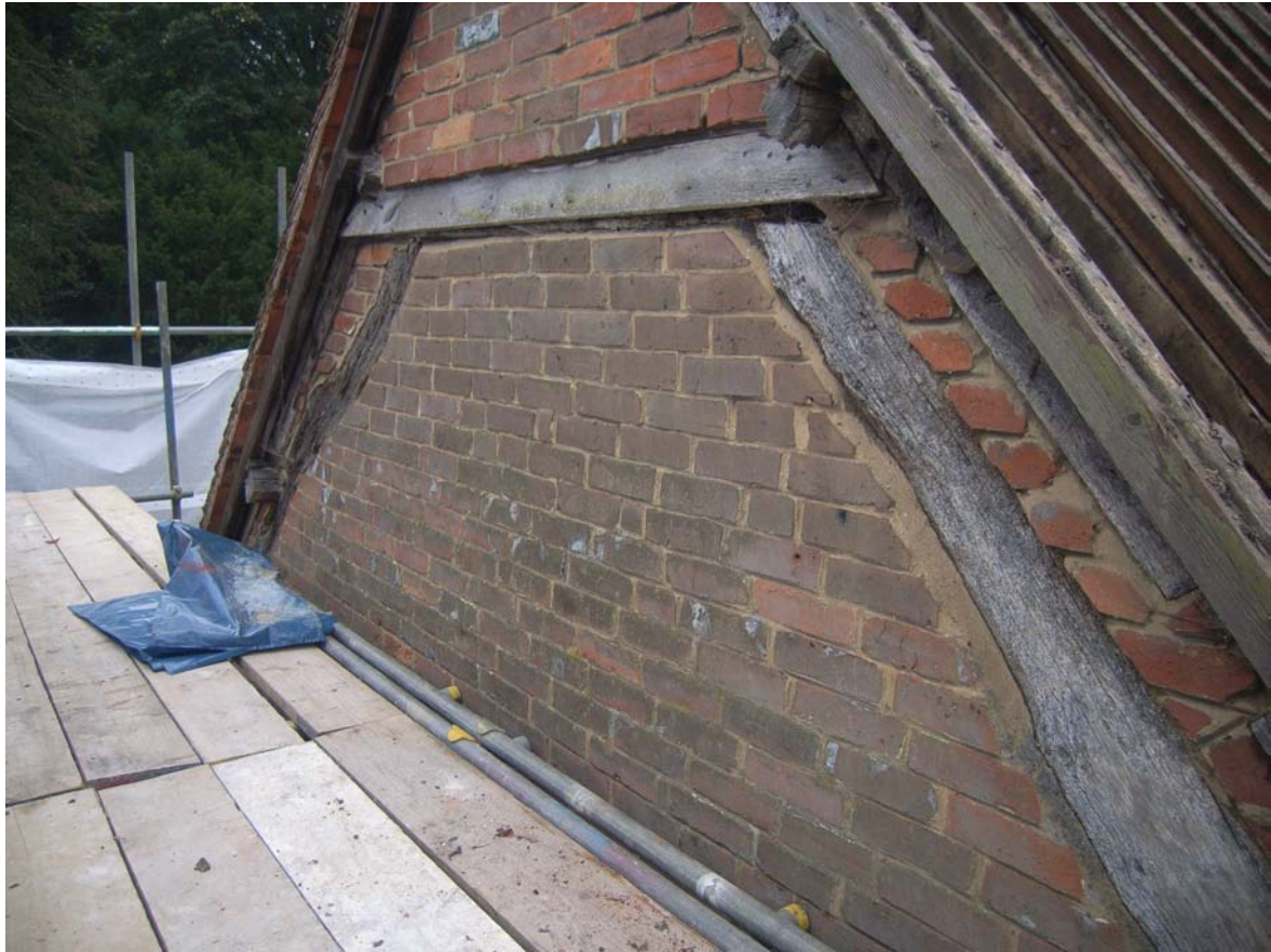
Plate 25: Curved inner principals (or crucks) in northern gable
