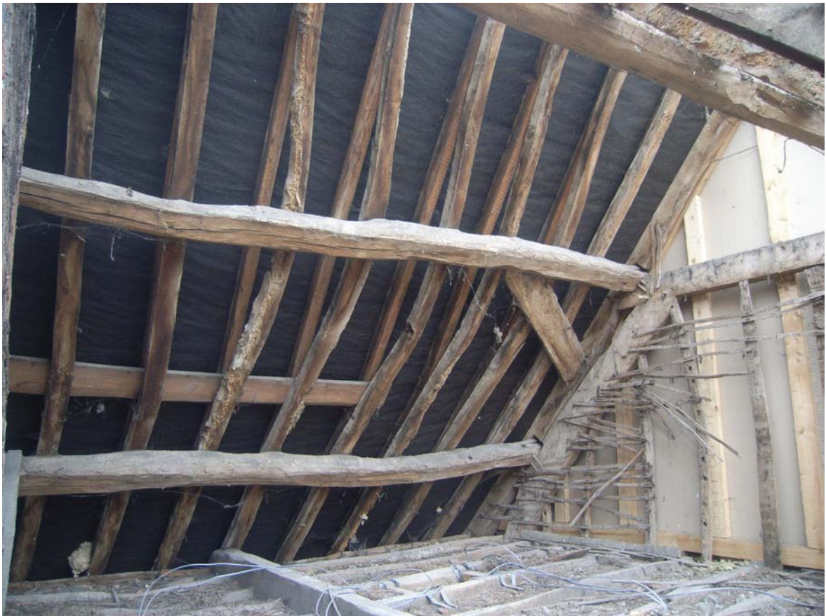
Plate 22: Northern bay roof space looking south-east
