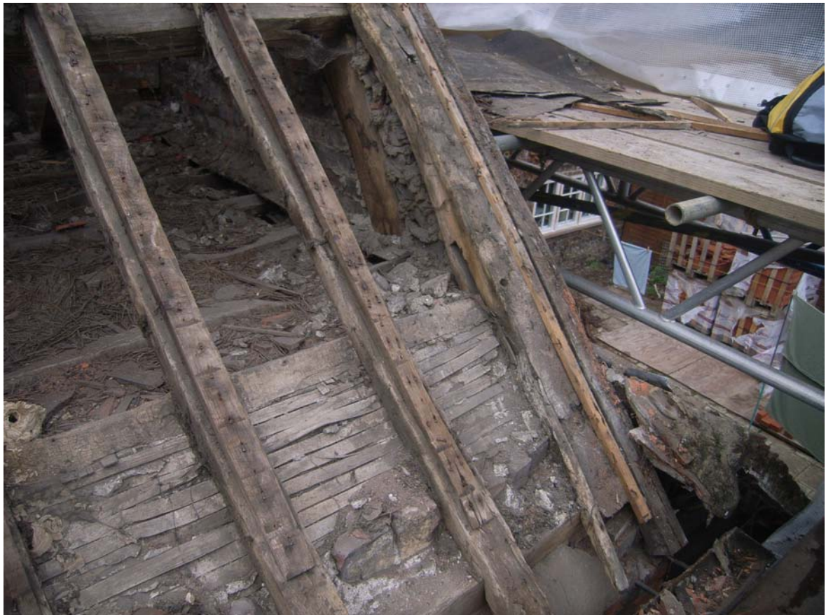
Plate 34: East slope northern end of roof
