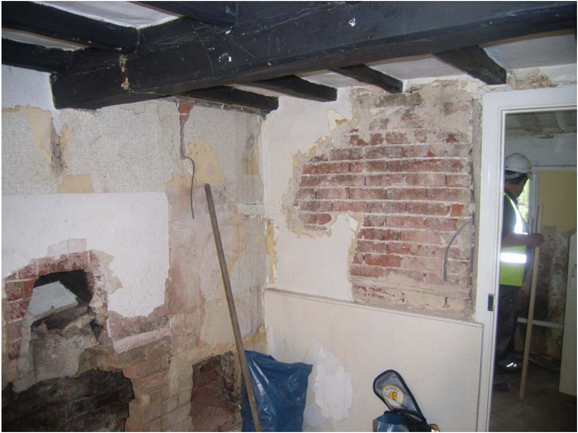
Plate 39: East wall in Room 33A
