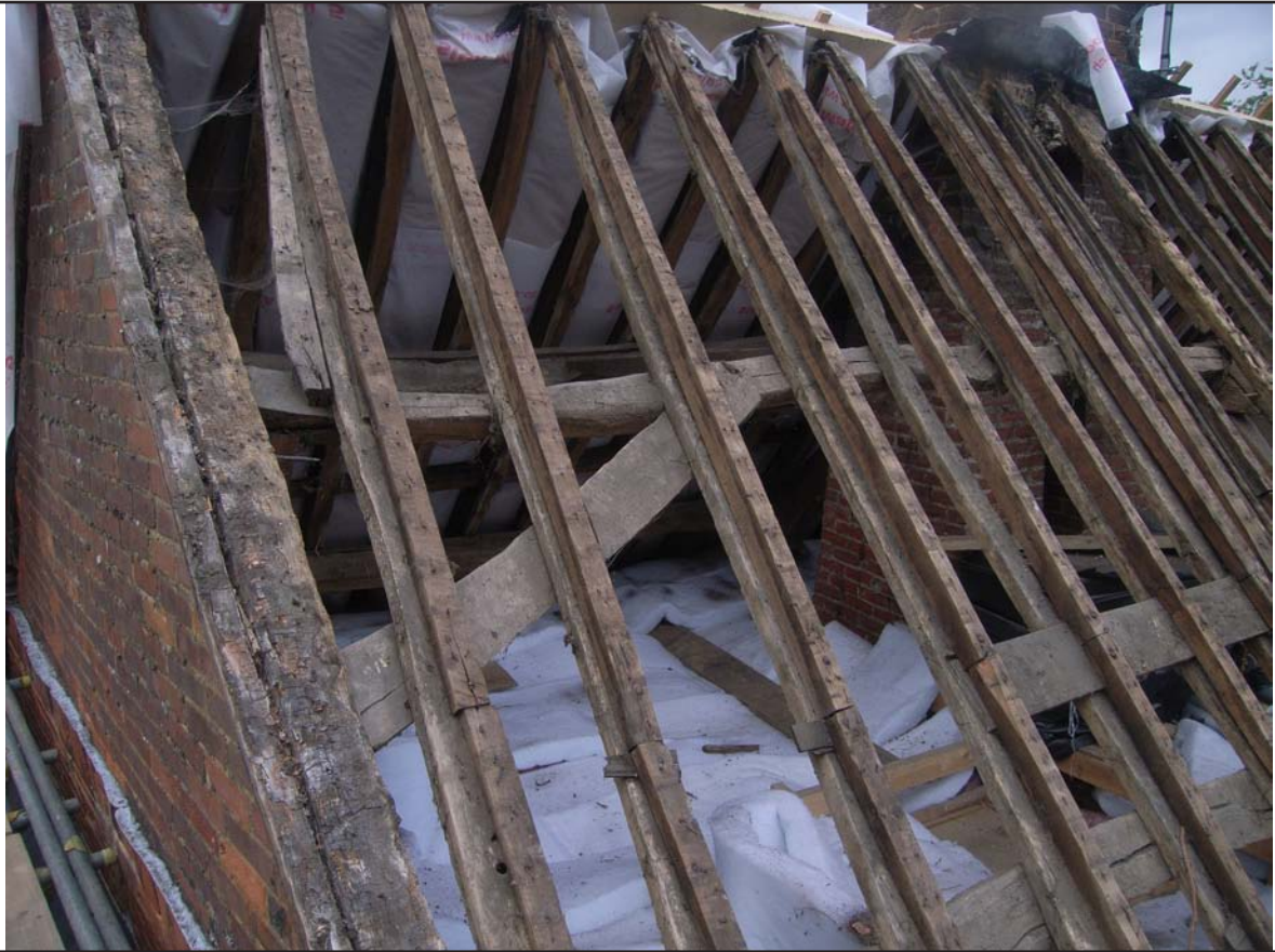
Plate 33: East slope southern end of roof
