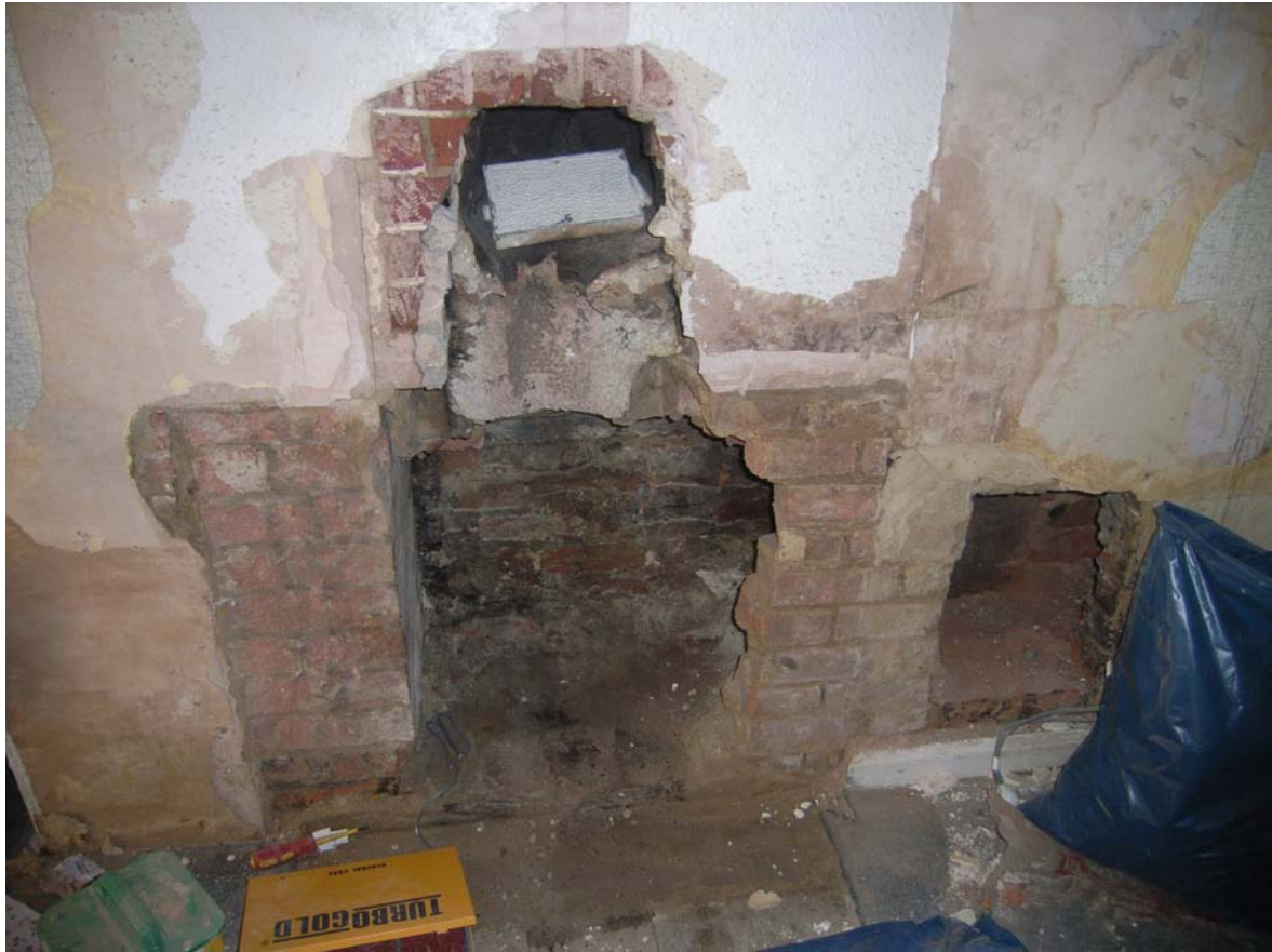
Plate 37: Fireplace in ground floor front room (No.33A)
