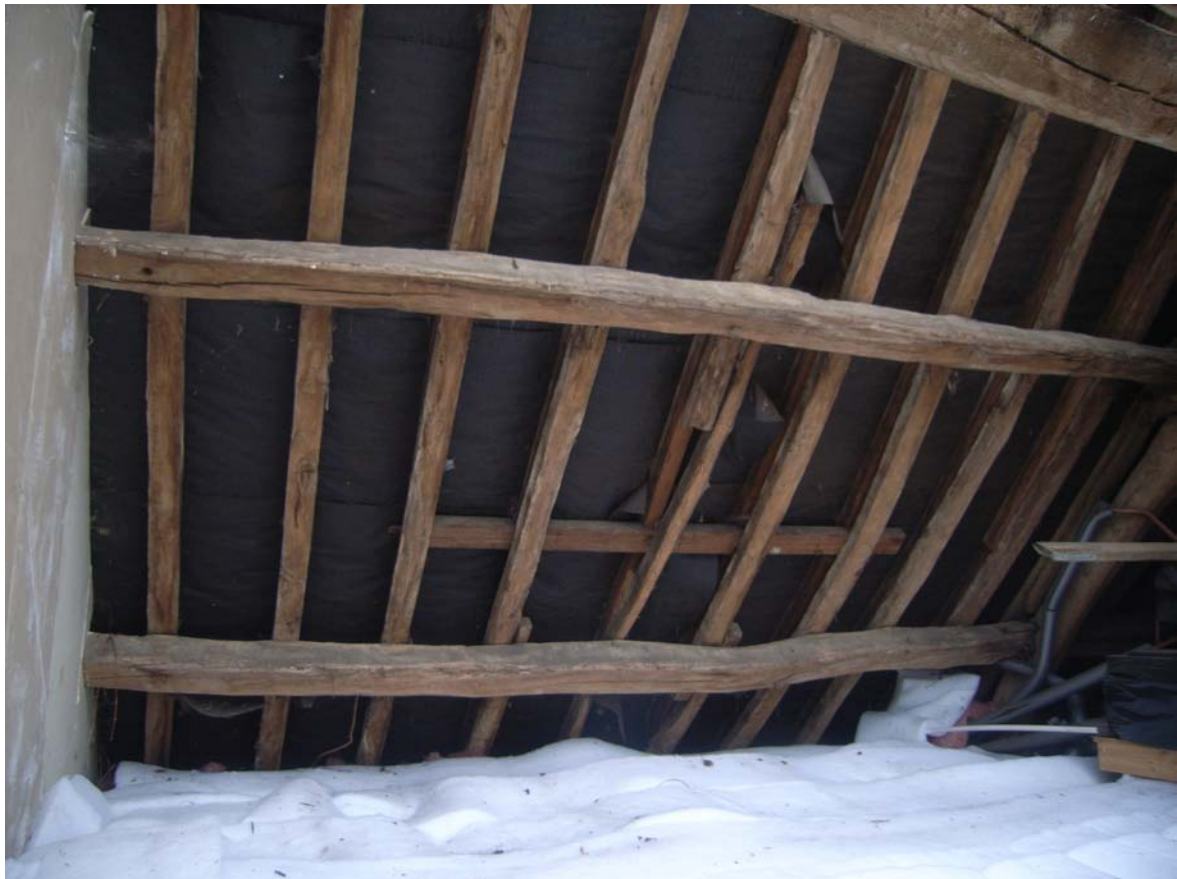
Plate 26: Central bay of roof space, east slope
