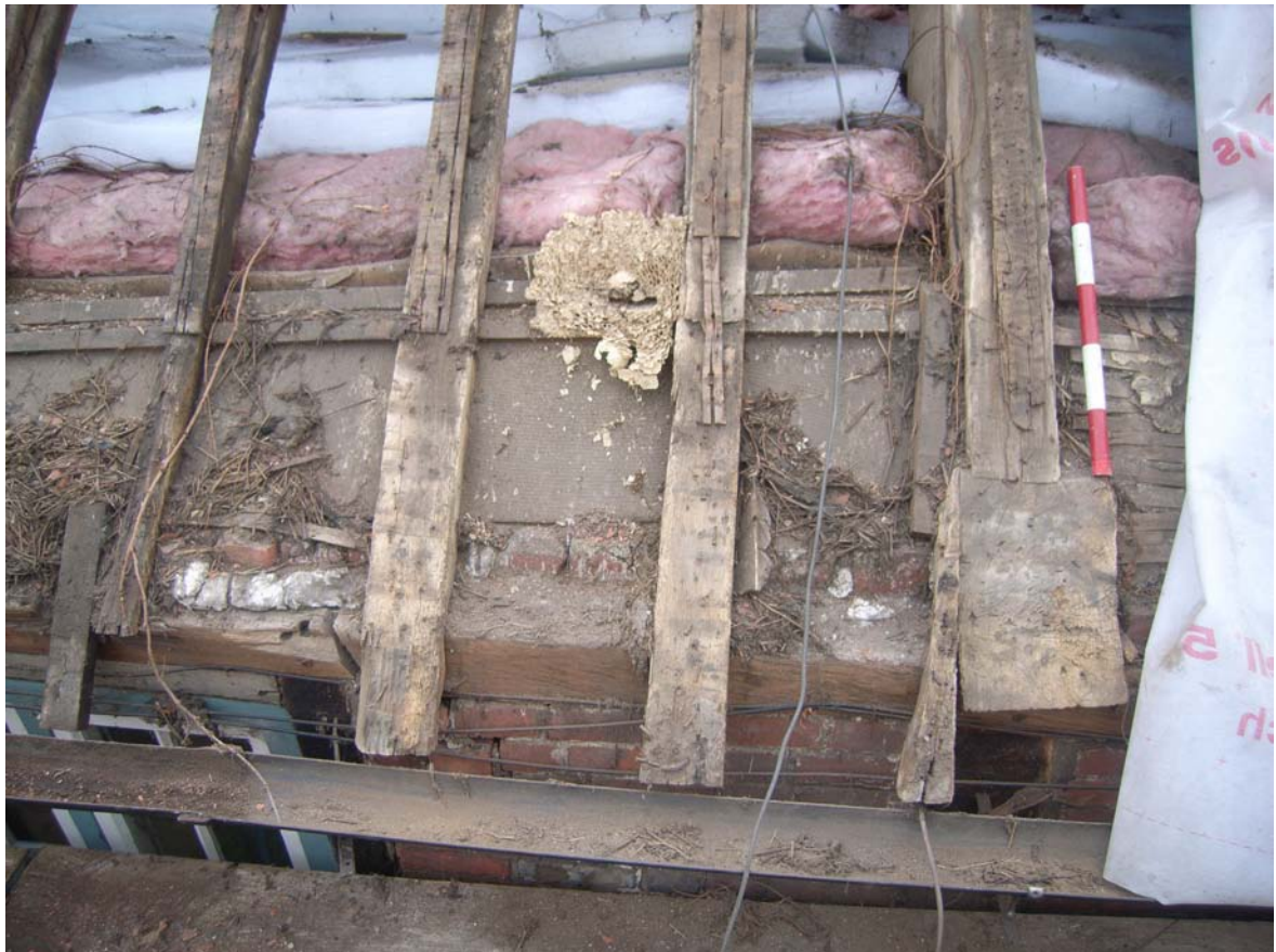
Plate 10: Tie beam and rafter feet in west slope
