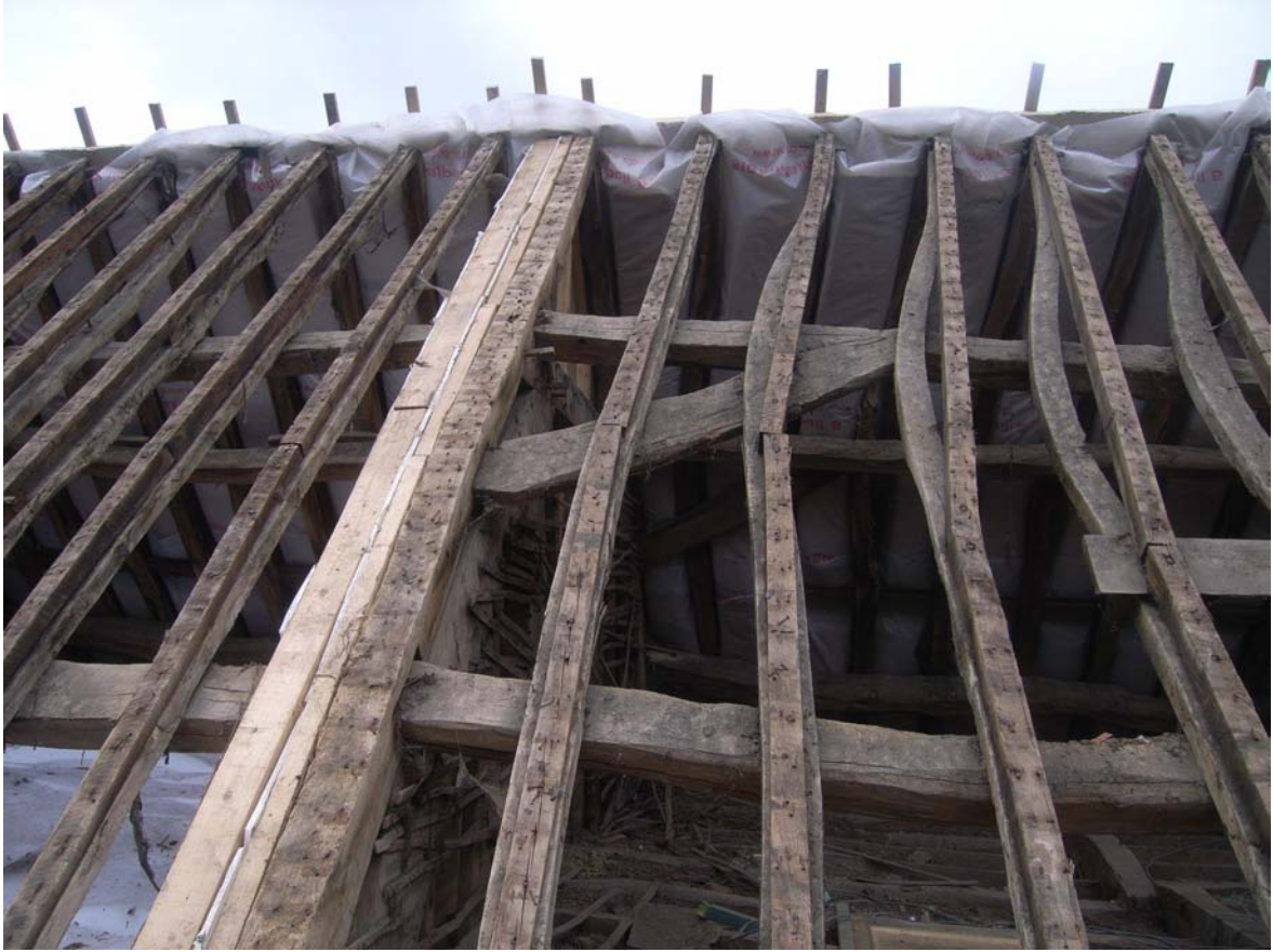
Plate 31: East slope wind brace in northern bay
