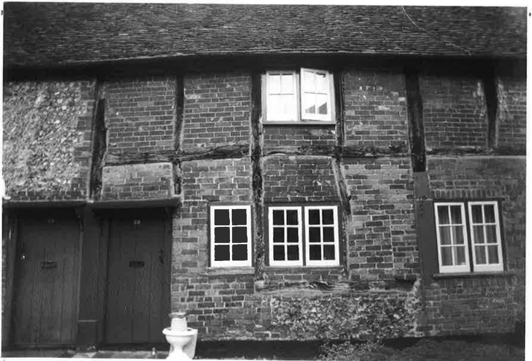
CENTRAL PART OF FRONT ELEVATION. R.251 N.28.
