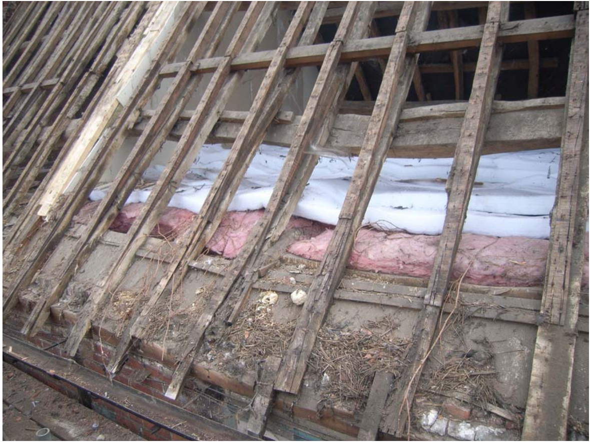
Plate 9: West slope of central bay
