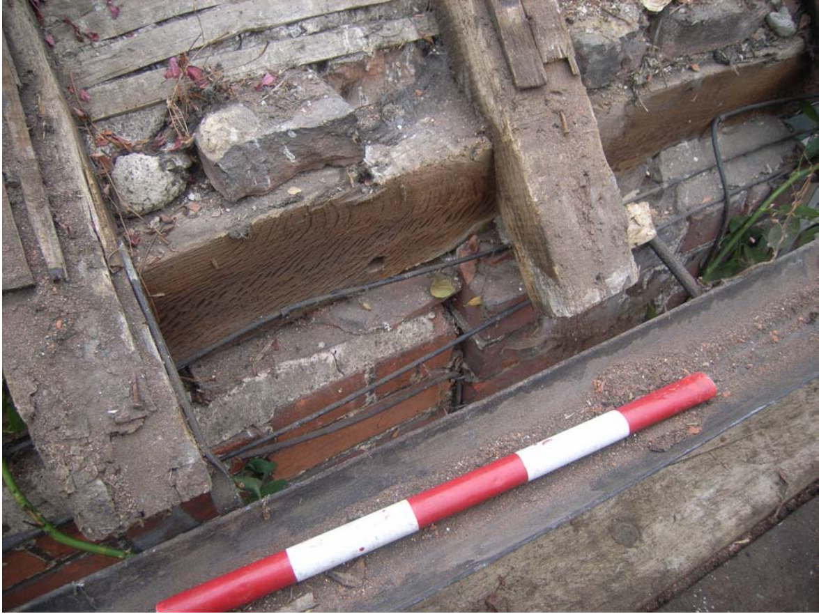
Plate 19: Rafter feet in west slope
