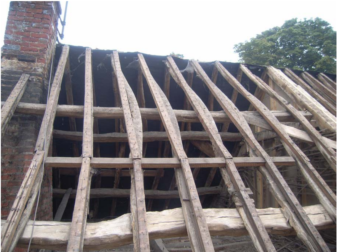
Plate 14: West slope of north bay
