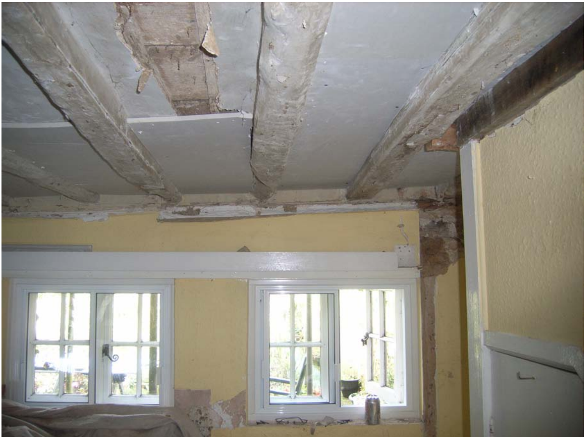
Plate 40: Rear room in No.33 (Room 33B)
