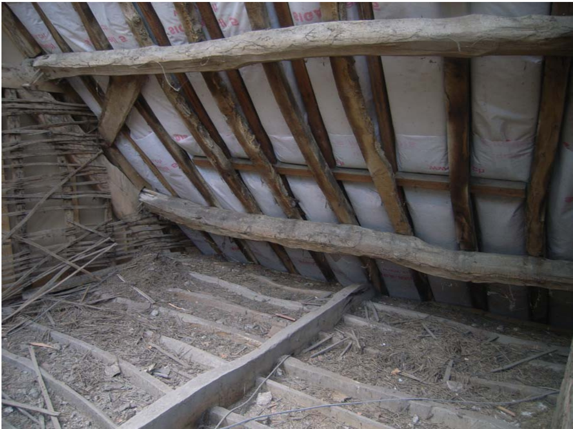
Plate 20: Northern bay roof space looking south-west
