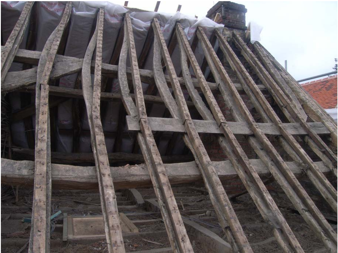
Plate 32: East slope northern bay
