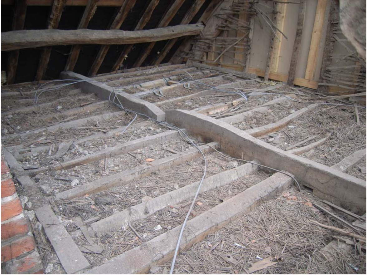
Plate 21: Ceiling joists in northern bay
