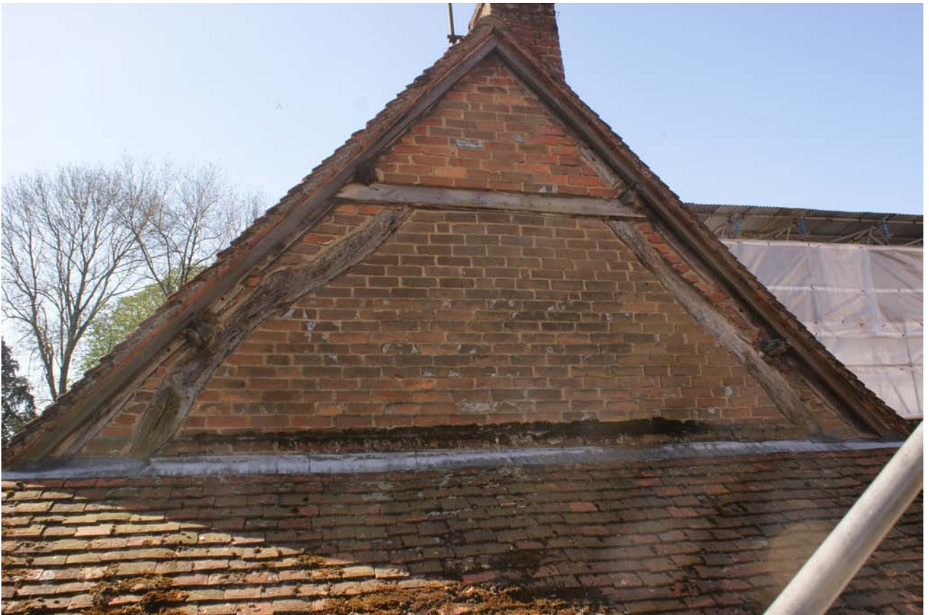
Plate 2: Gable of north elevation above 20th-century lean-to
