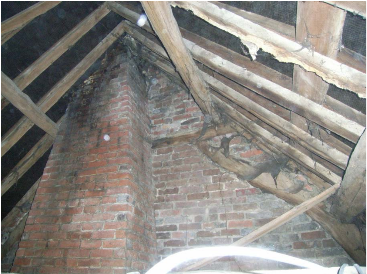
Plate 24: Northern bay of roof space looking north through hatch
