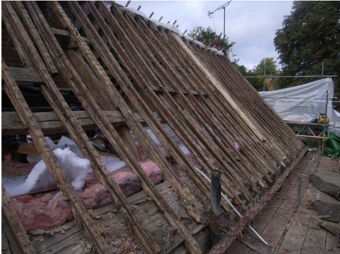
Plate 29: East slope of roof looking north
