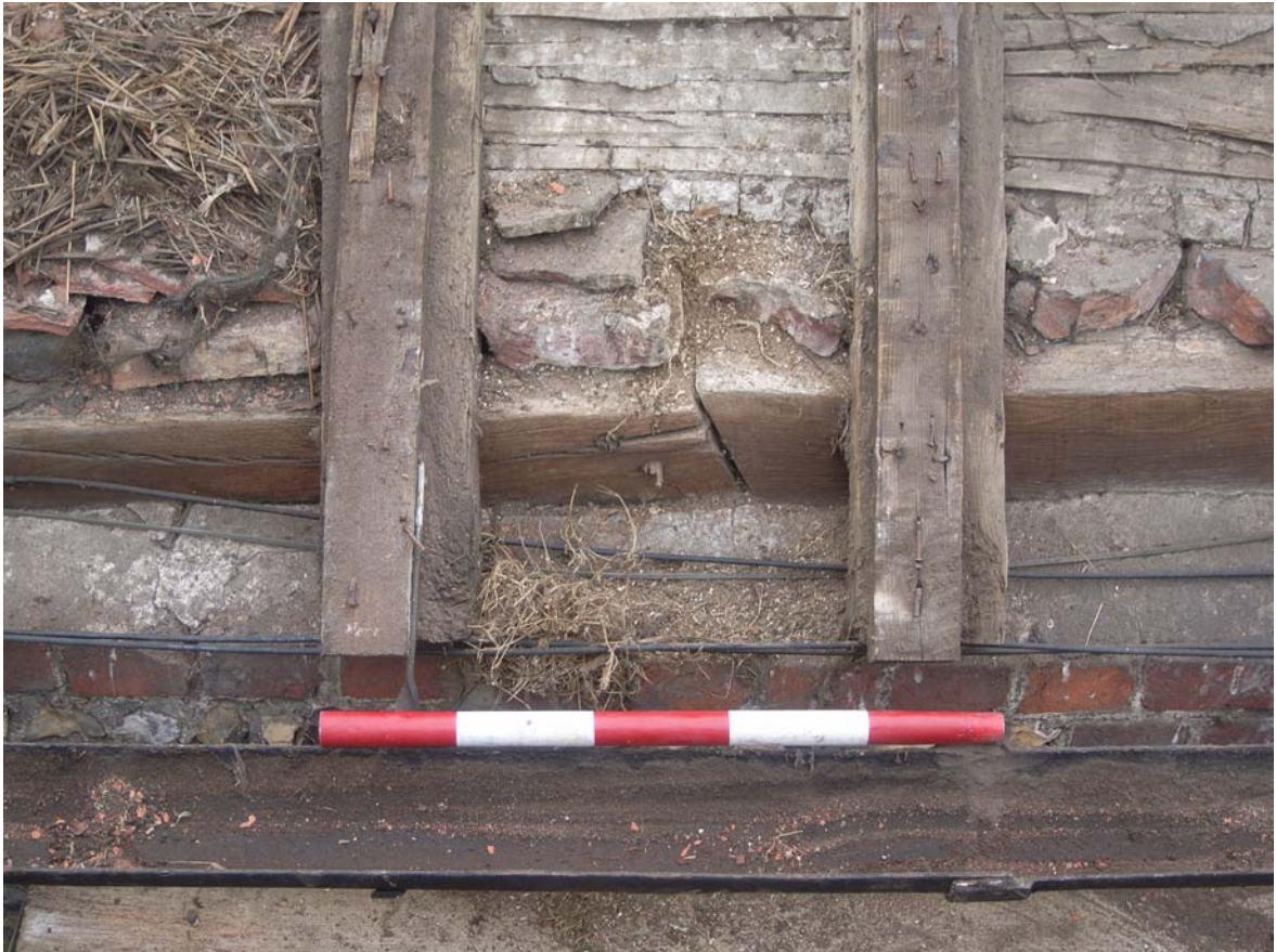
Plate 36: Rafter feet detail
