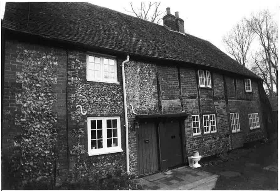
VIEW FROM NORTH-WEST. R.251 N.27
