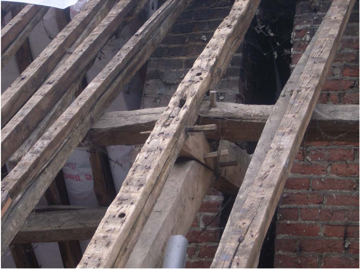
Plate 35: Detail of collar, clasped purlin and curved inner principal
