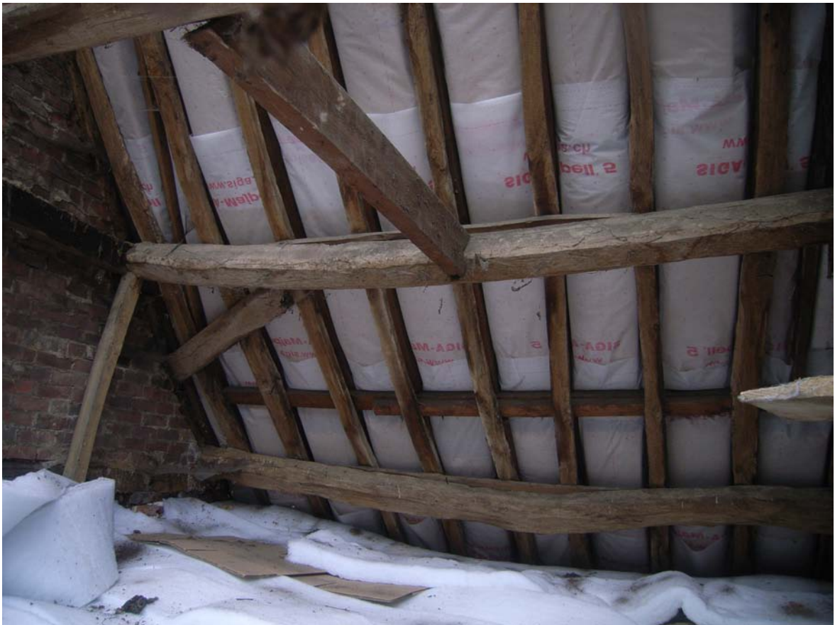
Plate 28: Southern bay roof space, west slope
