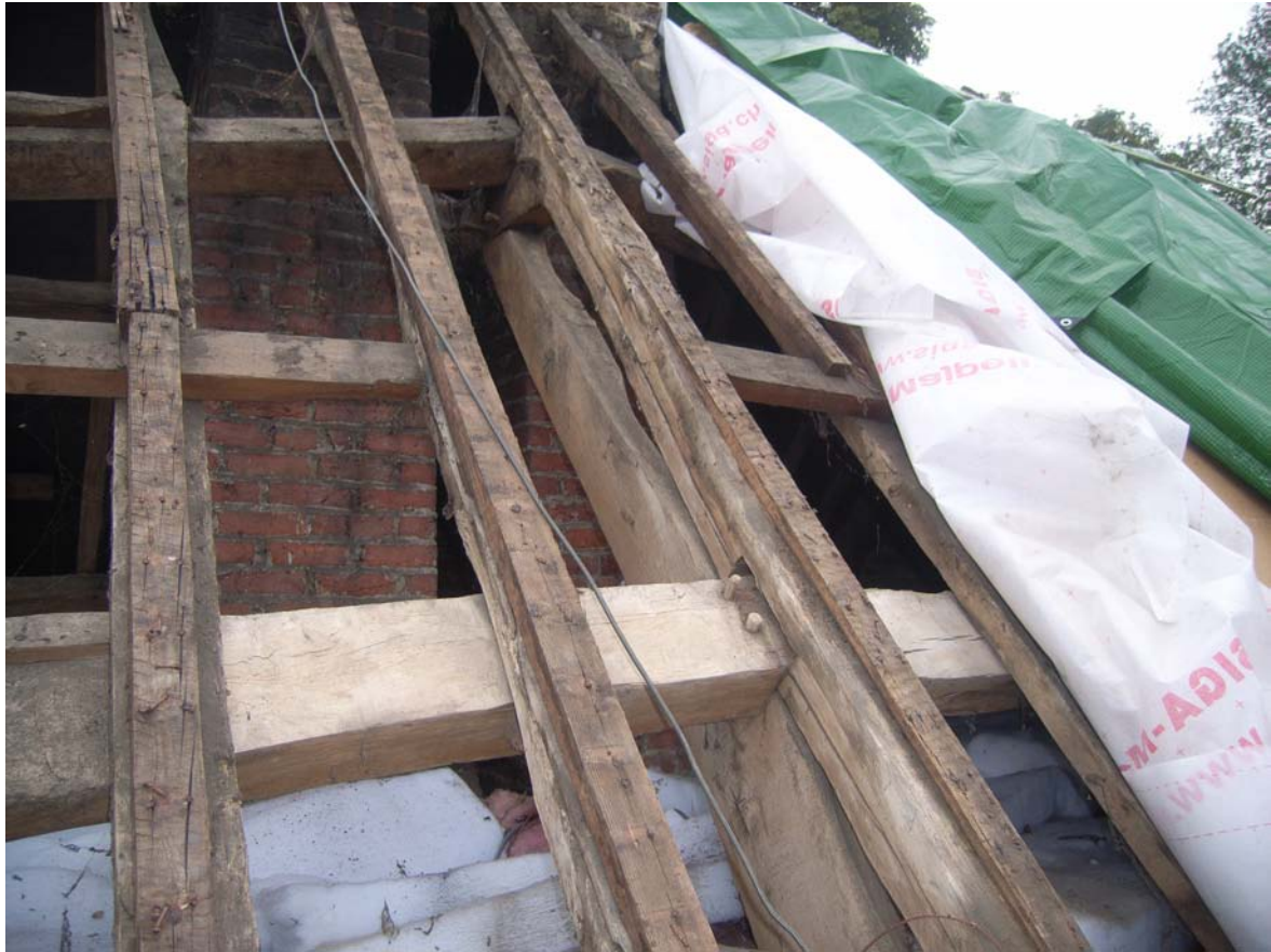
Plate 11: Truss 2 detail, west slope
