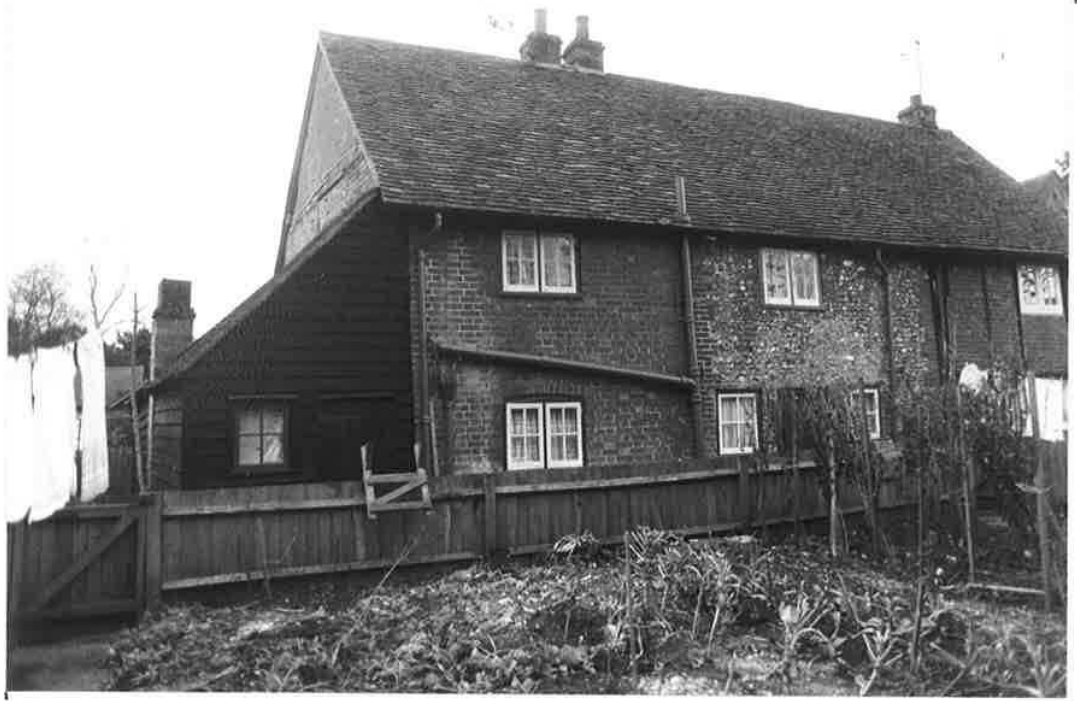
VIEW FROM SOUTH-EAST. R.251 N.25
