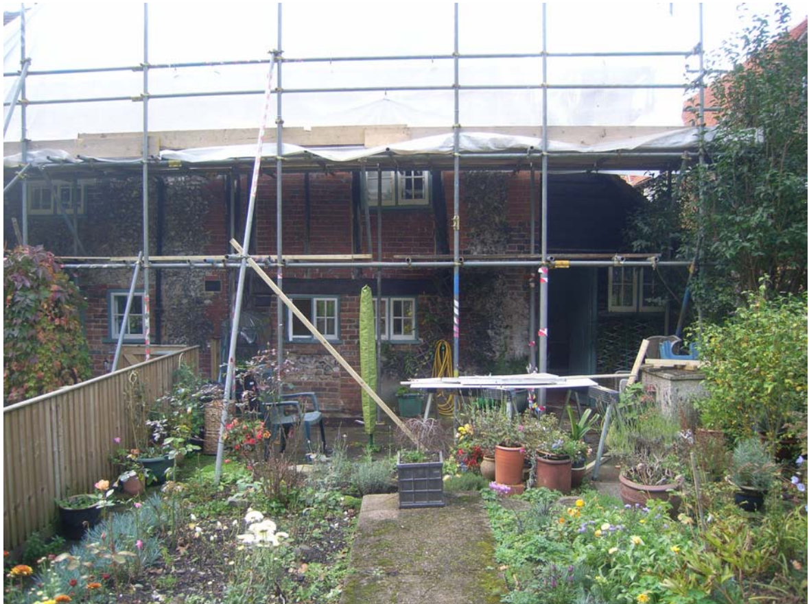
Plate 4: East elevation beneath scaffolding
