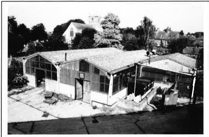
Plate 13: Block 11 towards east side of site
