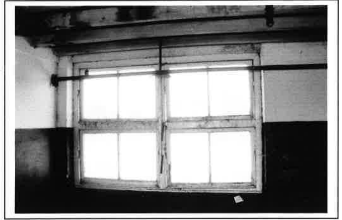
Plate 18: Typical window. West wall of Block 2
