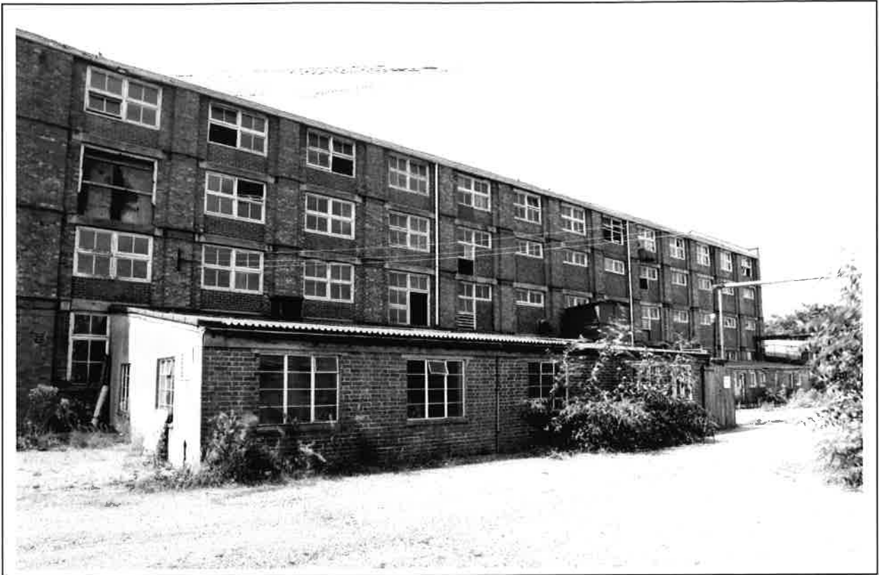
Plate 3: East elevation of main tannery building (Block 2)
