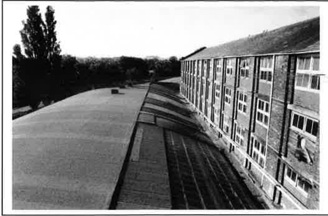
Plate 9: Arched roof over tan yard viewed from Block 1
