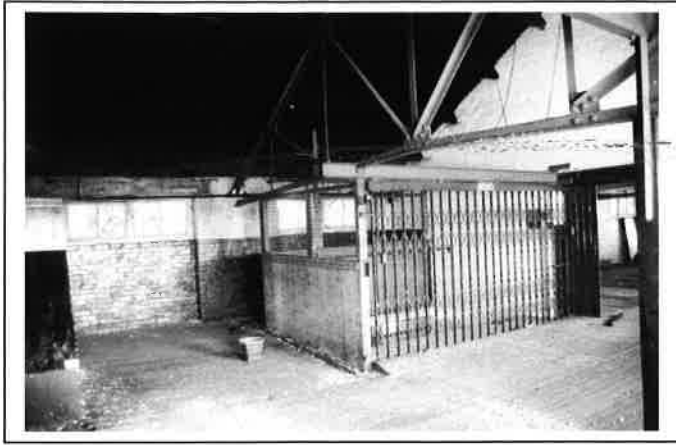
Plate 17: Lift at third floor level
