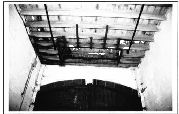
Plate 20: trapdoors over main entrance from south
