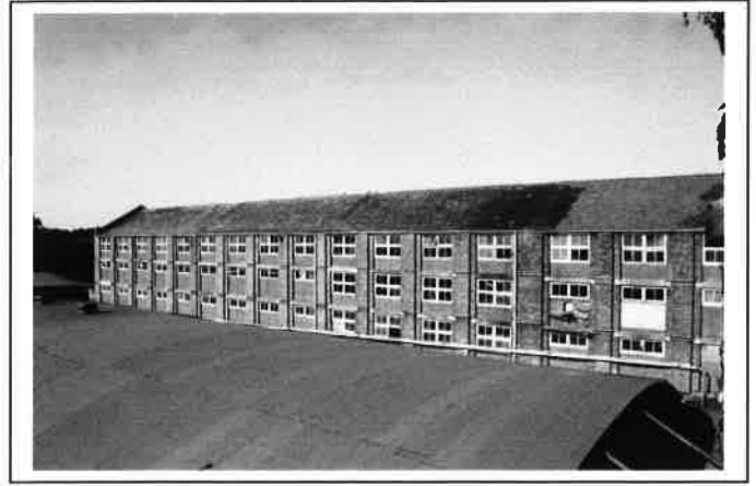
Plate 10: West elevation of Block 2
