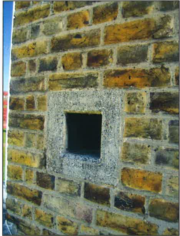
Plate 14: Cable opening in north elevation
