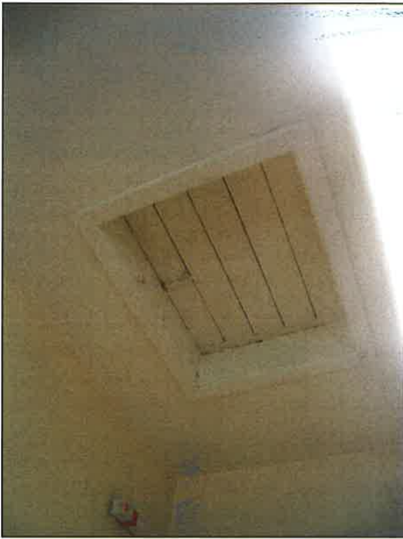
Plate 21: Hatch in ceiling of W/T workshop
