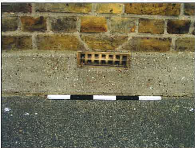
Plate 15: Ventilation hole in north elevation
