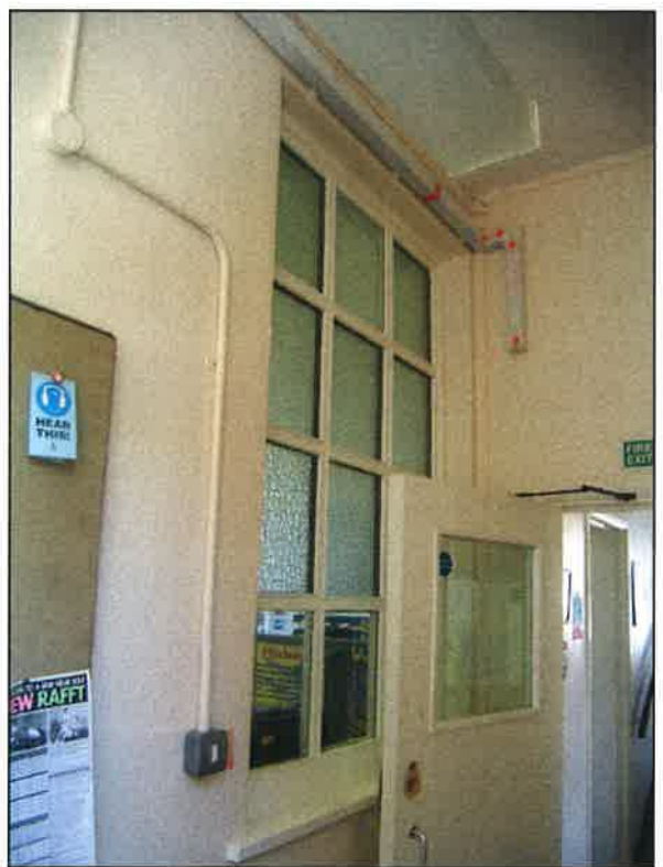
Plate 24: Internal window in former wireless room
