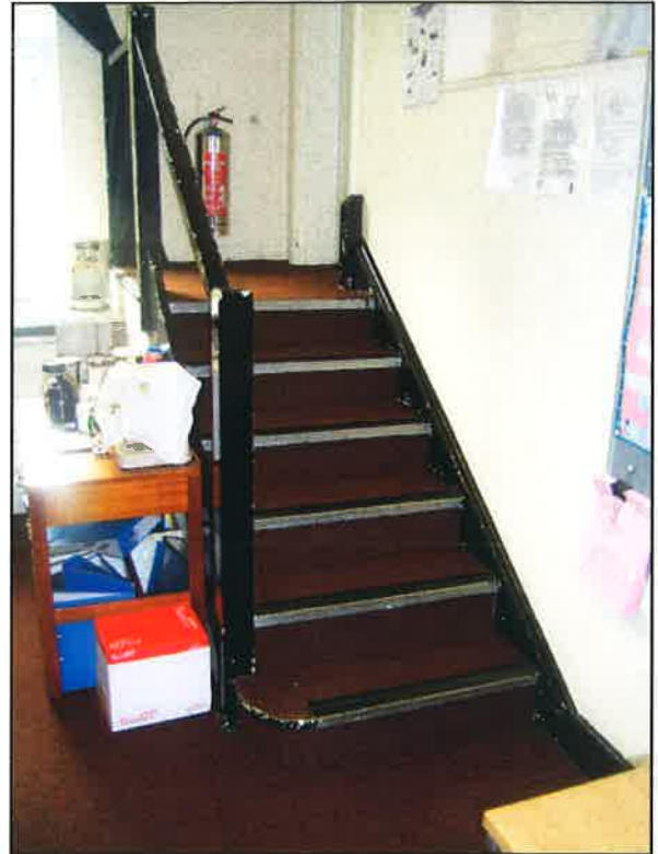
Plate 30: Stairs (probably relocated) in Operations Room
