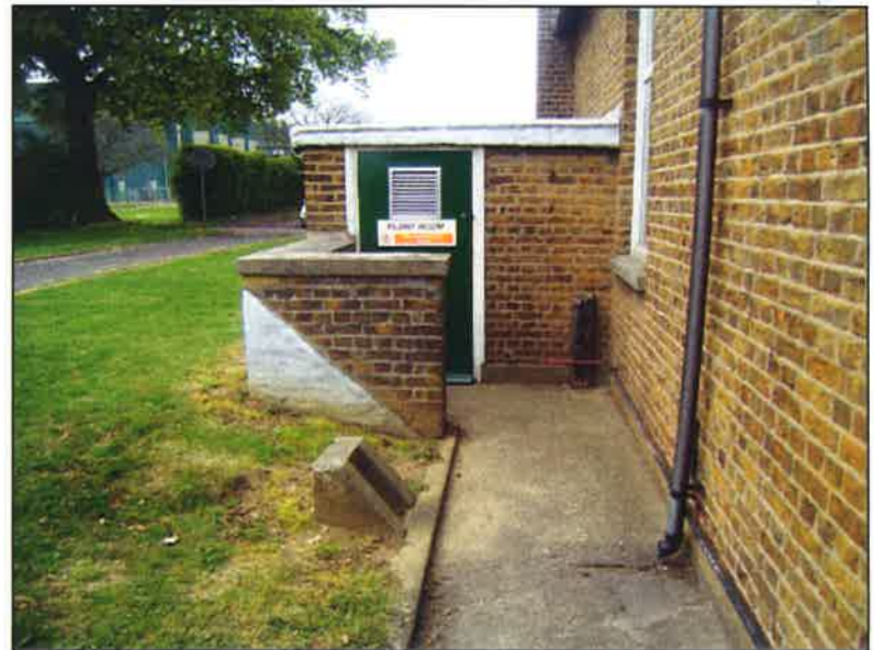
Plate 8: Plant room showing outline of former blast bank and concrete 'shield' around stop cock
