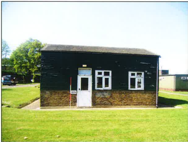
Plate 3: East elevation of 1930s extension
