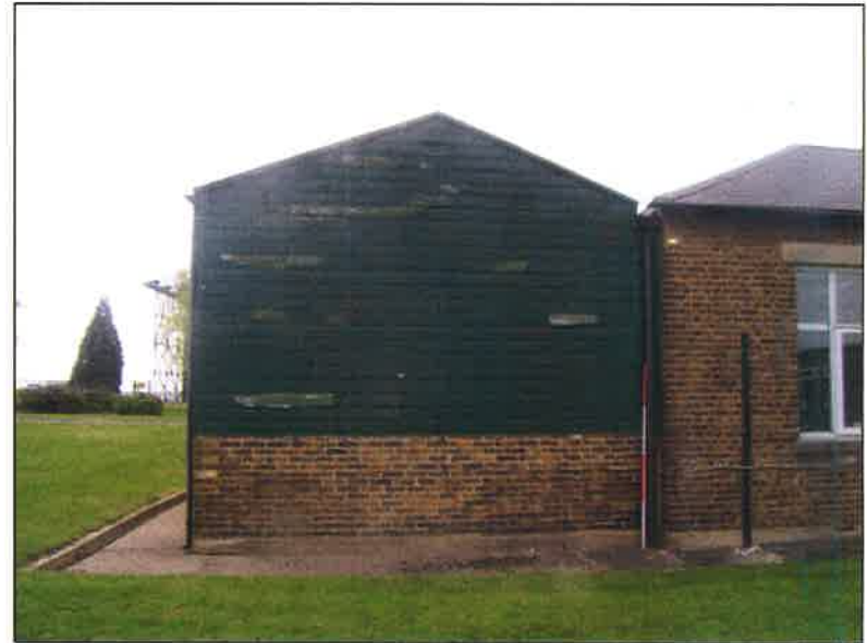
Plate 2: North elevation of 1930s extension
