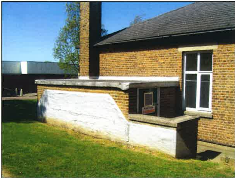
Plate 7: Plant room at west end of south elevation
