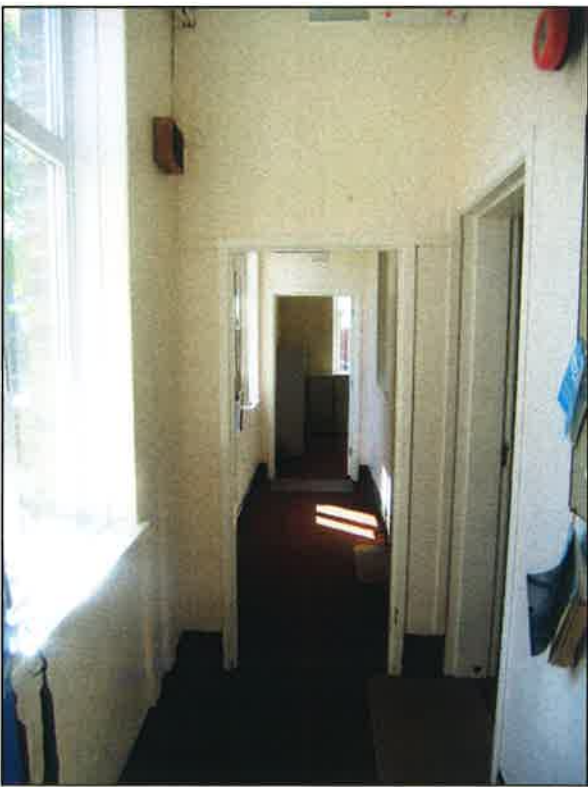
Plate 23: Corridor along south side of building
