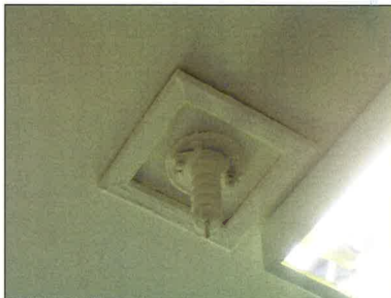
Plate 20: Truncated cable in ceiling of wireless room
