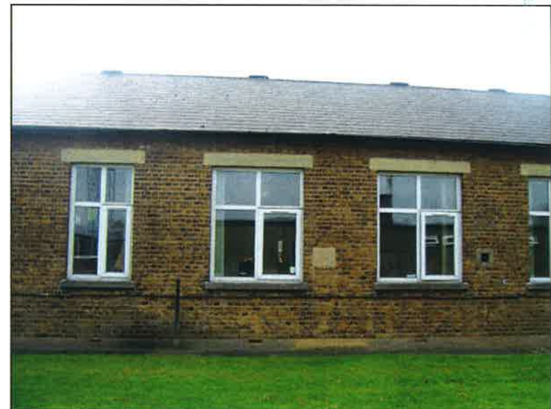
Plate 12: Central section of north elevation
