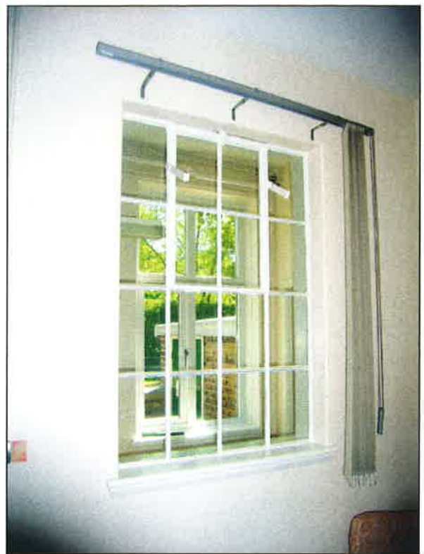
Plate 22: Internal window in former PBX room
