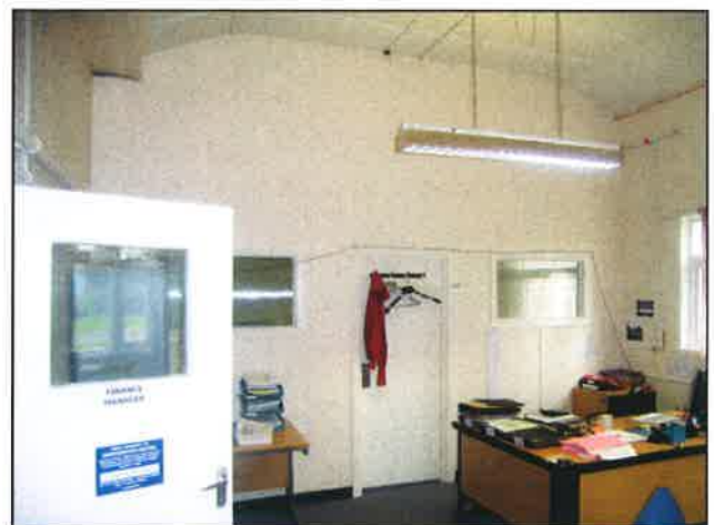
Plate 32: Extension at East end of building
