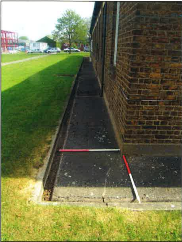
Plate 13: Walkways at north-west corner of building
