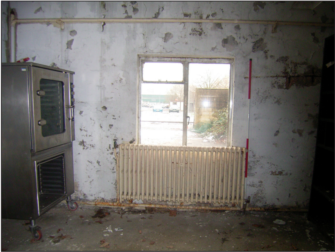
Plate 17: Building 007 - Room E
