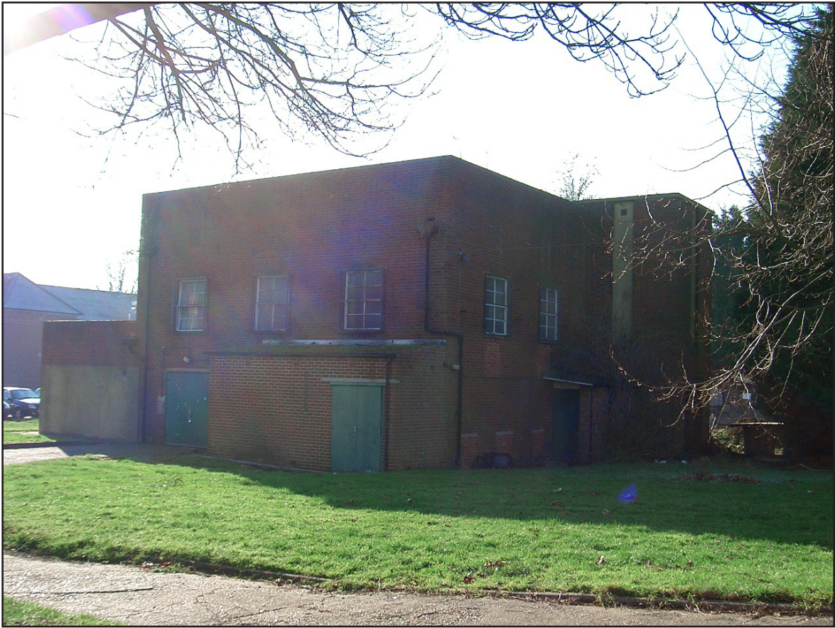
Plate 19: Building 007 - Extension 2 Exterior
