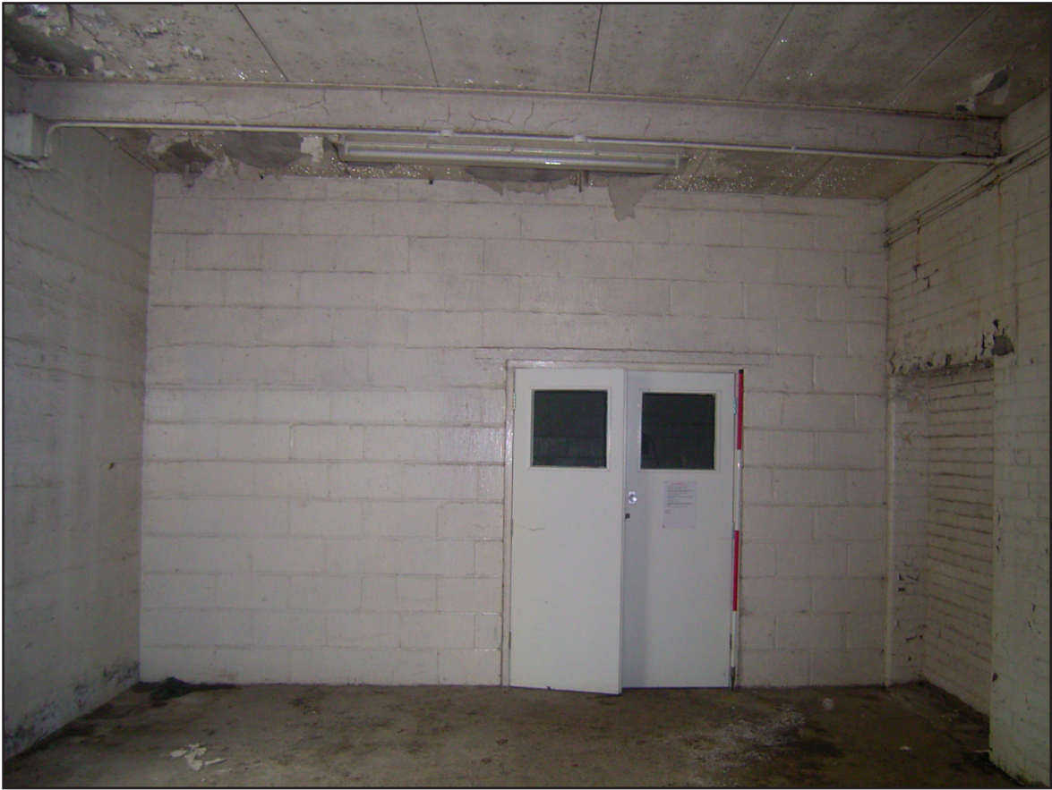
Plate 15: Building 007 - Room C (Respirator Facility)
