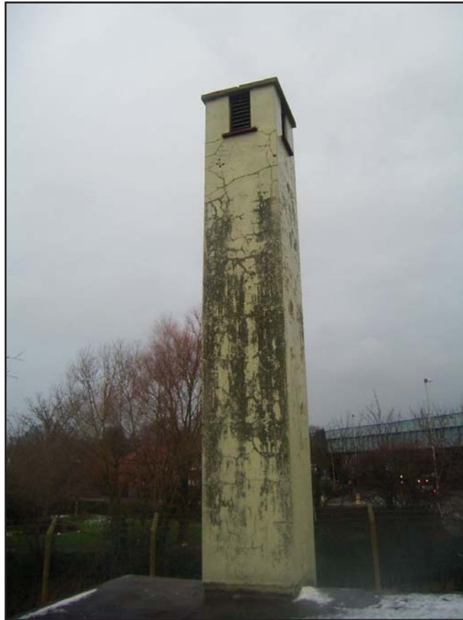
Plate 25: Building 112 - Air-Intake Shaft
