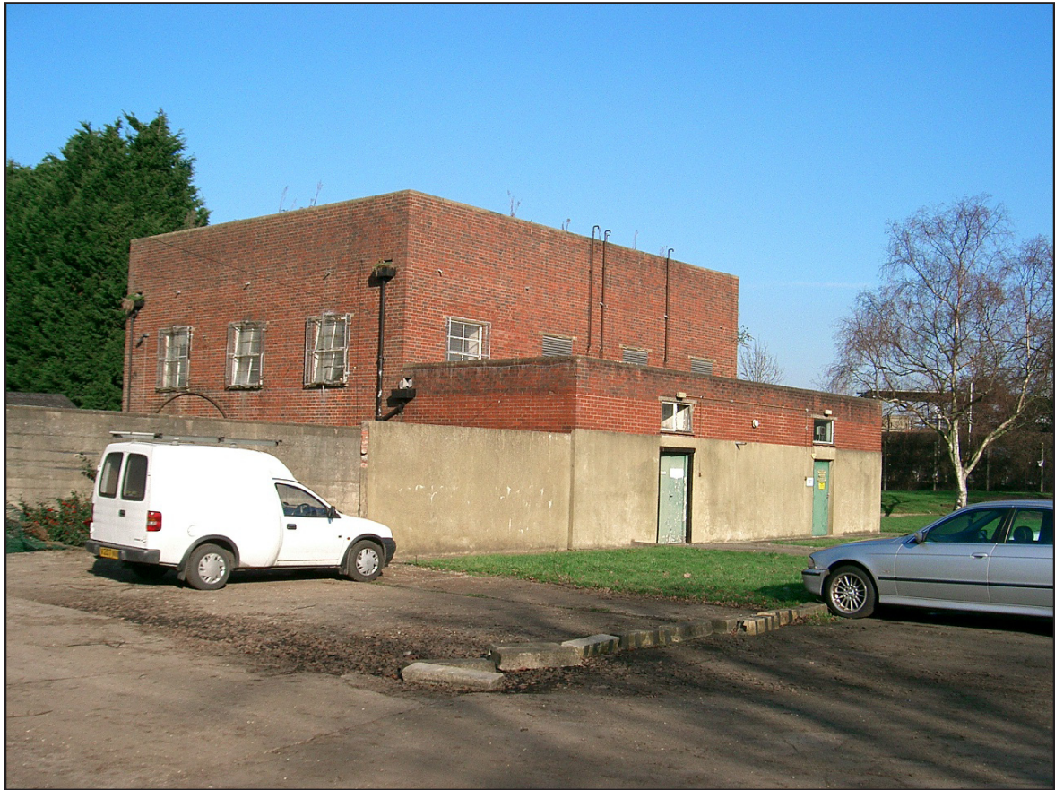
Plate 13: Building 007 - Extension 1 Exterior
