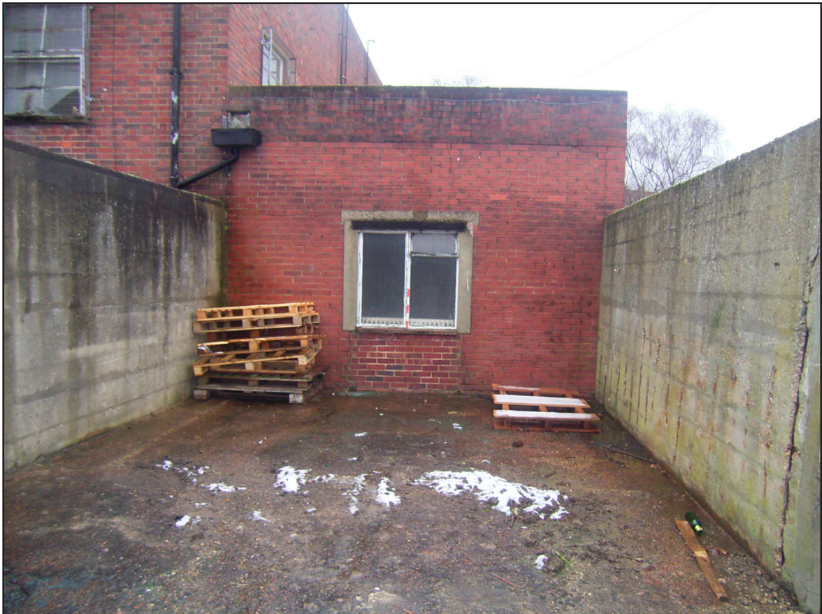
Plate 18: Building 007 - External Storage Area
