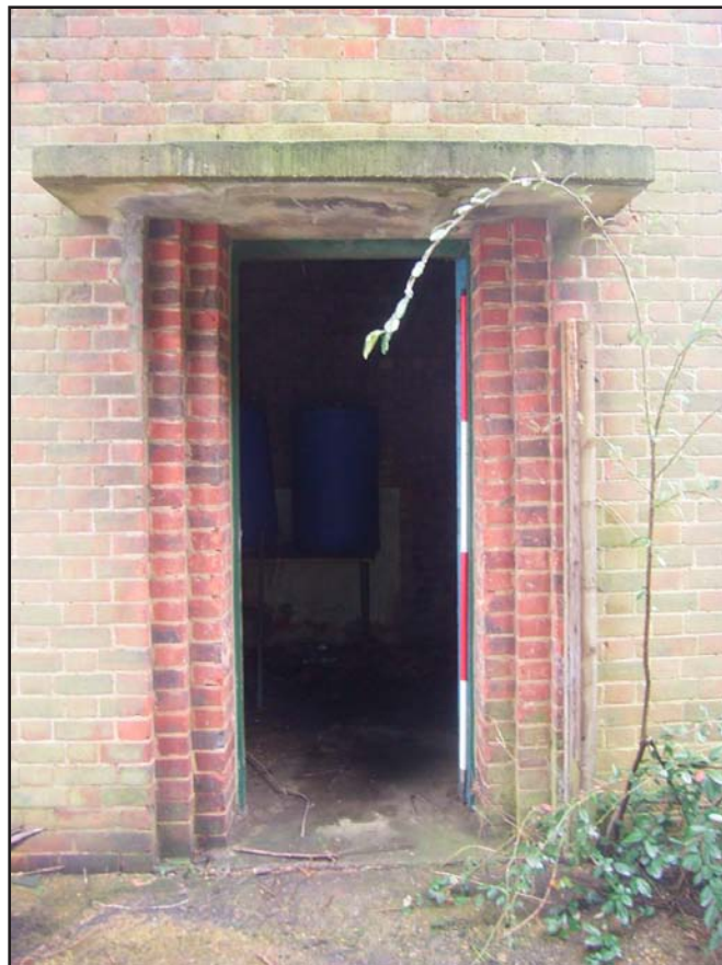
Plate 12: Building 007 - Tower Doorway
