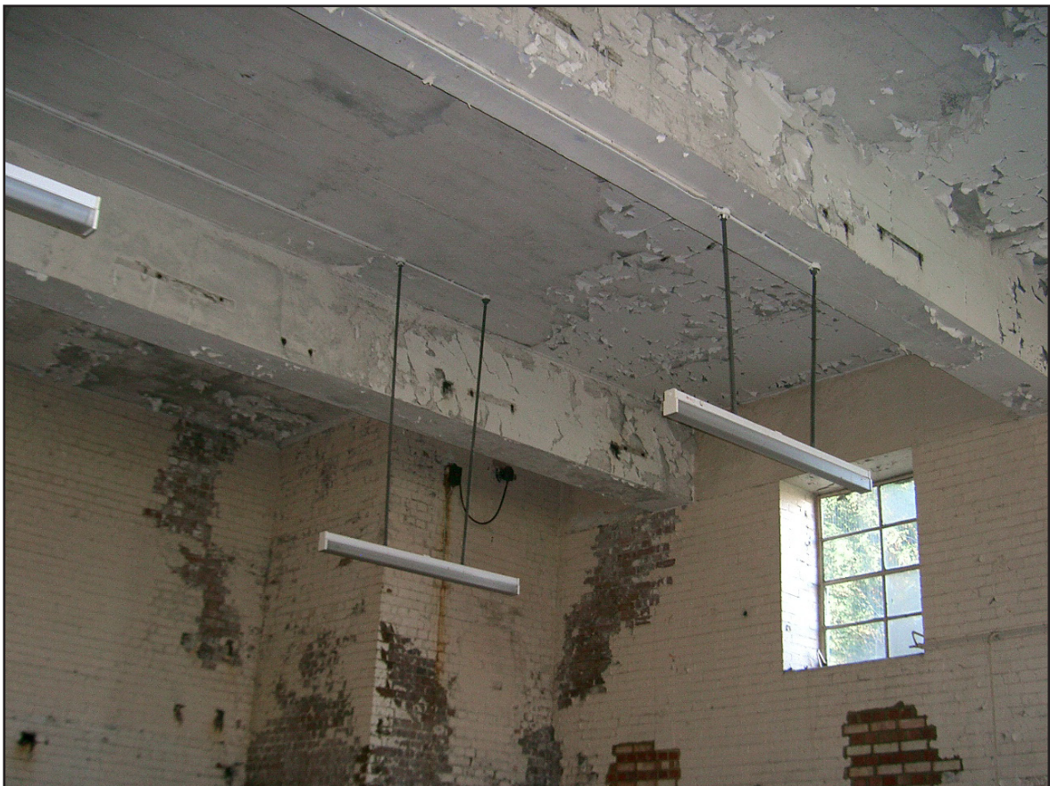
Plate 8: Building 007 - Main Build Interior Showing Concrete Beams
