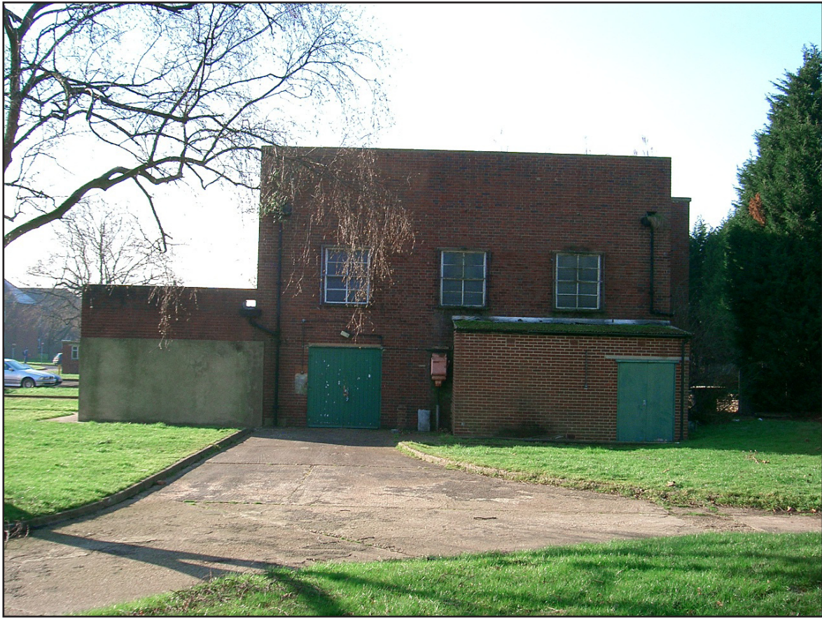
Plate 1: Building 007 - South West Facing Elevation
