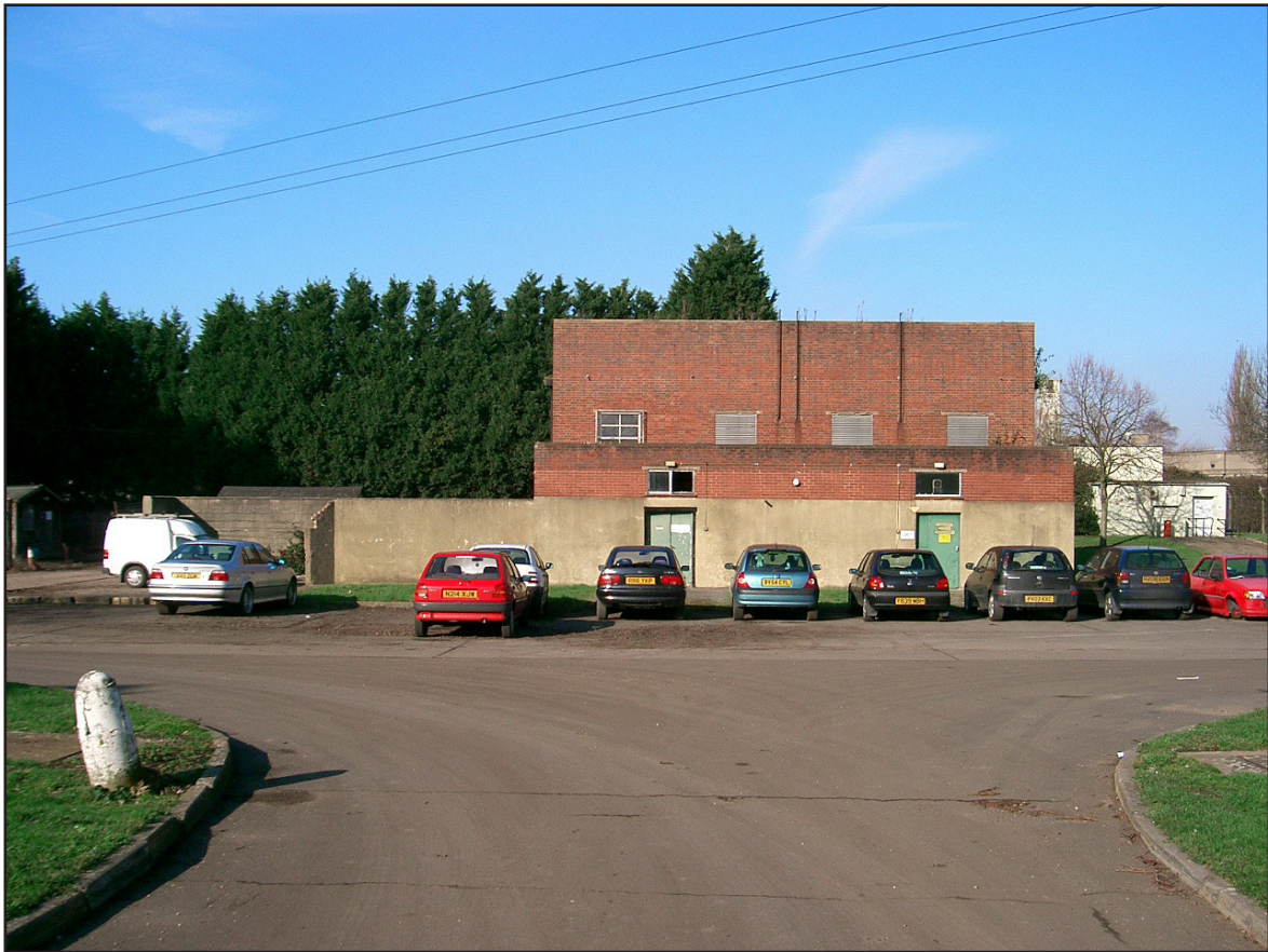
Plate 2: Building 007 - North West Facing Elevation
