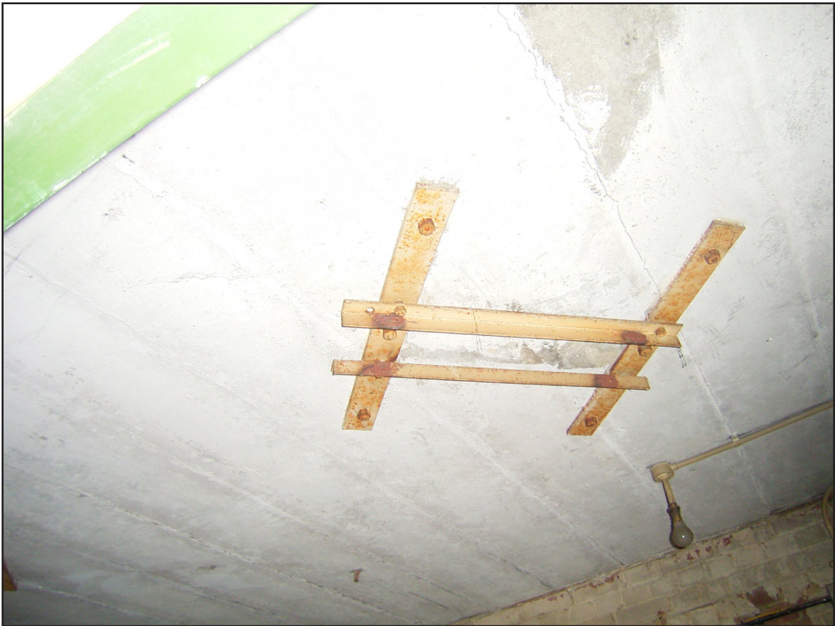
Plate 36: Building 112 - Original Fixtures
