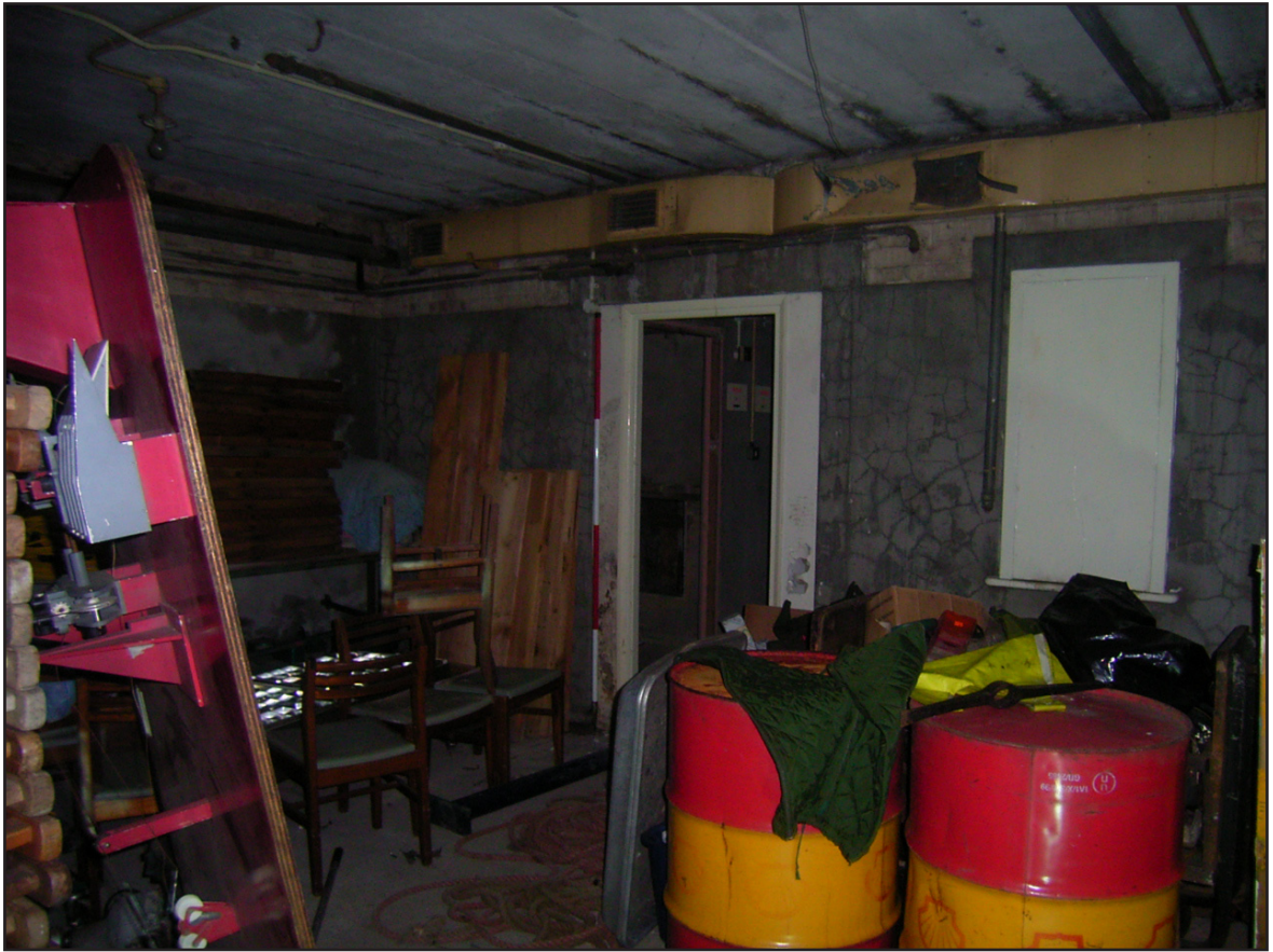
Plate 29: Building 112 - Room 2 Looking Through to Room 6 (Corridor)
