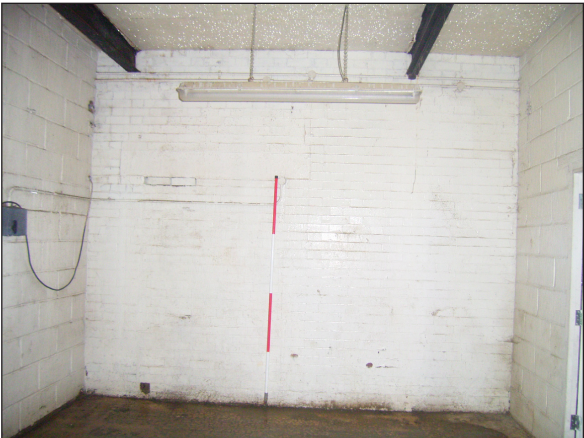
Plate 16: Building 007 - Room D (Respirator Facility)
