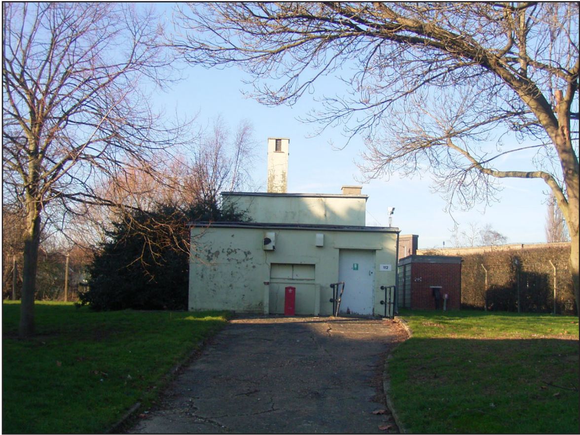
Plate 21: Building 112 - North West Facing Elevation
