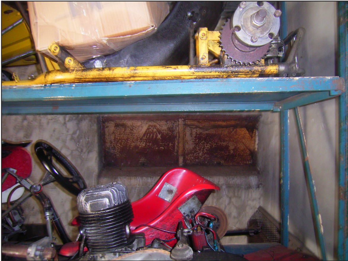
Plate 27: Building 112 - Contaminated Clothing Hatches
