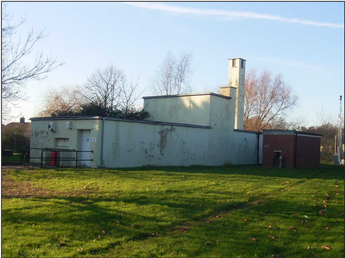
Plate 22: Building 112 - South West Facing Elevation
