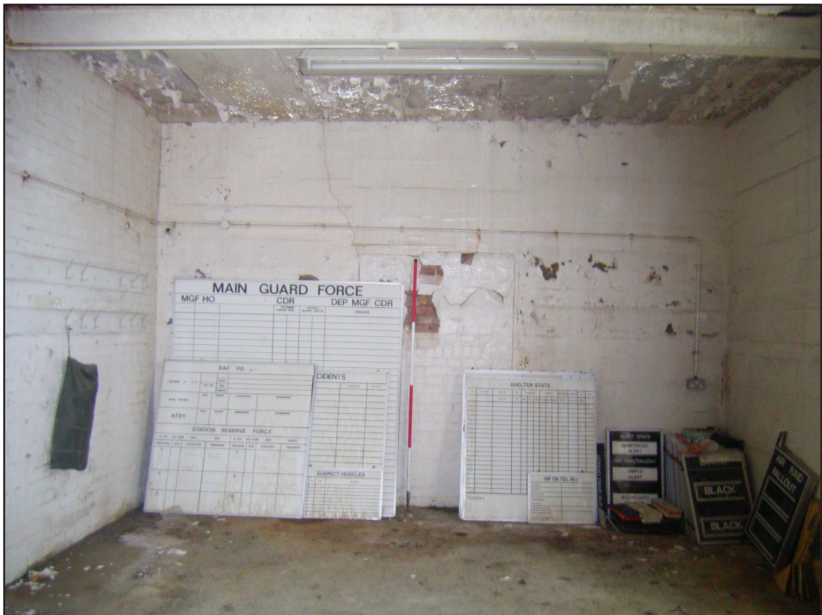
Plate 14: Building 007 - Room C (Respirator Facility)
