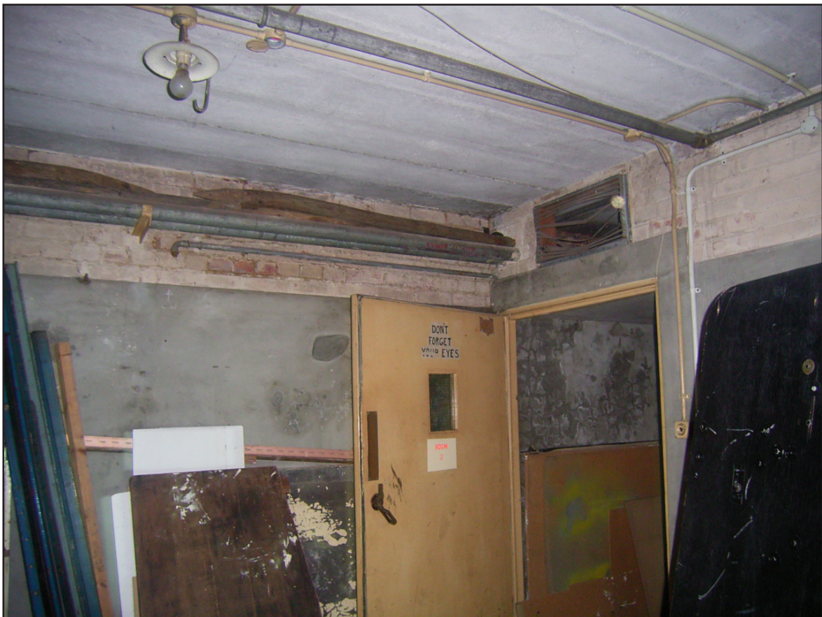
Plate 28: Building 112 - Room 2 Looking Through To Airlock in Room 1
