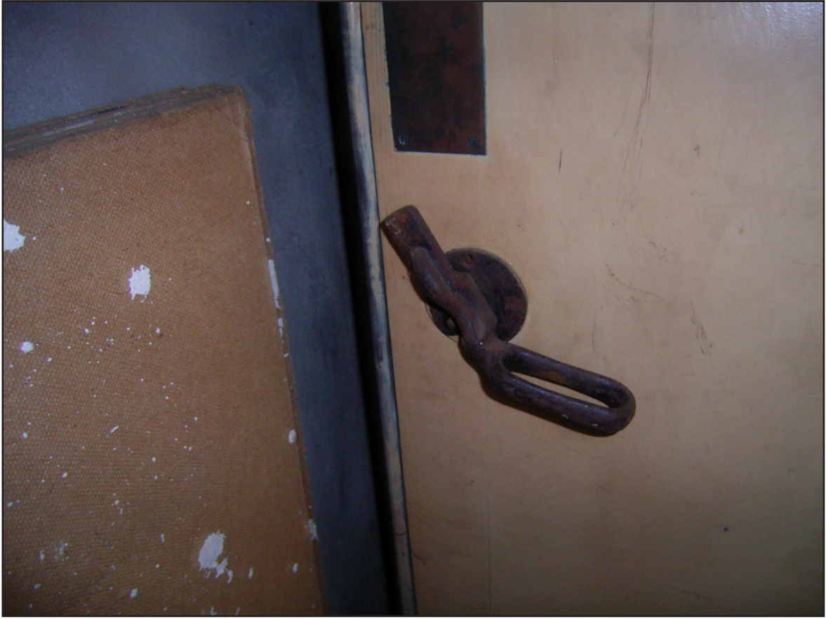
Plate 37: Building 112 - Original Fixtures
