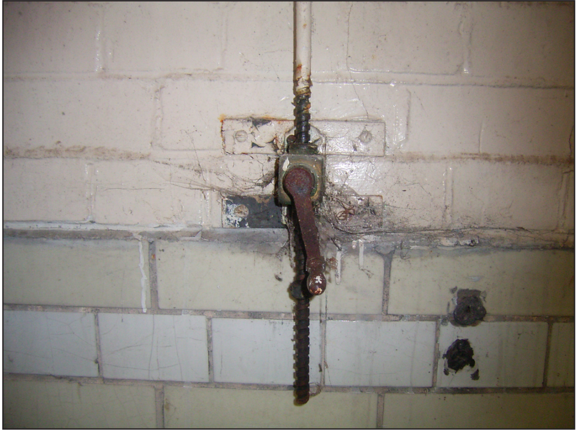
Plate 9: Building 007 - Original Window Fixtures
