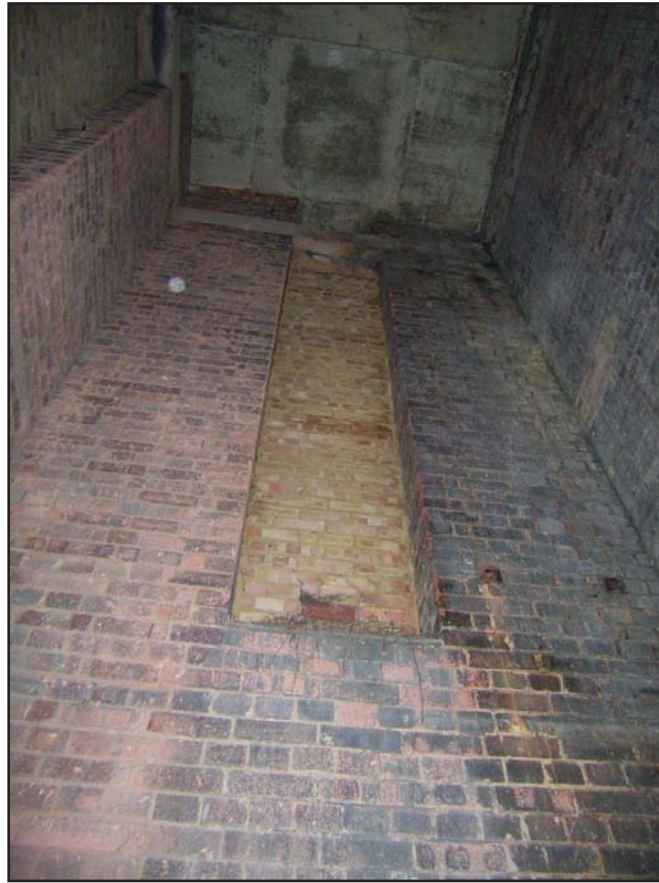
Plate 11: Building 007 - Tower Interior
