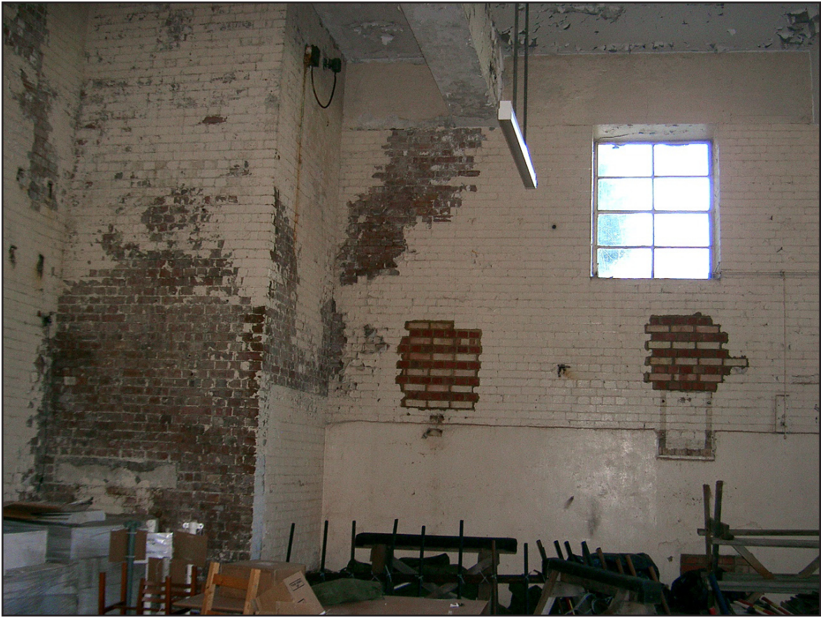
Plate 5: Building 007 - Room A (Main Build Interior)
