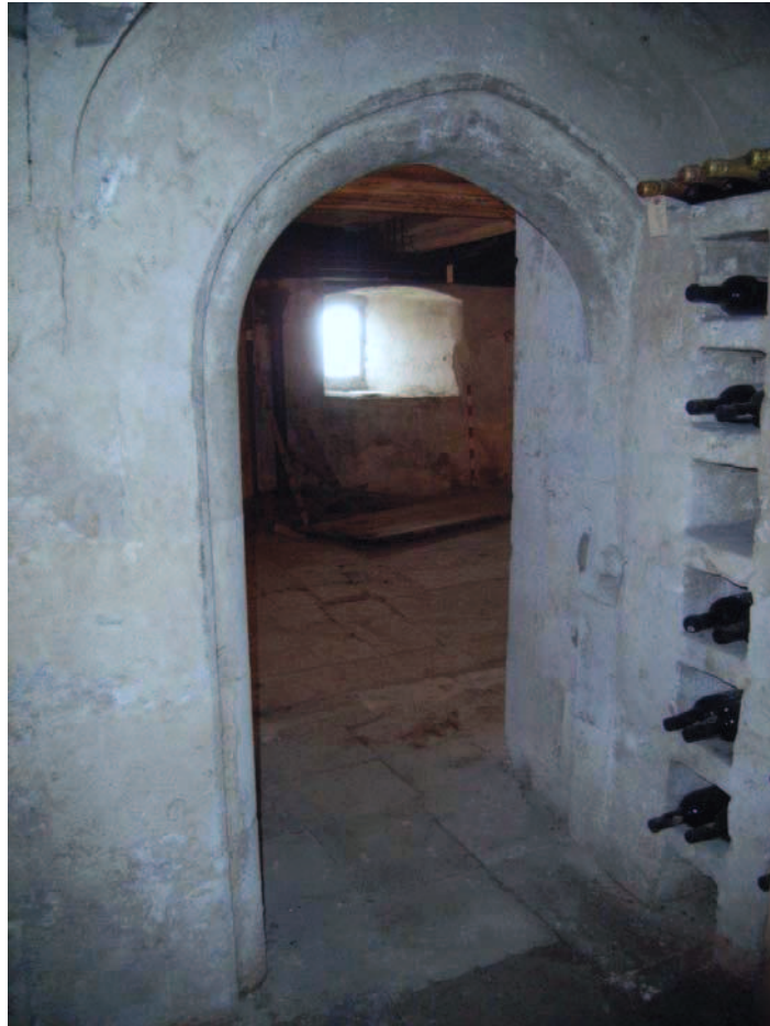
Plate 21: Doorway of Wine Cellar, facing north
