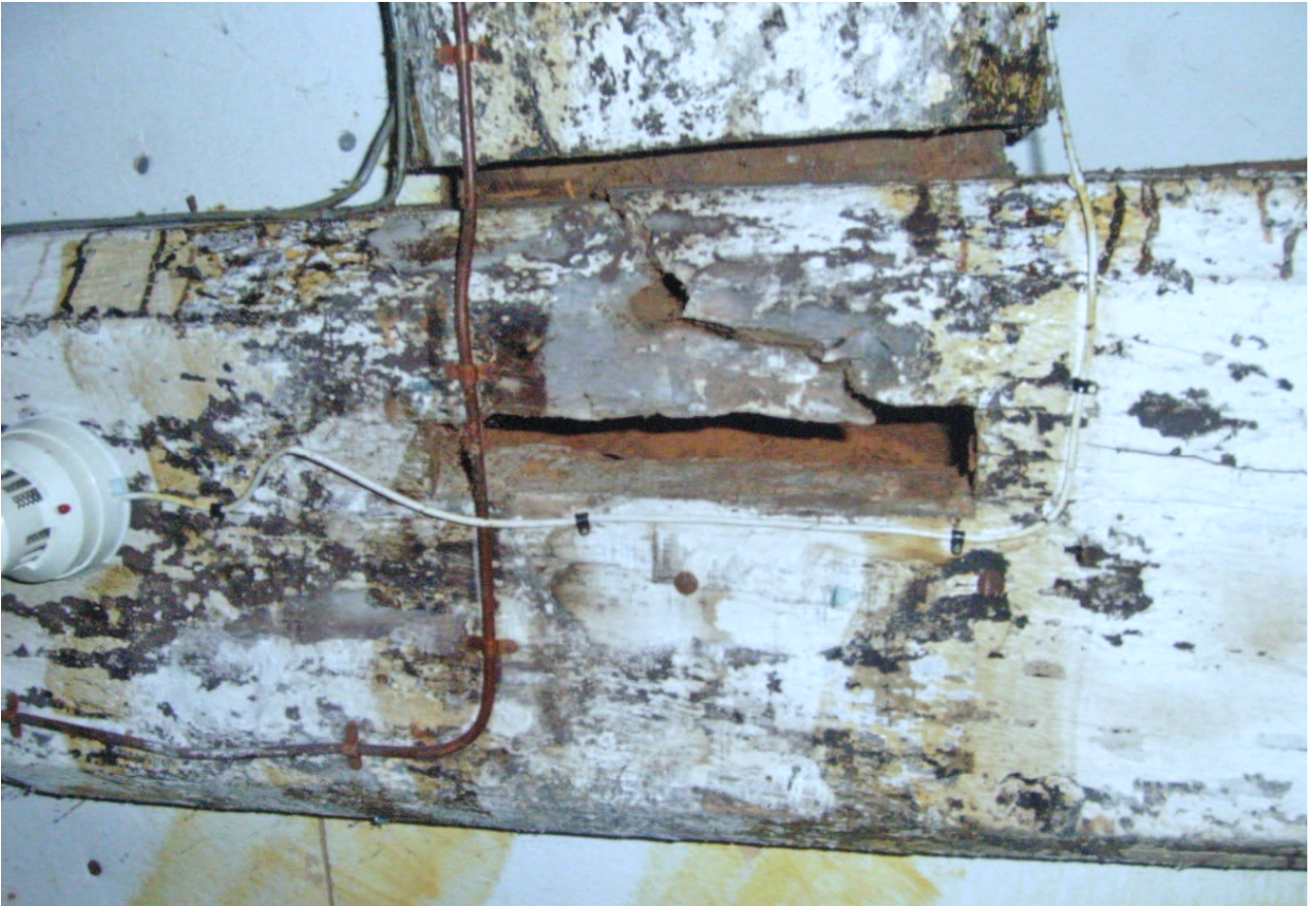
Plate 29: Tenon in Transverse Beam 12 in Area 3
