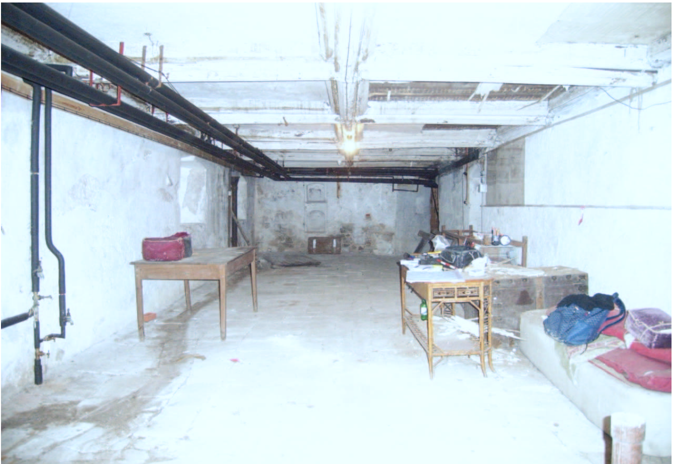
Plate 6: General, Area 2, facing east
