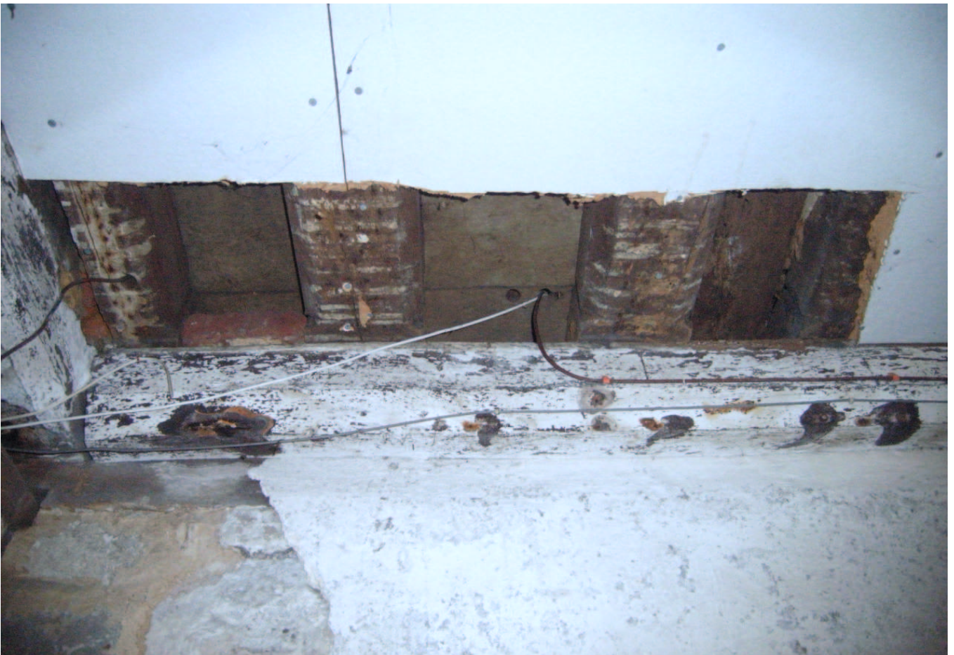
Plate 16: Chamfered common joists in Area 2, facing south
