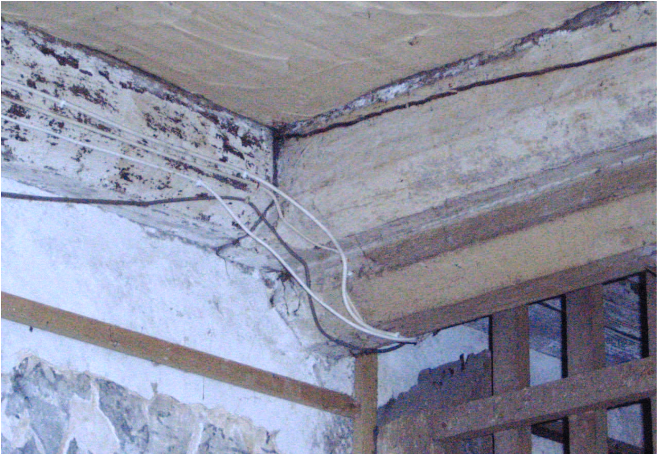
Plate 13: Transverse beam and wall plate in Area 2, facing south west
