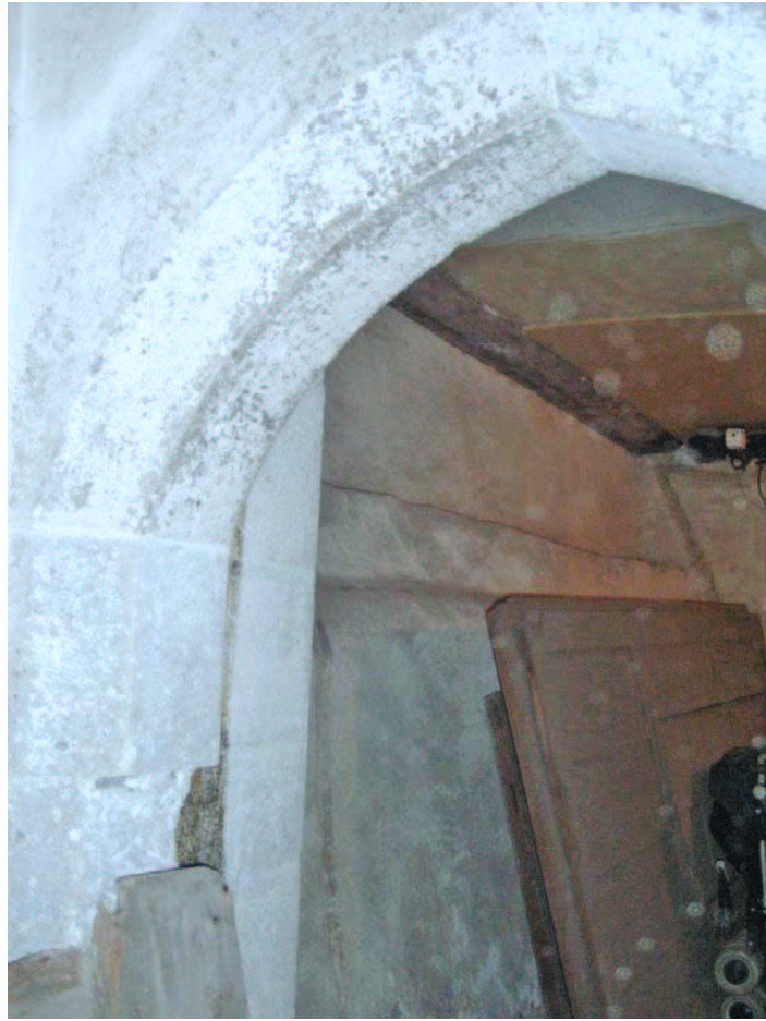
Plate 33: Chamfer on doorway in east wall of Area 4, facing south west
