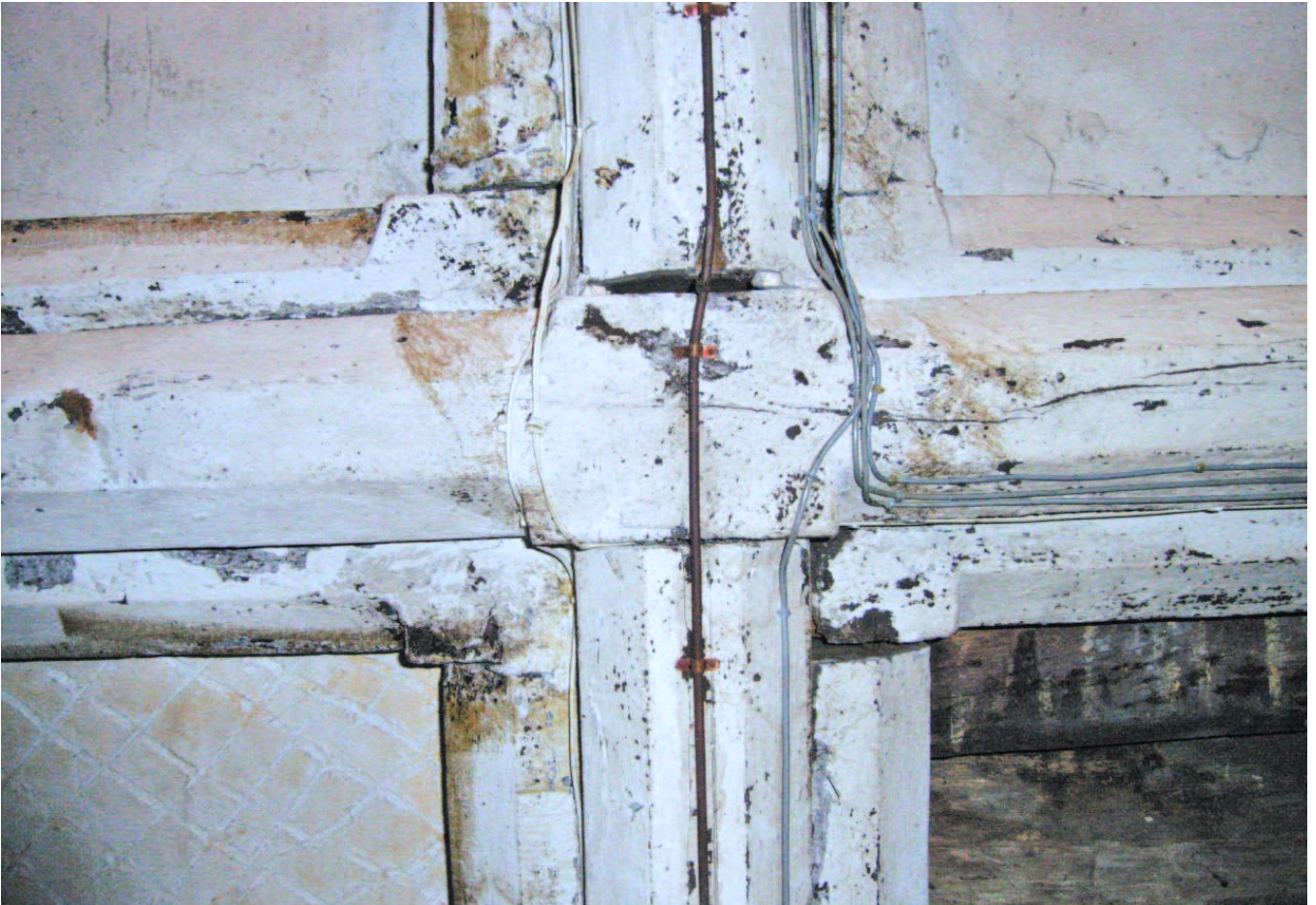
Plate 15: Applied mouldings in roof structure of Area 2
