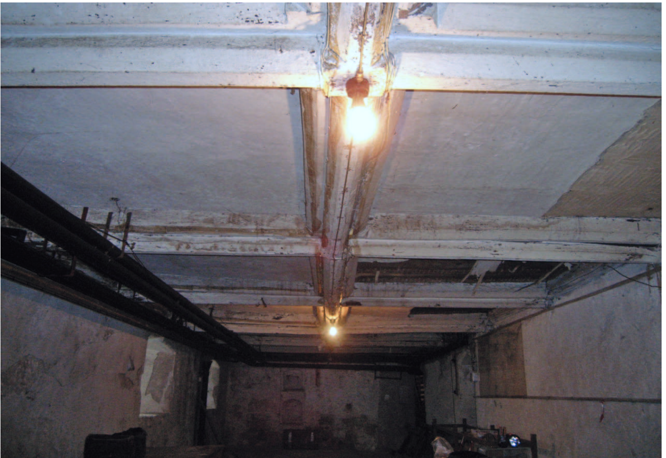
Plate 12: Roof Structure in Area 2, facing west
