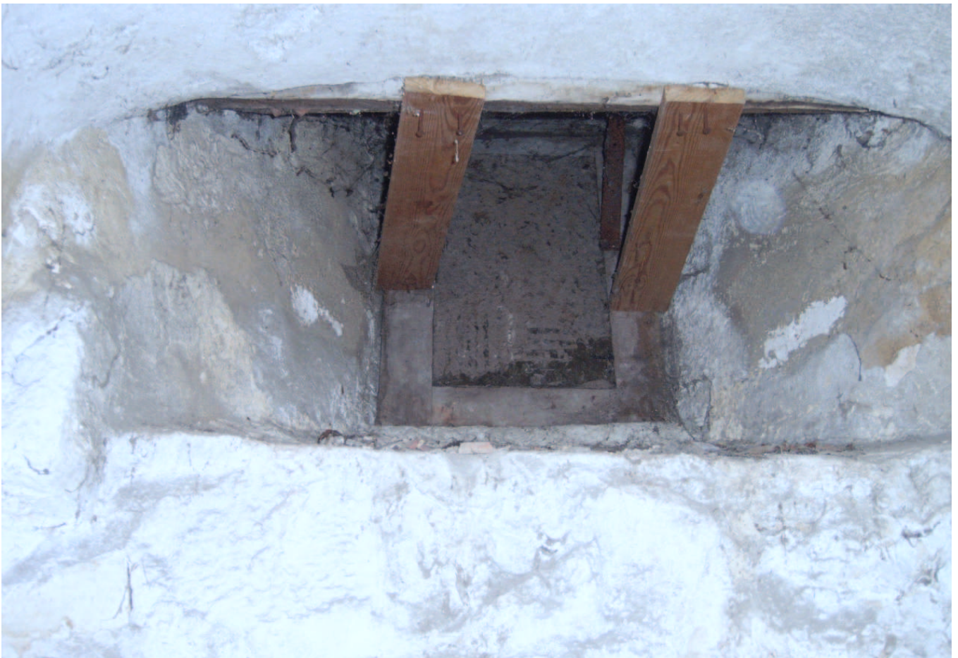
Plate 34: Blocked window at the end of passage in Area 4, facing east
