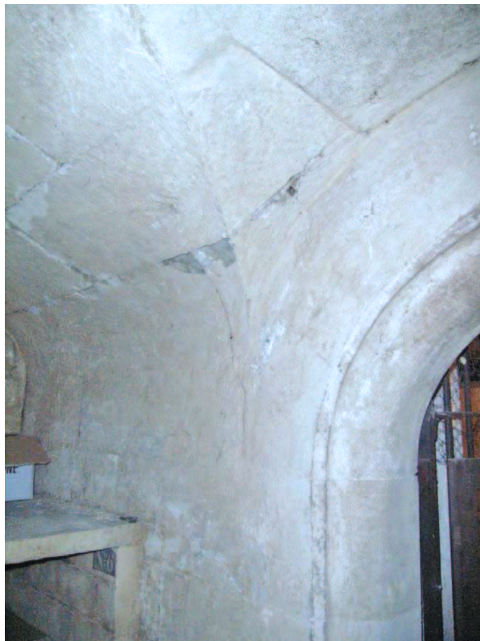
Plate 20: Vaulted roof of Wine Cellar
