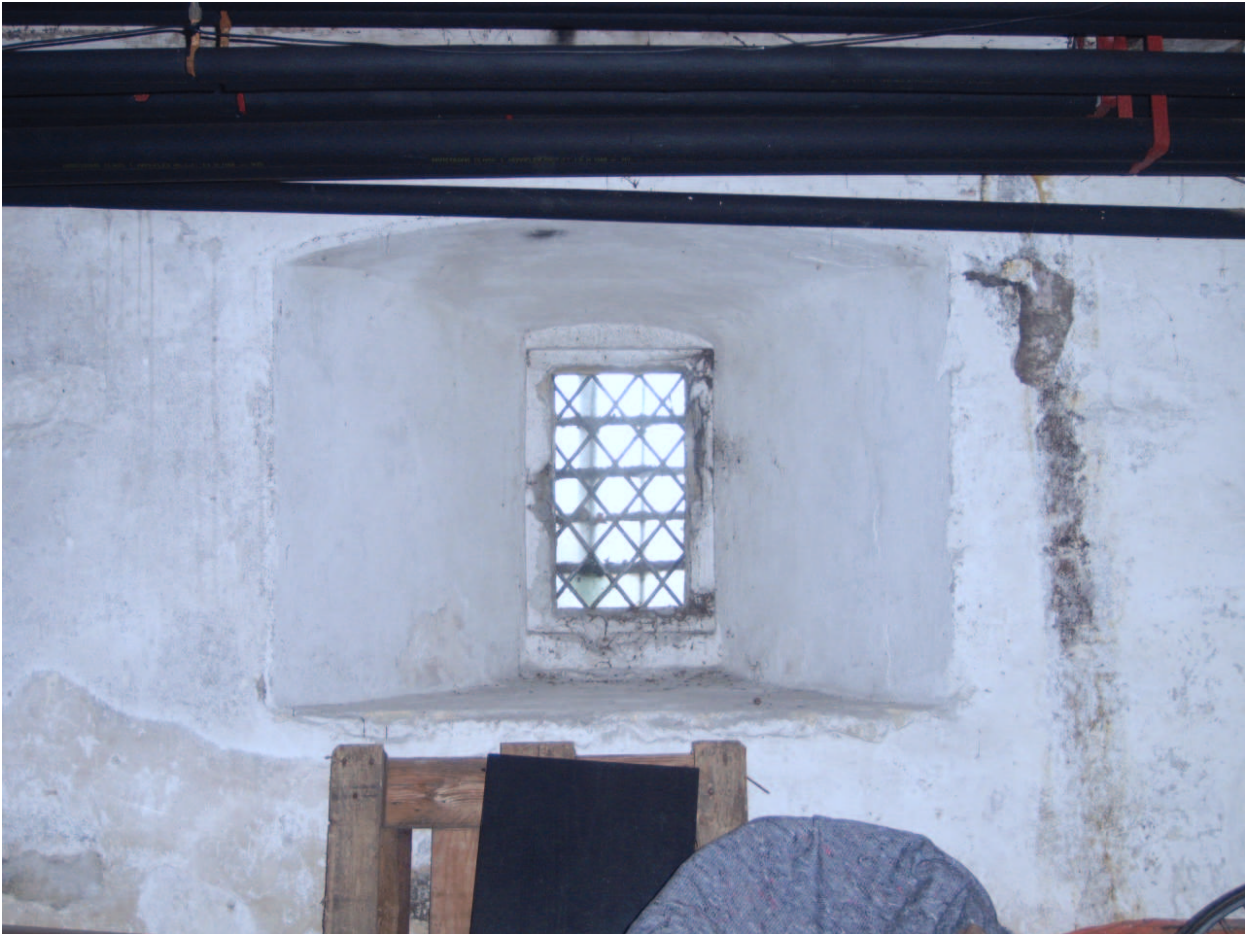
Plate 25: Window in north wall of Area 3
