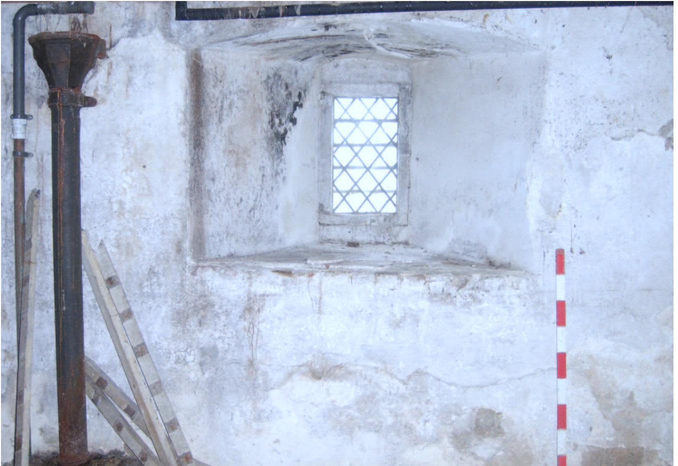
Plate 9: Window in North wall of Area 2
