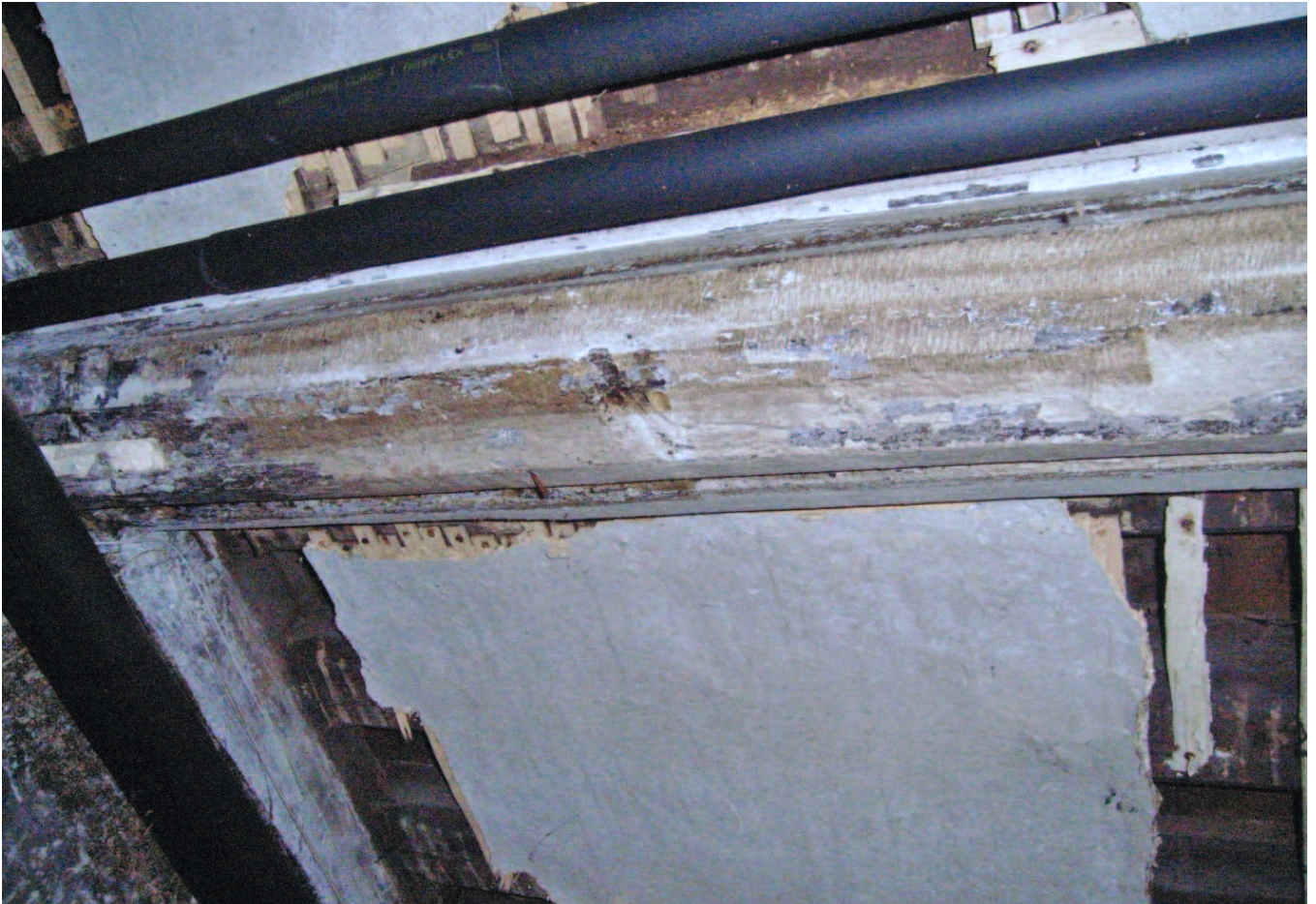
Plate 17: Transverse Beam 1 in Bay 1 of Area 2
