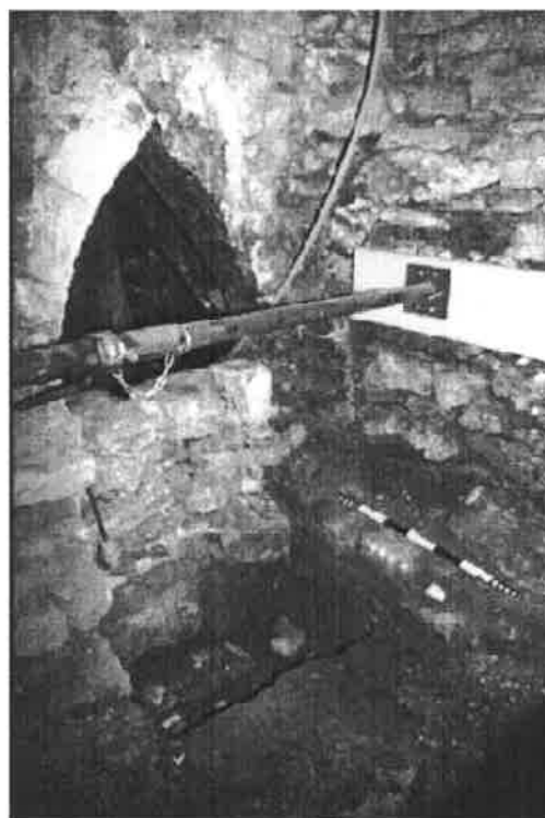
PLATE 5: Blocked archway leading to undercroft
