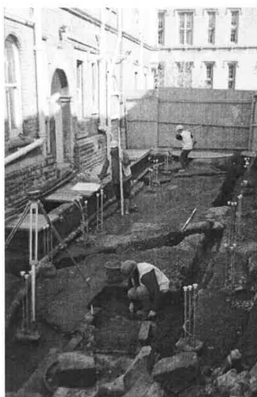
PLATE 6: Excavation of the new linking range footprint to the north of the NE chancel aisle.
