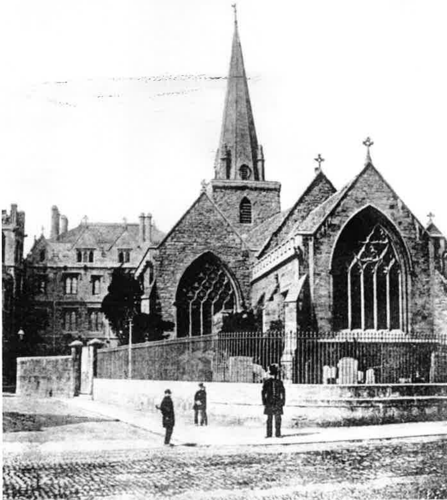
(a) c.1861; note West Family mortuary chapel at east end of south aisle
