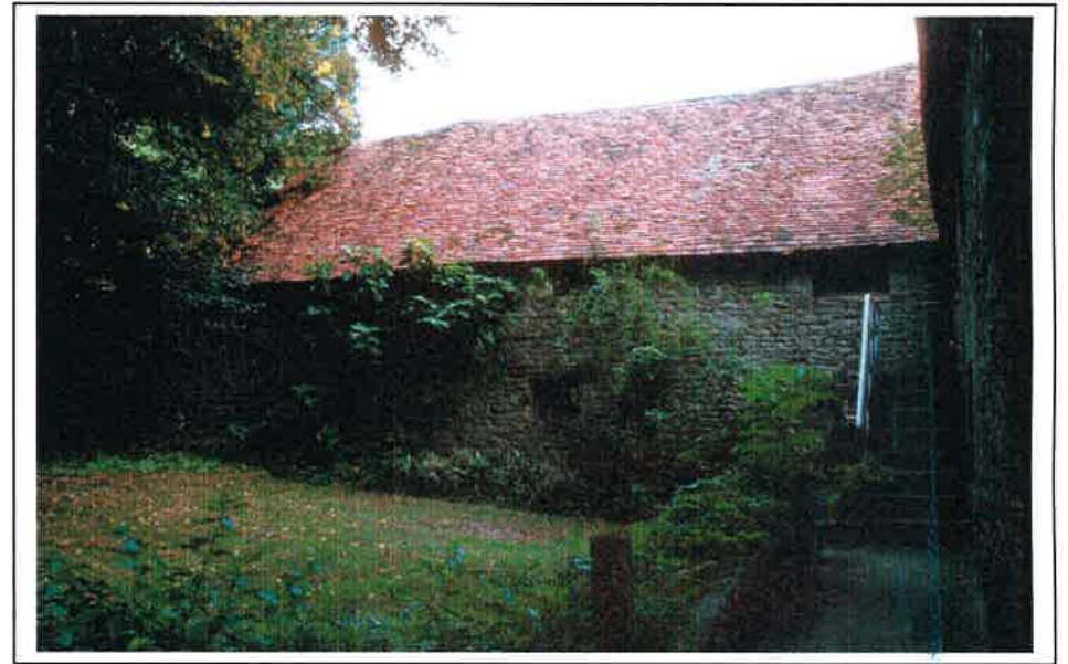
Plate 2: West elevation of 'Brewhouse'
