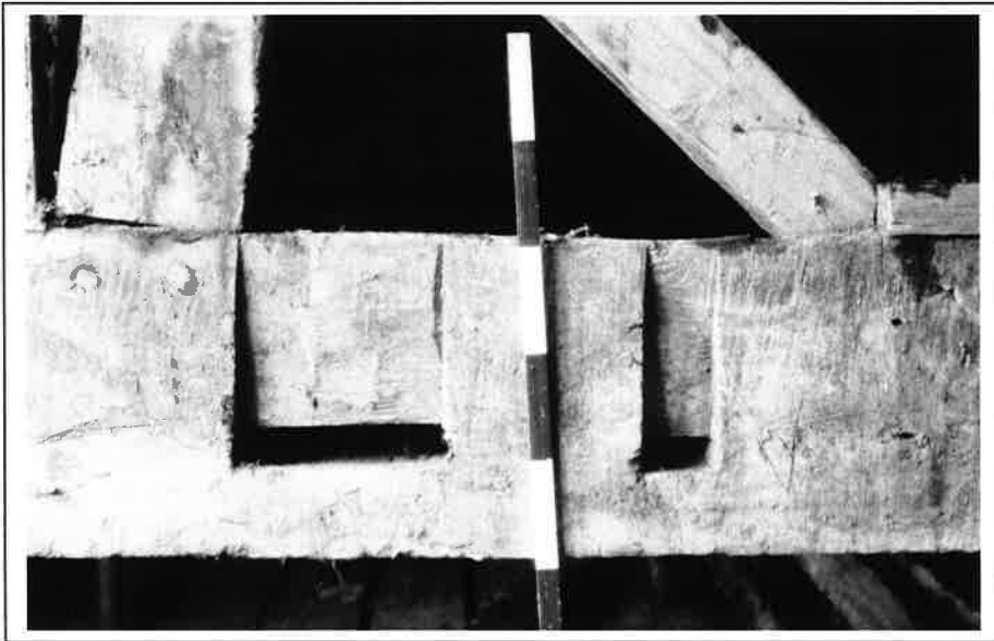
Plate 17: Detail of joist sockets in north face of truss 3, immediately to west of eastern queen strut.
