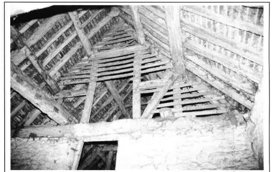
Plate 14: South face of truss 6 (formerly north end of building)
