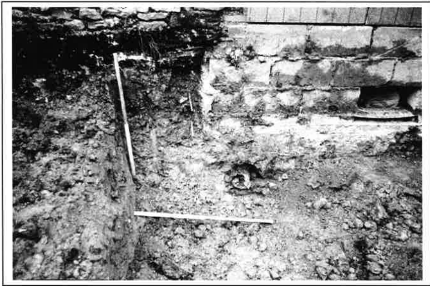
Plate 25: footings exposed beneath east wall of brewhouse
