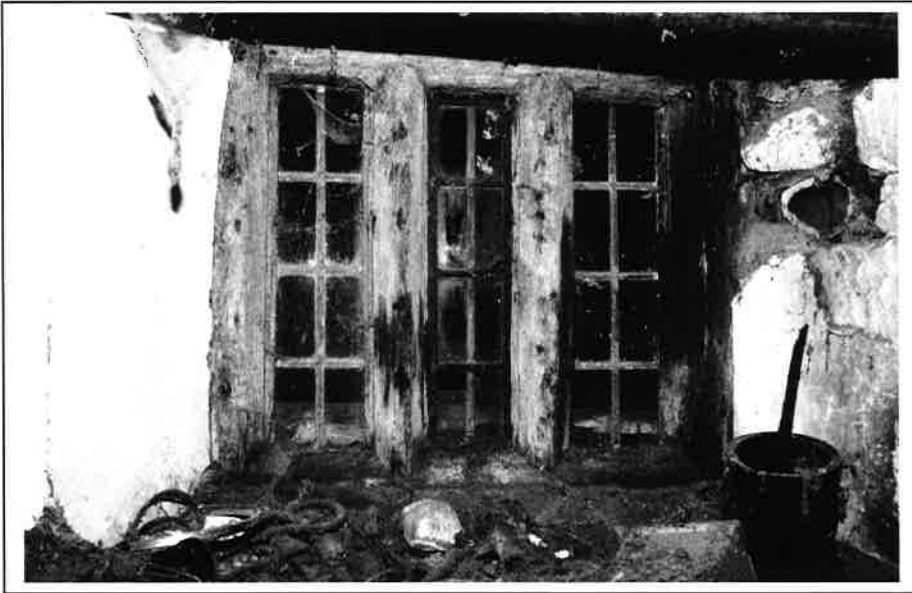
Plate 9: Reused lower centre window in west wall of 'brewhouse'. with high quality joinery
