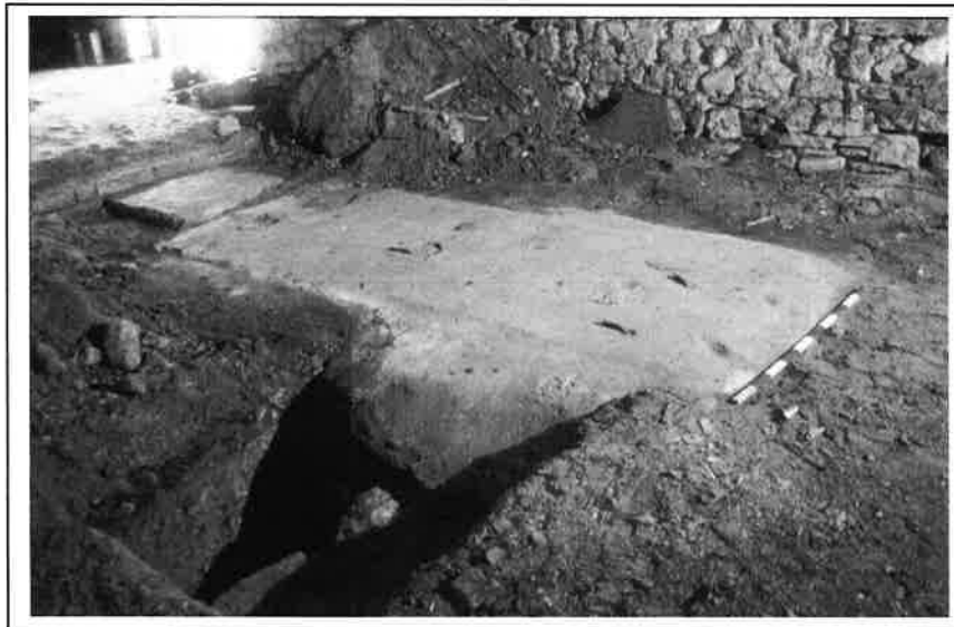
Plate 23: Gas plant foundation towards centre of 'Brewhouse'
