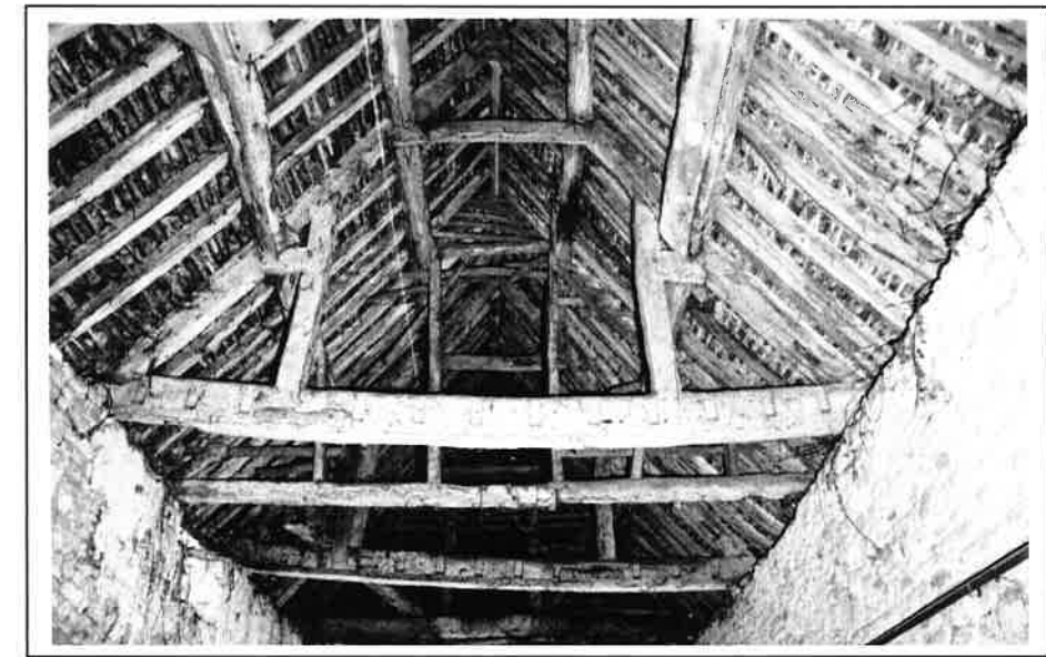
Plate 16: North face of truss 5
