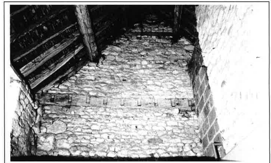
Plate 12: South wall of 'brewhouse showing tie-beam embedded in stone gable
