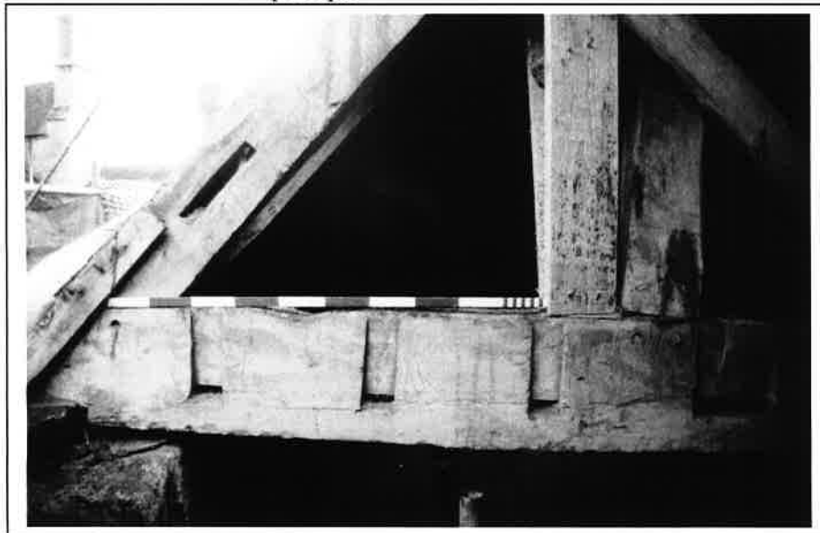
Plate 19: East end of north face of truss 3 showing empty mortice of former wind-brace in principal rafter
