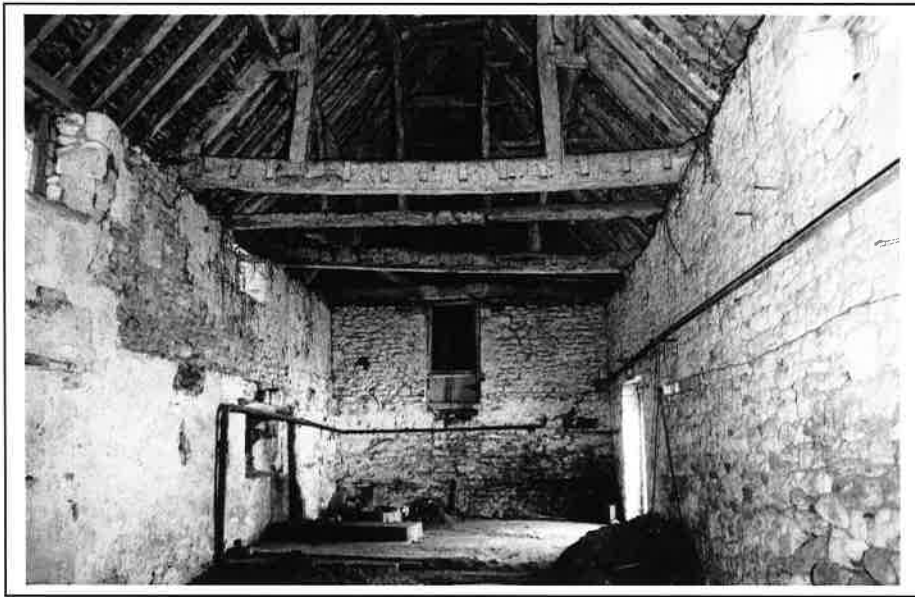
Plate 5: General view within 'brewhouse' towards north.
