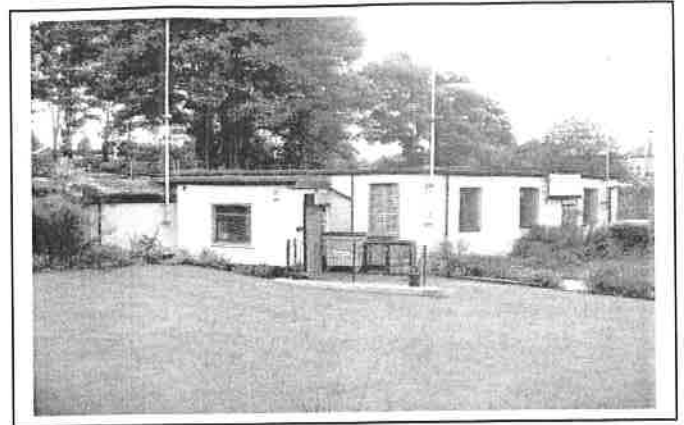
Plate 6: Former mill viewed from north-east
