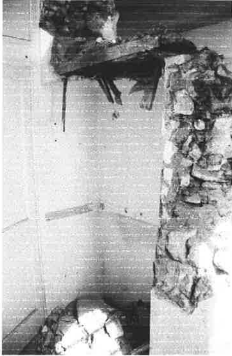
Plate 7: Blocked doorway in former Scouts room at east end of south range
