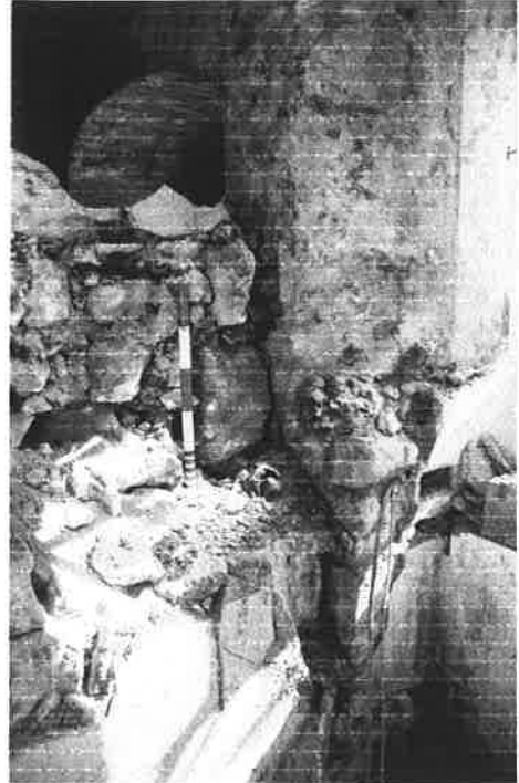
Plate 8: Straight joint between external ashlar construction and rubble internal partition wall, location as Plate 7
