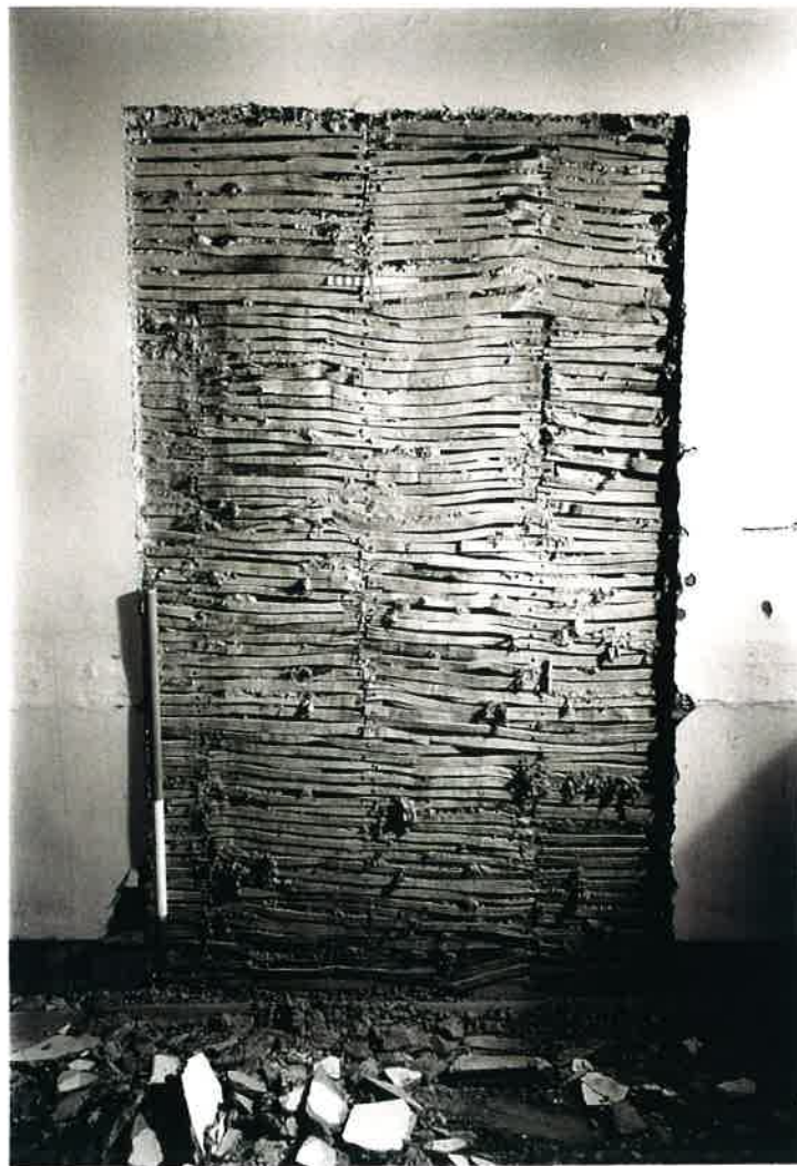
Plate 2: East side - Lath and stud base for plaster surface
