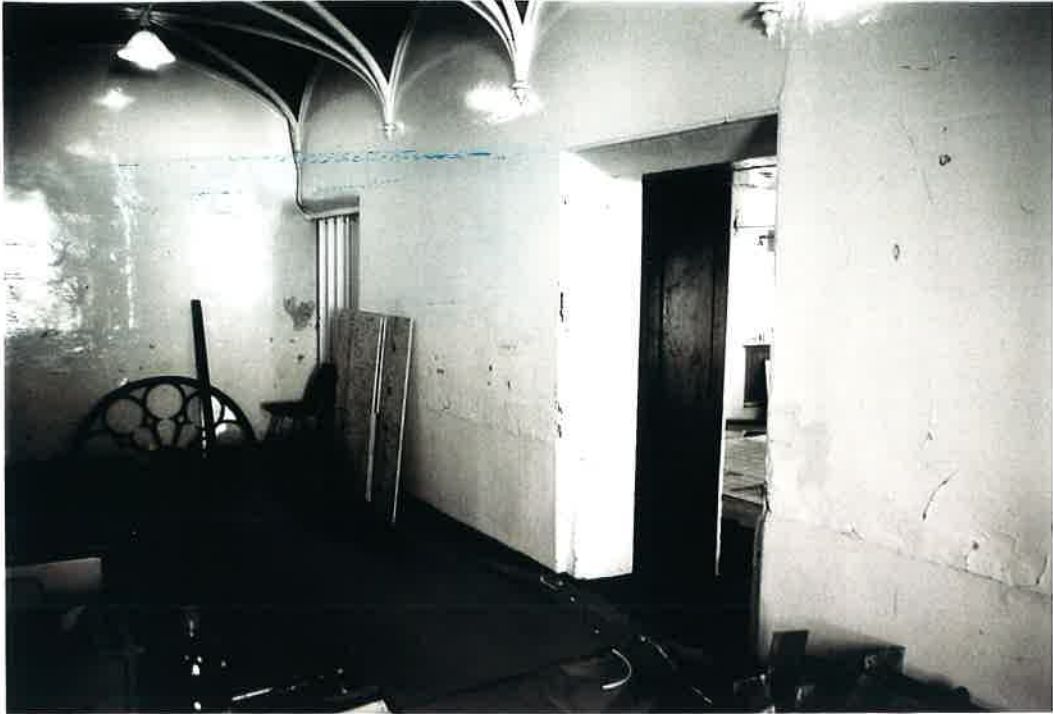
Plate 1: Screens Passage: existing doorway and area of investigation
