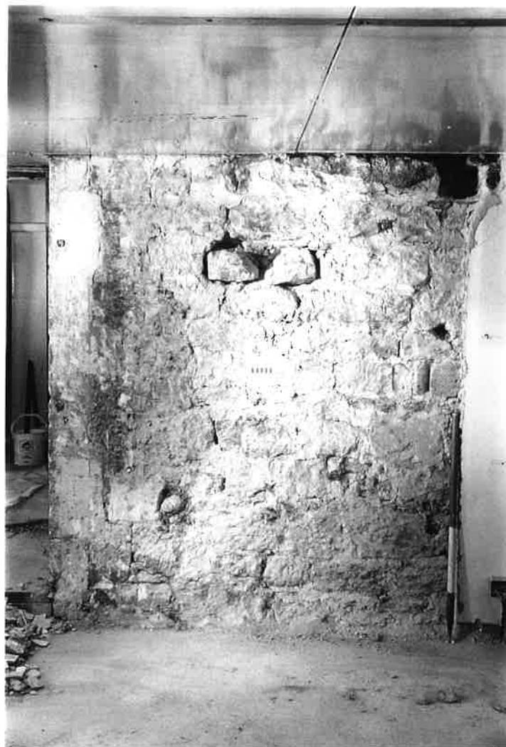
Plate 7: West side - Coursed rubble wall surface
