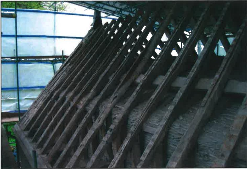
Plate 19: North slope of roof above chancel
