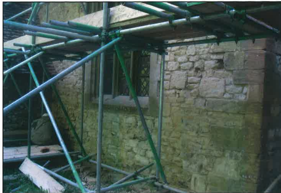
Plate 12: Rebuilt wall at north-west corner of nave
