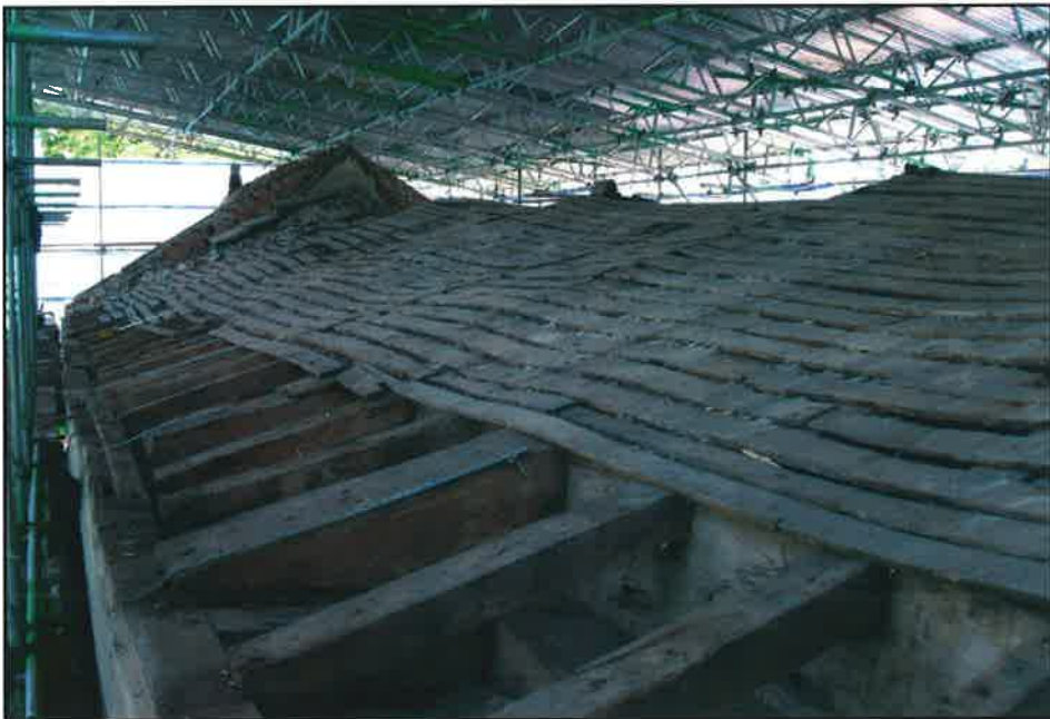
Plate 21: Roof above nave from west
