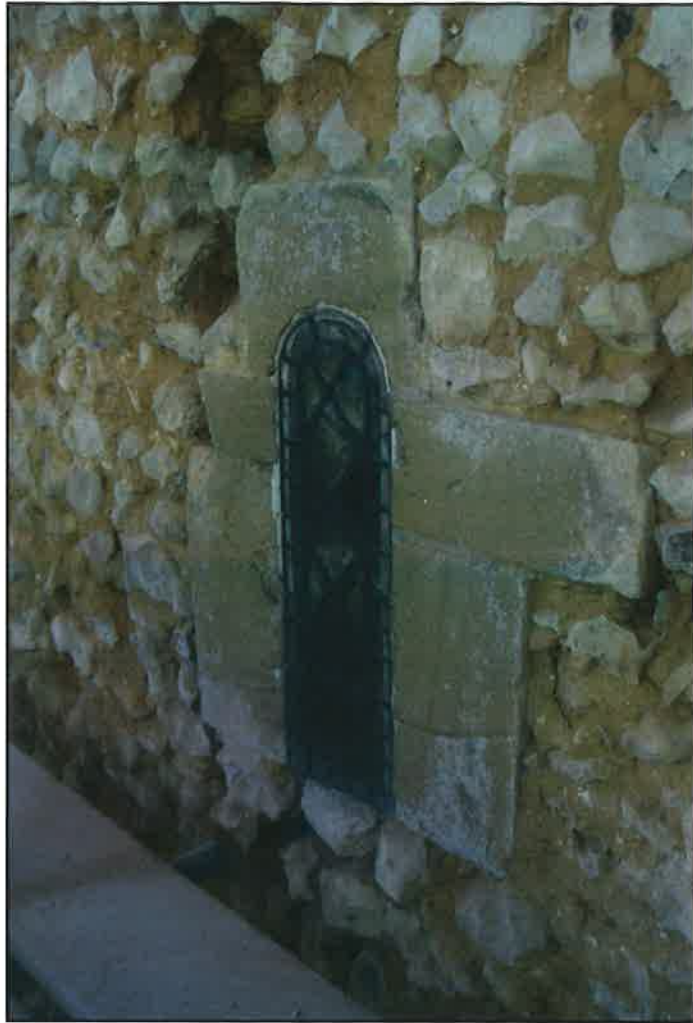
Plate 7: Primary window in north wall of chancel after render removal
