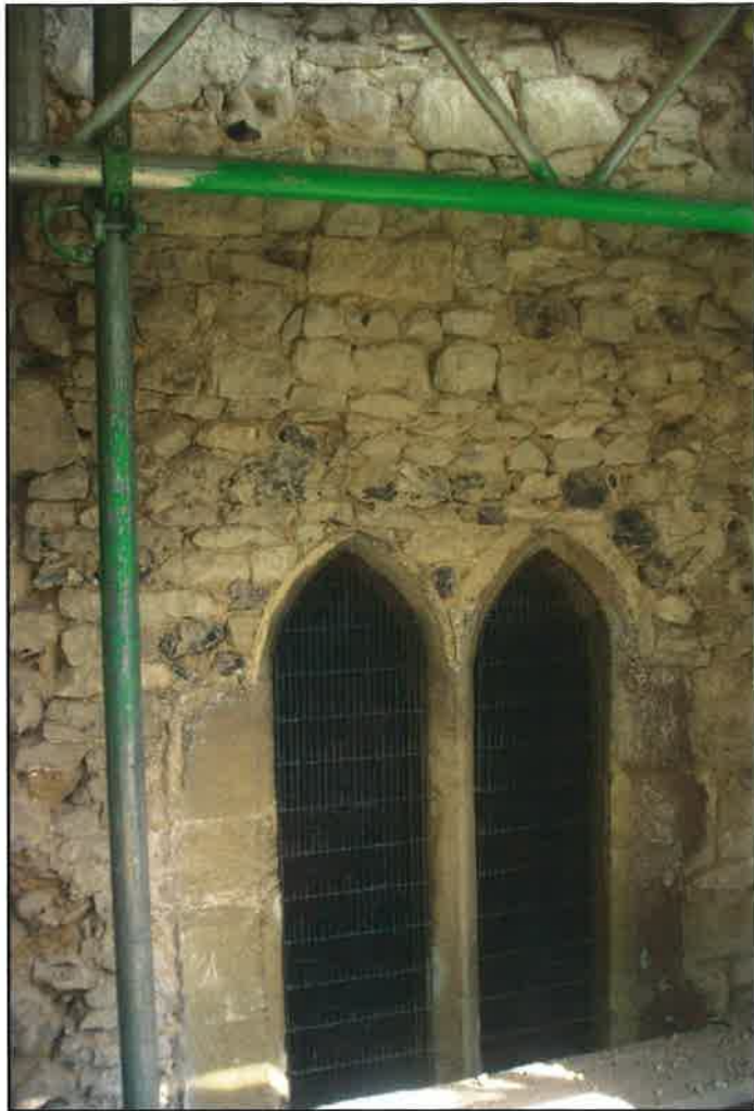
Plate 13: Inserted window in south wall of chancel
