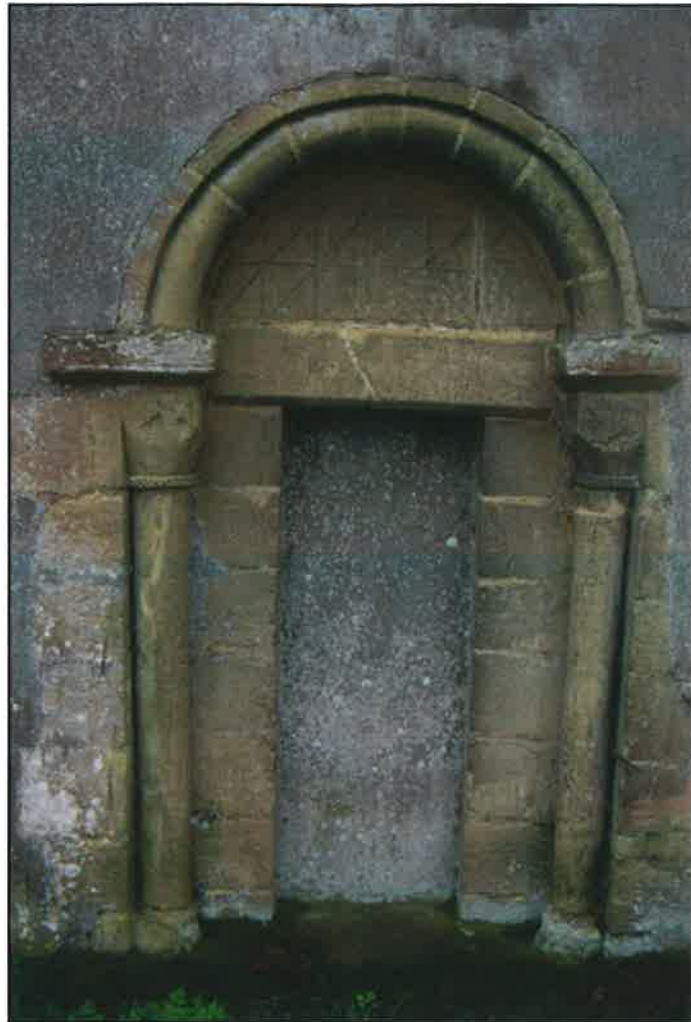
Plate 5: Primary 12th-century door in north wall of chancel
