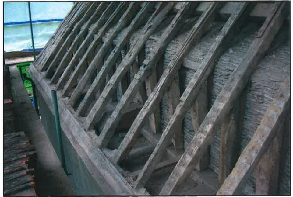
Plate 20: North slope of roof above chancel
