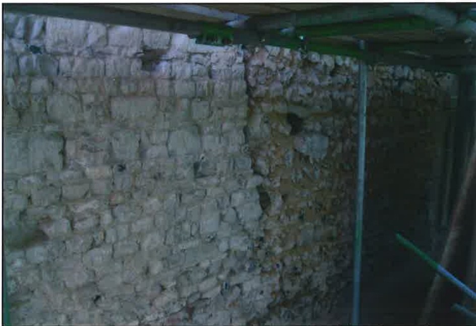
Plate 9: North wall of chancel showing primary wall to right and extension to left
