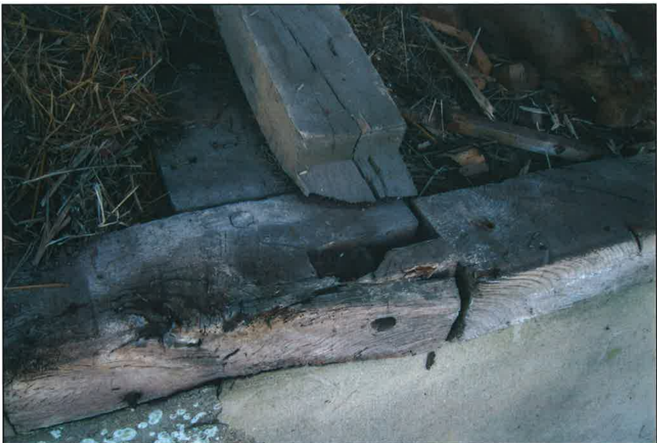
Plate 24: Scarf joint in wall plate on north side of nave
