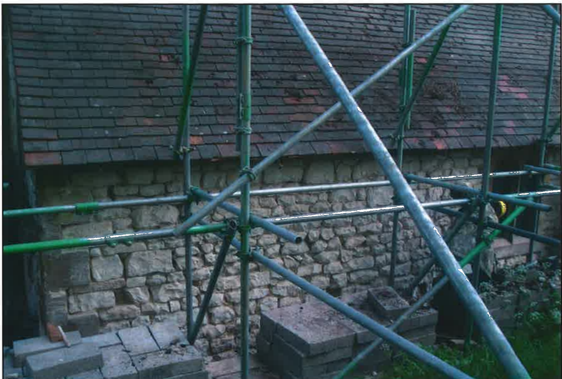
Plate 14: South wall of 19th-century south aisle
