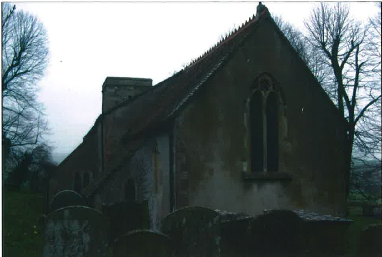
Plate 2: View from the east before the start of works
