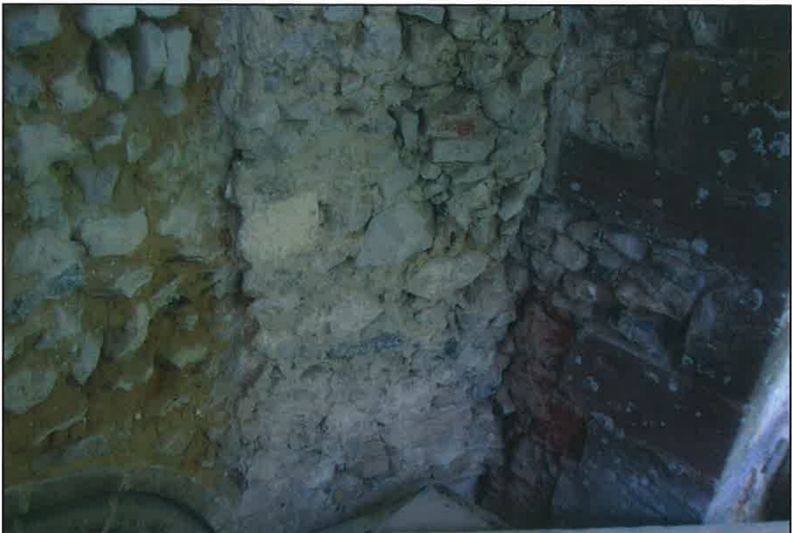
Plate 8: Patching at west end of chancel adjacent to nave
