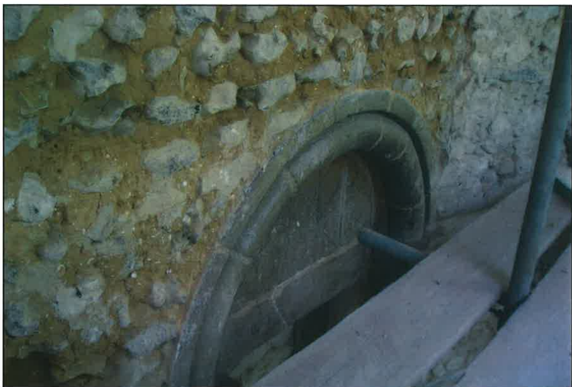
Plate 6: Arch over door after removal of cement render
