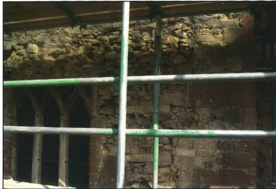
Plate 10: Partially rebuilt south wall of nave
