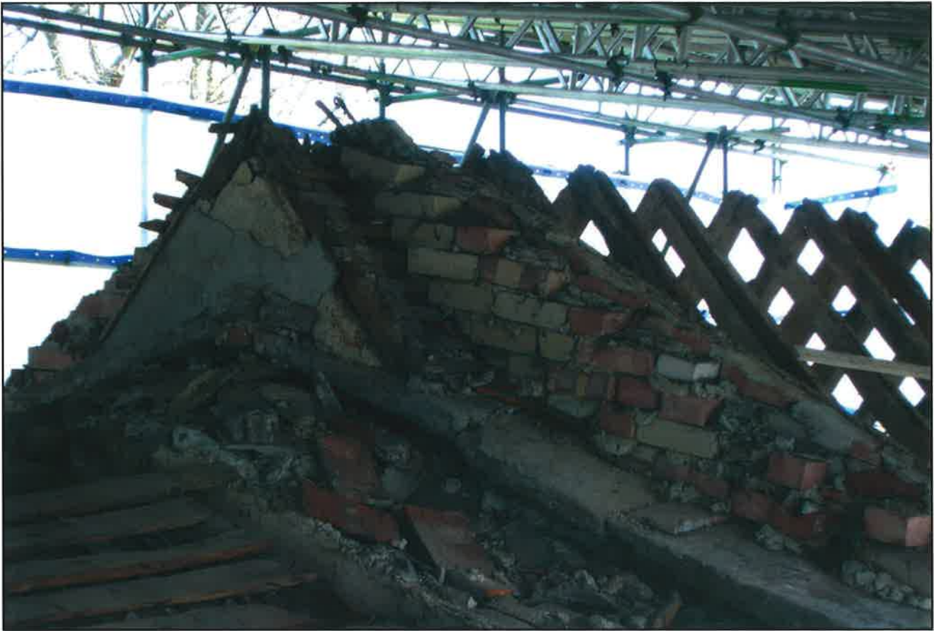
Plate 23: East end of nave roof at junction with chancel
