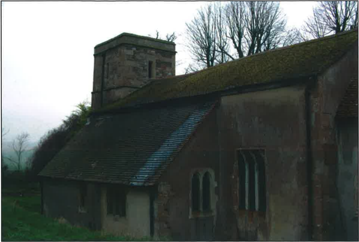
Plate 1: The church from the south-east before the start of works
