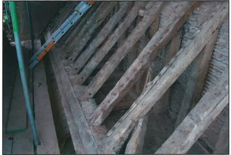
Plate 18: Feet of rafters in roof above chancel
