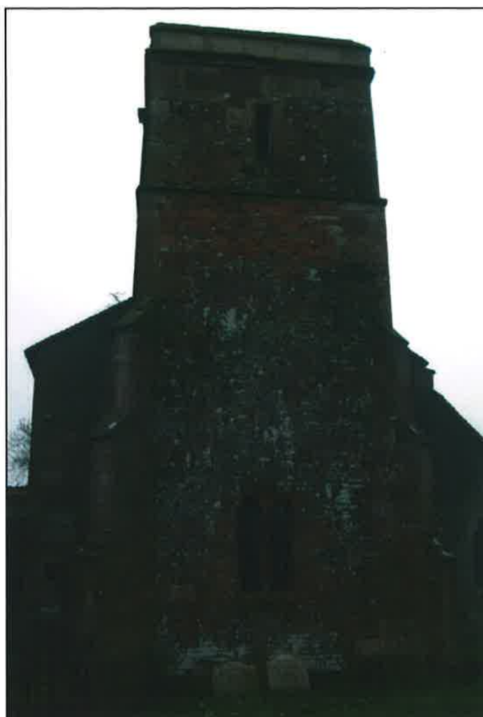
Plate 4: Tower at west end before the start of works
