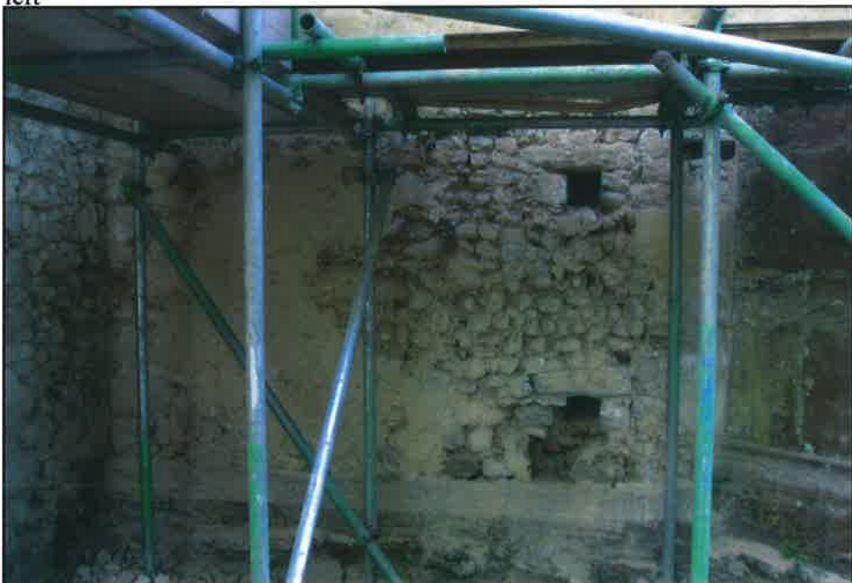
Plate 11: North wall of tower showing put-log holes
