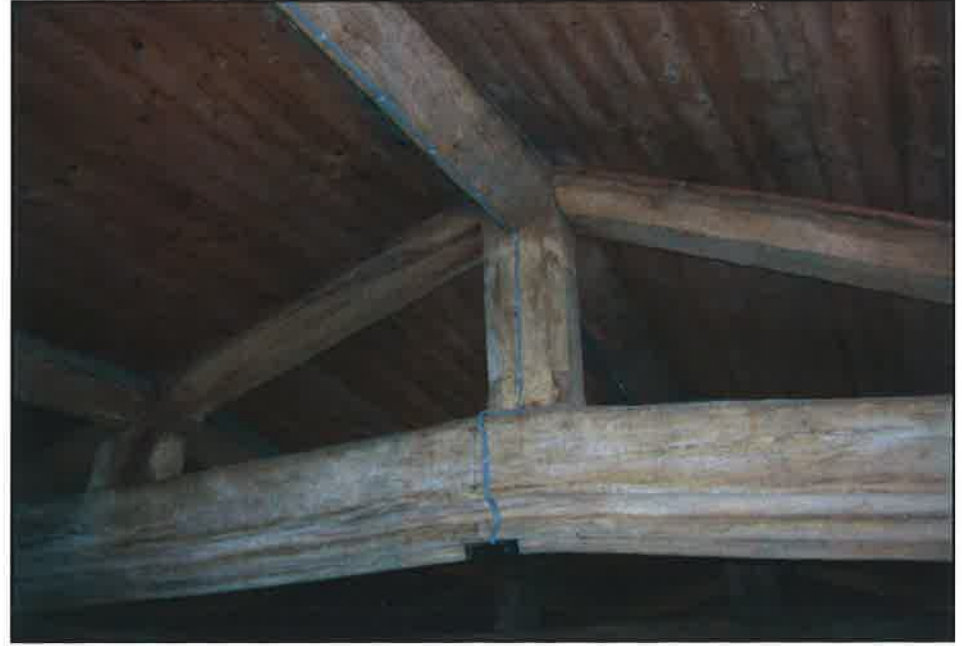
Plate 16: Roof truss above nave (possibly 17th century)
