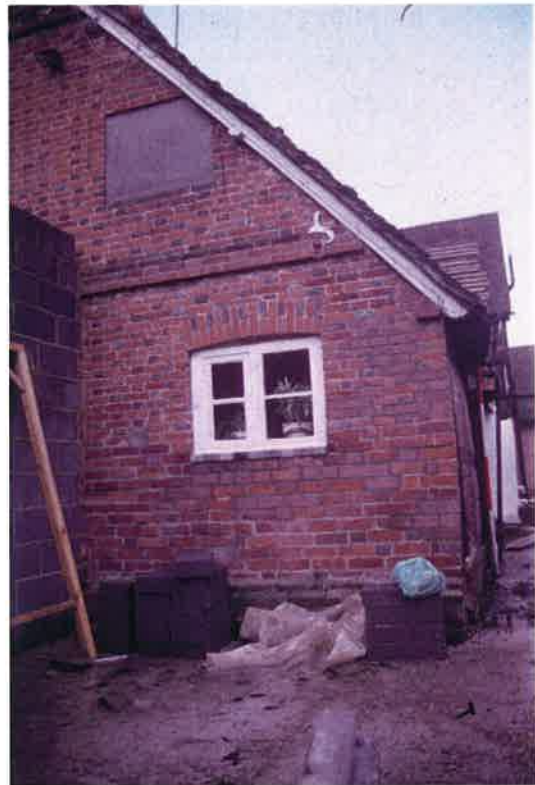
Plate 3 External Side Wall
