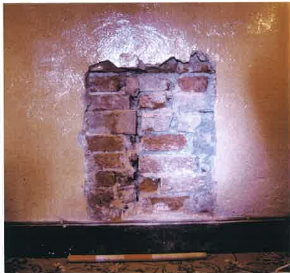
Plate 1 Internal Wall Plaster Removal
